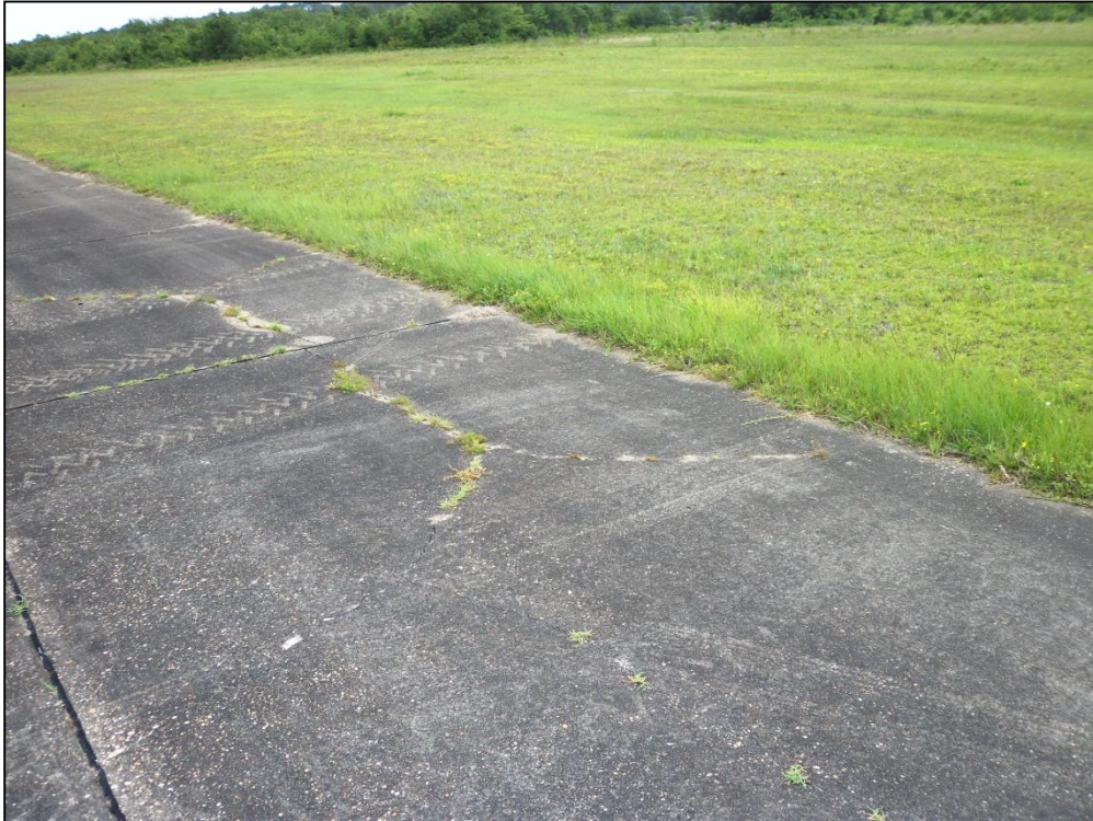
Runway 16-36, Section 6310, Sample Unit 544 – Medium Severity (65) Joint Seal Damage, Low Severity (72) Shattered Slab
