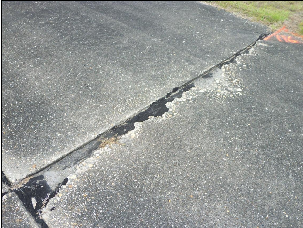
Runway 16-36, Section 6310, Sample Unit 116 – High Severity (74) Joint Spalling, Medium Severity (65) Joint Seal Damage
