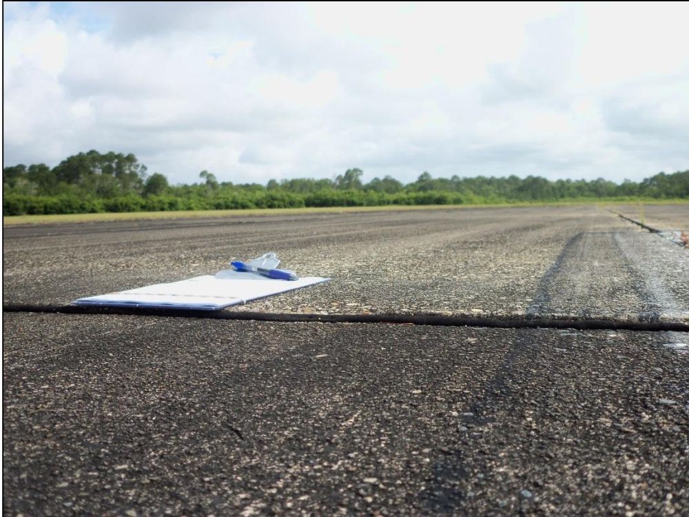
Runway 18-36, Section 6305, Sample Unit 374 –Low Severity (71) Settlement or Faulting
