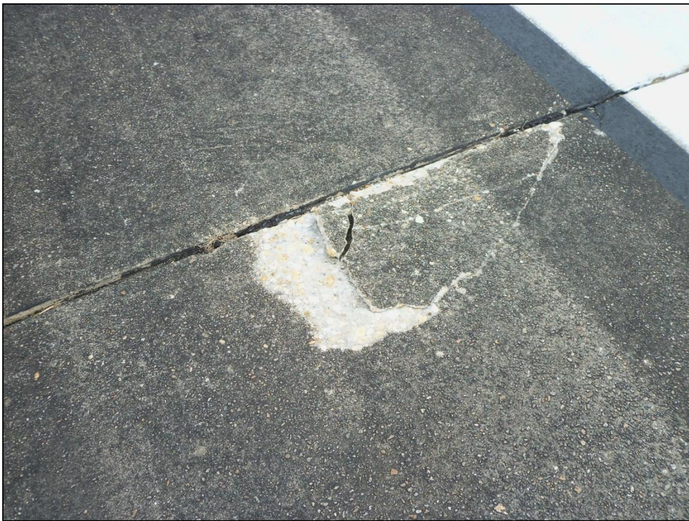
Runway 14-32, Section 6110, Sample Unit 548 -High Severity (74) Joint Spalling, Medium Severity (65) Joint Seal Damage
