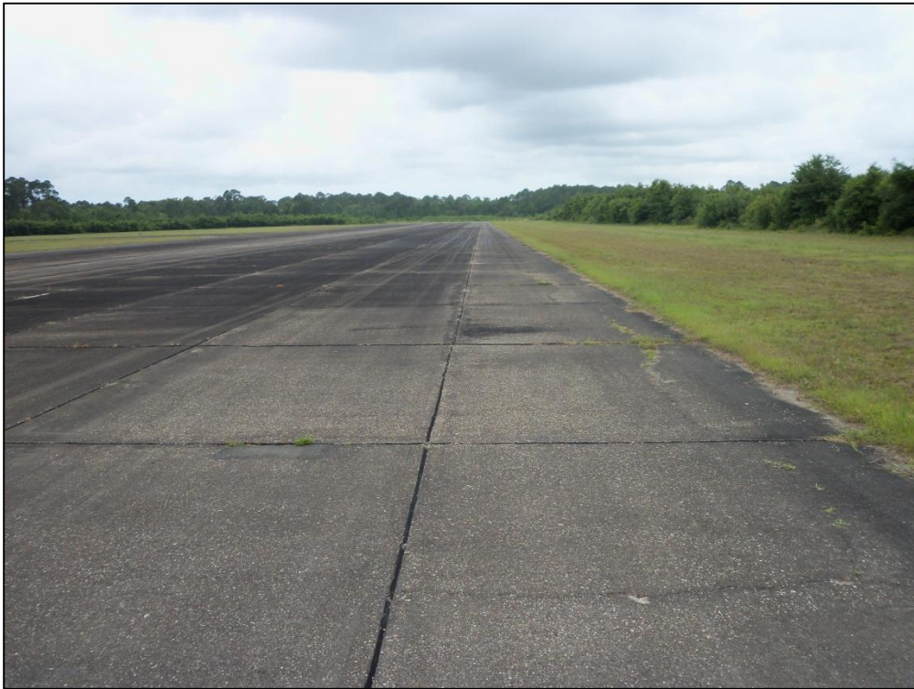
Runway 18-36, Section 6310, Sample Unit 564 –Low Severity (66) Small Patching, Medium Severity (65) Joint Seal Damage, Low Severity (63) Longitudinal, Transverse and Diagonal Cracking, Shrinkage Cracks (73)
