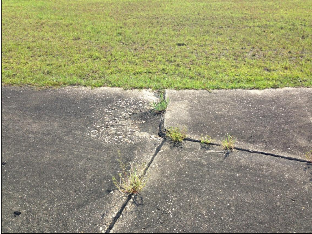
Taxiway C, Section 105, Sample Unit 129 – Medium Severity (65) Joint Seal Damage, High Severity (75) Corner Spalling
