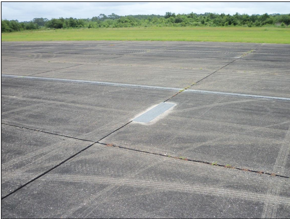
Runway 18-36, Section 6305, Sample Unit 344 – Medium Severity (65) Joint Seal Damage, Low Severity (66) Small Patching
