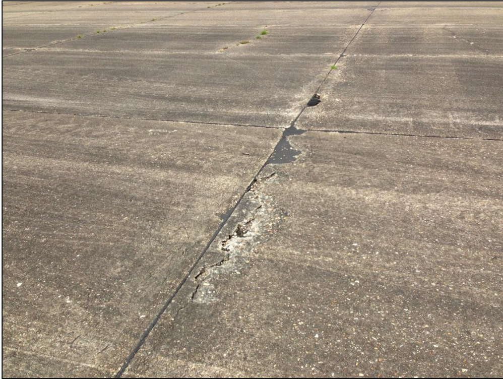
Apron, Section 4105, Sample Unit 210 – Low Severity (63) Longitudinal, Transverse, and Diagonal Cracking, Low and Medium Severity (74) Joint Spalling, Low Severity (75) Corner Spalling
