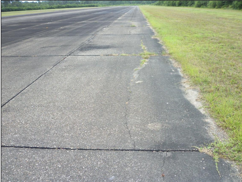
Runway 18-36, Section 6310, Sample Unit 564 – Medium Severity (65) Joint Seal Damage, Low Severity (63) Longitudinal, Transverse and Diagonal Cracking
