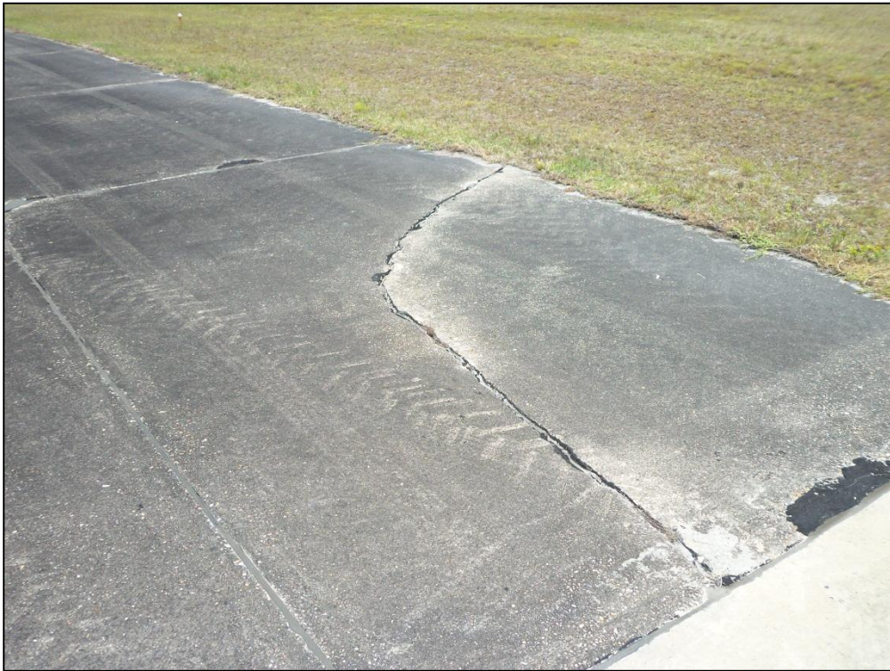
Runway 6-24, Section 6210, Sample Unit 540 – Low Severity (74) Joint Spalling, Medium Severity (63) Longitudinal, Transverse, and Diagonal Cracking
