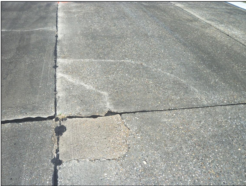
Runway 14-32, Section 6110, Sample Unit 504 –Low Severity (63) Longitudinal, Transverse, and Diagonal Cracking, Low Severity (62) Corner Break, Low Severity (70) Scaling, Map Cracking, and Cracking, Medium Severity (66) Small Patching, Medium Severity (65) Joint Seal Damage
