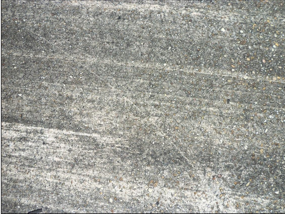
Runway 6-24, Section 6205, Sample Unit 312 – Low Severity (70) Scaling, Map Cracking, Crazing
