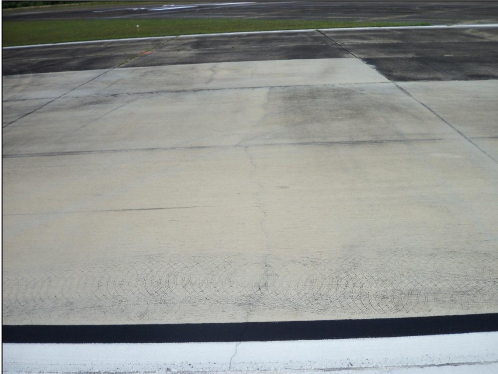
Runway 14-32, Section 6105, Sample Unit 301 – Low Severity (63) Longitudinal, Transverse, and Diagonal Cracking
