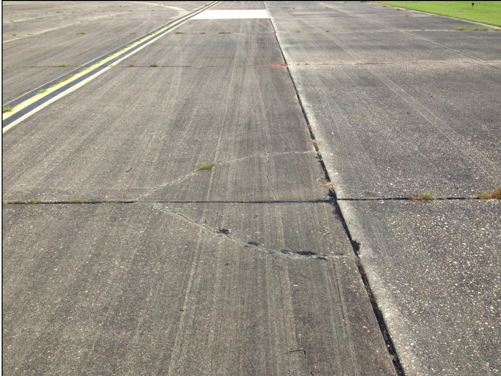
Taxiway A5, Section 205, Sample Unit 101 – Medium Severity (65) Joint Seal Damage, Low Severity (62) Corner Break, Low Severity (70) Scaling, Map Cracking, Crazing
