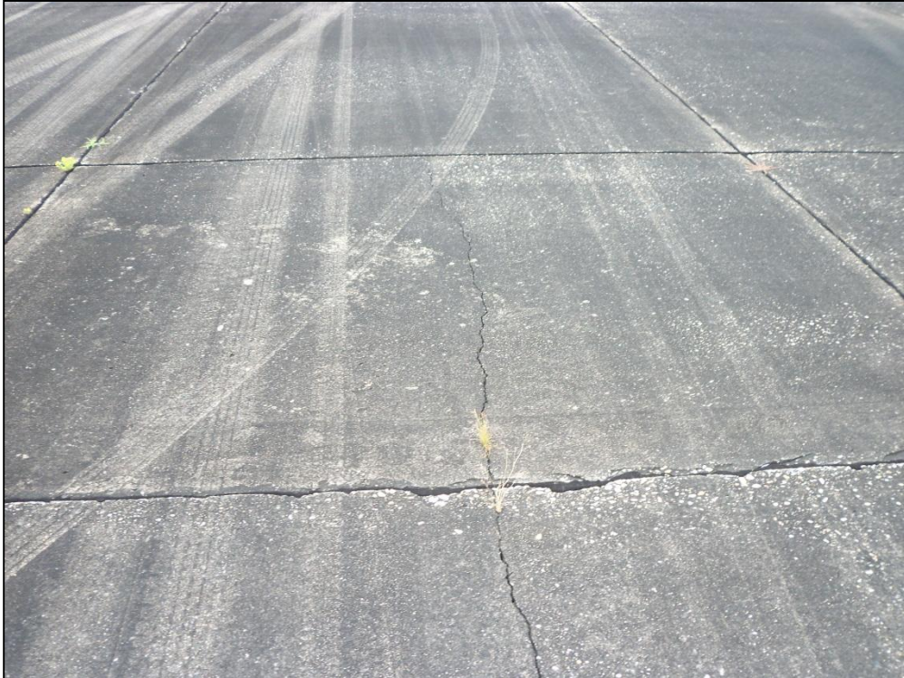
Runway 18-36, Section 6305, Sample Unit 350 – Medium Severity (74) Joint Spalling, Medium Severity (65) Joint Seal Damage, Low Severity (63) Longitudinal, Transverse and Diagonal Cracking
