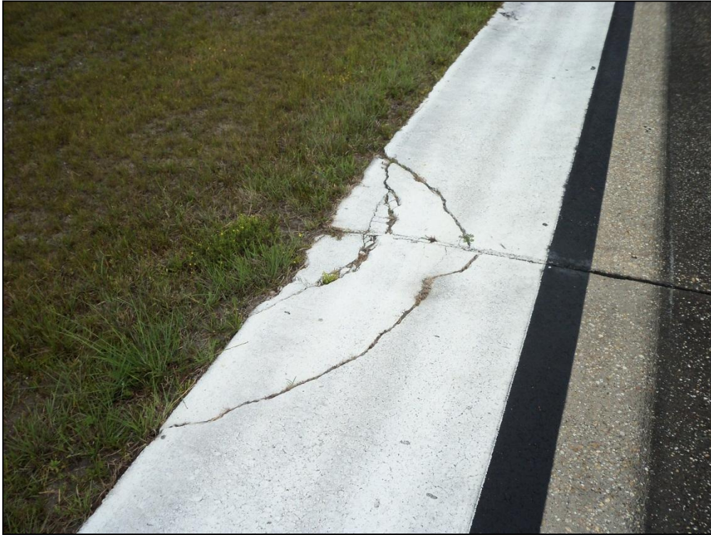
Runway 14-32, Section 6110, Sample Unit 104 -Medium Severity (62) Corner Break
