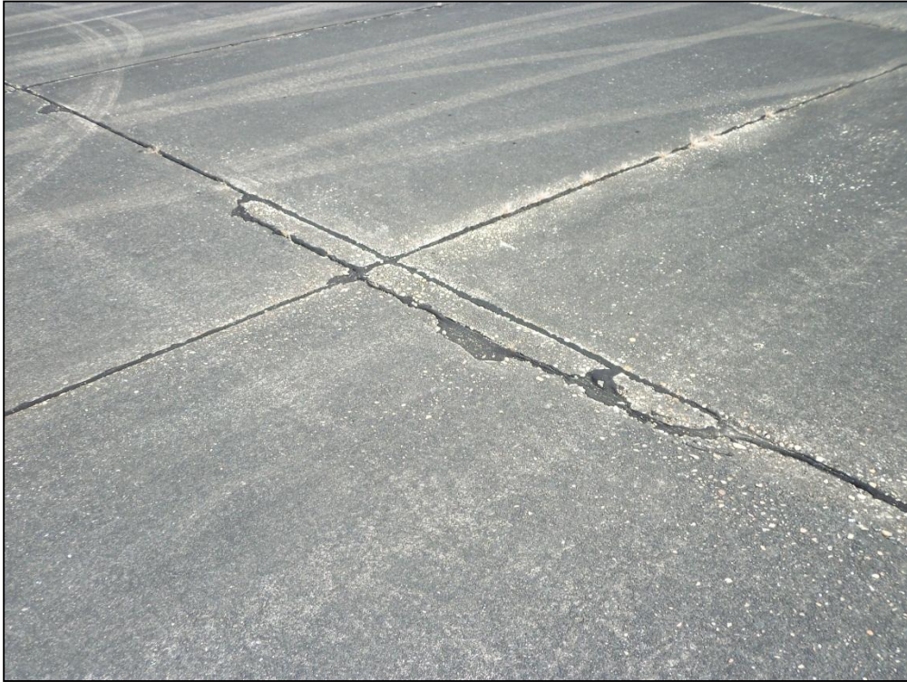
Runway 18-36, Section 6305, Sample Unit 374 – Low and Medium Severity (74) Joint Spalling, Medium Severity (65) Joint Seal Damage
