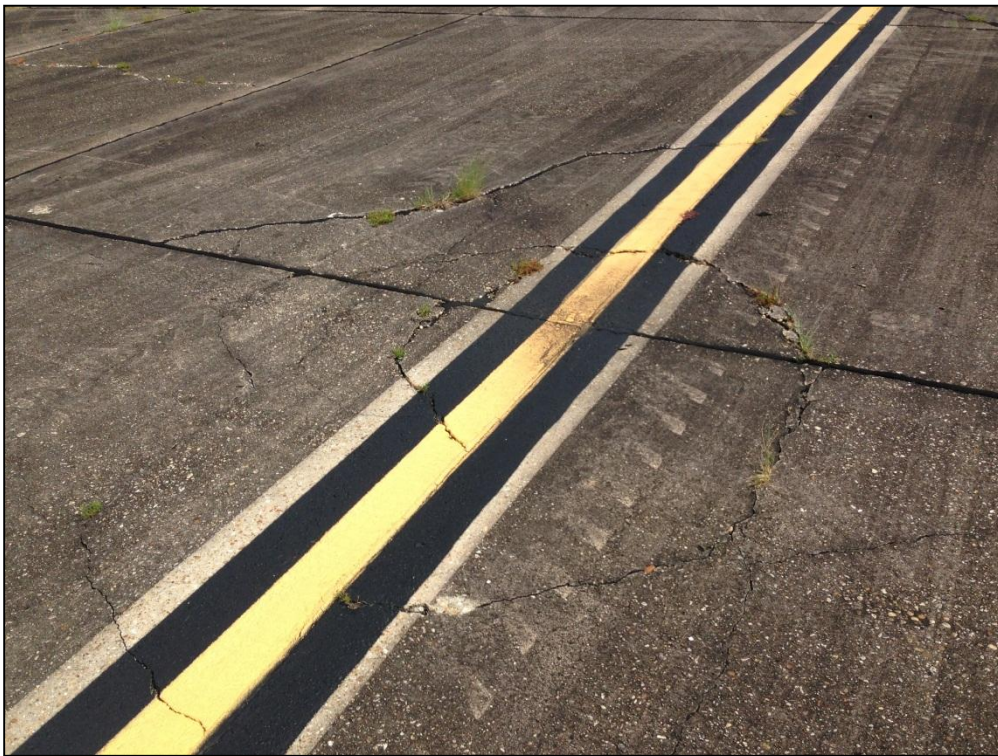
Taxiway D, Section 335, Sample Unit 103 – Low Severity (65) Joint Seal Damage, Medium Severity (63) Longitudinal, Transverse, and Diagonal Cracking, Low and Medium Severity (62) Corner Break, (73) Shrinkage Cracking
