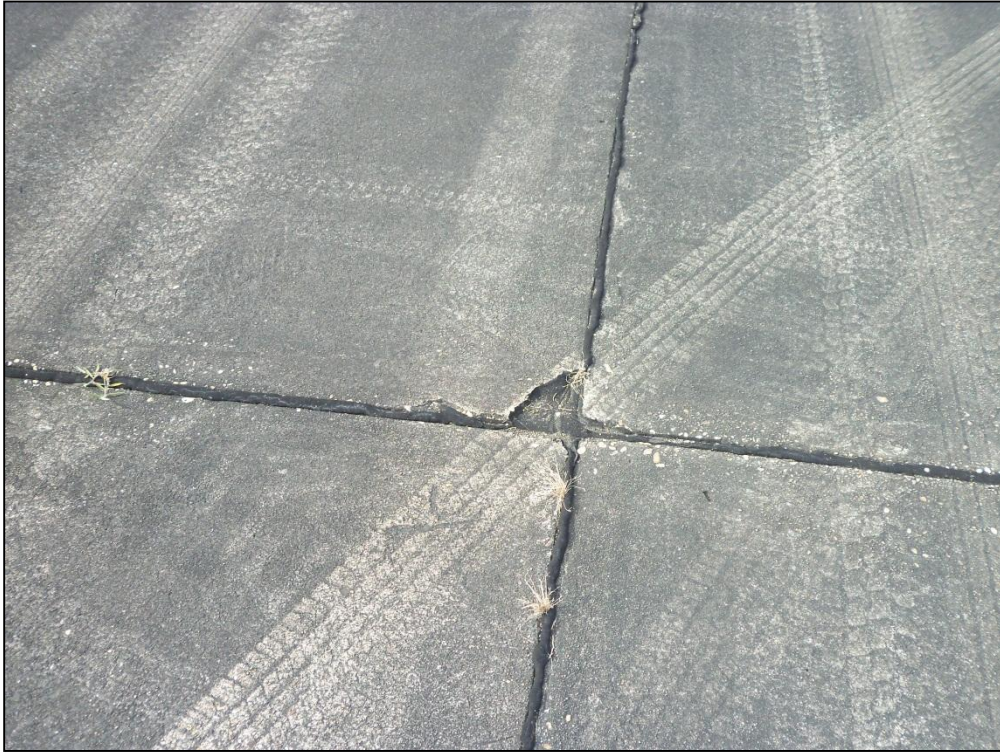
Runway 18-36, Section 6305, Sample Unit 374 –Low Severity (75) Corner Spalling, Medium Severity (65) Joint Seal Damage
