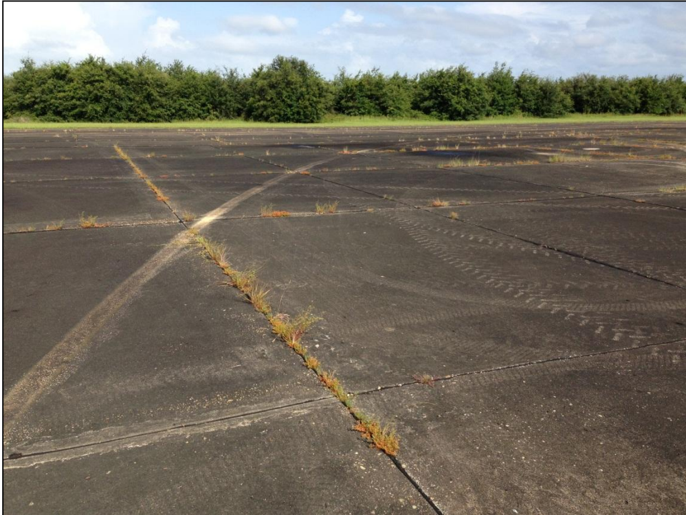
Taxiway C1, Section 160, Sample Unit 103 – Medium Severity (65) Joint Seal Damage
