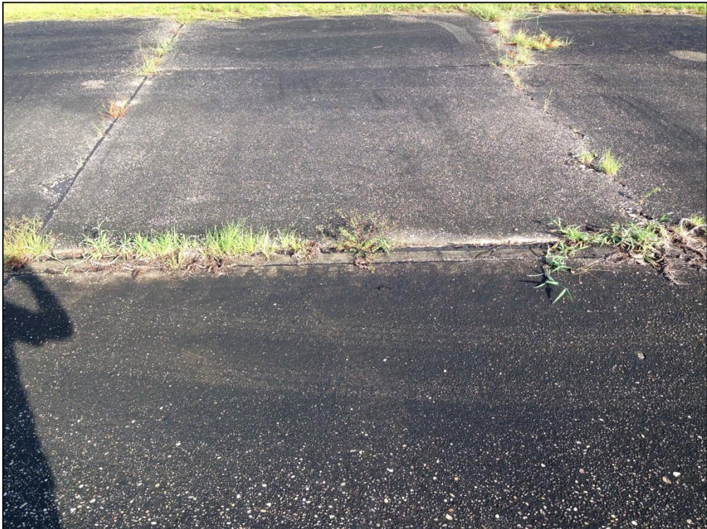
Taxiway C, Section 110, Sample Unit 206 – Medium Severity (65) Joint Seal Damage, Medium Severity (63) Longitudinal, Transverse, and Diagonal Cracking, Medium Severity (71) Faulting
