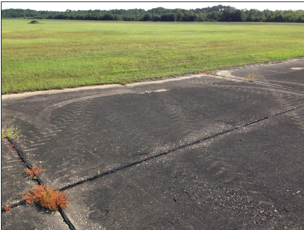
Taxiway C1, Section 160, Sample Unit 103 – Medium Severity (65) Joint Seal Damage, Low Severity (63) Longitudinal, Transverse, and Diagonal Cracking
