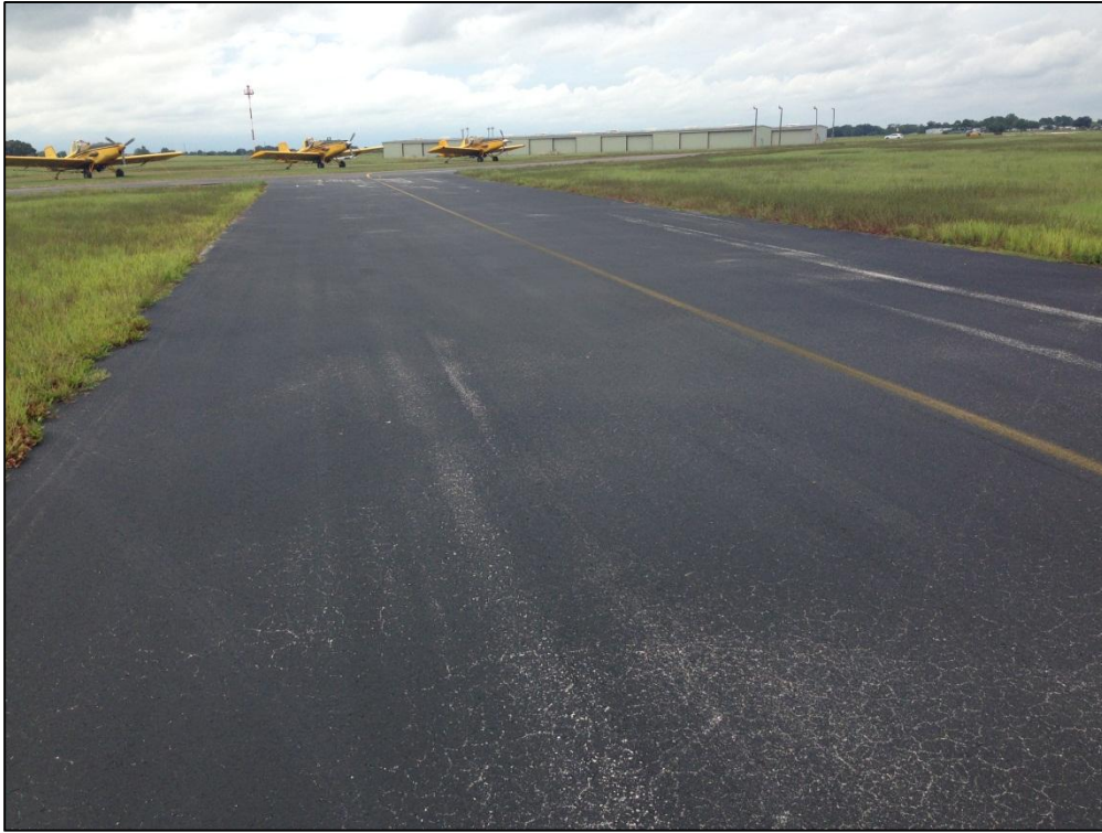
Taxiway A, Section 130, Sample Unit 121 – Low Severity (57) Weathering
