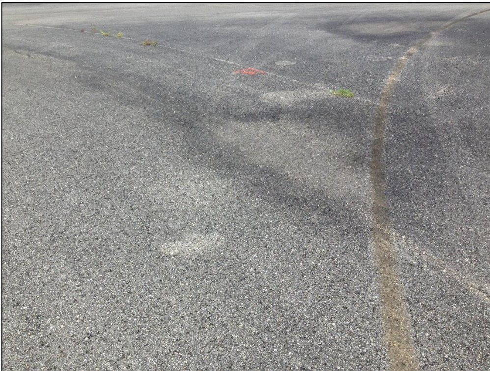
Taxiway D, Section 415, Sample Unit 101 – Low Severity (45) Depression, Medium Severity (57) Weathering
