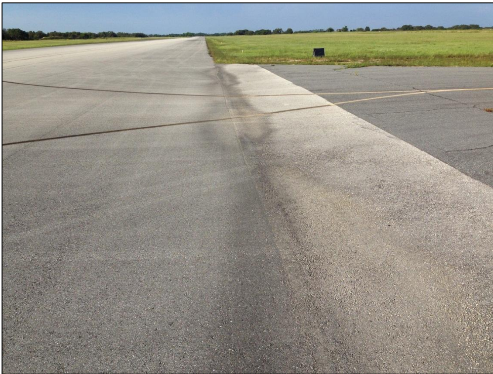
Runway 5-23, Section 6104, Sample Unit 348 –Low Severity (45) Depression, Low Severity (57) Weathering
