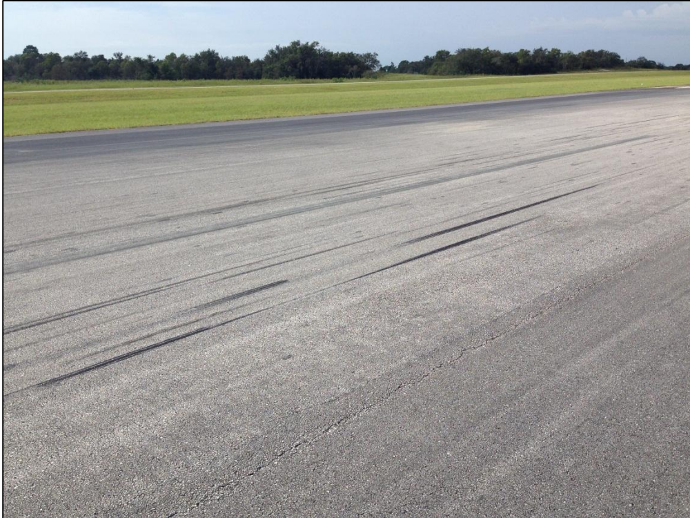
Runway 5-23, Section 6102, Sample Unit 94 – Low Severity (48) Longitudinal and Transverse Cracking, Low Severity (57) Weathering
