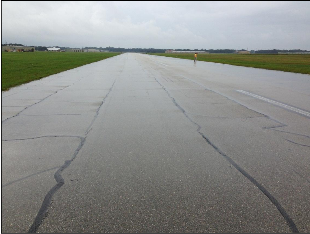
Runway 10-28, Section 6205, Sample Unit 115 – Low Severity (48) Longitudinal and Transverse Cracking, Low Severity (57) Weathering
