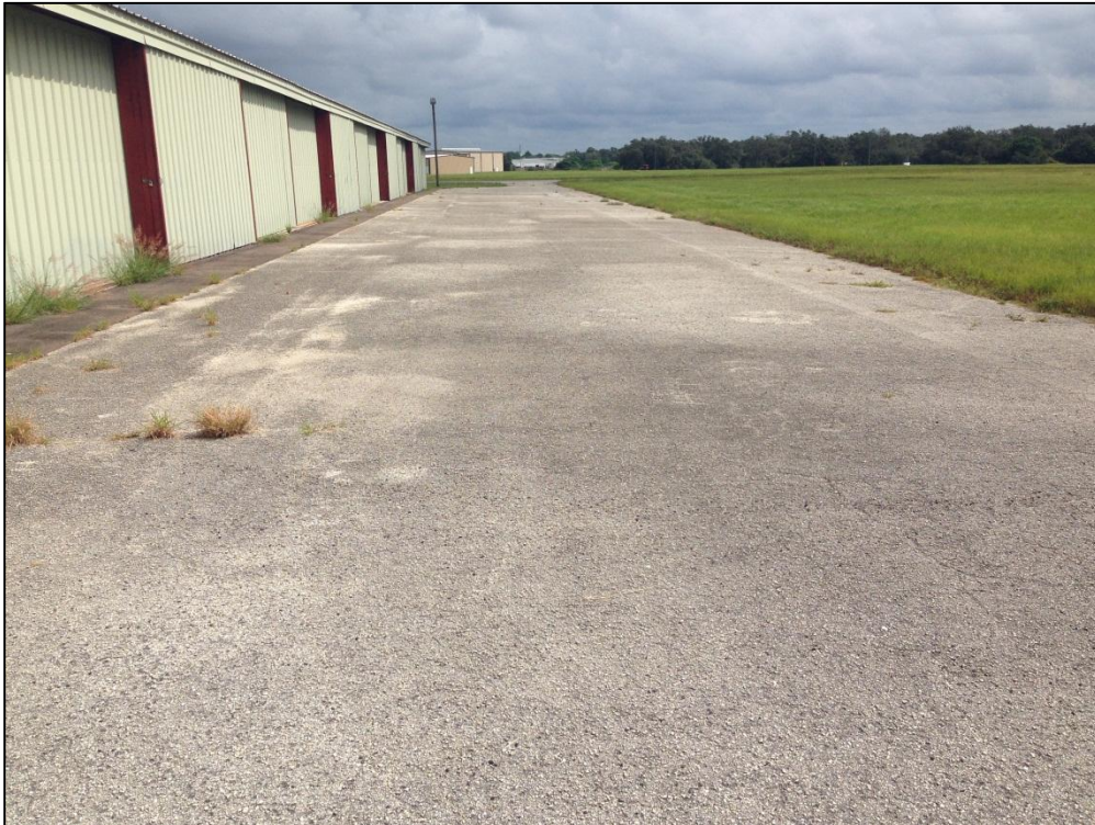
Apron S, Section 4305, Sample Unit 400 – Low Severity (43) Block Cracking, Medium Severity (52) Raveling
