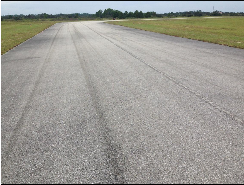
Taxiway E, Section 502, Sample Unit 104 – Low Severity (48) Longitudinal and Transverse Cracking, Low and Medium Severity (57) Weathering
