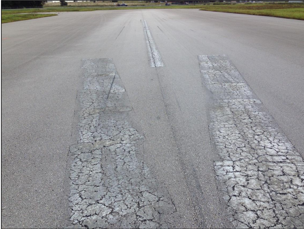
Runway 5-23, Section 6110, Sample Unit 171 – Low Severity (57) Weathering, Low Severity (52) Raveling
