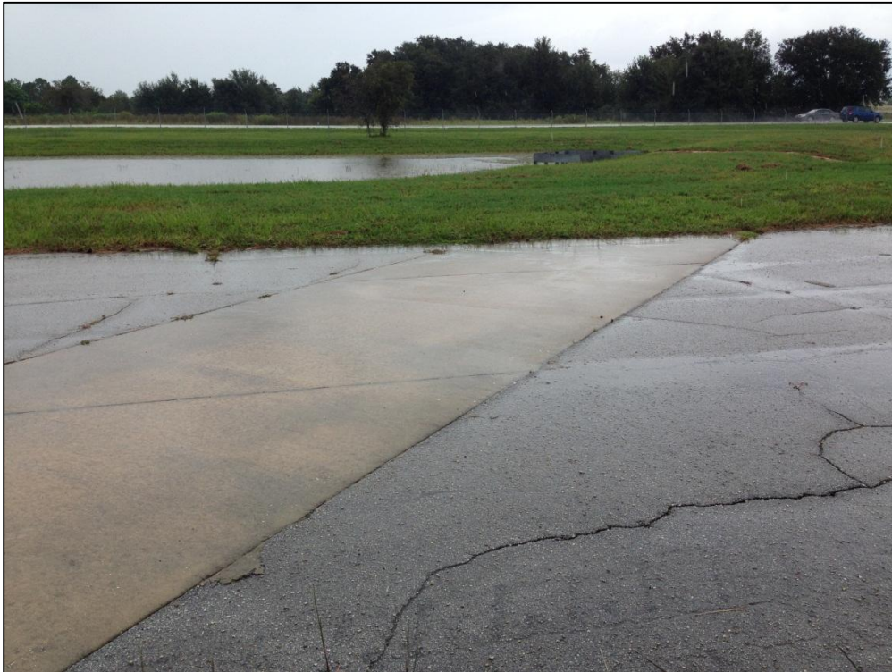
Taxiway F, Section 405, Sample Unit 101 – Low Severity (43) Block Cracking, Low Severity (50) Patching, Low Severity (52) Raveling, Low (57) Weathering
