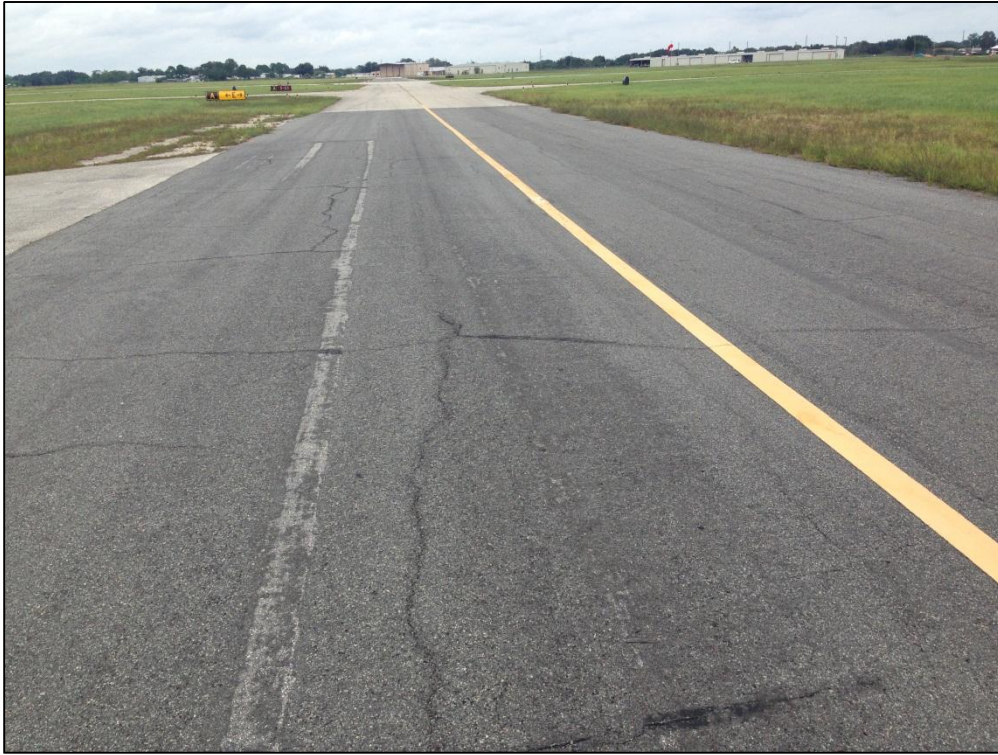
Taxiway A, Section 115, Sample Unit 105 – Low Severity (43) Block Cracking, Medium Severity (57) Weathering
