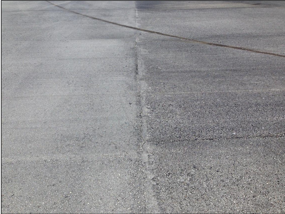
Runway 5-23, Section 6102, Sample Unit 99 – Low and Medium Severity (48) Longitudinal and Transverse Cracking, Low Severity (57) Weathering
