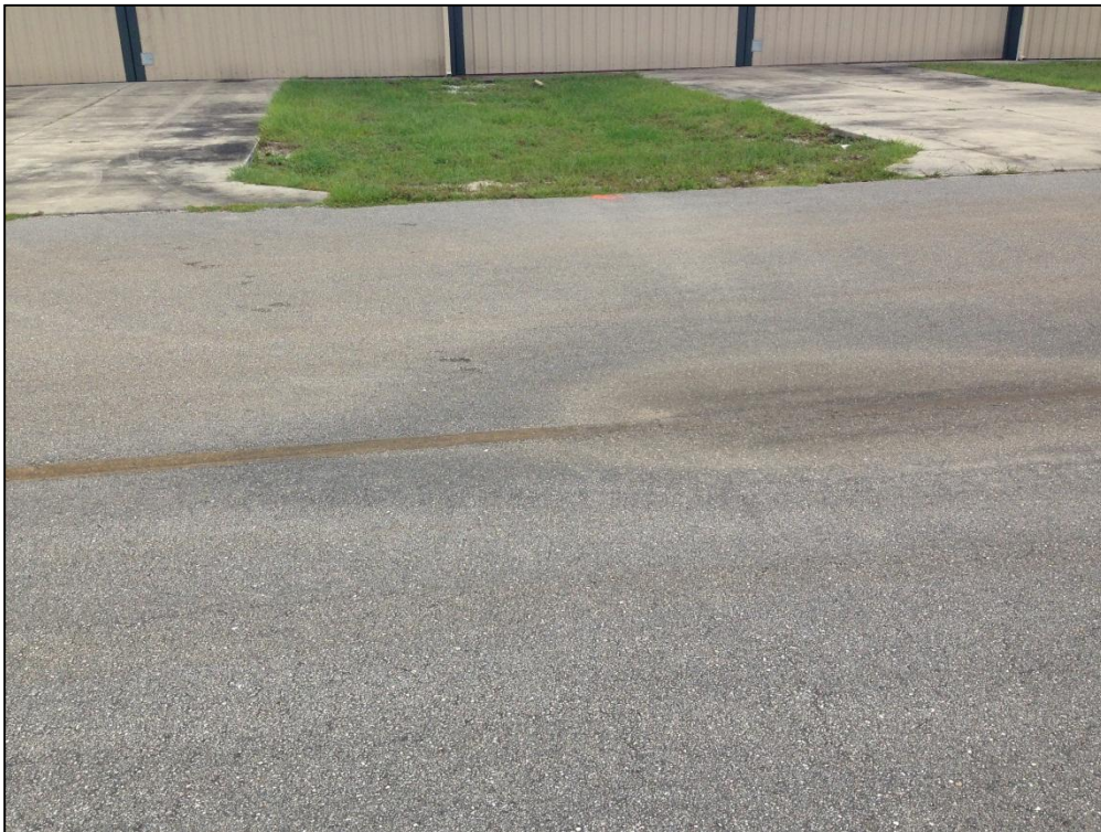
Apron T-Hang, Section 4605, Sample Unit 402 – Low Severity (45) Depression, Low Severity (57) Weathering
