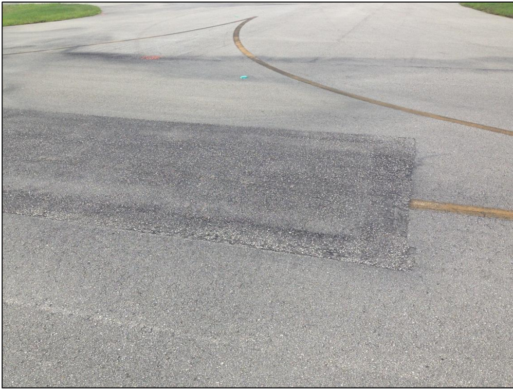
Taxiway H, Section 605, Sample Unit 102 – Medium Severity (50) Patching, Low Severity (57) Weathering
