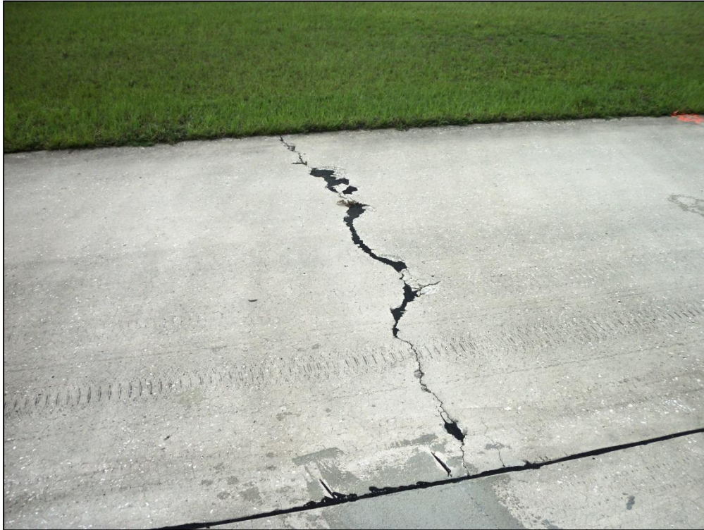
Runway 3-21, Section 6205, Sample Unit 164 – Low Severity (66) Small Patching, Medium Severity (63) Longitudinal, Transverse and Diagonal Cracking, (73) Shrinkage Cracking
