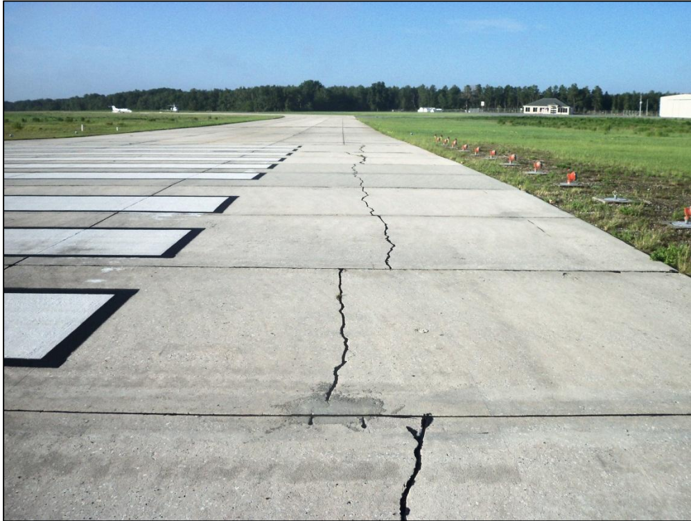
Runway 9-27, Section 6110, Sample Unit 300 – Low Severity (66) Small Patching, Low Severity (63) Longitudinal, Transverse and Diagonal Cracking
