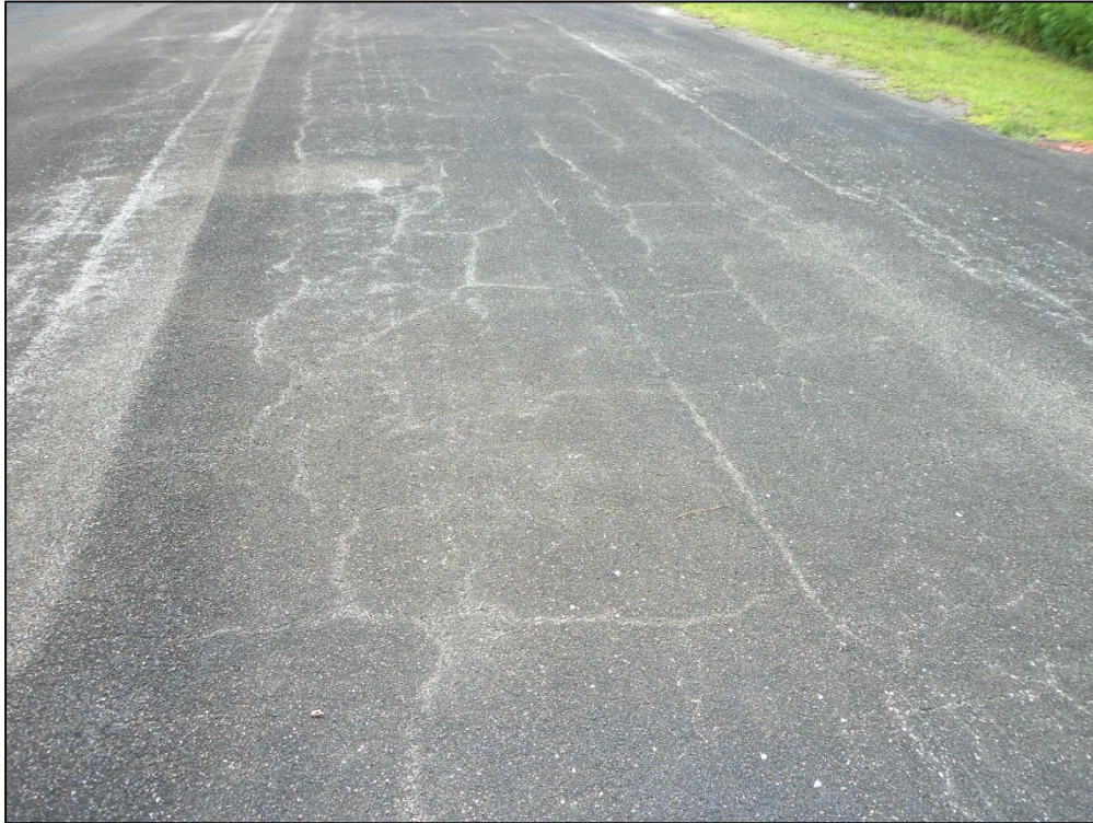
Apron North East, Section 4105, Sample Unit 852 – Low Severity (43) Block Cracking, Low Severity (48) Longitudinal and Transverse Cracking, Low Severity (57) Weathering, Low and High Severity (52) Raveling
