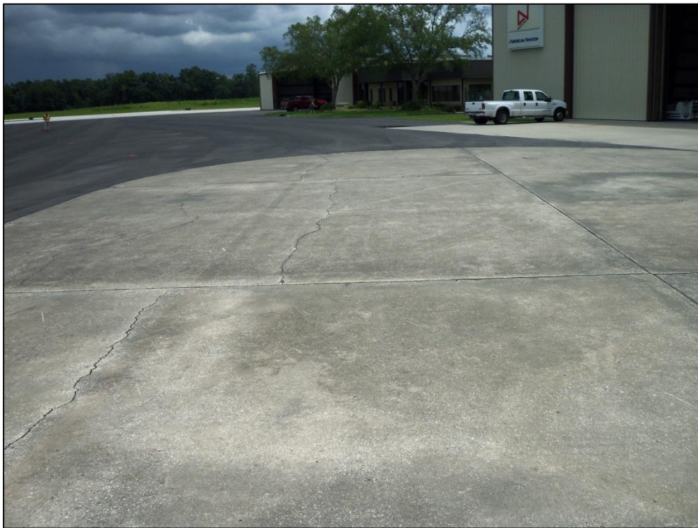
Apron North East, Section 4130, Sample Unit 100 – Low Severity (63) Longitudinal, Transverse and Diagonal Cracking
