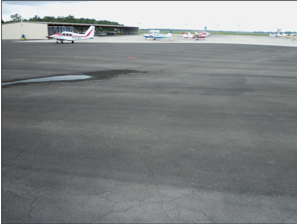
Apron North East, Section 4147, Sample Unit 155 – Low Severity (45) Depression, Low Severity (43) Block Cracking
