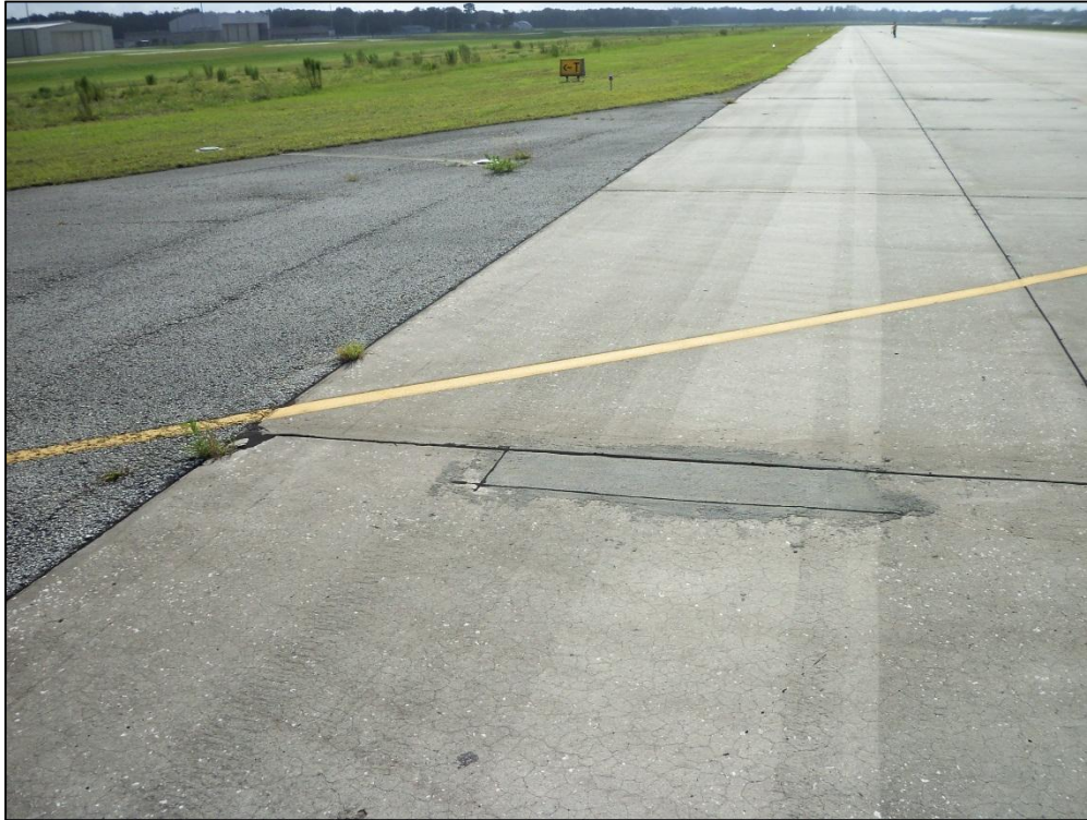
Runway 9-27, Section 6105, Sample Unit 168 –Medium Severity (70) Scaling, Map Cracking, Crazing, Low Severity (66) Small Patching, Low Severity (75) Corner Spalling
