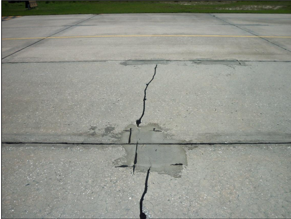
Taxiway A9, Section 140, Sample Unit 902 – Low and Medium Severity (70) Scaling, Map Cracking, Crazing, Low Severity (66) Small Patching, Low Severity (63) Longitudinal, Transverse and Diagonal Cracking
