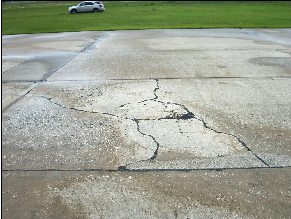
Runway 3-21, Section 6210, Sample Unit 313 – High Severity (72) Shattered Slab
