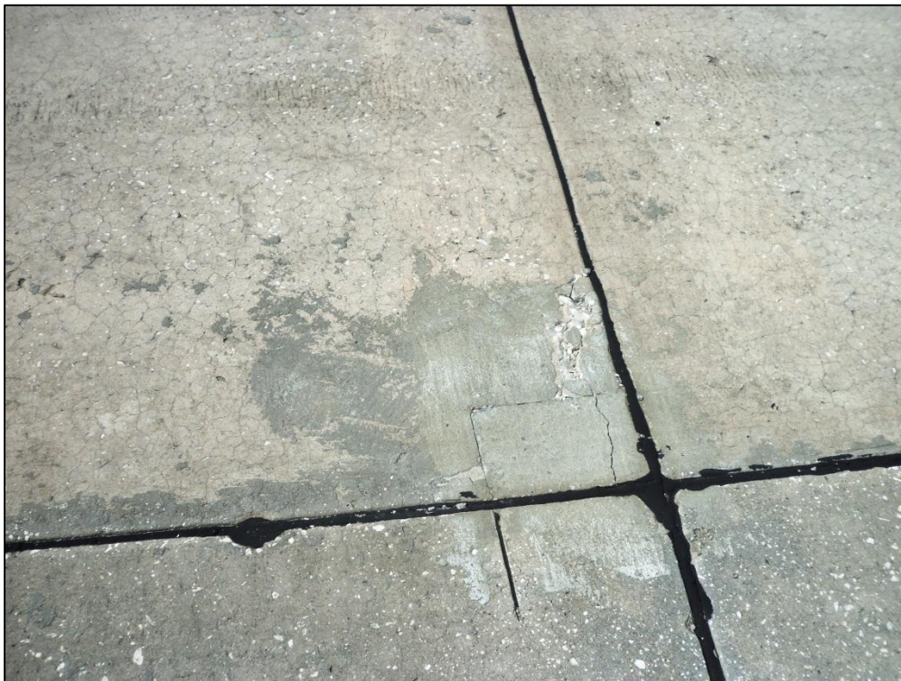
Taxiway Alpha, Section 105, Sample Unit 254 –Medium Severity (70) Scaling, Map Cracking, Crazing, Low Severity (66) Small Patching, Low Severity (74) Joint Spalling
