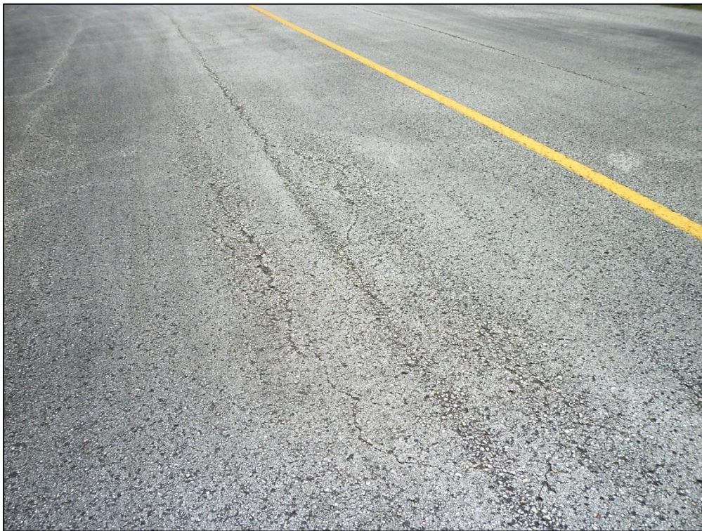
Taxiway A6, Section 135, Sample Unit 606 –Low and Medium Severity (48) Longitudinal and Transverse Cracking, Medium and High Severity (52) Raveling
