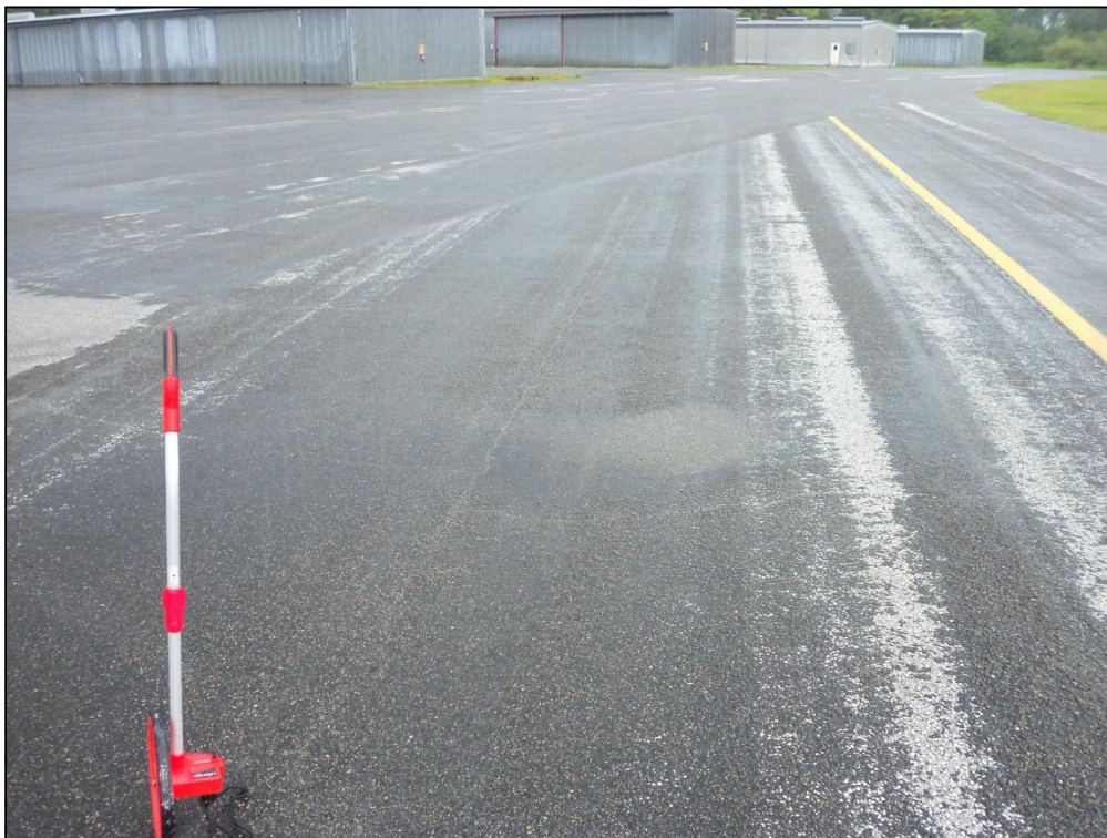
Taxiway A1, Section 112, Sample Unit 119 – Low Severity (45) Depression, Low Severity (57) Weathering, Low and Medium Severity (52) Raveling, Low Severity (48) Longitudinal and Transverse Cracking
