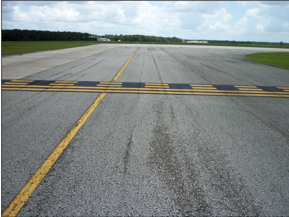
Taxiway A6, Section 125, Sample Unit 301 –Low and Medium Severity (48) Longitudinal and Transverse Cracking, Medium and High Severity (52) Raveling
