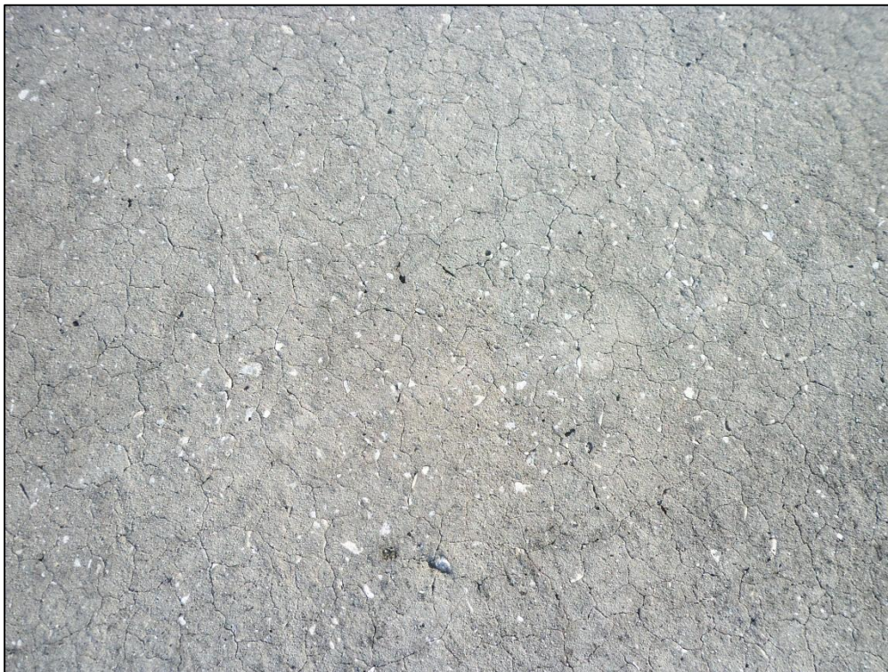
Runway 9-27, Section 6105, Sample Unit 104 – Medium Severity (70) Scaling, Map Cracking, Crazing
