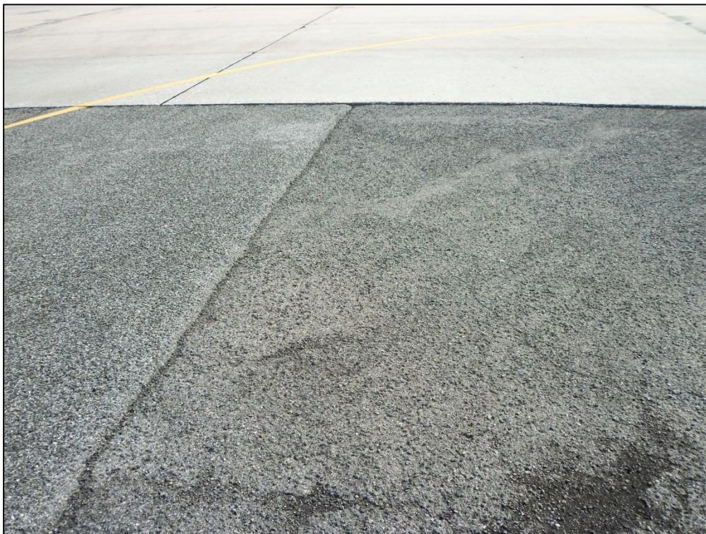
Taxiway Bravo, Section 205, Sample Unit 148 – Low and Medium Severity (48) Longitudinal and Transverse Cracking, Medium and High Severity (52) Raveling
