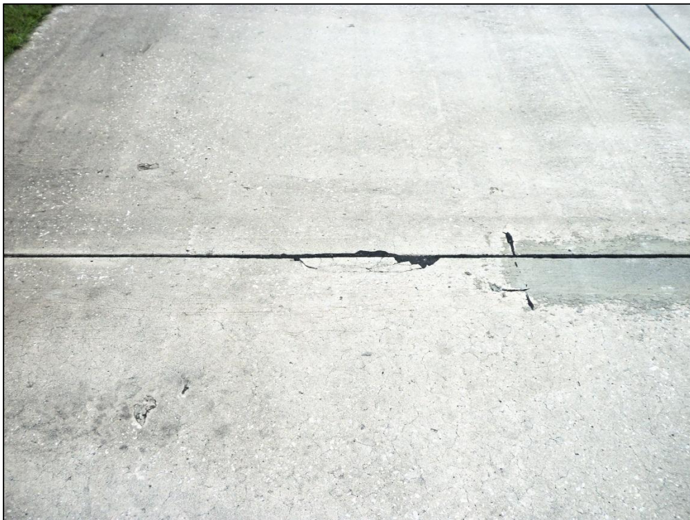
Runway 3-21, Section 6205, Sample Unit 592 –Low Severity (70) Scaling, Map Cracking, Crazing, Low Severity (66) Small Patching, Low Severity (74) Joint Spalling
