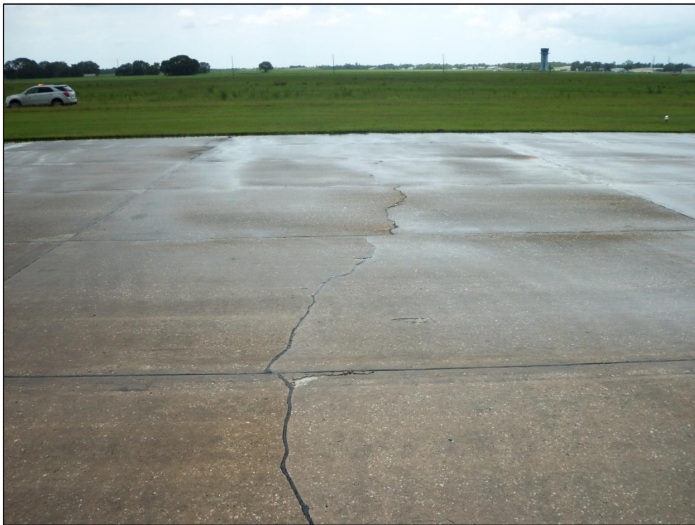
Runway 3-21, Section 6210, Sample Unit 337 – Low Severity (63) Longitudinal, Transverse and Diagonal Cracking, Medium Severity (74) Joint Spalling
