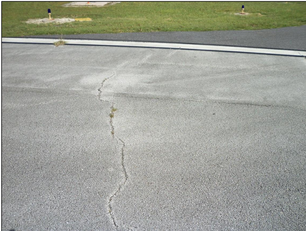
Runway 5-23, Section 6315, Sample Unit 187 – Low Severity (52) Raveling, Low Severity (57) Weathering, Medium Severity (48) Longitudinal and Transverse Cracking
