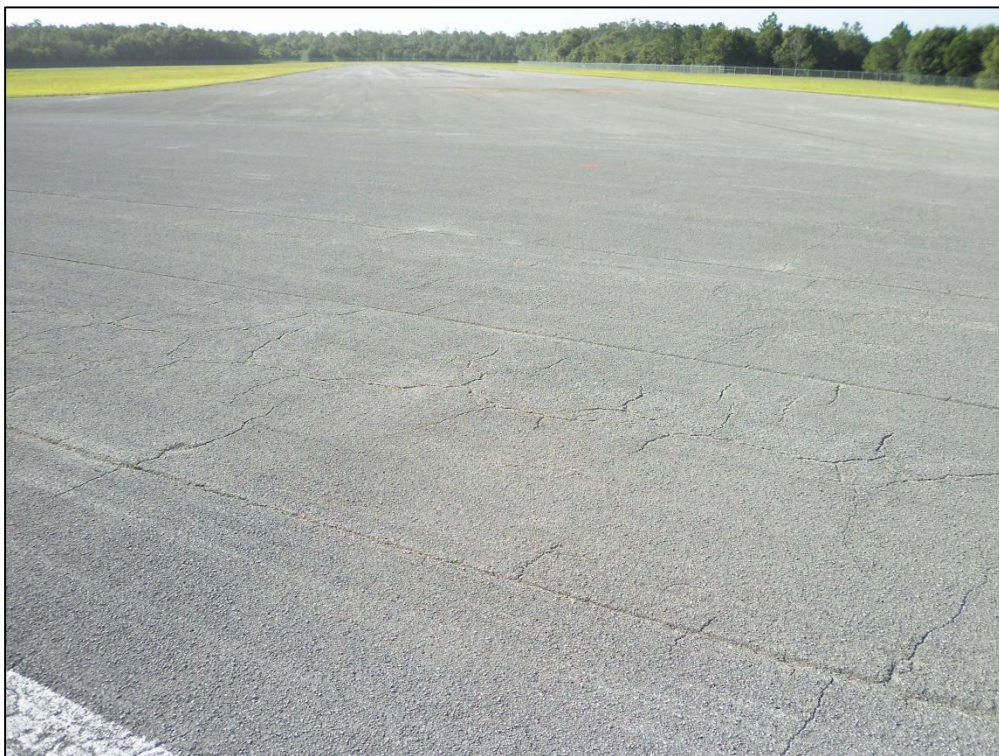
Runway 9R-27L, Section 6205, Sample Unit 354 – Medium Severity (52) Raveling, Medium Severity (43) Block Cracking
