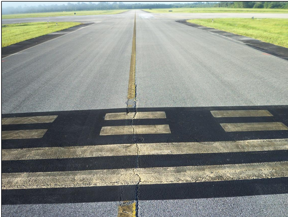
Taxiway C, Section 310, Sample Unit 106 – Low Severity (52) Raveling, Low Severity (57) Weathering, Low and Medium Severity (48) Longitudinal and Transverse Cracking
