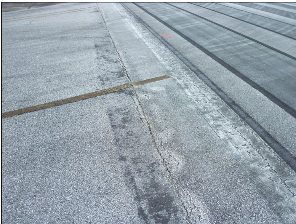
Taxiway C3, Section 320, Sample Unit 112 – Low Severity (52) Raveling, Low Severity (57) Weathering, Low Severity (48) Longitudinal and Transverse Cracking
