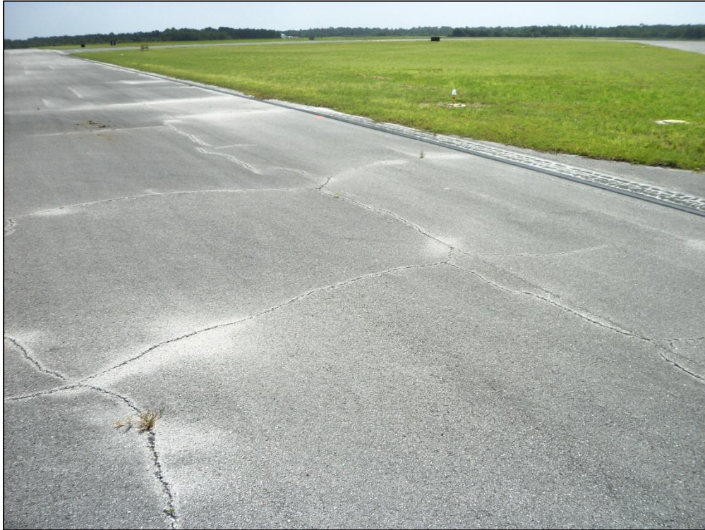
Runway 5-23, Section 6315, Sample Unit 145 – Low Severity (52) Raveling, Low Severity (57) Weathering, Medium Severity (43) Block Cracking
