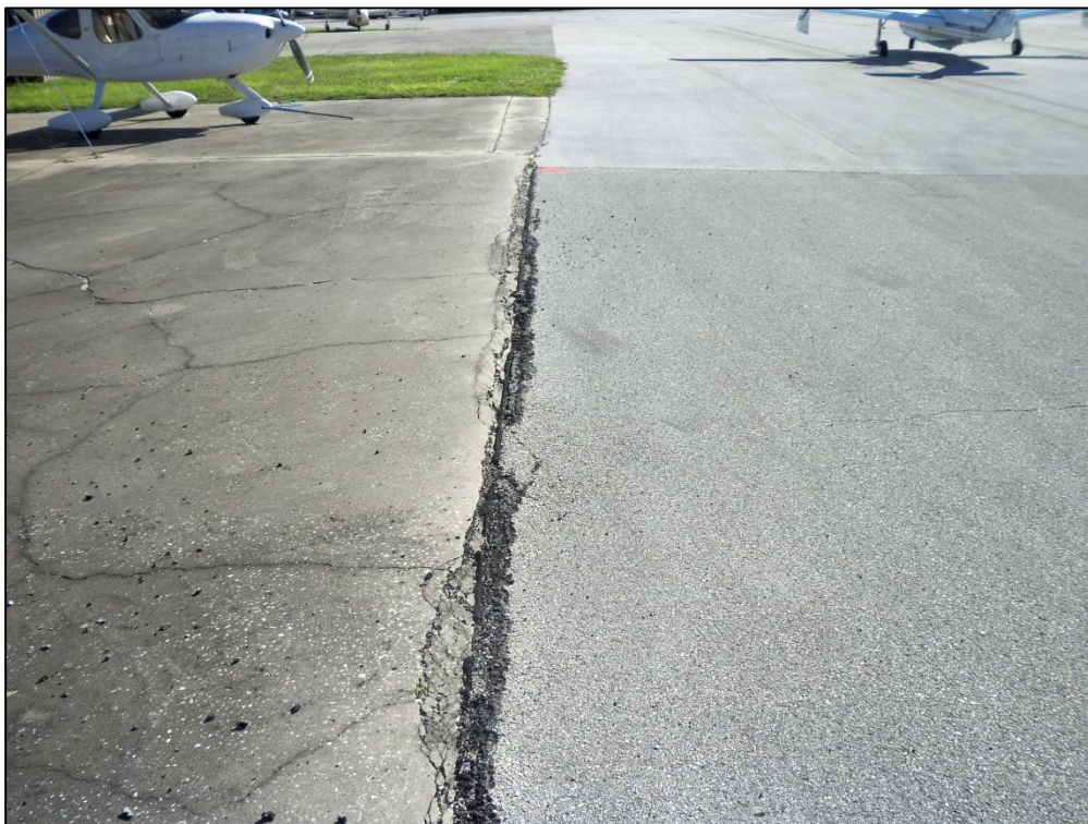
Apron North, Section 4120, Sample Unit 106 – Low Severity (52) Raveling, Low Severity (57) Weathering, Medium Severity (54) Shoving
