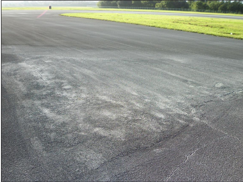
Runway 9R-27L, Section 6205, Sample Unit 329 – Medium Severity (50) Patching
