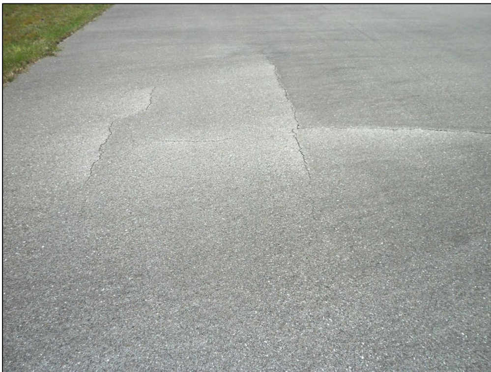
Runway 9L-27R, Section 6110, Sample Unit 104 –Low Severity (57) Weathering, Low Severity (48) Longitudinal and Transverse Cracking
