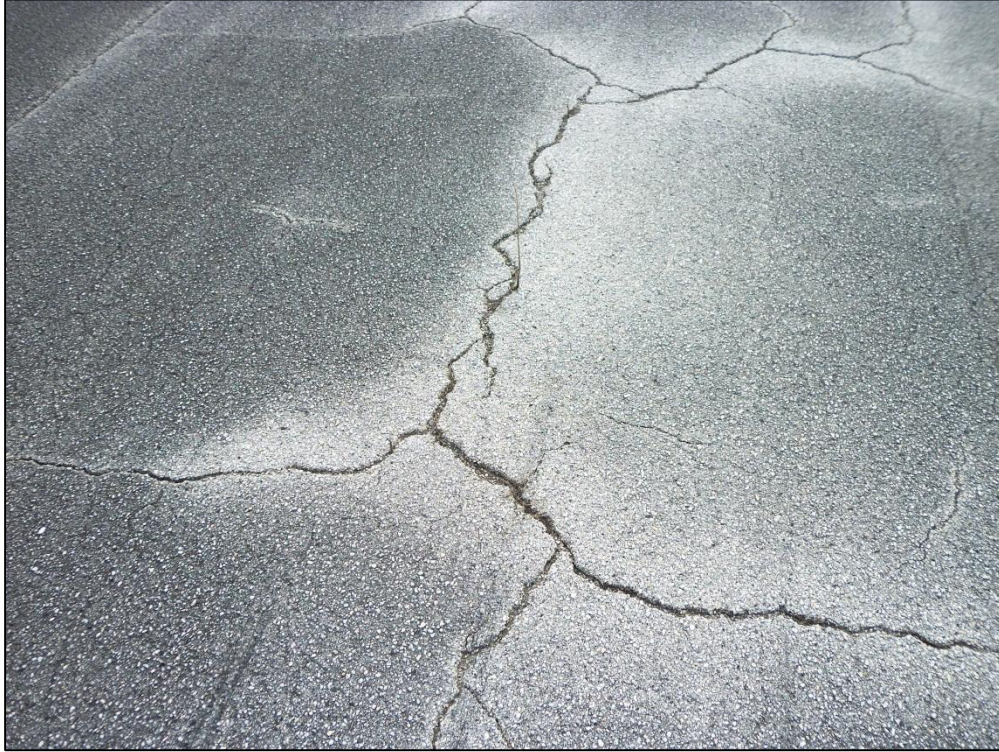
Runway 9R-27L, Section 6205, Sample Unit 378 – Medium Severity (52) Raveling, Medium Severity (43) Block Cracking
