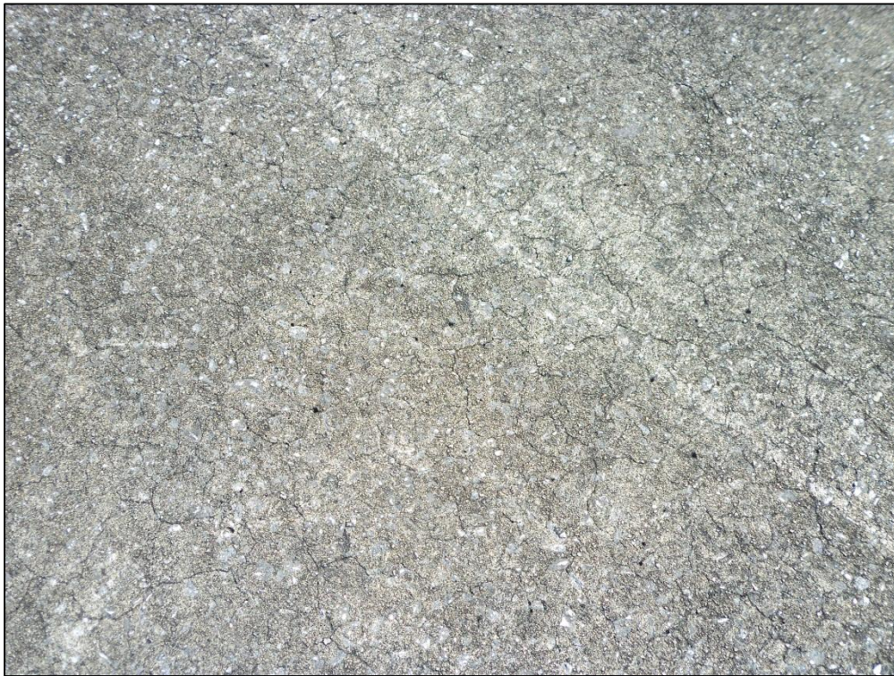
Runway 9R-27L, Section 6220, Sample Unit 184 – Low Severity (70) Scaling, Map Cracking, Crazing
