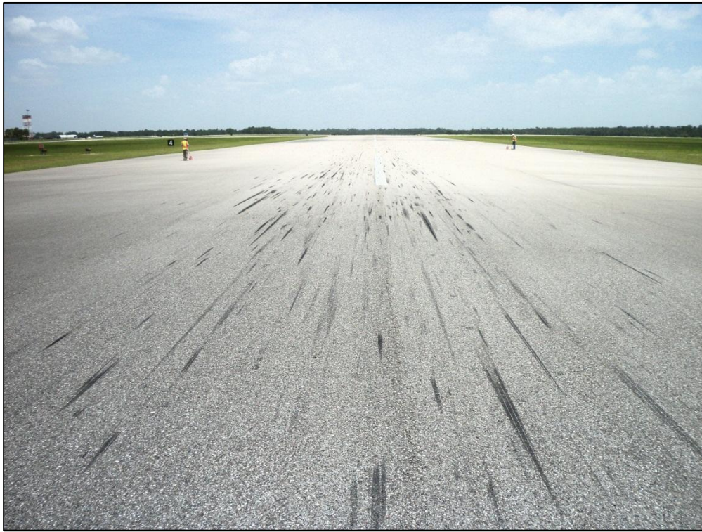
Runway 9L-27R, Section 6115, Sample Unit 310 –Medium Severity (57) Weathering
