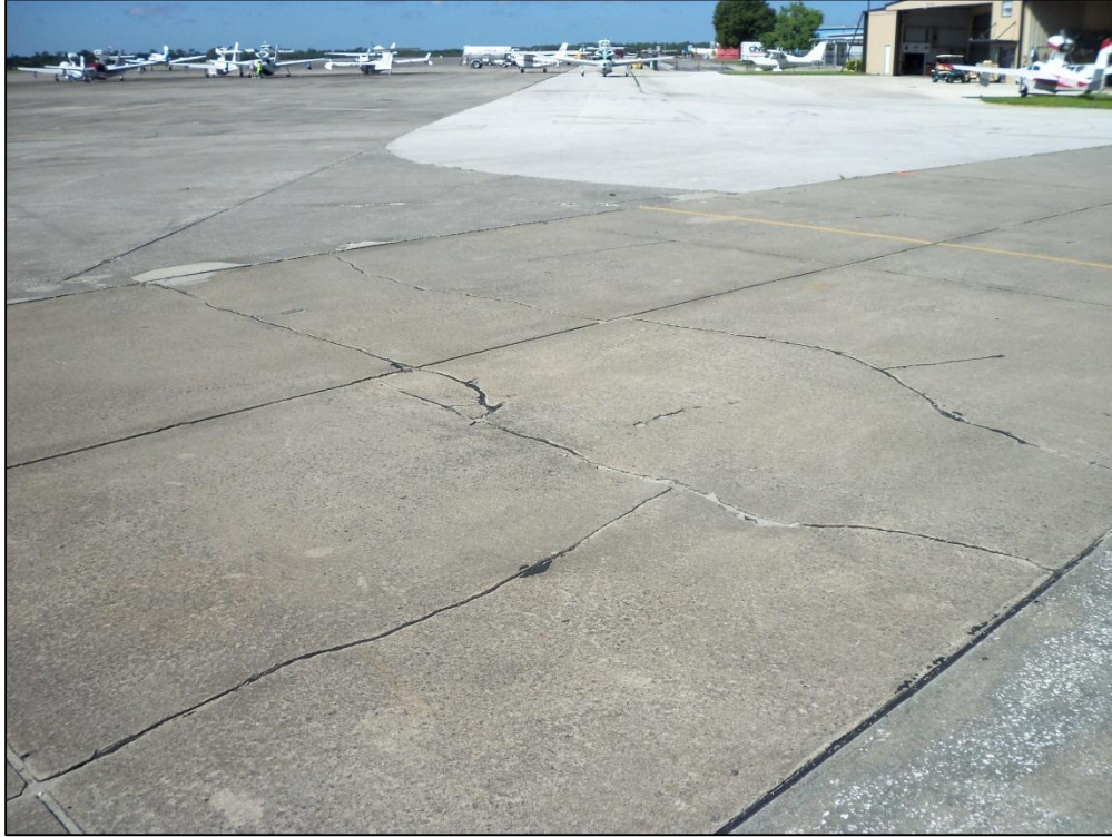
Apron North, Section 4132, Sample Unit 602 – Low Severity (72) Shattered Slab
