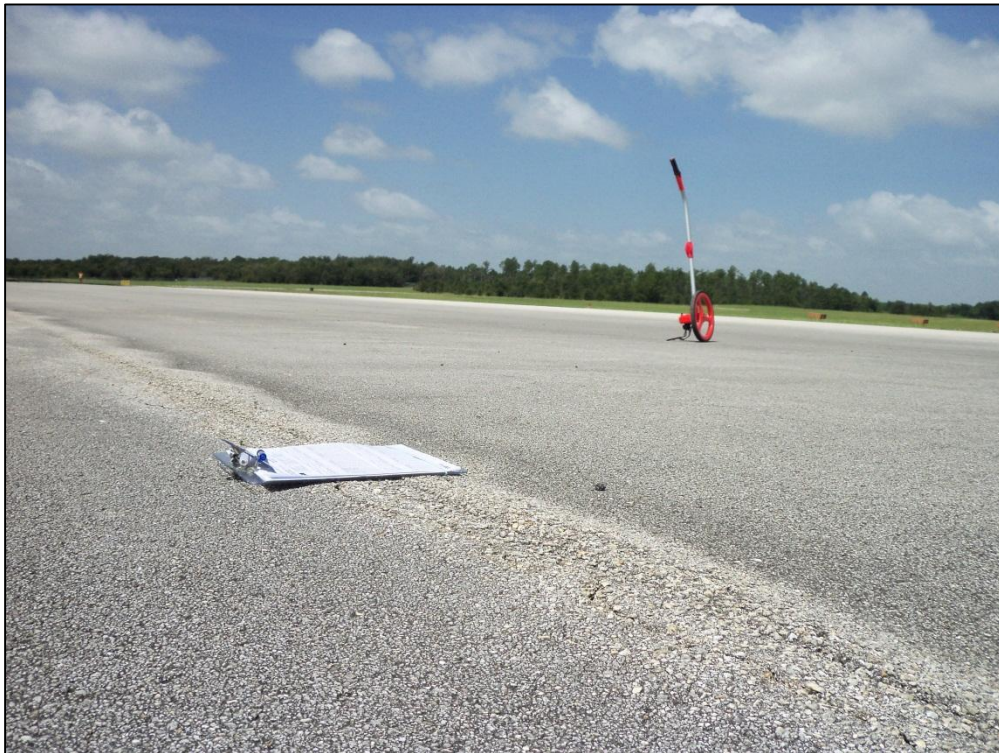
Runway 5-23, Section 6315, Sample Unit 117 – Low Severity (52) Raveling, Low Severity (57) Weathering, Medium Severity (56) Swelling
