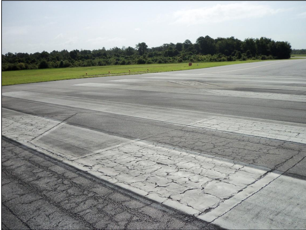
Runway 5-23, Section 6315, Sample Unit 198 – Medium Severity (52) Raveling, Low Severity (48) Longitudinal and Transverse Cracking
