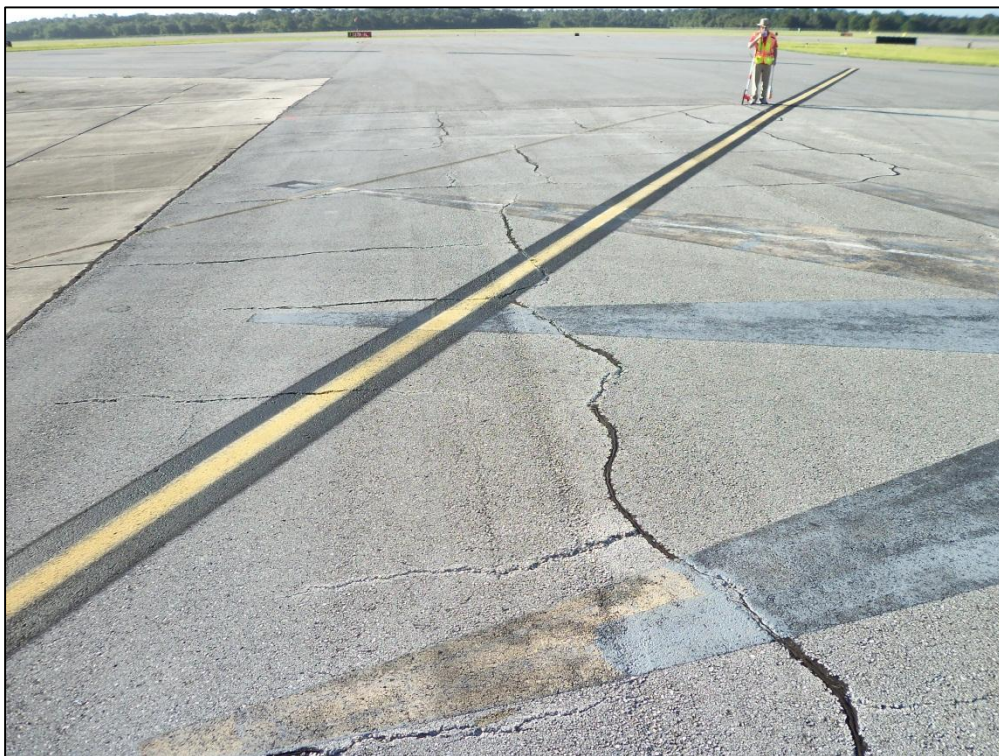
Apron North, Section 4105, Sample Unit 200 – Low and Medium Severity (52) Raveling, Medium Severity (43) Block Cracking
