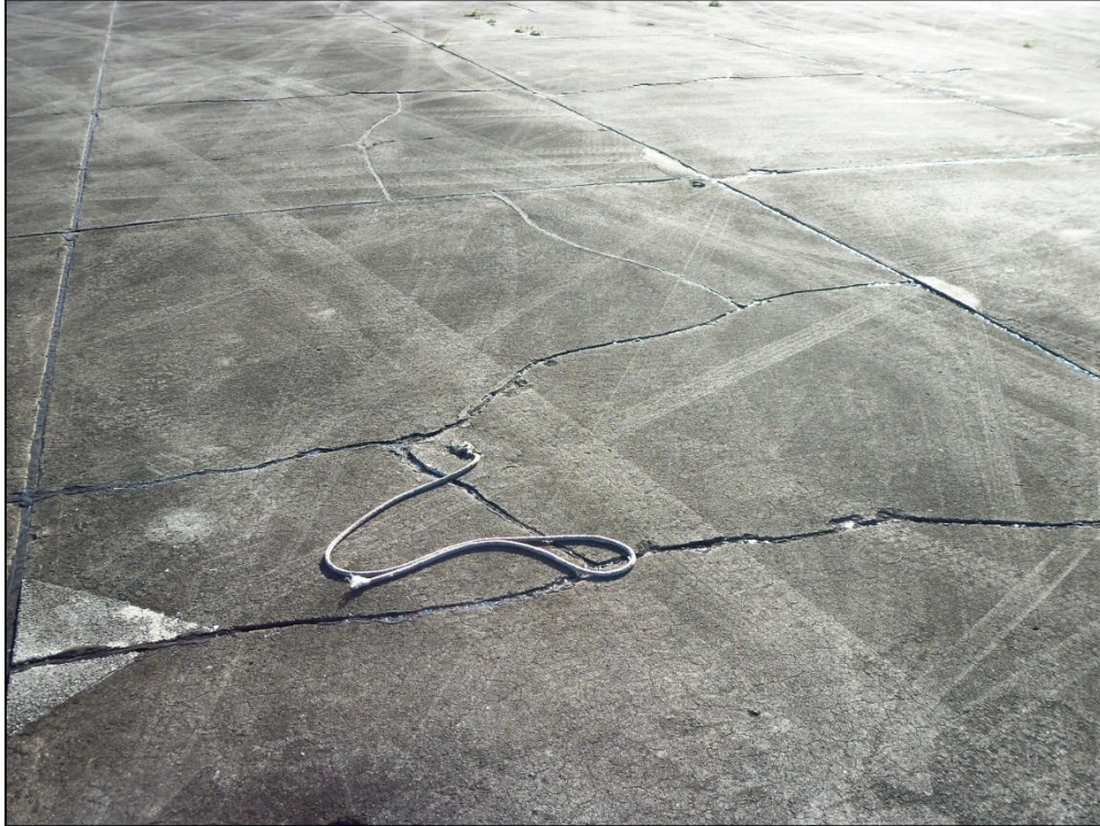
Apron North, Section 4110, Sample Unit 802 – Low Severity (72) Shattered Slab
