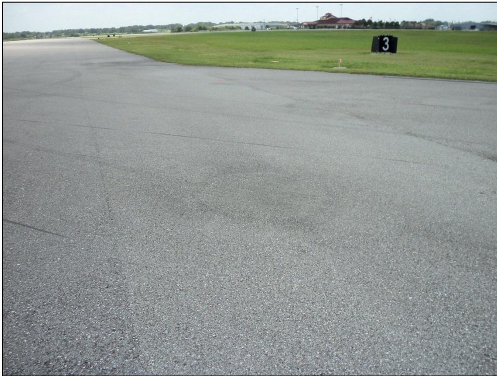
Runway 9L-27R, Section 6124, Sample Unit 160 –Low Severity (57) Weathering, Low Severity (45) Depression
