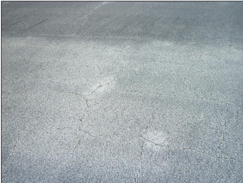
Runway 9R-27L, Section 6210, Sample Unit 512 – Medium (52) Raveling, Low Severity (43) Block Cracking
