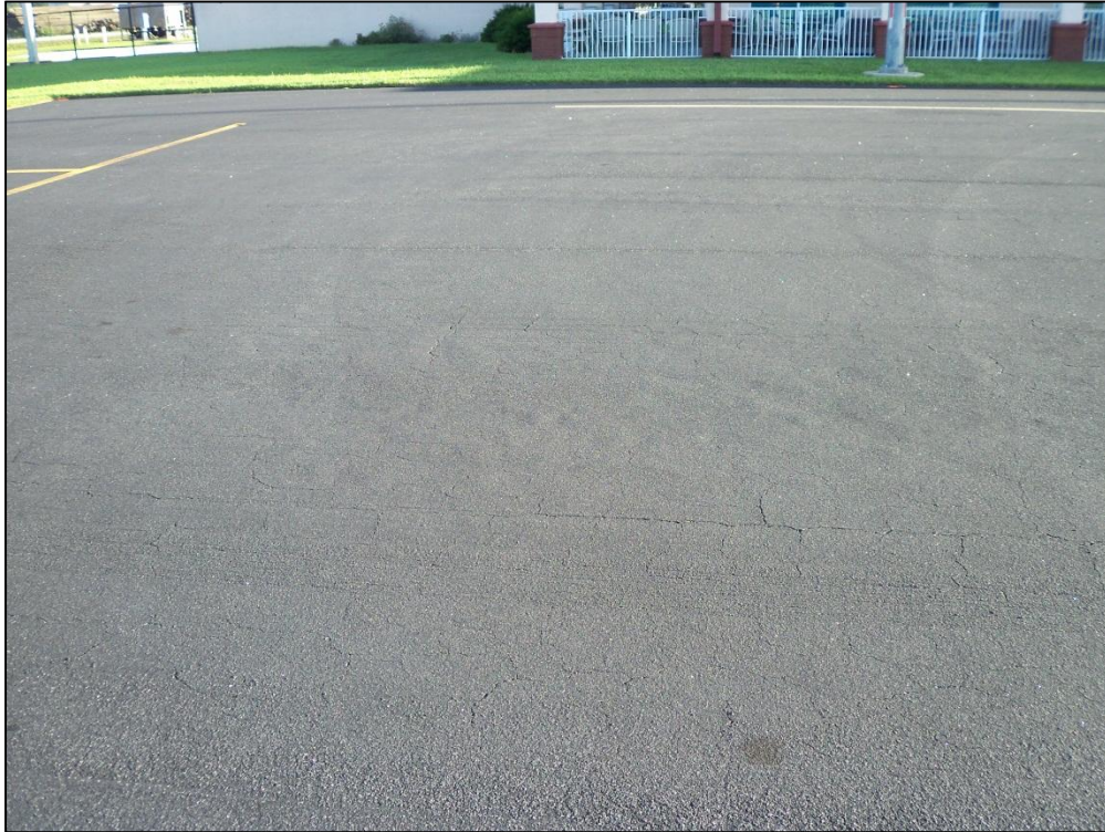
Apron FBO, Section 4405, Sample Unit 100 – Low Severity (57) Weathering
