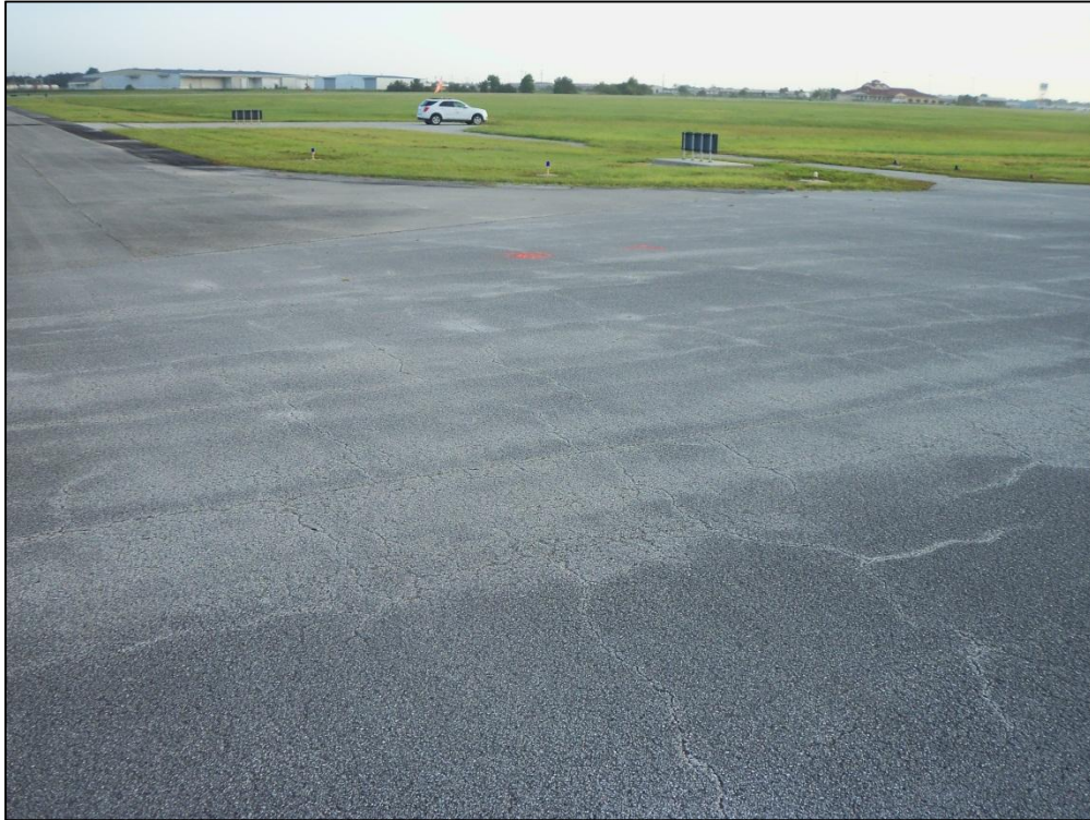
Runway 9R-27L, Section 6205, Sample Unit 300 – Medium Severity (52) Raveling, Low Severity (43) Block Cracking
