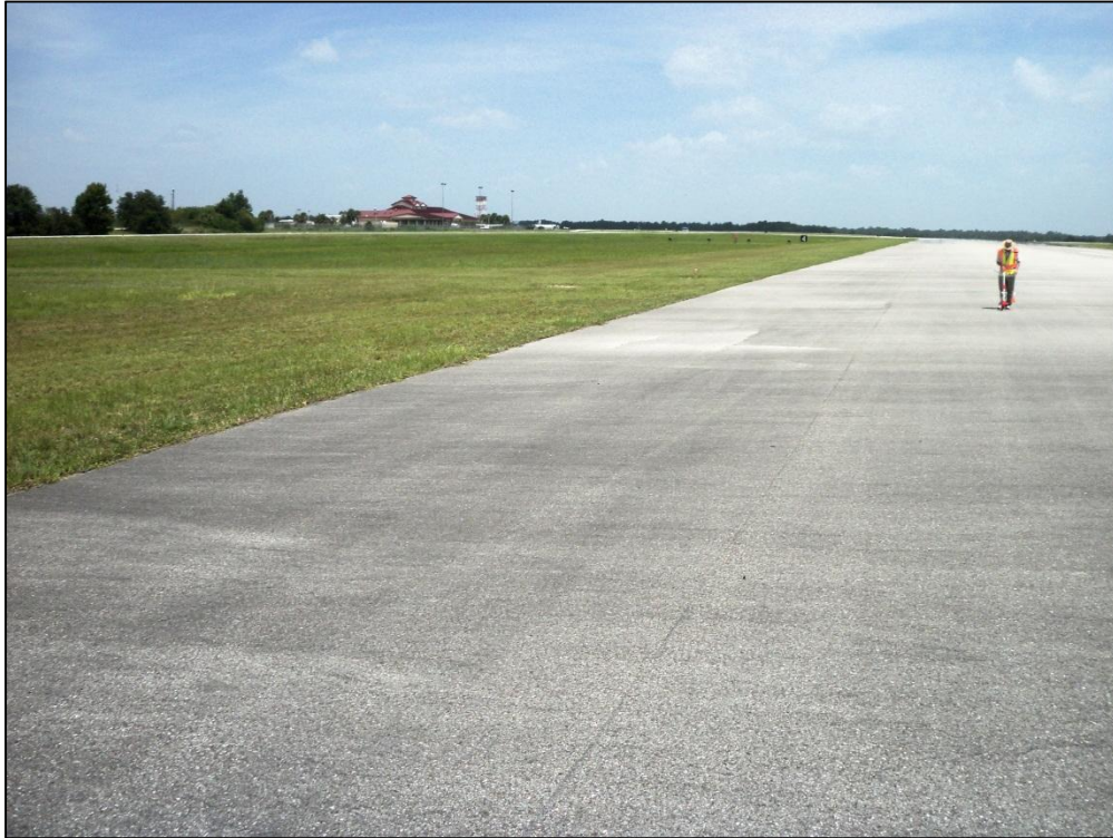
Runway 9L-27R, Section 6110, Sample Unit 104 – Low Severity (57) Weathering
