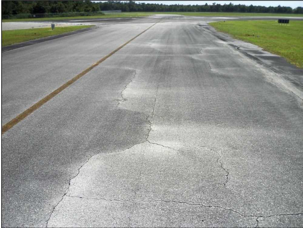
Taxiway A3, Section 115, Sample Unit 109 – Low Severity (52) Raveling, Low Severity (57) Weathering, Low and Medium Severity (48) Longitudinal and Transverse Cracking
