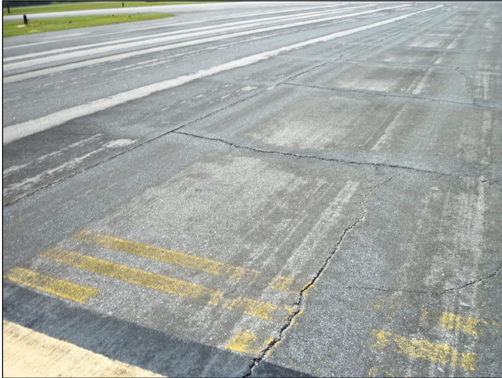
Taxiway F, Section 610, Sample Unit 103 – Medium Severity (57) Weathering, Medium Severity (43) Block Cracking
