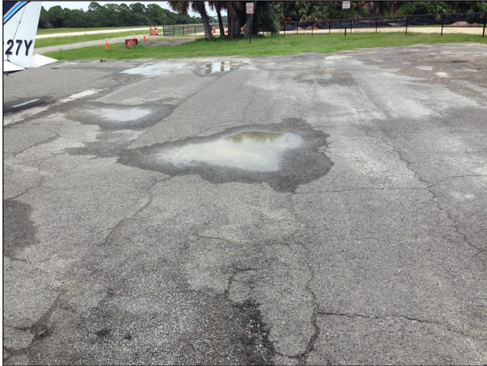
Apron, Section 4105, Sample Unit 100 – Low Severity (43) Block Cracking, Medium and High Severity (52) Raveling, Low and Medium Severity (45) Depression
