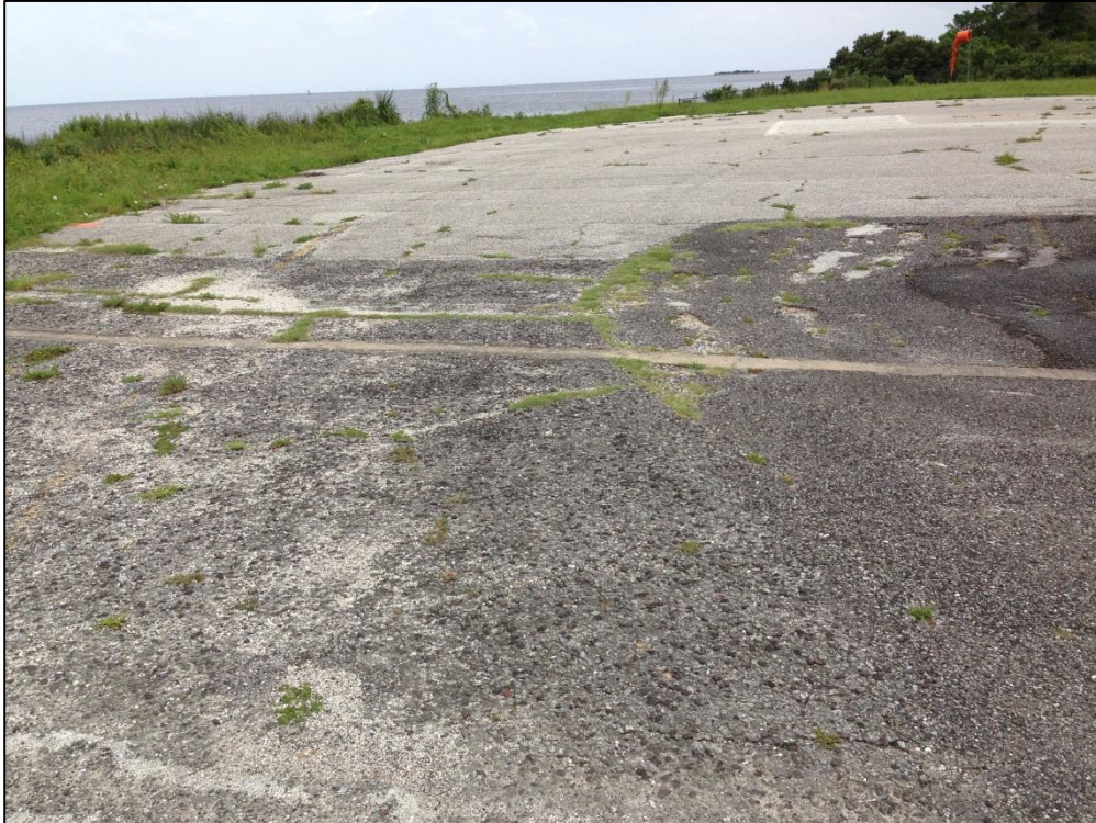
Taxiway A, Section 105, Sample Unit 100 – Medium Severity (43) Block Cracking, High Severity (52) Raveling, Medium Severity (50) Patching
