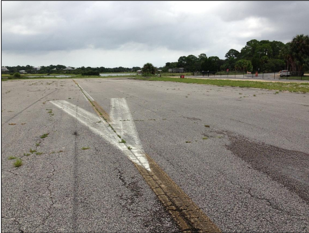
Runway 5-23, Section 6105, Sample Unit 143 – Low Severity (43) Block Cracking, Low and Medium Severity (52) Raveling, Low Severity (57) Weathering
