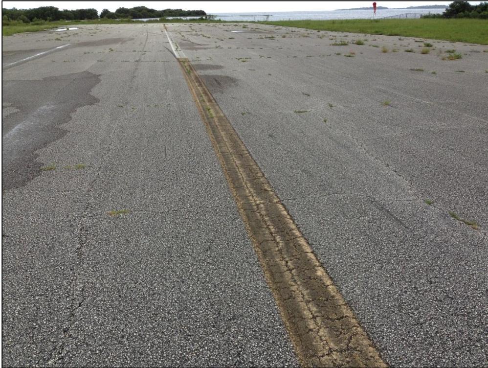
Runway 5-23, Section 6105, Sample Unit 105 – Low Severity (43) Block Cracking, Low and Medium Severity (52) Raveling, Low Severity (45) Depression, Low Severity (57) Weathering
