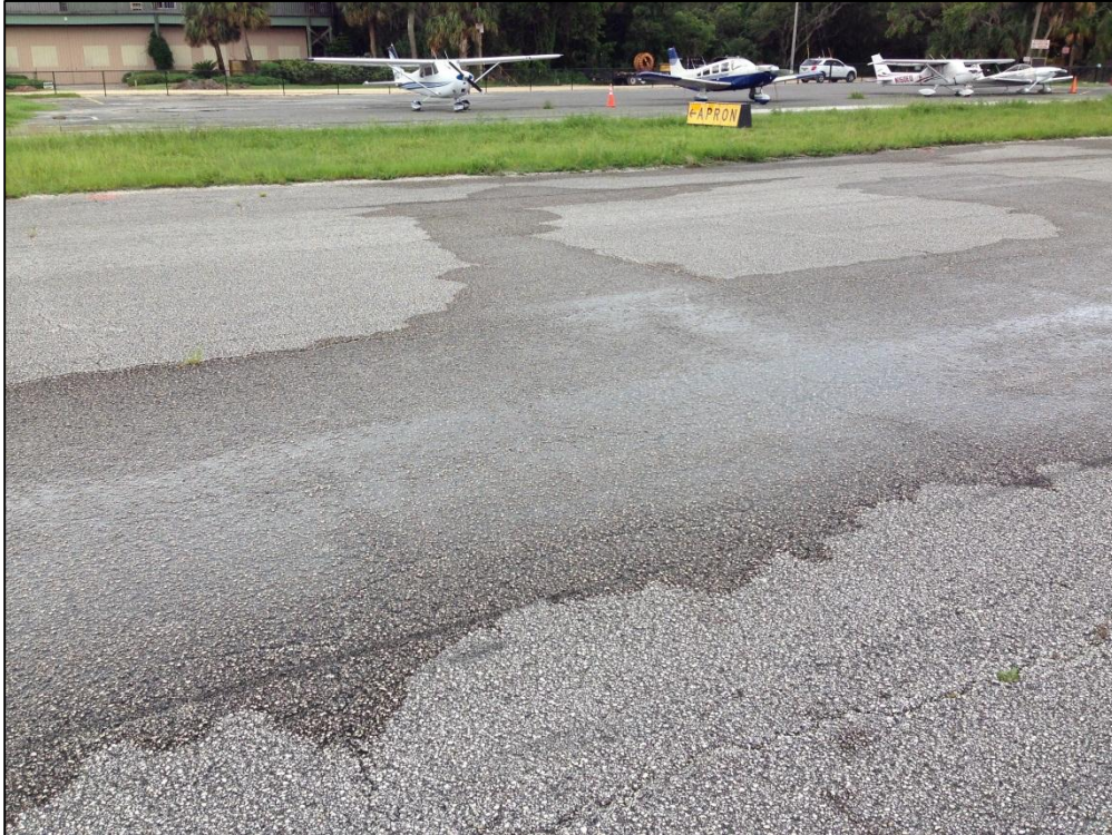
Runway 5-23, Section 6105, Sample Unit 105 – Low and Medium Severity (52) Raveling, Low Severity (45) Depression, Low Severity (43) Block Cracking, Low Severity (57) Weathering
