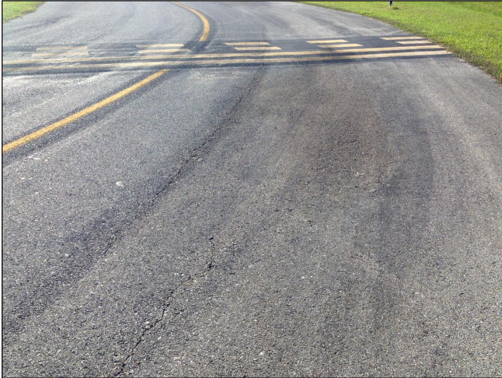
Taxiway Parallel, Section 105, Sample Unit 101 – Low Severity (48) Longitudinal and Transverse Cracking, Low Severity (52) Raveling, Low Severity (57) Weathering, Low Severity (45) Depression
