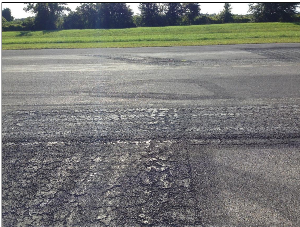
Runway 18-36, Section 6105, Sample Unit 101 – Low Severity (48) Longitudinal and Transverse Cracking, Low and Medium Severity (52) Raveling, Low Severity (57) Weathering
