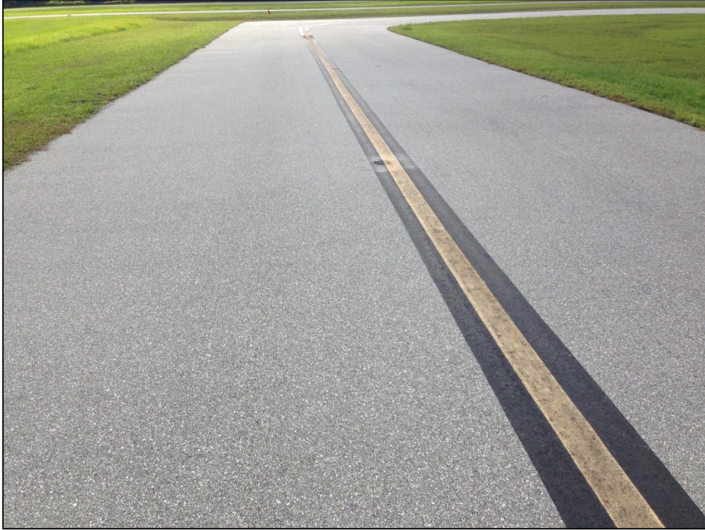
T-Hangar North, Section 240, Sample Unit 400 – Low Severity (57) Weathering
