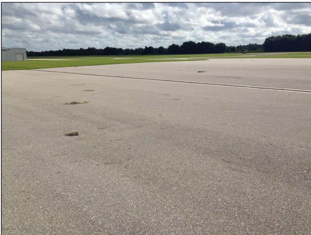
Apron, Section 4205, Sample Unit 101 – Low Severity (57) Weathering
