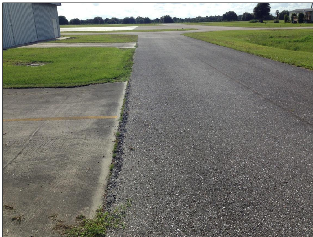
Taxiway T-Hangar, Section 210, Sample Unit 102 – Low Severity (52) Raveling, Low Severity (57) Weathering, Low Severity (54) Shoving
