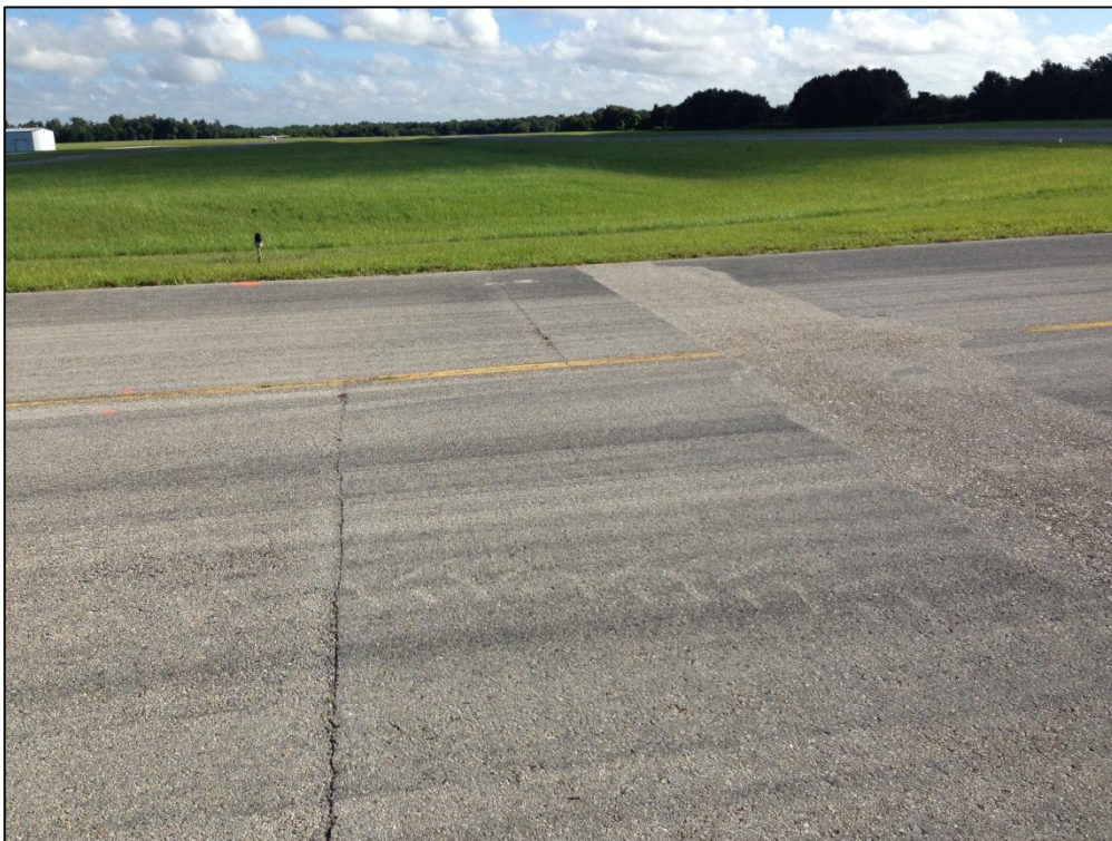
Taxiway T-Hangar, Section 205, Sample Unit 100 – Low Severity (48) Longitudinal and Transverse Cracking, Low Severity (52) Raveling, Low Severity (57) Weathering
