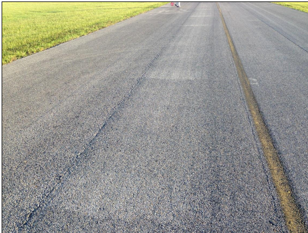
Taxiway Parallel, Section 125, Sample Unit 101 – Low Severity (48) Longitudinal and Transverse Cracking, Low Severity (52) Raveling, Low Severity (57) Weathering
