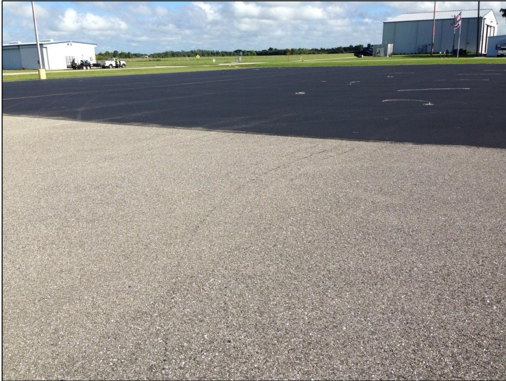
Apron, Section 4105, Sample Unit 102 – Low Severity (52) Raveling, Low Severity (57) Weathering
