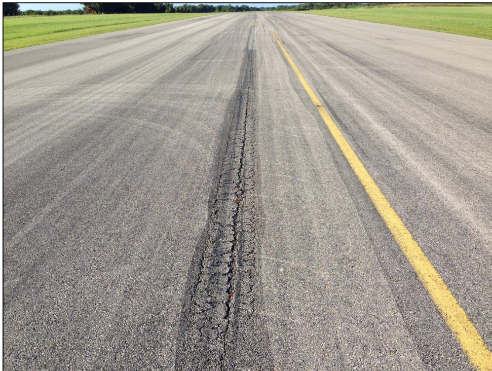
Runway 18-36, Section 6105, Sample Unit 136 – Low Severity (48) Longitudinal and Transverse Cracking, Low Severity (52) Raveling, Low Severity (57) Weathering
