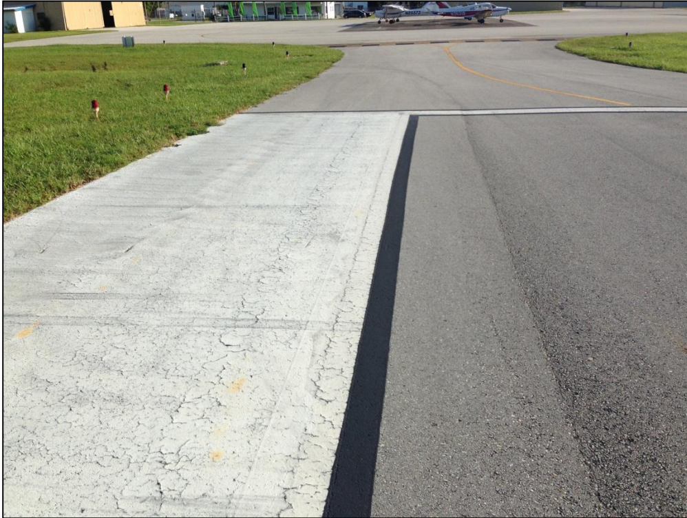
Runway 11-29, Section 6105, Sample Unit 100 – Low Severity (48) Longitudinal and Transverse Cracking, Low Severity (57) Weathering, Low Severity (52) Raveling
