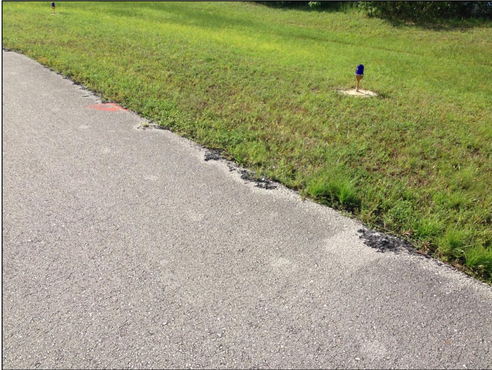
Apron Run-Up Runway 29, Section 5105, Sample Unit 102 – Low Severity (57) Weathering, Medium Severity (52) Raveling
