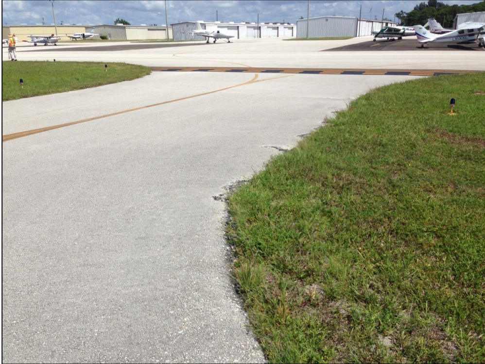
Taxiway B4, Section 410, Sample Unit 400 – Low Severity (48) Longitudinal and Transverse Cracking, Low Severity (57) Weathering, Low and Medium Severity (52) Raveling
