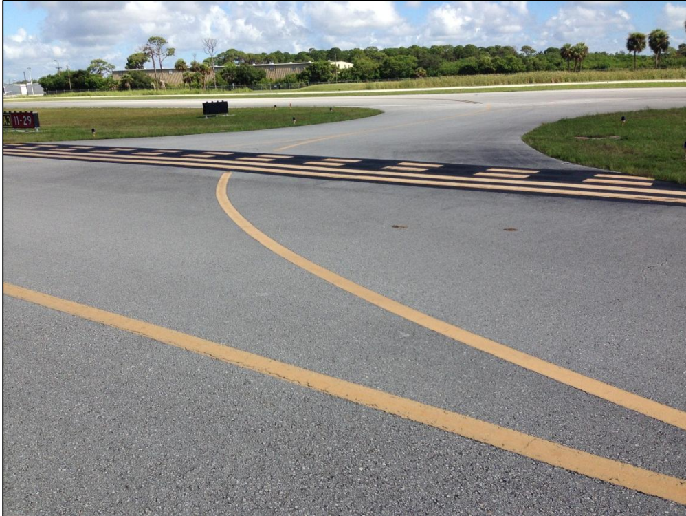
Taxiway A, Section 105, Sample Unit 115 – Low Severity (48) Longitudinal and Transverse Cracking, Low Severity (57) Weathering
