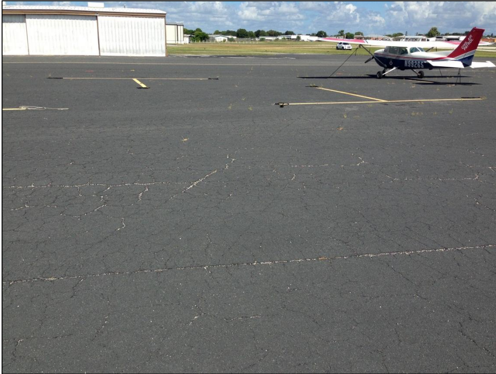
Apron S, Section 4115, Sample Unit 406 –Medium Severity (43) Block Cracking, Medium Severity (52) Raveling
