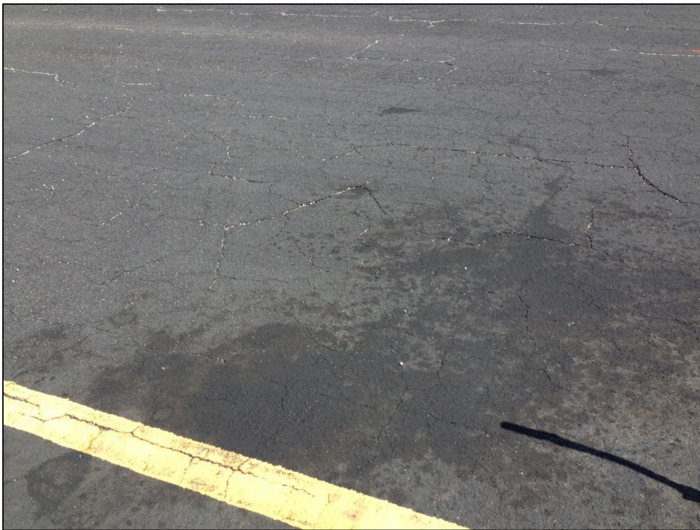
Apron S, Section 4105, Sample Unit 201 –Medium Severity (43) Block Cracking, Medium Severity (52) Raveling, Oil Spillage (49)
