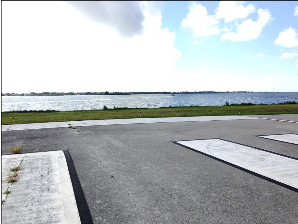
Runway 11-29, Section 6105, Sample Unit 167 – Low Severity (48) Longitudinal and Transverse Cracking, Low Severity (57) Weathering, Low Severity (52) Raveling
