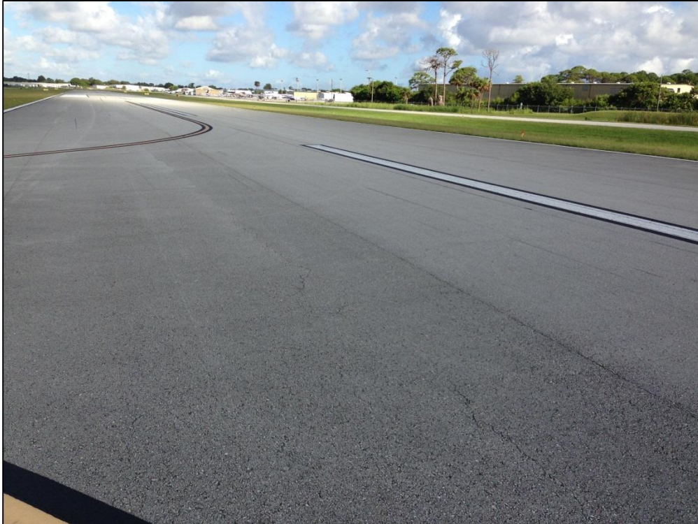
Runway 11-29, Section 6105, Sample Unit 103 – Low Severity (48) Longitudinal and Transverse Cracking, Low Severity (57) Weathering, Low Severity (52) Raveling
