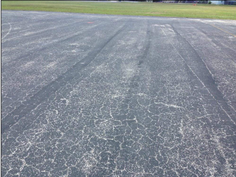
Apron N, Section 4205, Sample Unit 197 – Medium Severity (43) Block Cracking, Medium Severity (52) Raveling
