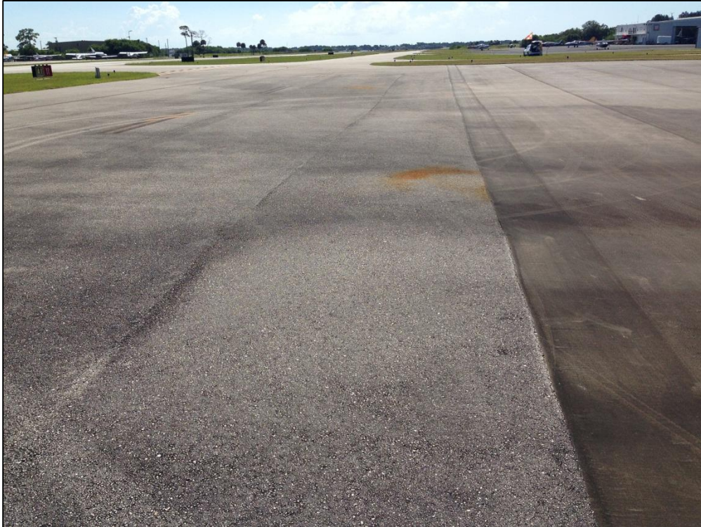
Apron SW, Section 4310, Sample Unit 101 – Low Severity (48) Longitudinal and Transverse Cracking, Low Severity (57) Weathering
