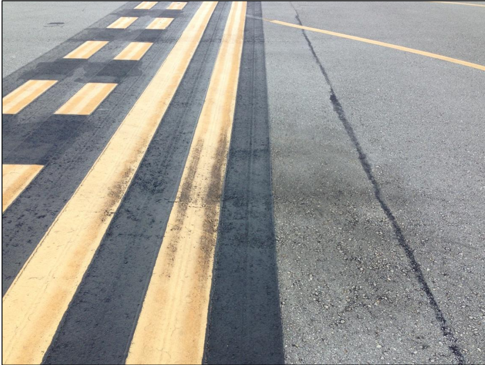
Taxiway A, Section 110, Sample Unit 101 – Low Severity (48) Longitudinal and Transverse Cracking, Low Severity (45) Depression, Low Severity (52) Raveling
