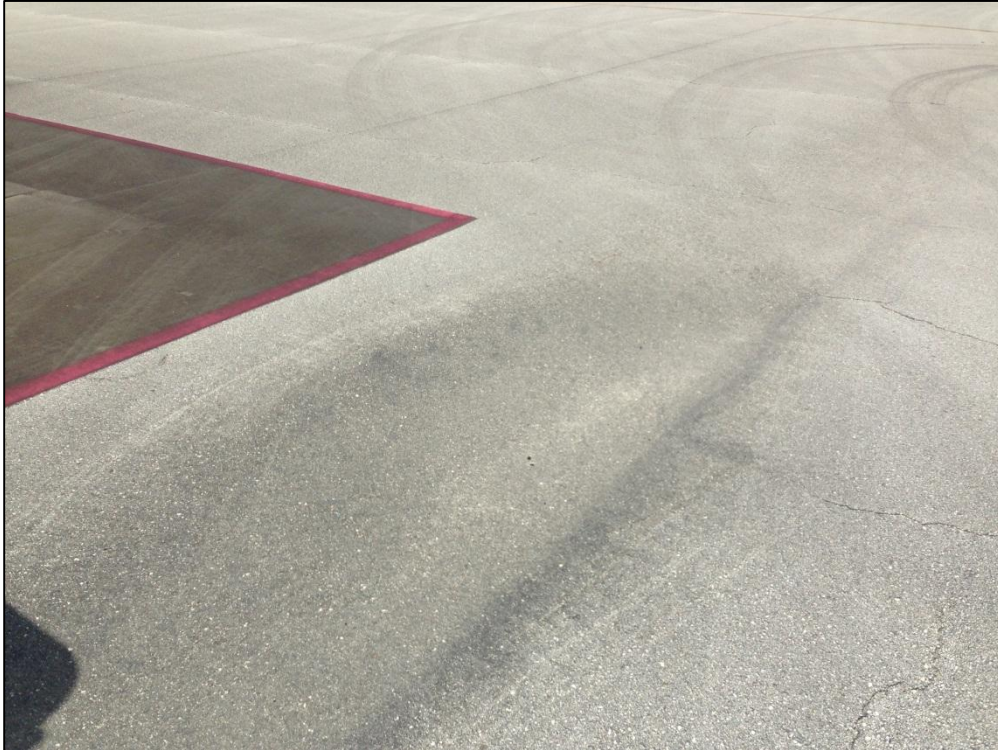
Apron N, Section 4215, Sample Unit 355 – Low Severity (48) Longitudinal and Transverse Cracking, Low Severity (57) Weathering, Low Severity (45) Depression
