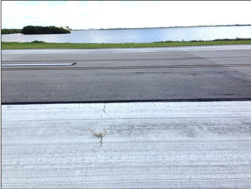
Runway 11-29, Section 6105, Sample Unit 149 – Low Severity (48) Longitudinal and Transverse Cracking, Low Severity (57) Weathering, Low Severity (52) Raveling
