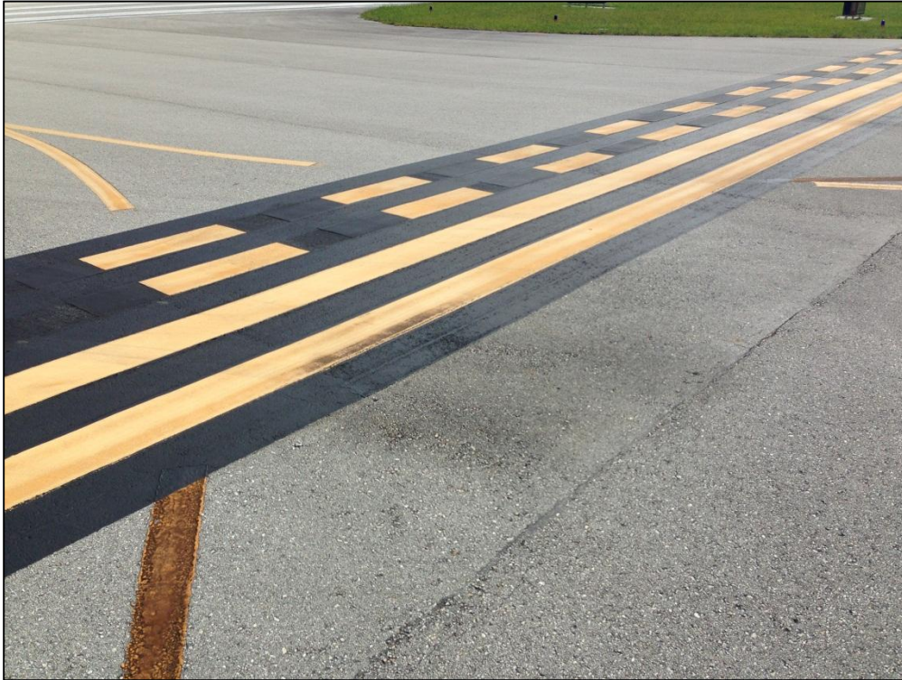
Taxiway A1, Section 305, Sample Unit 101 – Low Severity (48) Longitudinal and Transverse Cracking, Low Severity (45) Depression, Low Severity (57) Weathering
