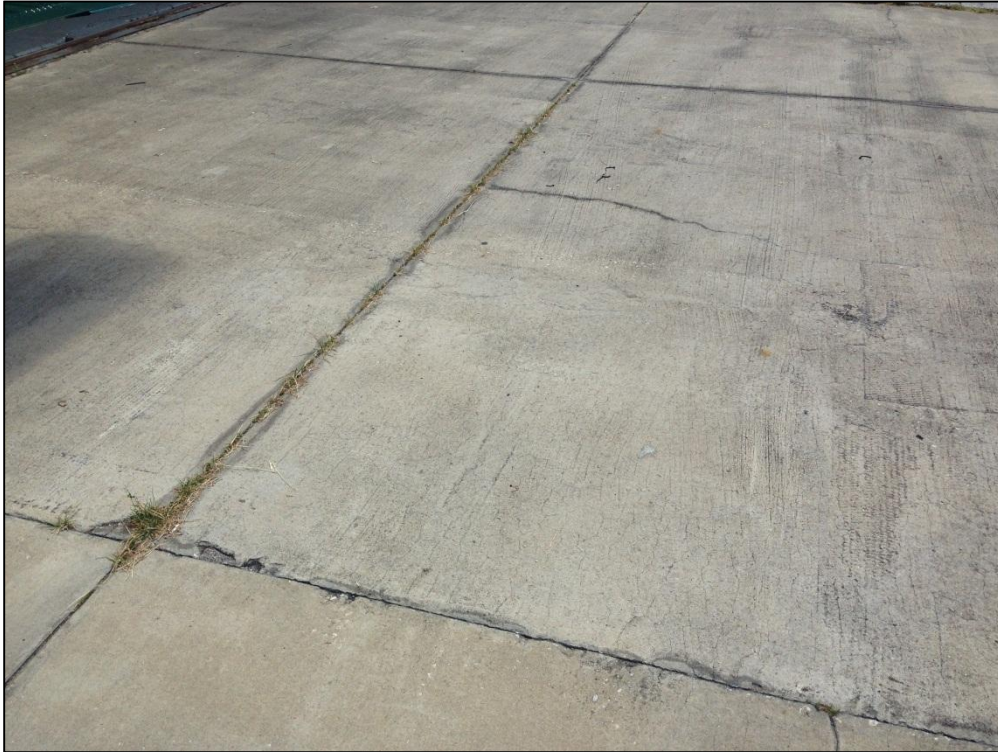
Apron N, Section 4203, Sample Unit 100 – Low Severity (70) Scaling, Map Cracking, Crazing, Low Severity (74) Joint Spalling, Shrinkage Cracking (73)
