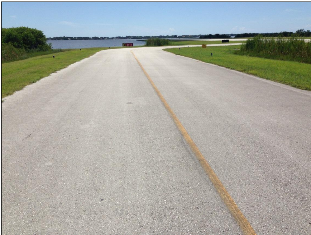
Taxiway B, Section 210, Sample Unit 123 – Low Severity (57) Weathering, Low Severity (52) Raveling
