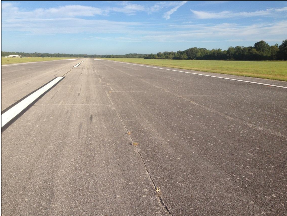
Runway 13-31, Section 6105, Sample Unit 192 – Low and Medium Severity (48) Longitudinal and Transverse Cracking, Low Severity (57) Weathering, Low Severity (52) Raveling
