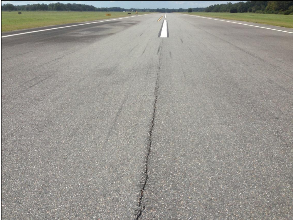
Runway 4-22, Section 6210, Sample Unit 180 – Medium Severity (48) Longitudinal and Transverse Cracking, Low Severity (52) Raveling, Low Severity (57) Weathering
