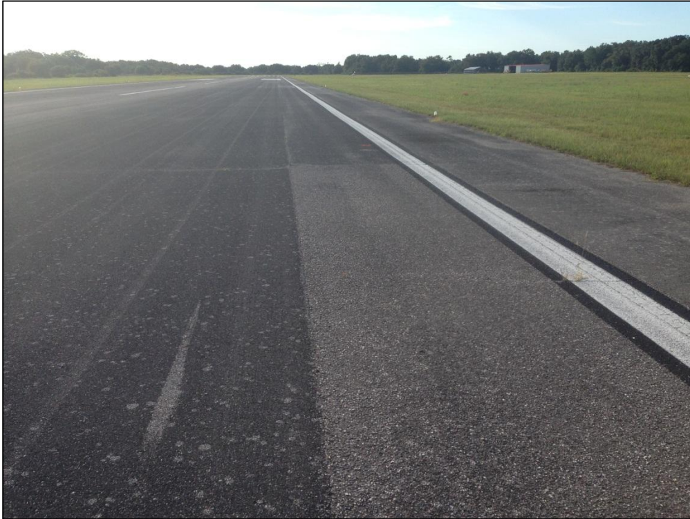
Runway 13-31, Section 6105, Sample Unit 164 – Low, Medium, and High Severity (52) Raveling
