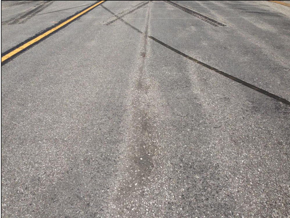
Runway 4-22, Section 6205, Sample Unit 100 – Low Severity (48) Longitudinal and Transverse Cracking, Low, Medium, and High Severity (52) Raveling
