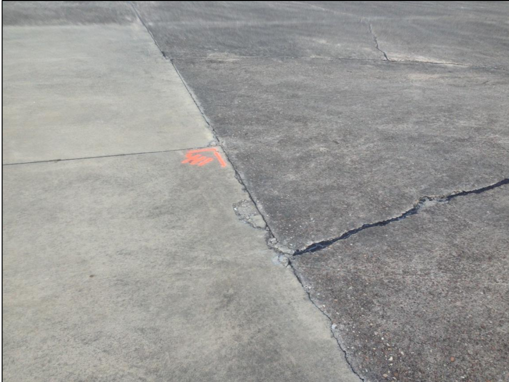
Apron, Section 4110, Sample Unit 411 – Low Severity (65) Joint Seal Damage, High Severity (74) Joint Spalling
