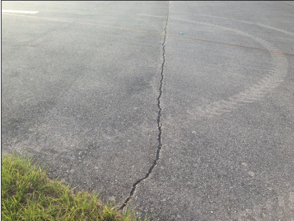
Taxiway A, Section 175, Sample Unit 101 – High Severity (48) Longitudinal and Transverse Cracking, Low Severity (52) Raveling, Low Severity (57) Weathering
