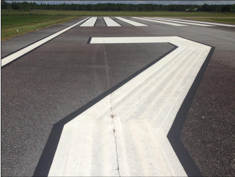
Runway 4-22, Section 6210, Sample Unit 201 – Low Severity (48) Longitudinal and Transverse Cracking, Low Severity (52) Raveling, Low Severity (57) Weathering
