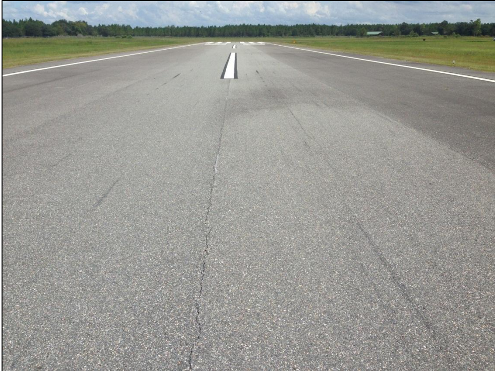
Runway 4-22, Section 6210, Sample Unit 192 – Low Severity (48) Longitudinal and Transverse Cracking, Low Severity (52) Raveling, Low Severity (57) Weathering
