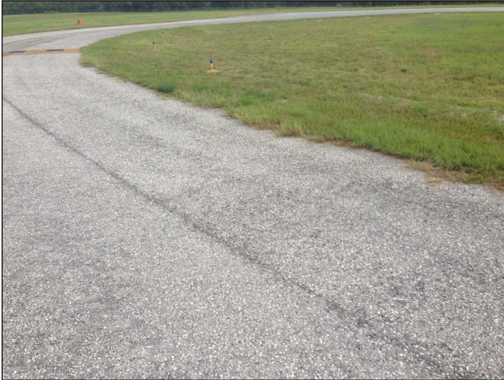
Taxiway A, Section 105, Sample Unit 102 – Low Severity (48) Longitudinal and Transverse Cracking, Medium Severity (52) Raveling
