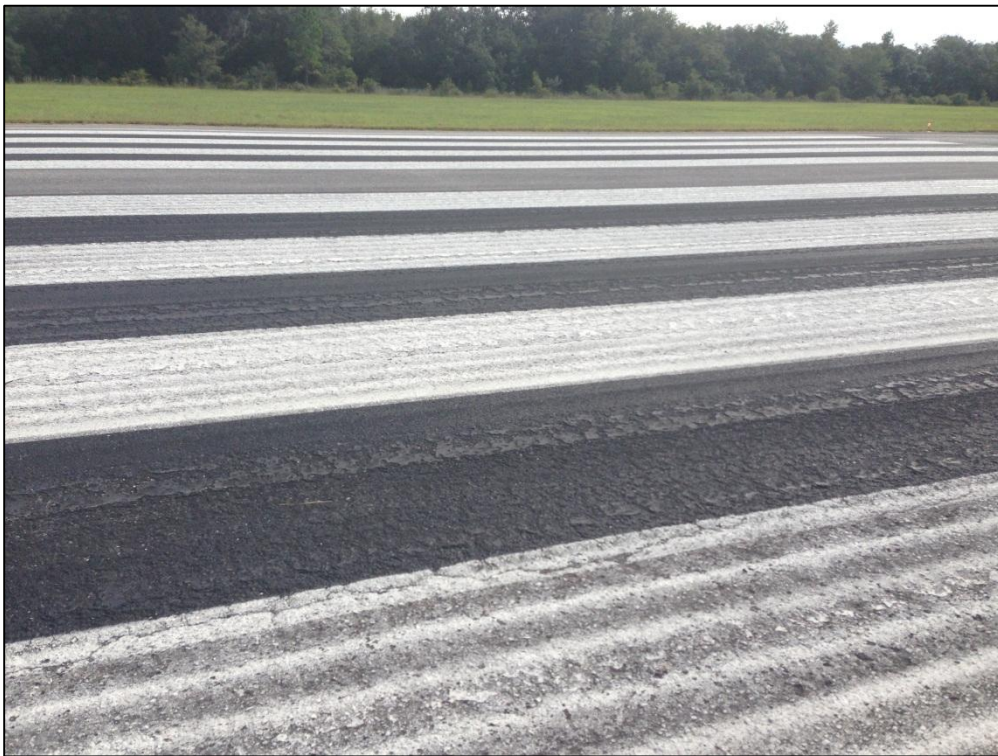
Runway 13-31, Section 6105, Sample Unit 101 – Medium and High Severity (52) Raveling
