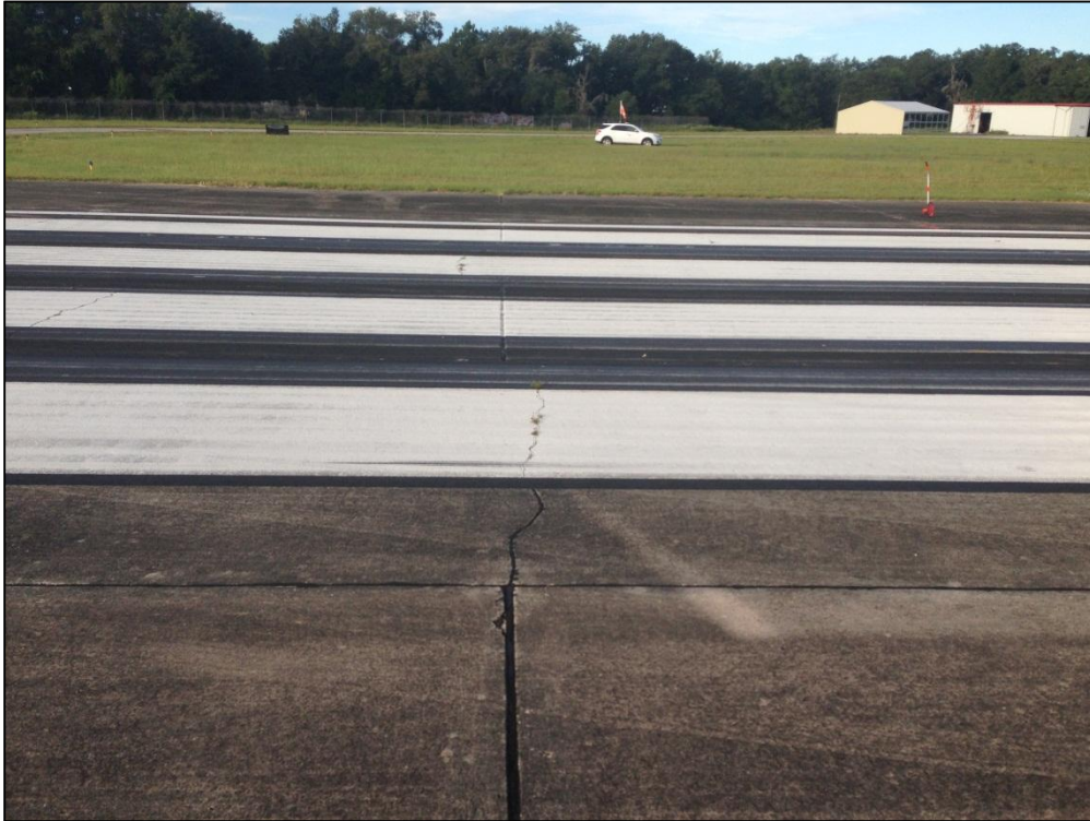
Runway 13-31, Section 6110, Sample Unit 196 – Medium Severity (65) Joint Seal Damage, Low Severity (63) Longitudinal, Transverse, and Diagonal Cracking
