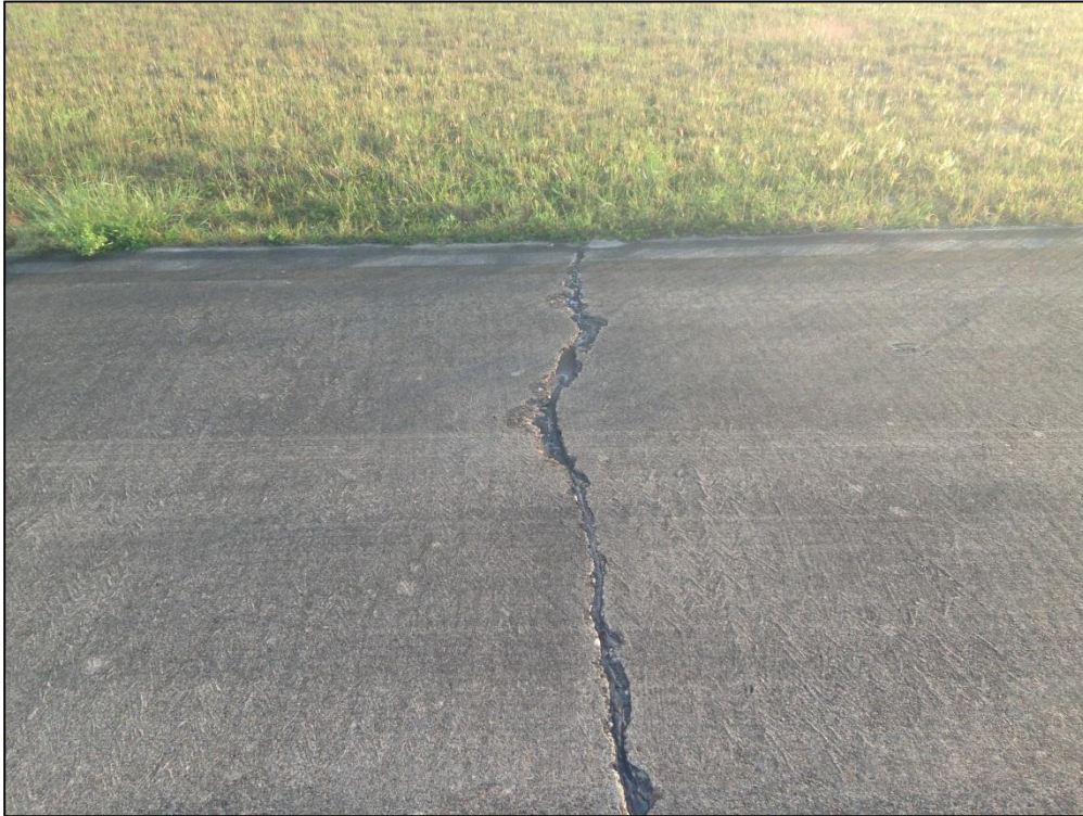
Apron, Section 4105, Sample Unit 407 – Low Severity (65) Joint Seal Damage, Medium Severity (63) Longitudinal, Transverse, and Diagonal Cracking
