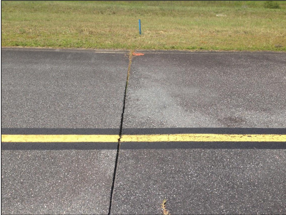
Taxiway B, Section 207, Sample Unit 103 – High Severity (48) Longitudinal and Transverse Cracking, Low Severity (52) Raveling, Low Severity (57) Weathering
