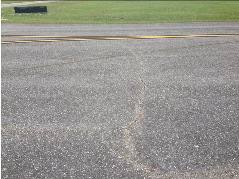
Taxiway A2, Section 160, Sample Unit 102 – Low and Medium Severity (48) Longitudinal and Transverse Cracking, Low and Medium Severity (52) Raveling
