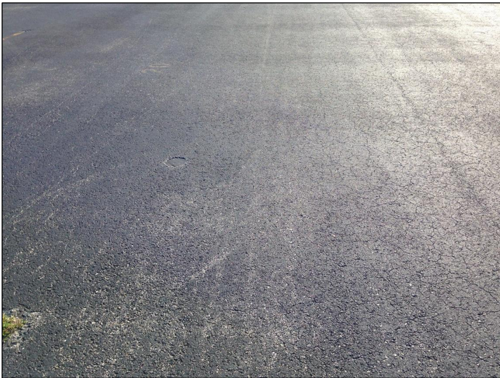
Apron S, Section 4205, Sample Unit 300 – Low Severity (43) Block Cracking, Low Severity (57) Weathering
