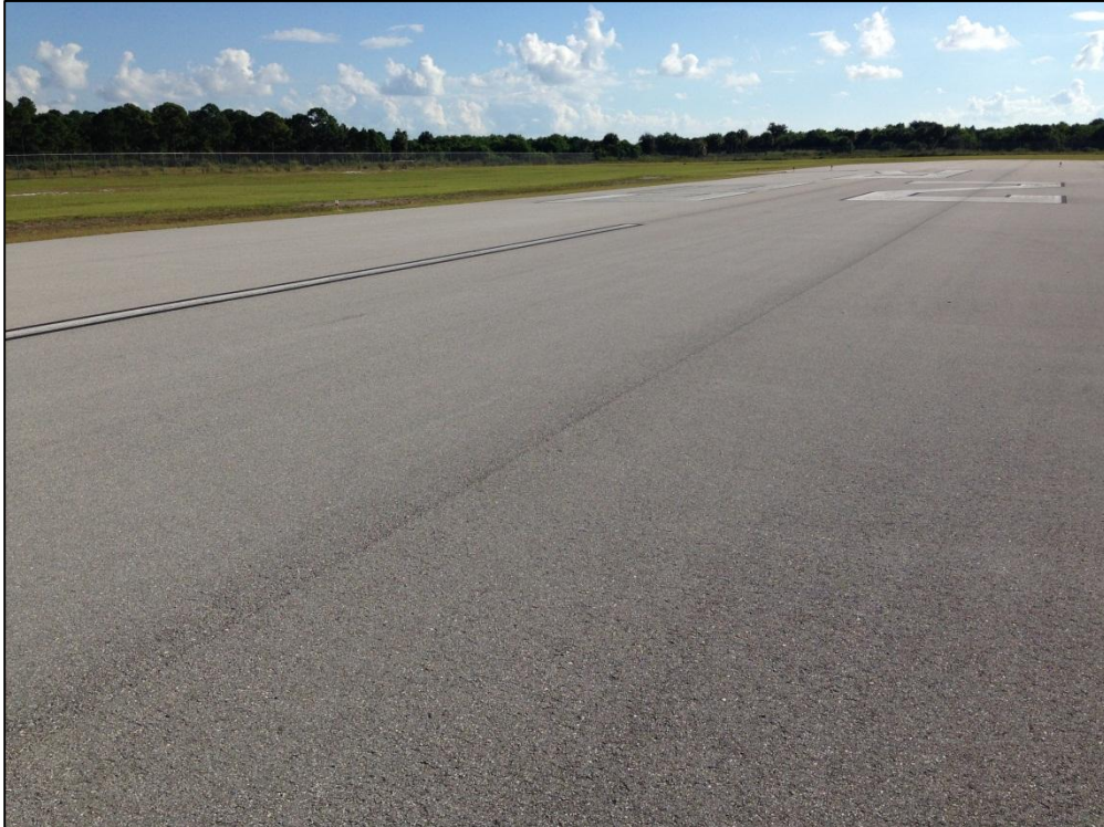
Runway 10L-28R, Section 6305, Sample Unit 174 – Low Severity (57) Weathering
