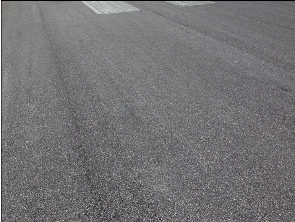
Runway 14-32, Section 6205, Sample Unit 103 – Low Severity (48) Longitudinal and Transverse Cracking, Low Severity (56) Swelling, Low Severity (57) Weathering
