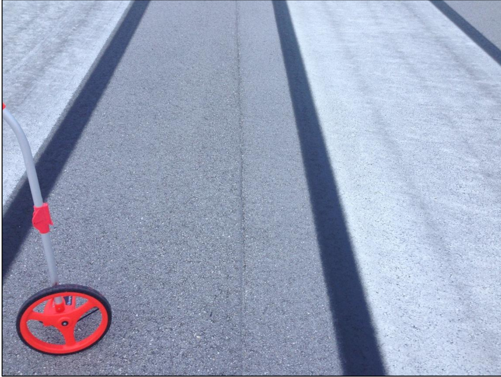
Runway 10R-28L, Section 6130, Sample Unit 163 – Low Severity (48) Longitudinal and Transverse Cracking, Low Severity (57) Weathering
