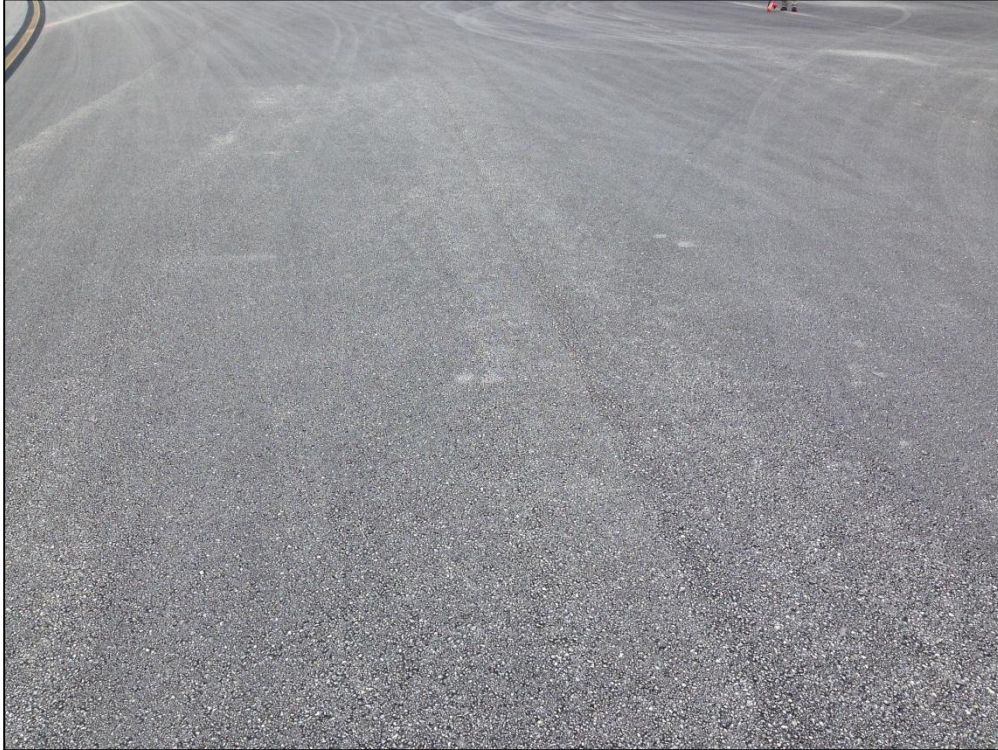
Taxiway A1, Section 140, Sample Unit 107 – Low Severity (57) Weathering
