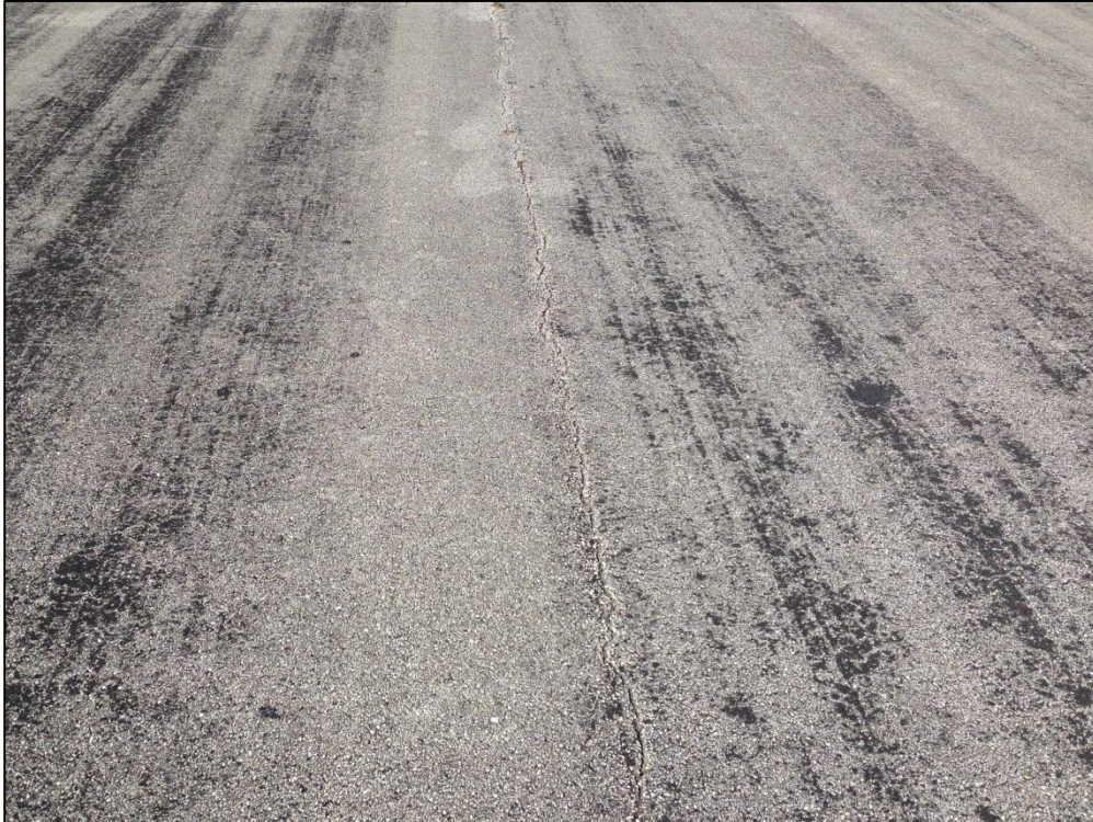
Apron SE, Section 4310, Sample Unit 801 – Medium Severity (48) Longitudinal and Transverse Cracking, Low Severity (56) Swelling, Low and Medium Severity (57) Weathering
