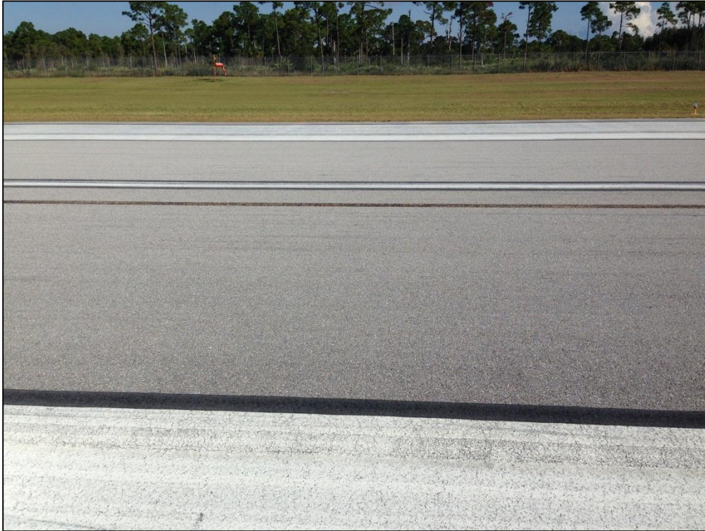
Runway 10L-28R, Section 6305, Sample Unit 122 – Low Severity (57) Weathering
