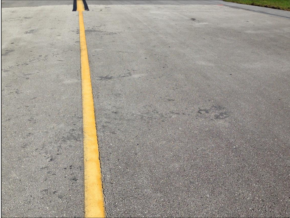
Taxiway B, Section 207, Sample Unit 122 – Low Severity (48) Longitudinal and Transverse Cracking, Low Severity (56) Swelling, Low Severity (57) Weathering
