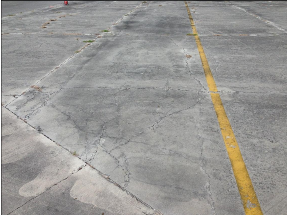
Apron Center, Section 4112, Sample Unit 303 – High Severity (65) Joint Seal Damage, High Severity (72) Shattered Slab
