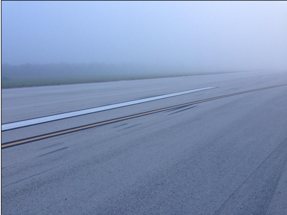
Runway 10R-28L, Section 6105, Sample Unit 342 – Low Severity (57) Weathering
