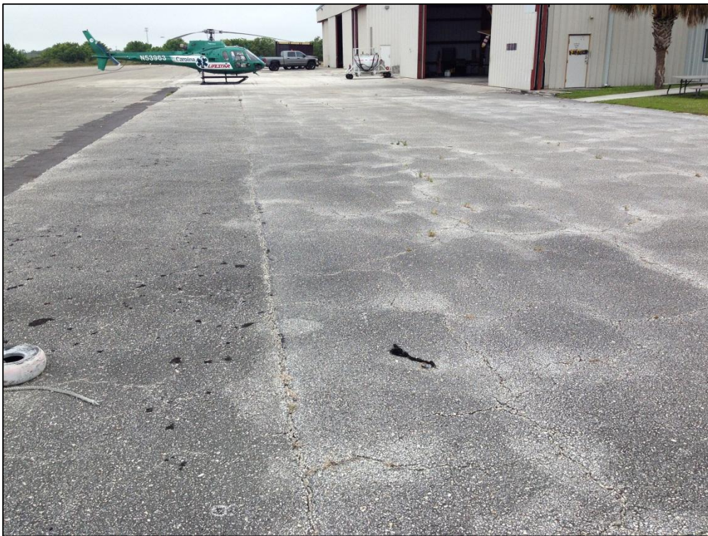
Apron Center, Section 4127, Sample Unit 98 – Low Severity (43) Block Cracking, Low Severity (52) Raveling, Low Severity (57) Weathering
