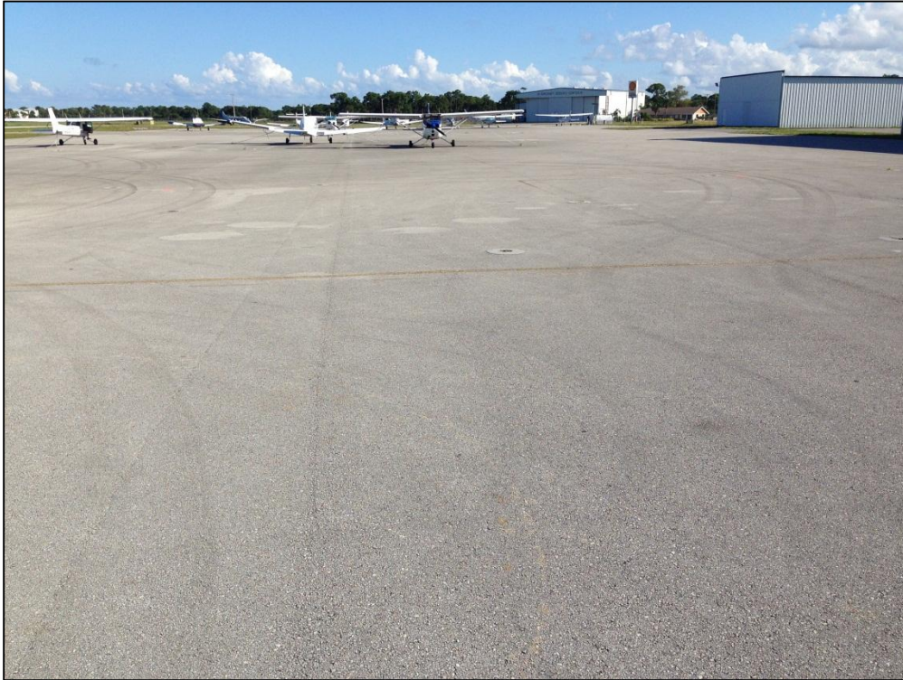
Apron S, Section 4240, Sample Unit 300 – Low Severity (57) Weathering
