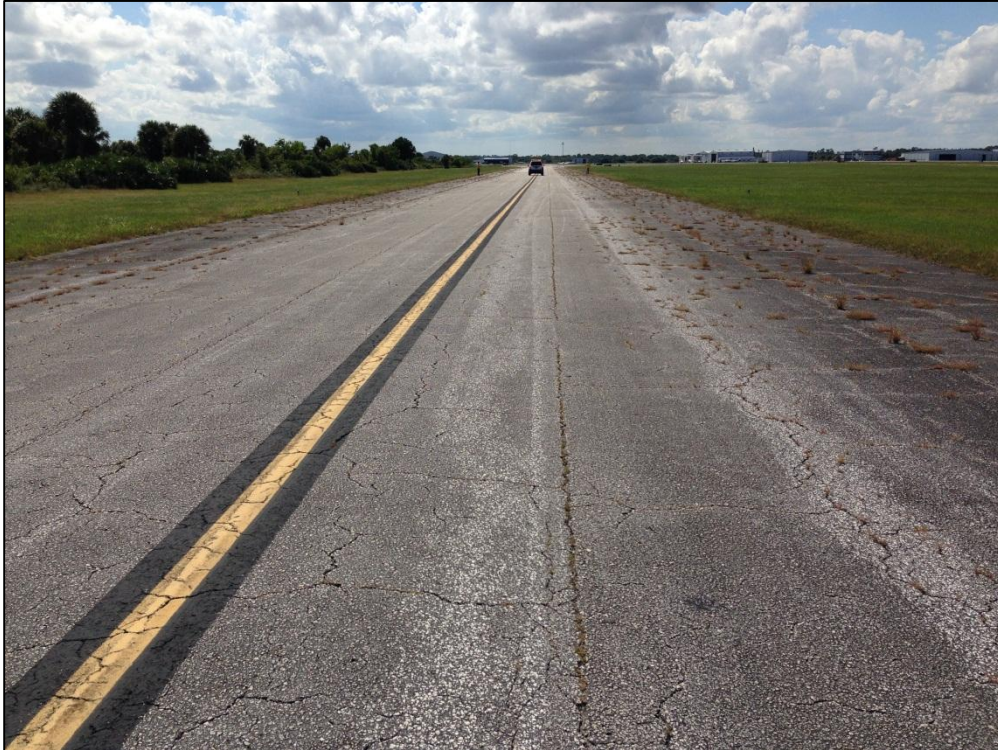
Taxiway D, Section 315, Sample Unit 318 – Medium Severity (43) Block Cracking, Low Severity (52) Raveling, Low Severity (57) Weathering
