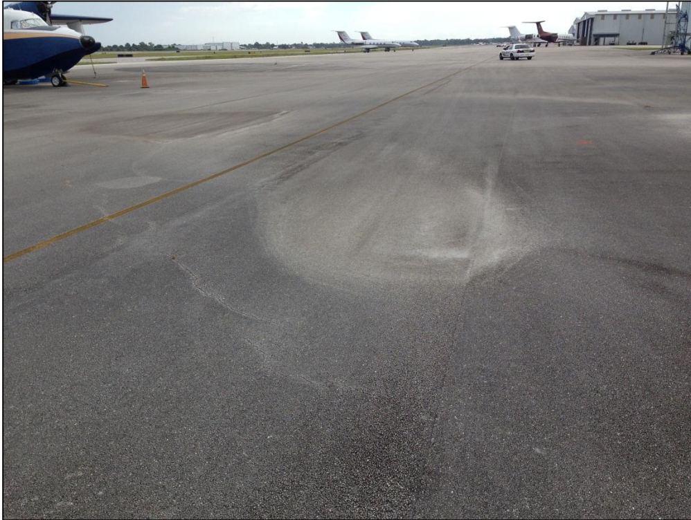
Apron Center, Section 4105, Sample Unit 402 – Low Severity (48) Longitudinal and Transverse Cracking, Medium Severity (45) Depression, Low Severity (56) Swelling, Low Severity (57) Weathering
