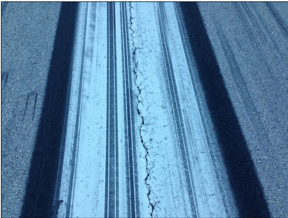
Runway 10R-28L, Section 6105, Sample Unit 350 – Low Severity (48) Longitudinal and Transverse Cracking, Low Severity (57) Weathering
