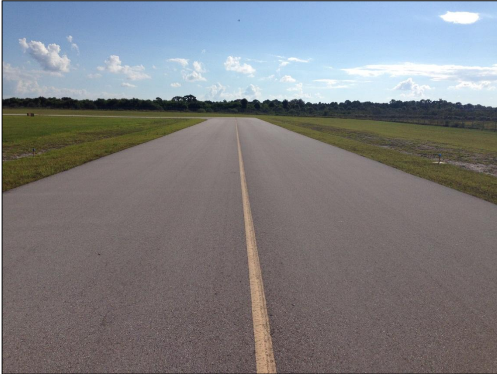
Taxiway F, Section 810, Sample Unit 636 – Low Severity (57) Weathering
