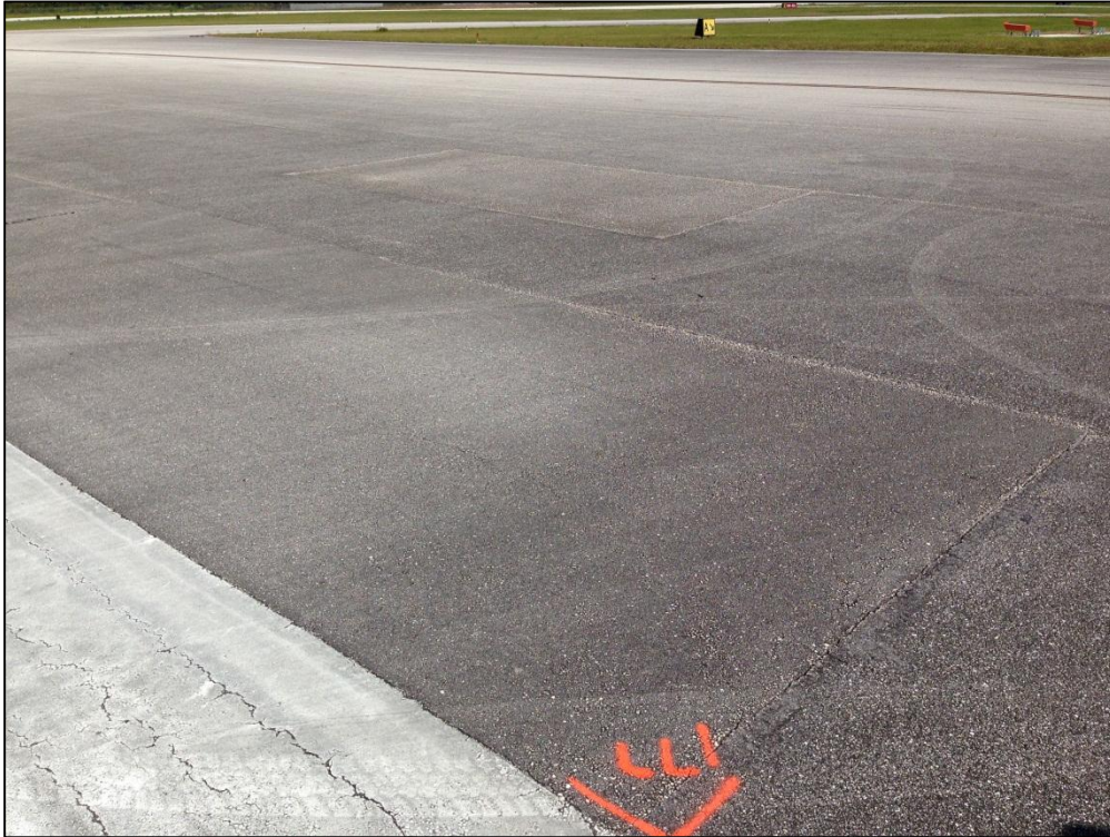
Runway 14-32, Section 6205, Sample Unit 177 – Low Severity (48) Longitudinal and Transverse Cracking, Low Severity (50) Patching, Low Severity (57) Weathering
