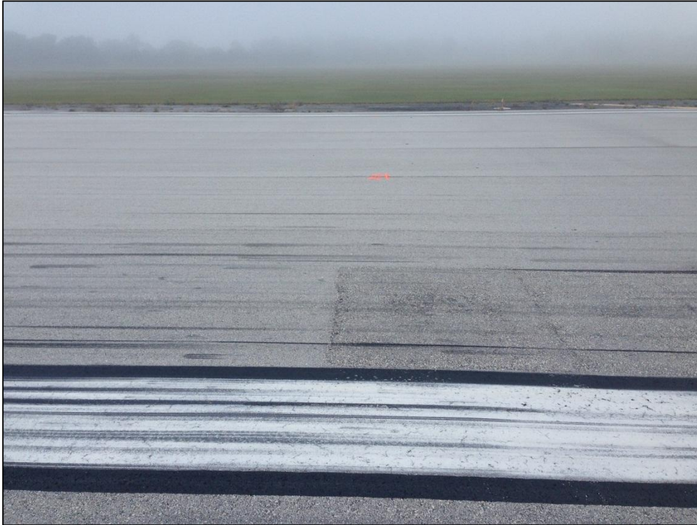
Runway 10R-28L, Section 6105, Sample Unit 316 – Low Severity (50) Patching, Low Severity (57) Weathering
