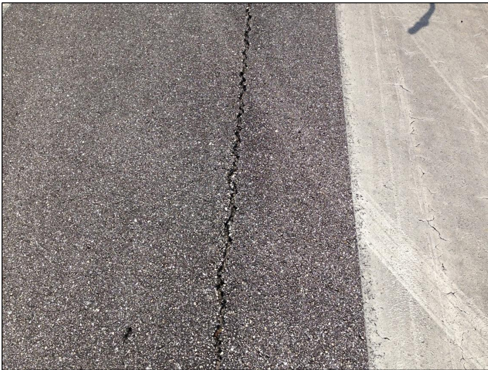
Runway 14-32, Section 6205, Sample Unit 184 – Medium Severity (48) Longitudinal and Transverse Cracking, Low Severity (57) Weathering
