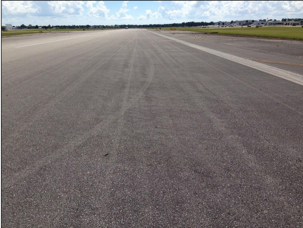
Runway 14-32, Section 6205, Sample Unit 149 – Low Severity (48) Longitudinal and Transverse Cracking, Low Severity (57) Weathering
