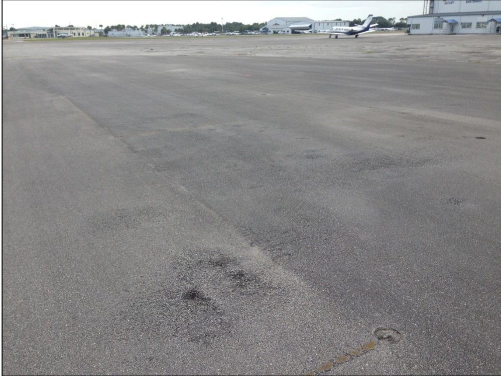
Apron Center, Section 4115, Sample Unit 301 – Low Severity (45) Depression, Low Severity (48) Longitudinal and Transverse Cracking, Low Severity (52) Raveling, Low Severity (57) Weathering
