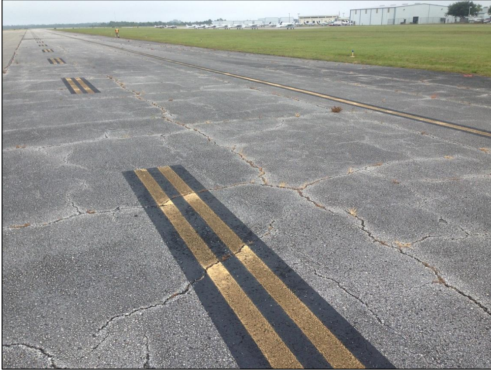
Taxiway E, Section 605, Sample Unit 618 – Medium Severity (43) Block Cracking, Low Severity (52) Raveling, Low Severity (57) Weathering
