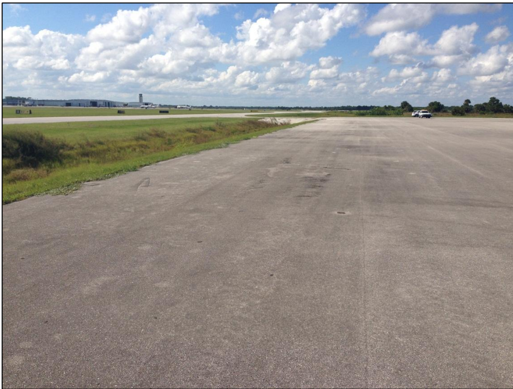
Apron E, Section 4405, Sample Unit 503 – Low Severity (48) Longitudinal and Transverse Cracking, Low and Medium Severity (57) Weathering, Low Severity (56) Swelling
