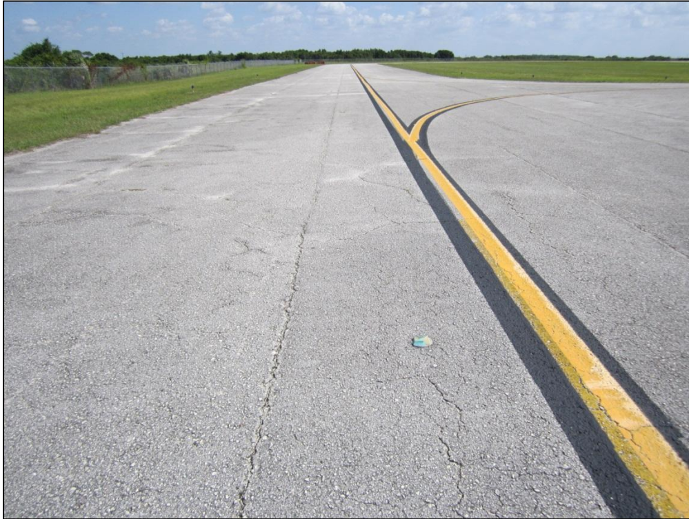
Taxiway Alpha, Section 205, Sample Unit 143 –Low and Medium Severity (43) Block Cracking, Medium Severity (52) Raveling
