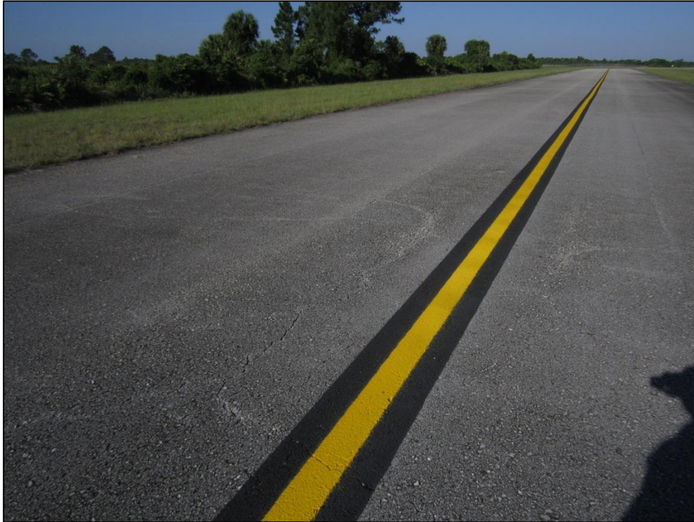
Taxiway Bravo, Section 110, Sample Unit 110 –Medium Severity (43) Block Cracking, Low Severity (48) Longitudinal and Transverse Cracking, Low Severity (52) Raveling, Low Severity (57) Weathering
