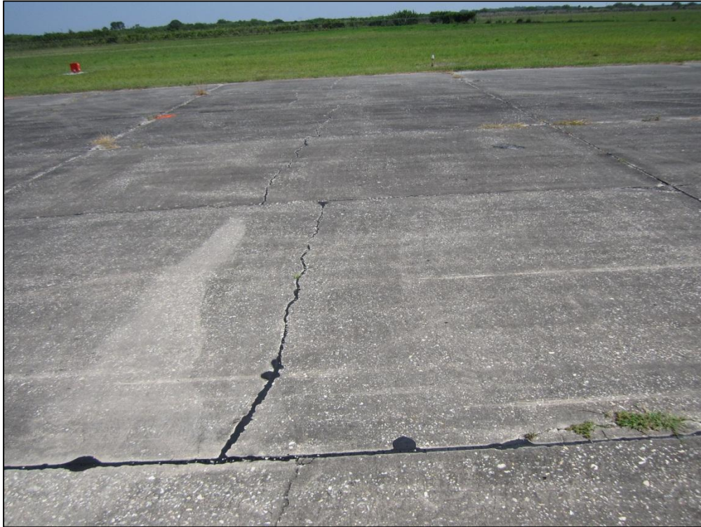
Runway 9-27, Section 6205, Sample Unit 301 – Medium Severity (63) Longitudinal, Transverse and Diagonal Cracking, Medium Severity (74) Joint Spalling, Medium Severity (65) Joint Seal Damage
