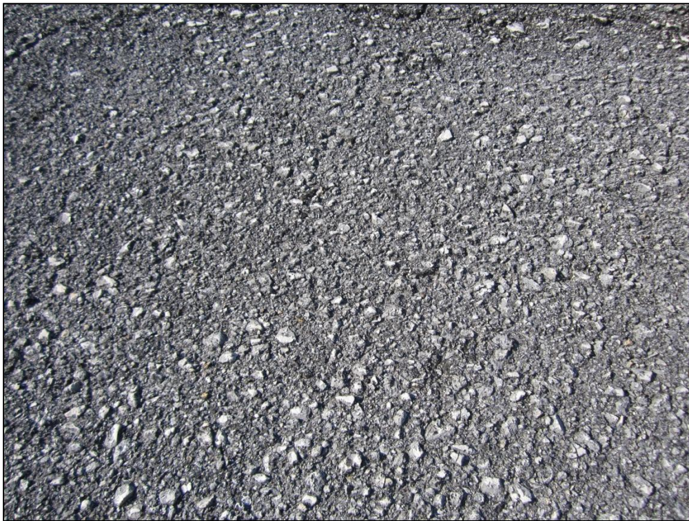
Runway 9-27, Section 6220, Sample Unit 576 –Medium Severity (52) Raveling
