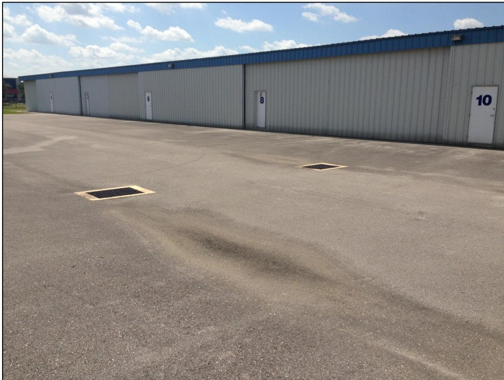
Apron Hangar, Section 4405, Sample Unit 200 – Low Severity (45) Depression, Low Severity (57) Weathering
