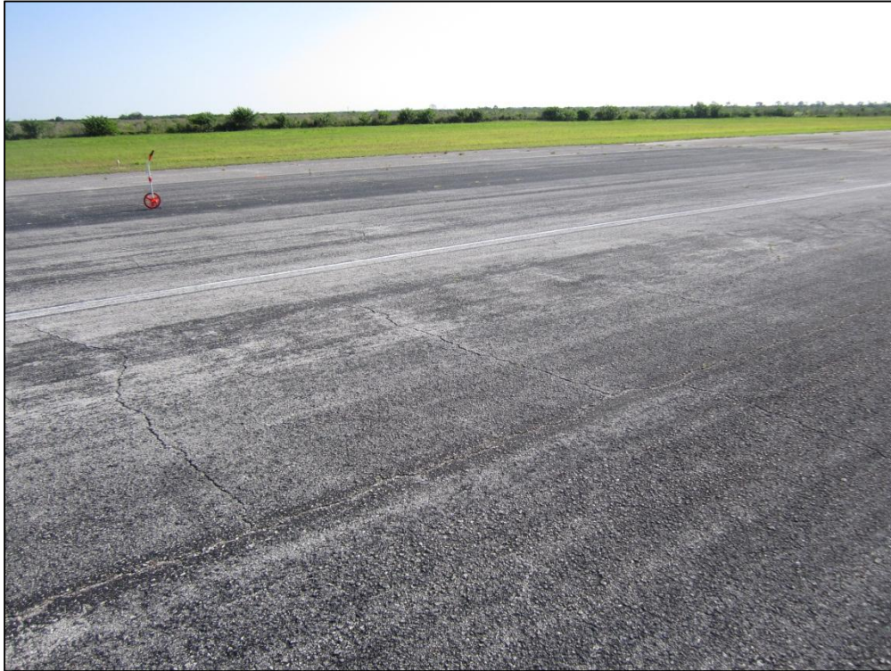
Runway 9-27, Section 6215, Sample Unit 383 – Low and Medium Severity (43) Block Cracking, Medium Severity (52) Raveling
