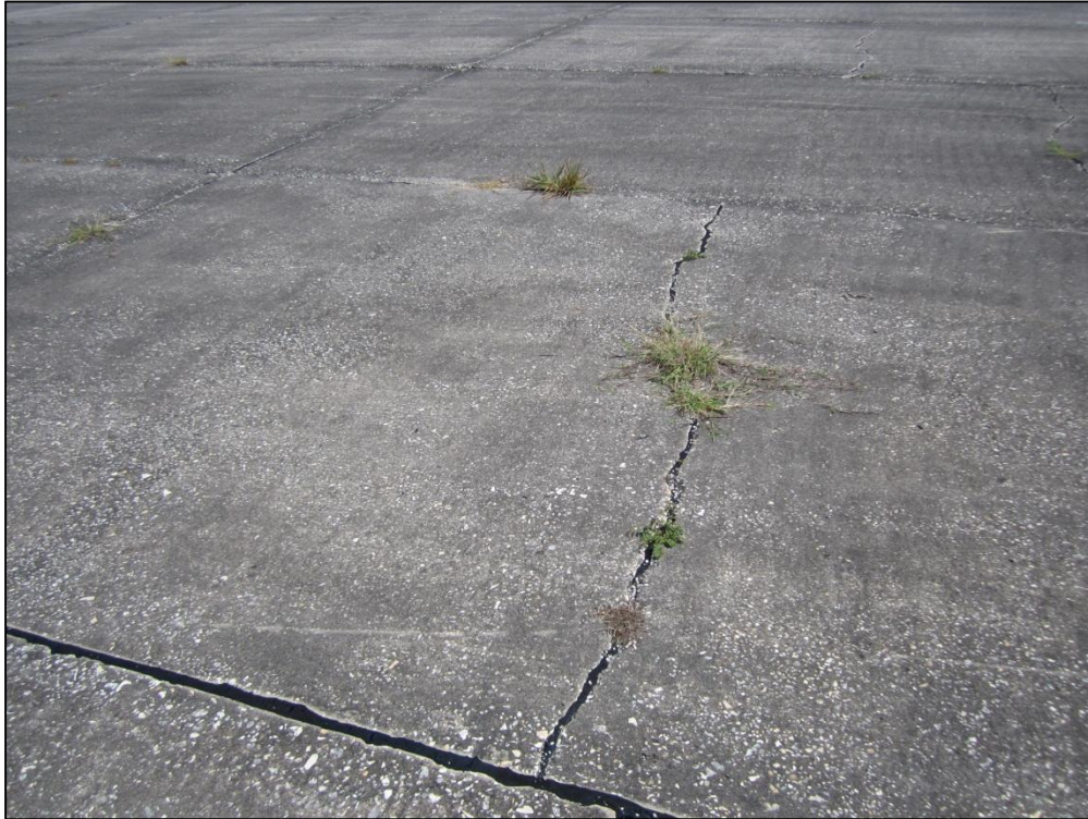
Runway 9-27, Section 6205, Sample Unit 301 –Medium Severity (63) Longitudinal, Transverse and Diagonal Cracking, Medium Severity (65) Joint Seal Damage
