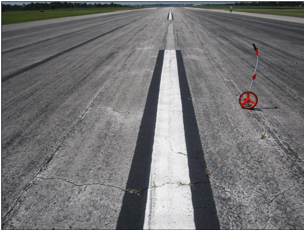
Runway18-36, Section 6115, Sample Unit 386 –Low Severity (43) Block Cracking, Low and Medium Severity (48) Longitudinal and Transverse Cracking, Medium Severity (52) Raveling
