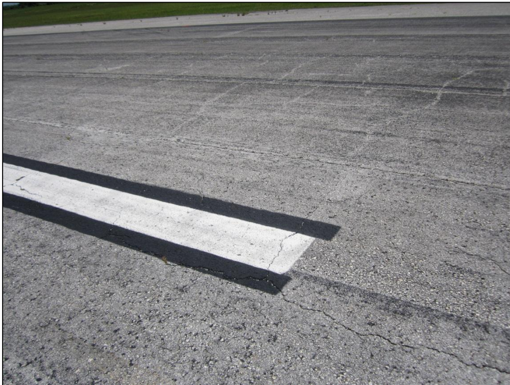
Runway 18-36, Section 6115, Sample Unit 351 – Low Severity (43) Block Cracking, Low and Medium Severity (48) Longitudinal and Transverse Cracking, Medium Severity (52) Raveling
