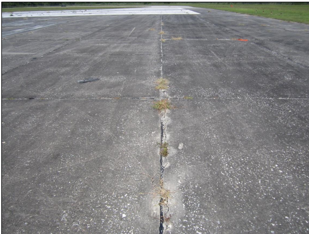
Runway 9-27, Section 6205, Sample Unit 301 –High Severity (74) Joint Spalling, Medium Severity (65) Joint Seal Damage
