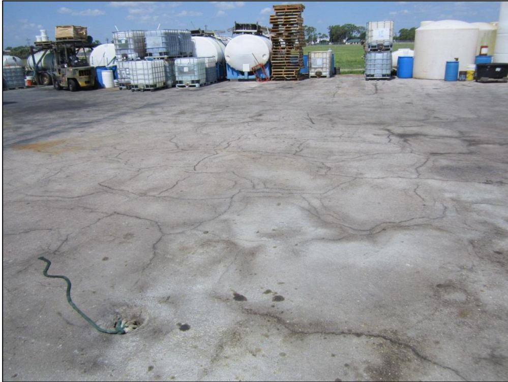
Crop Apron, Section 4105, Sample Unit 201 –Low Severity (43) Block Cracking, Low Severity (48) Longitudinal and Transverse Cracking, Low Severity (52) Raveling, Low Severity (57) Weathering, (49) Oil Spill
