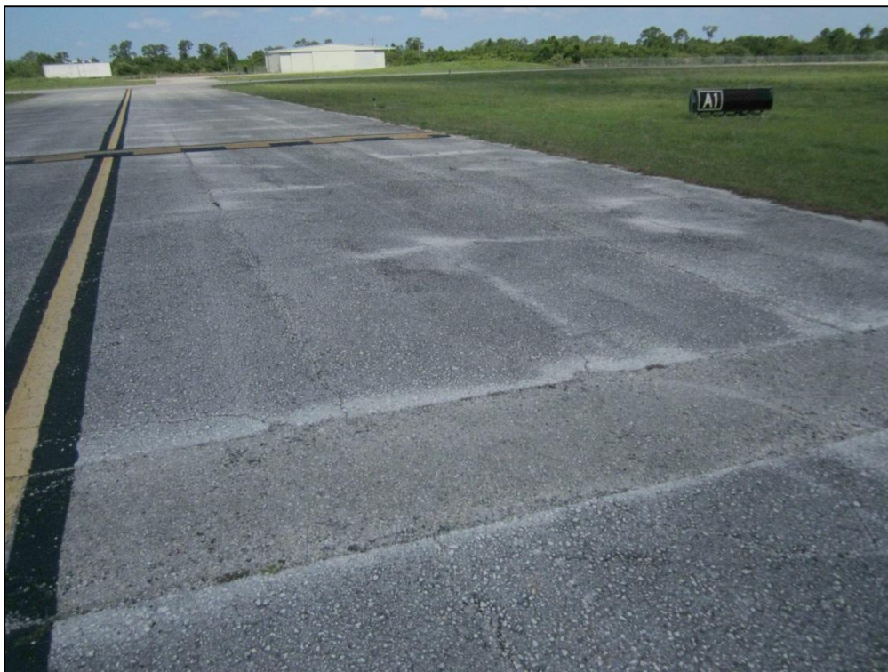
Taxiway Alpha, Section 210, Sample Unit 201 –Medium Severity (43) Block Cracking, High Severity (50) Patch, Medium Severity (52) Raveling
