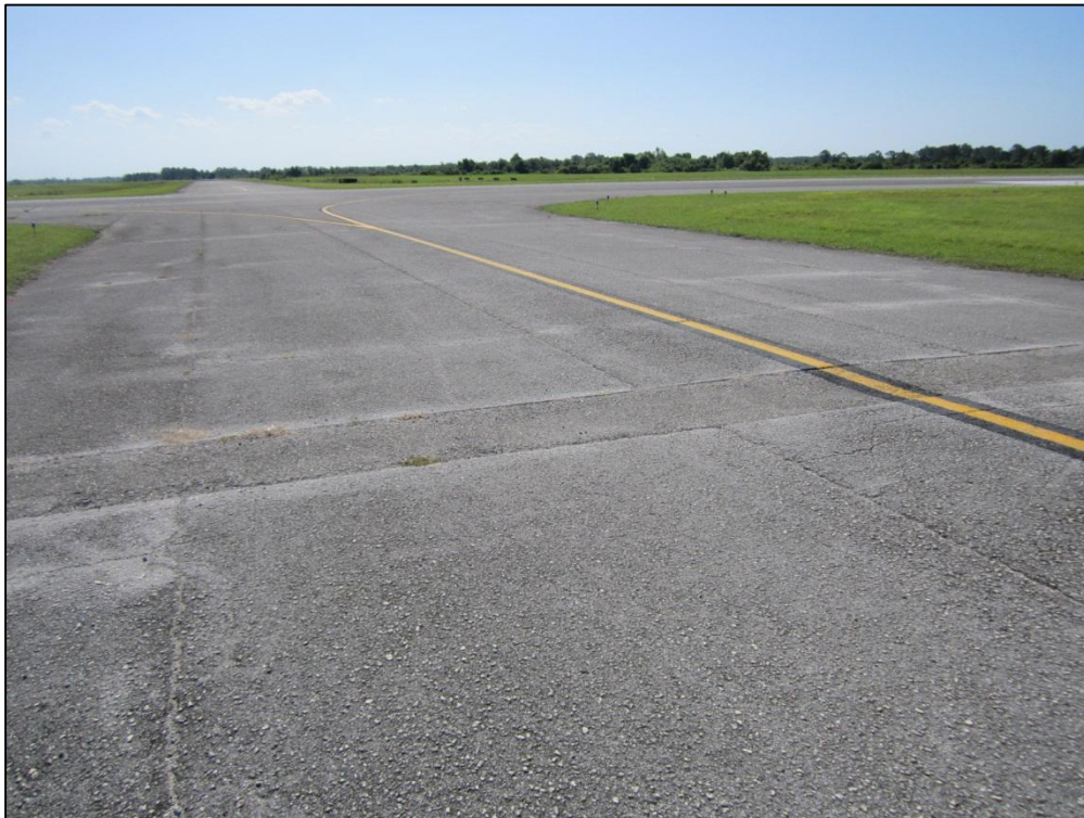
Taxiway A2, Section 220, Sample Unit 301 –Low and Medium Severity (43) Block Cracking, High Severity (50) Patch, Low and Medium Severity (48) Longitudinal and Transverse Cracking, Medium Severity (52) Raveling
