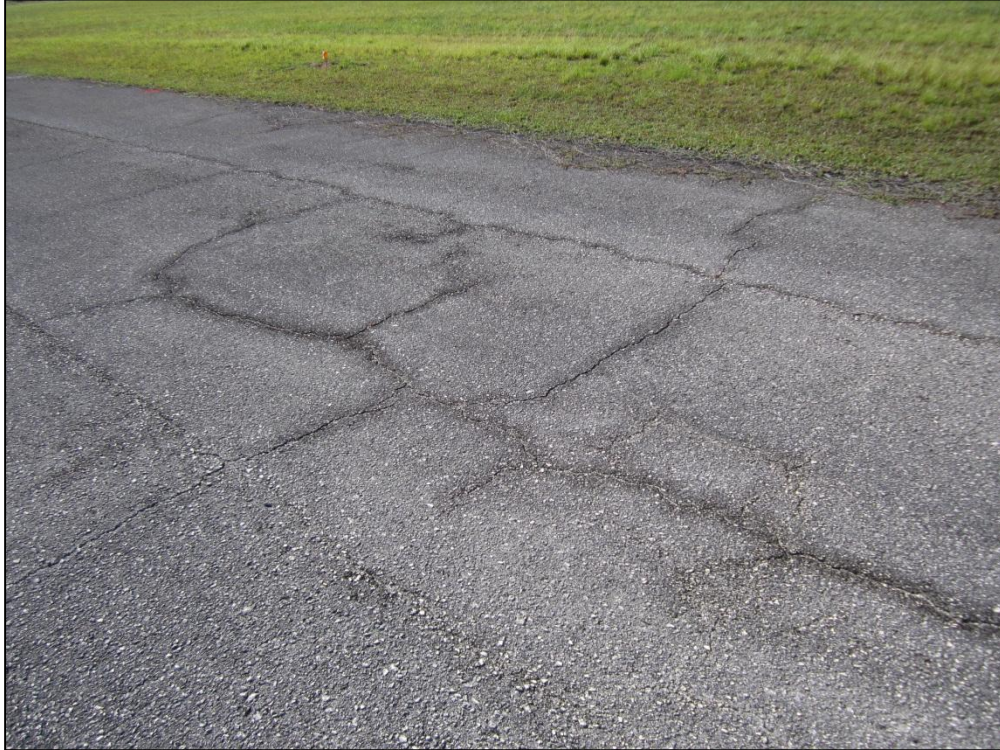
Runway 9-27, Section 6220, Sample Unit 576 – Low and Medium Severity (43) Block Cracking, Medium Severity (52) Raveling
