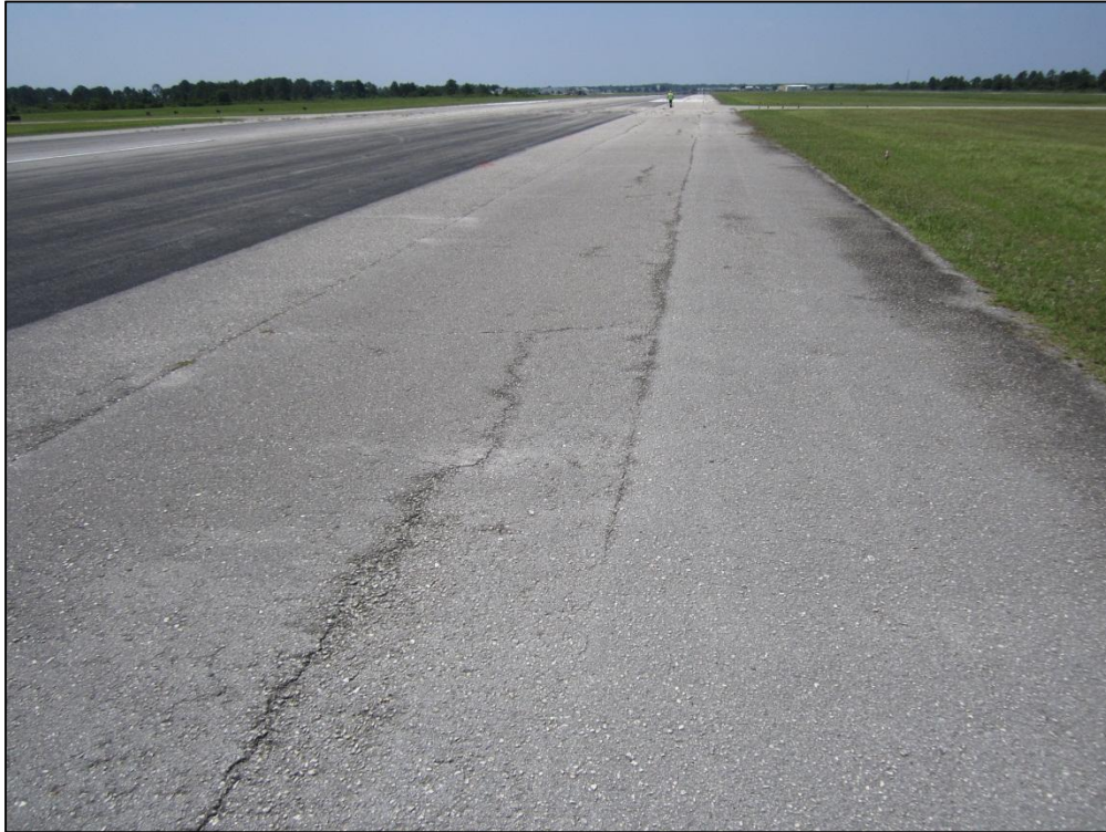
Runway18-36, Section 6120, Sample Unit 182 –Low Severity (48) Longitudinal and Transverse Cracking, Medium Severity (52) Raveling
