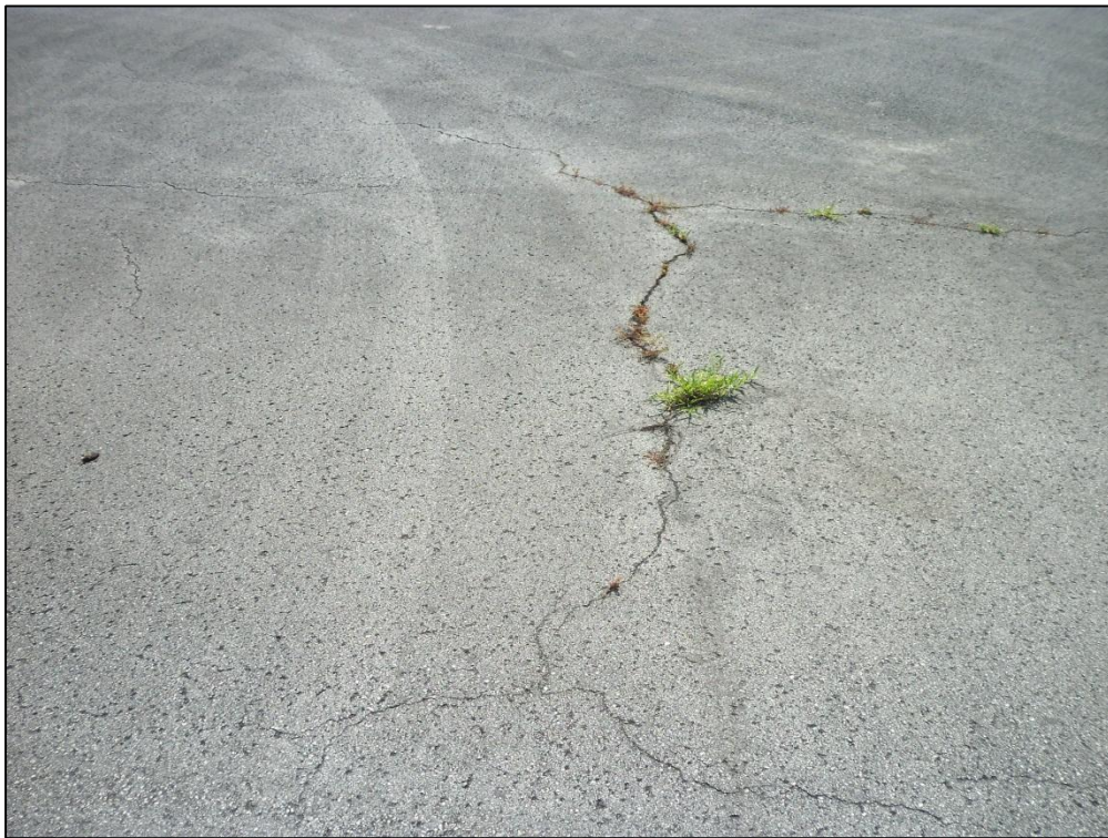
Apron GA, Section 4005, Sample Unit 604 – Low and Medium Severity (48) Longitudinal and Transverse Cracking, Low Severity (52) Raveling, Low Severity (57) Weathering
