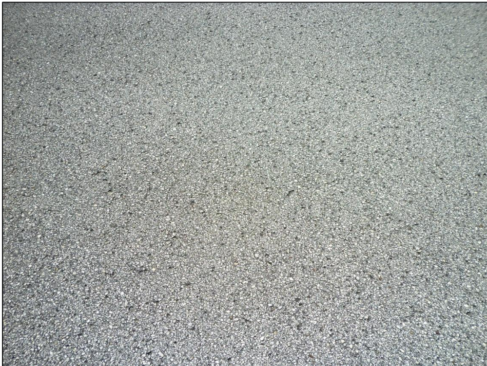
Taxiway GA AP, Section 205, Sample Unit 102 –Low Severity (52) Raveling, Low Severity (57) Weathering
