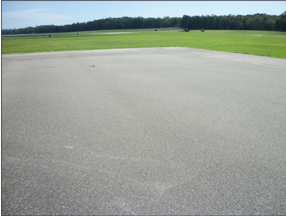
Apron GA, Section 4020, Sample Unit 100 –Low Severity (57) Weathering
