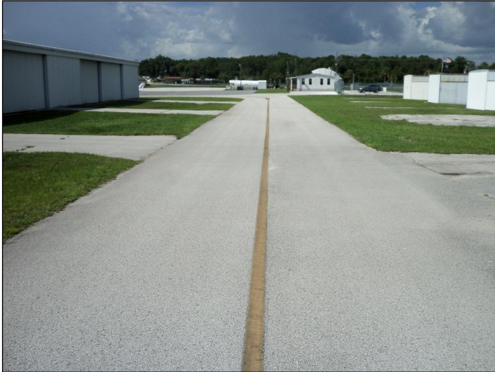
Taxiway GA AP, Section 205, Sample Unit 102 – Low Severity (48) Longitudinal and Transverse Cracking, Low Severity (52) Raveling, Low Severity (57) Weathering
