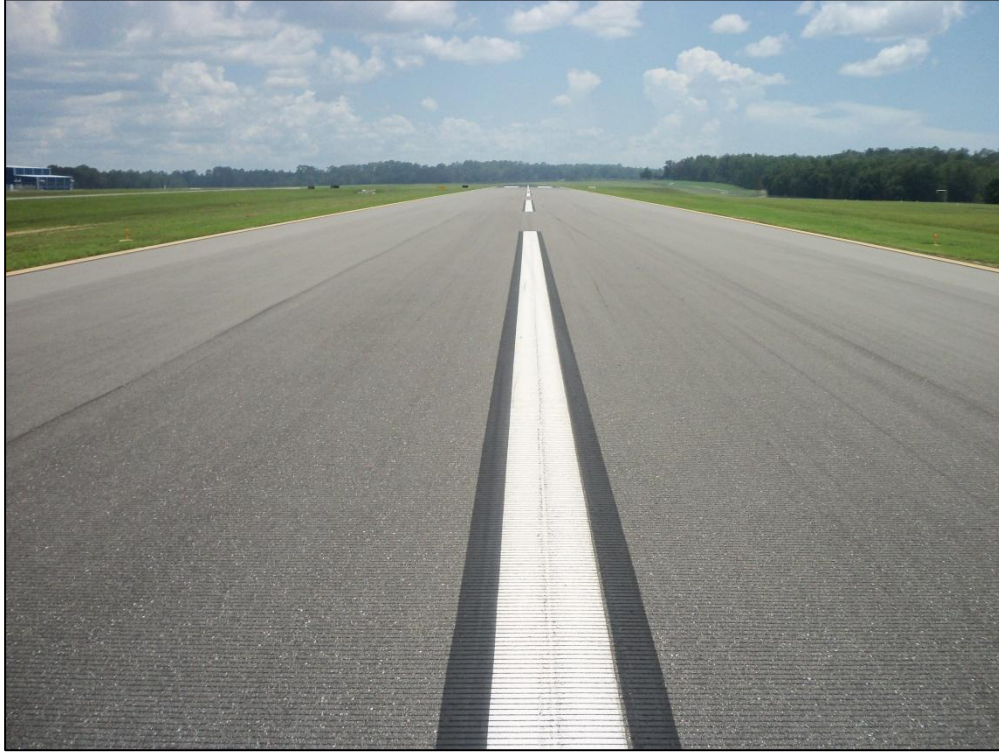
Runway 01-19, Section 6105, Sample Unit 144 – Low Severity (48) Longitudinal and Transverse Cracking
