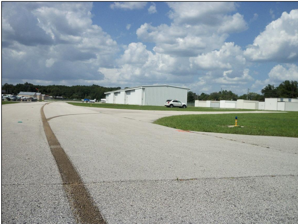
Taxiway GA AP, Section 205, Sample Unit 401 – Low Severity (48) Longitudinal and Transverse Cracking, Low Severity (52) Raveling, Low Severity (57) Weathering, Low Severity (56) Swelling
