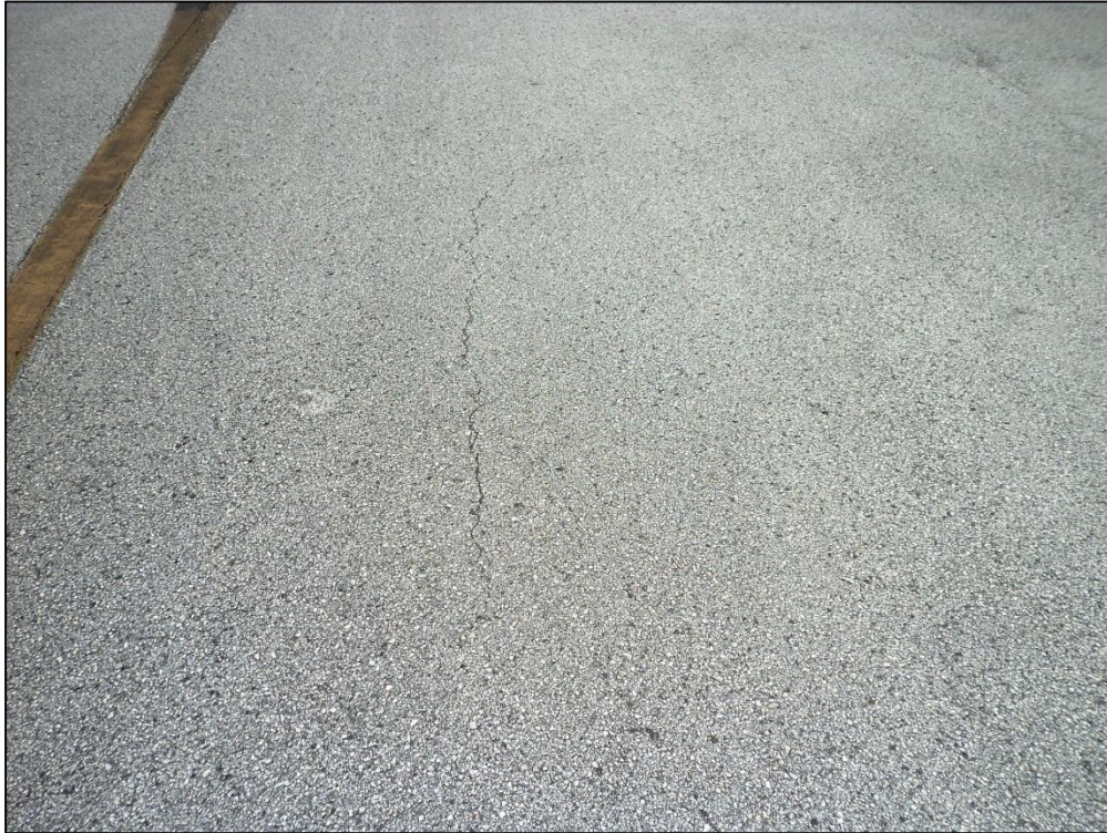
Taxiway GA AP, Section 205, Sample Unit 401 – Low Severity (48) Longitudinal and Transverse Cracking, Low Severity (52) Raveling, Low Severity (57) Weathering
