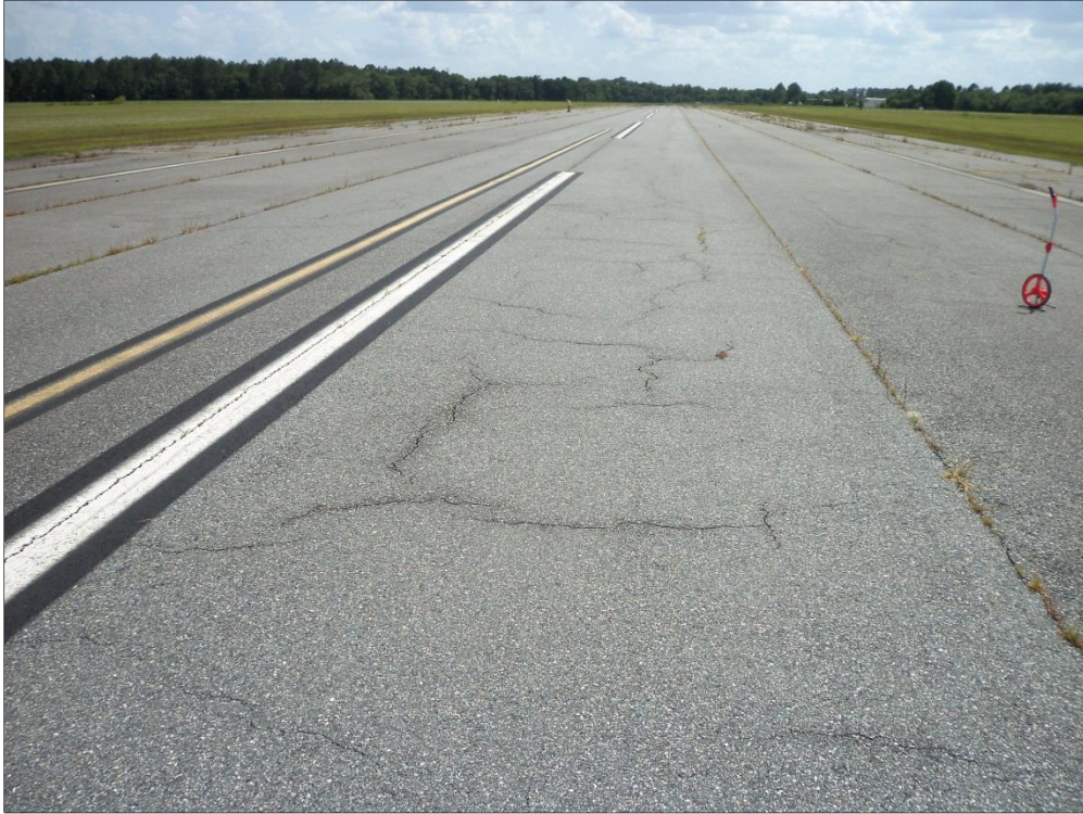
Runway 5-23, Section 6205, Sample Unit 135 – Medium Severity (57) Weathering, Low and Medium Severity (48) Longitudinal and Transverse Cracking, Low Severity (43) Block Cracking
