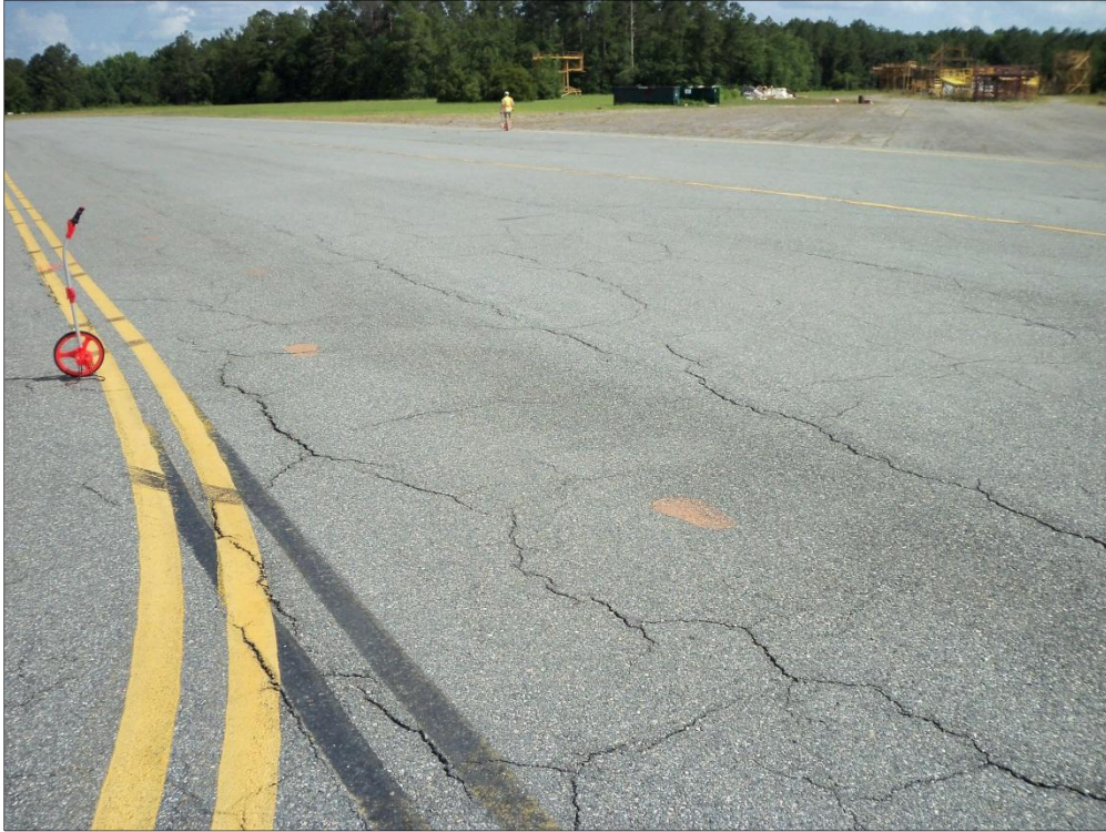
Taxiway B2, Section 220, Sample Unit 139 – Low Severity (43) Block Cracking, Medium Severity (57) Weathering, Low Severity (52) Raveling, Low Severity (53) Rutting
