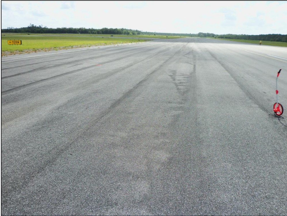
Runway 10-28, Section 6105, Sample Unit 400 – Low Severity (48) Longitudinal and Transverse Cracking, Low Severity (57) Weathering, Low Severity (56) Swelling
