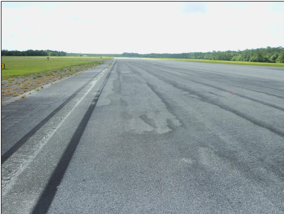
Runway 10-28, Section 6110, Sample Unit 200 – Low Severity (57) Weathering, Low Severity (56) Swelling
