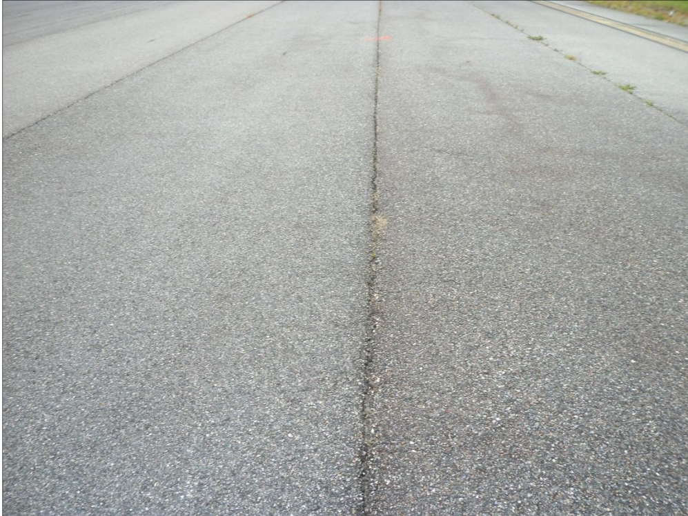
Runway 10-28, Section 6114, Sample Unit 419 – Medium Severity (48) Longitudinal and Transverse Cracking, Medium Severity (57) Weathering
