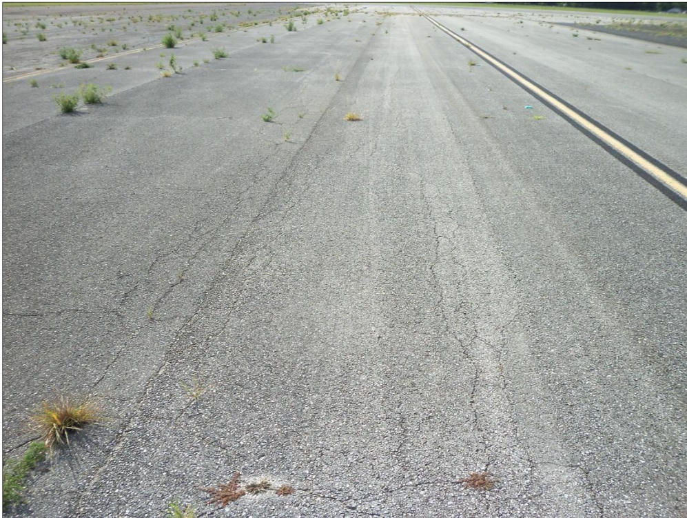
Taxiway B, Section 210, Sample Unit 140 – Low Severity (43) Block Cracking, Low Severity (57) Weathering, Low Severity (52) Raveling, Low Severity (41) Alligator Cracking
