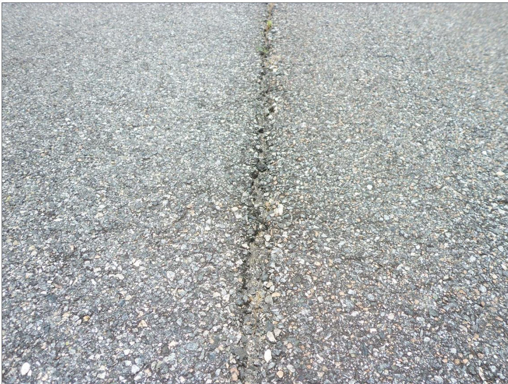
Runway 10-28, Section 6114, Sample Unit 419 – Medium Severity (48) Longitudinal and Transverse Cracking
