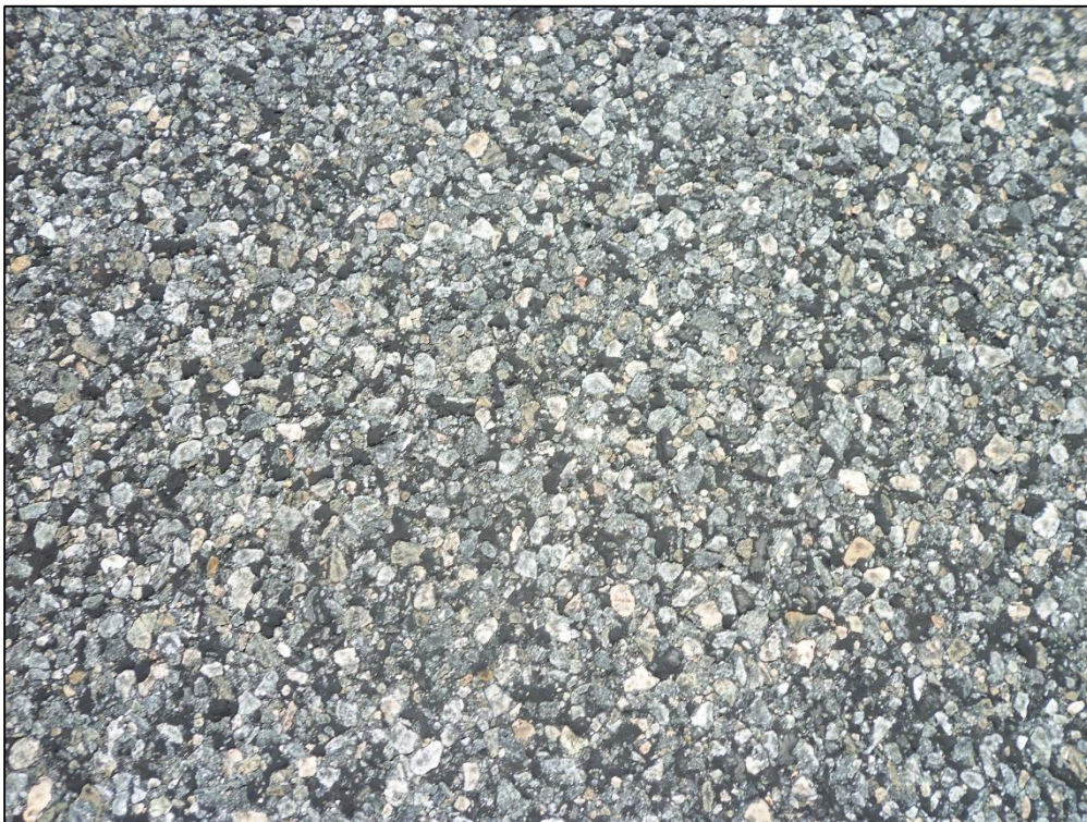
Runway 10-28, Section 6114, Sample Unit 423 – (42) Bleeding, Medium Severity (57) Weathering
