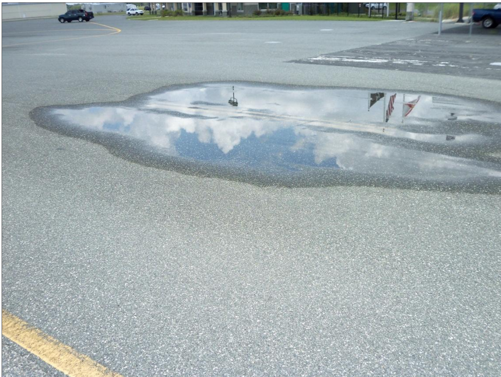
Taxiway D, Section 405, Sample Unit 112 – Low Severity (53) Rutting
