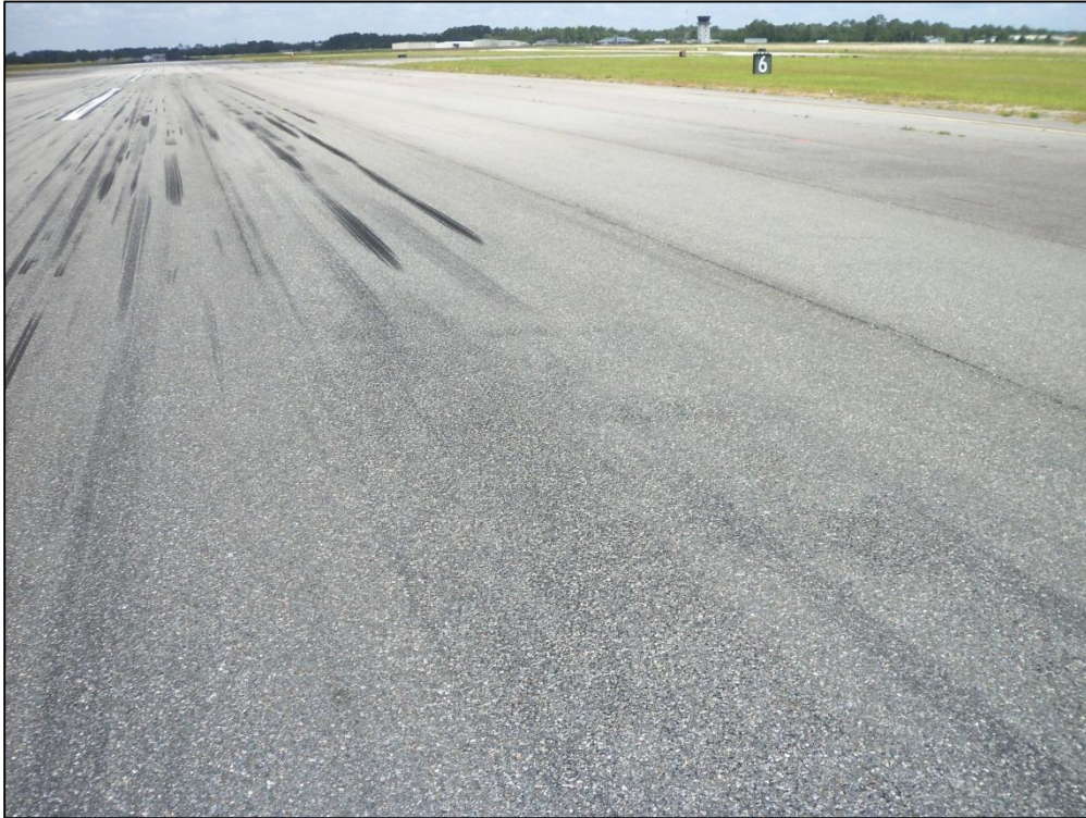
Runway 10-28, Section 6114, Sample Unit 423 – Low Severity (48) Longitudinal and Transverse Cracking, (42) Bleeding, Medium Severity (57) Weathering
