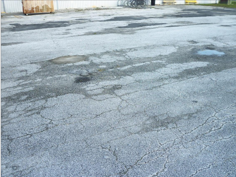
Apron E, Section 4228, Sample Unit 101 – Medium Severity (52) Raveling, High Severity (50) Patching, Medium Severity (45) Depression, Low Severity (43) Block Cracking, Low Severity (41) Alligator Cracking
