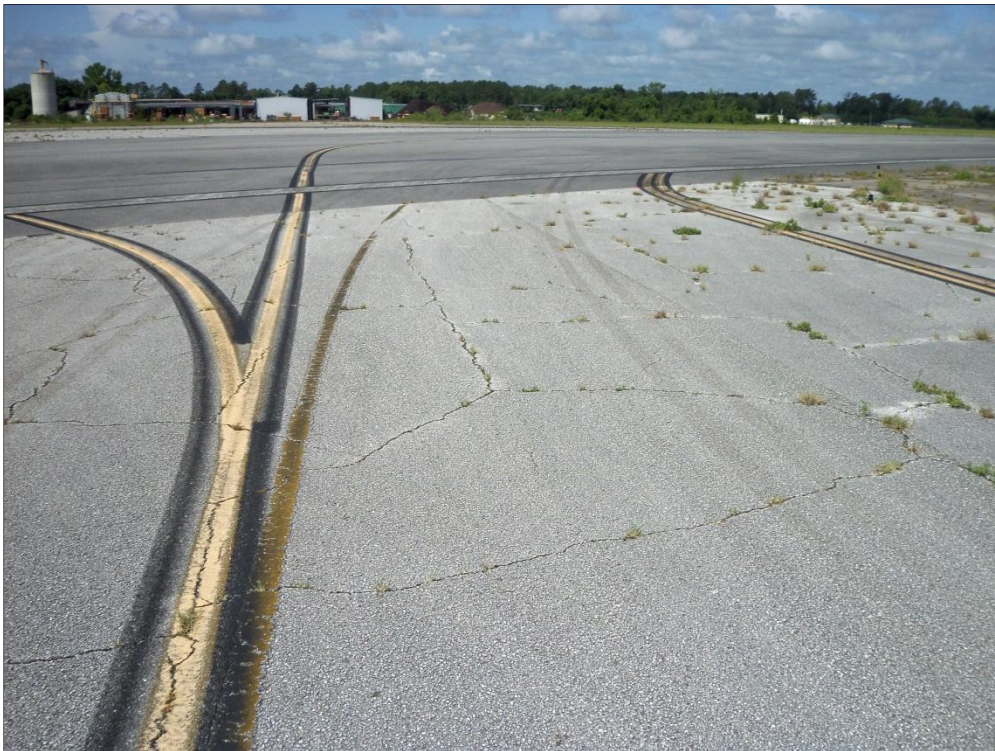
Taxiway C, Section 305, Sample Unit 100 – Low Severity (43) Block Cracking, Low Severity (52) Raveling, Low Severity (57) Weathering
