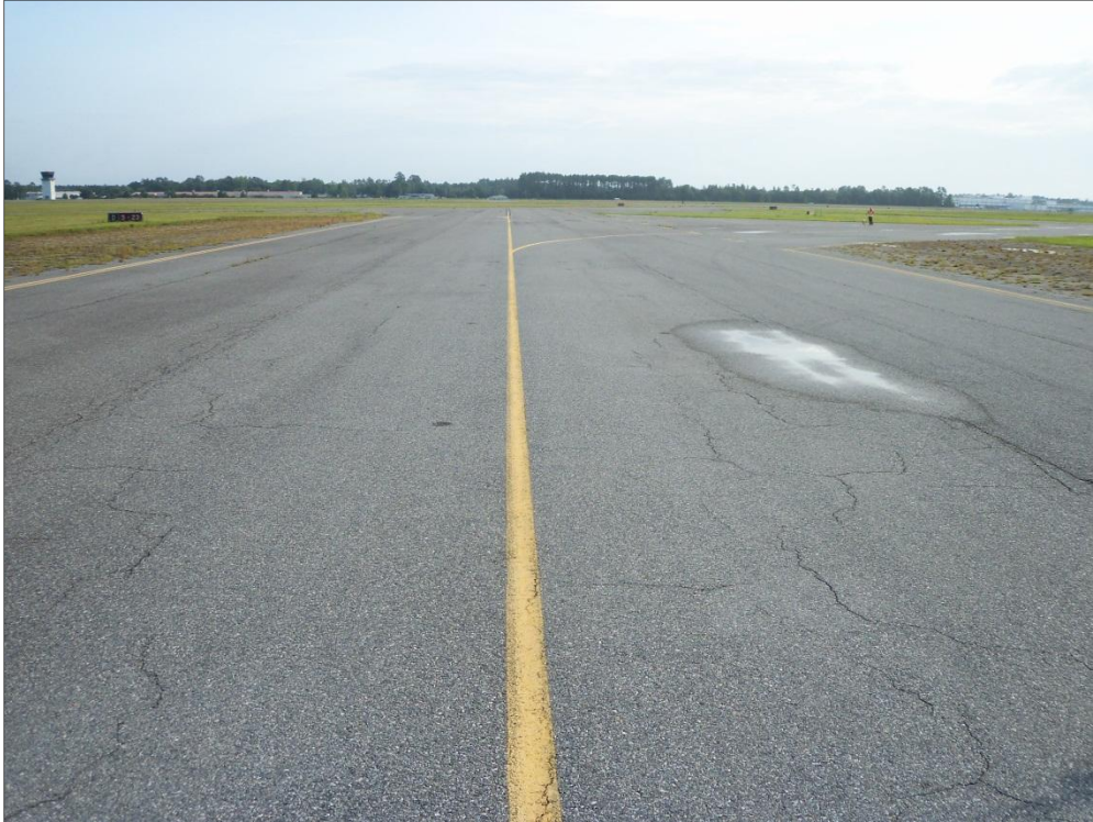
Taxiway D, Section 405, Sample Unit 112 – Low Severity (41) Alligator Cracking, Low and Medium Severity (48) Longitudinal and Transverse Cracking, Low Severity (52) Raveling, Low Severity (53) Rutting, Low Severity (57) Weathering
