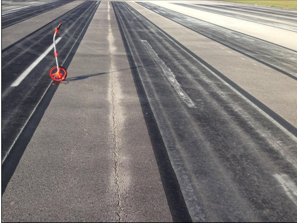
Runway 5-23, Section 6105, Sample Unit 349 – Low Severity (48) Longitudinal and Transverse Cracking, Low Severity (57) Weathering
