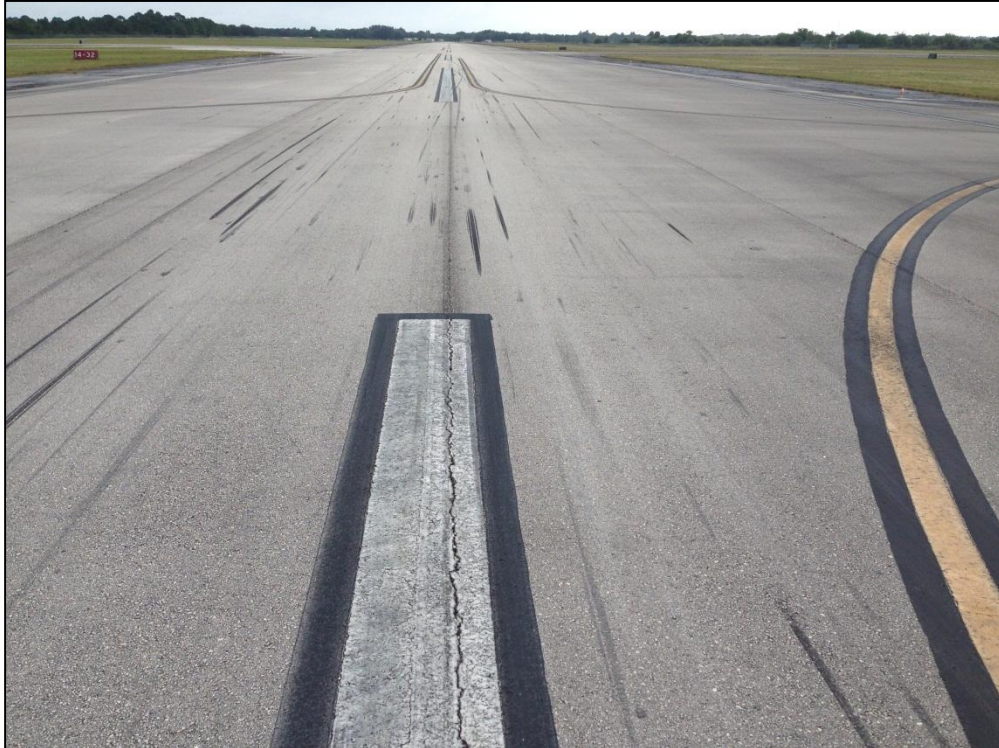
Runway 5-23, Section 6105, Sample Unit 314 – Low Severity (48) Longitudinal and Transverse Cracking, Low Severity (57) Weathering
