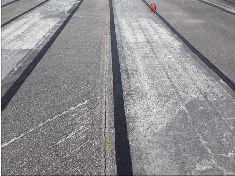
Runway 14-32, Section 6205, Sample Unit 301 – Medium Severity (48) Longitudinal and Transverse Cracking, Low and Medium Severity (52) Raveling
