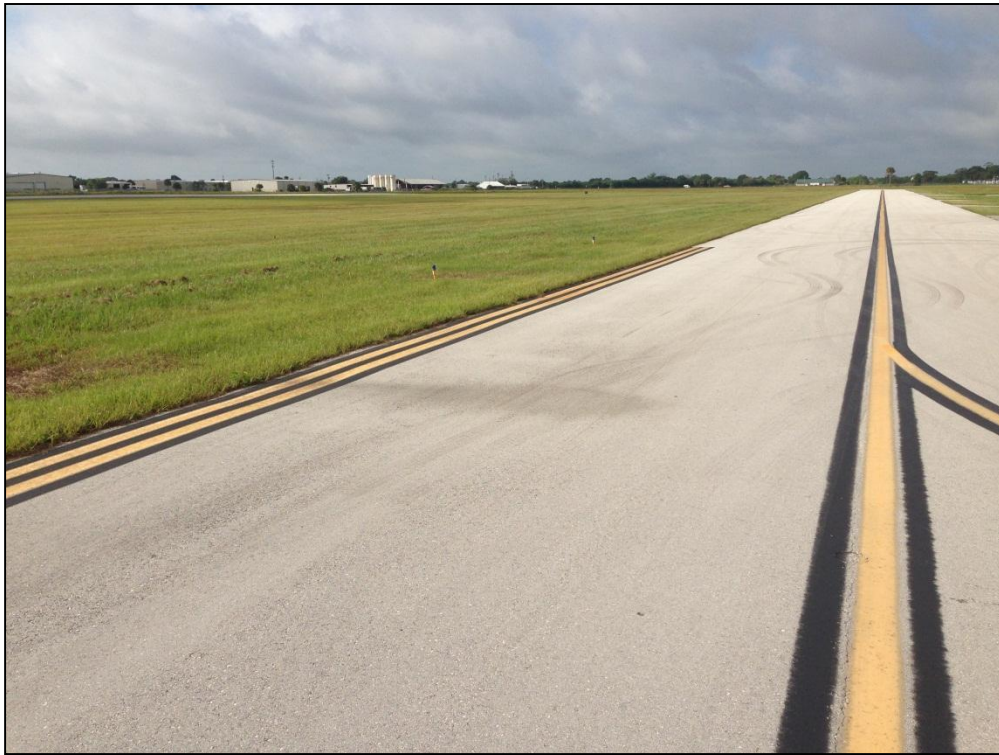
Taxiway A, Section 105, Sample Unit 114 – Low Severity (45) Depression, Low Severity (57) Weathering
