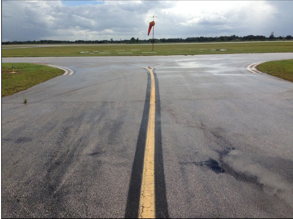
Taxiway A, Section 125, Sample Unit 700 – Low Severity (45) Depression, Low Severity (48) Longitudinal and Transverse Cracking, Low Severity (52) Raveling, Low Severity (57) Weathering
