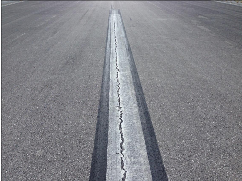
Runway 14-32, Section 6205, Sample Unit 315 – Medium Severity (48) Longitudinal and Transverse Cracking, Low Severity (57) Weathering
