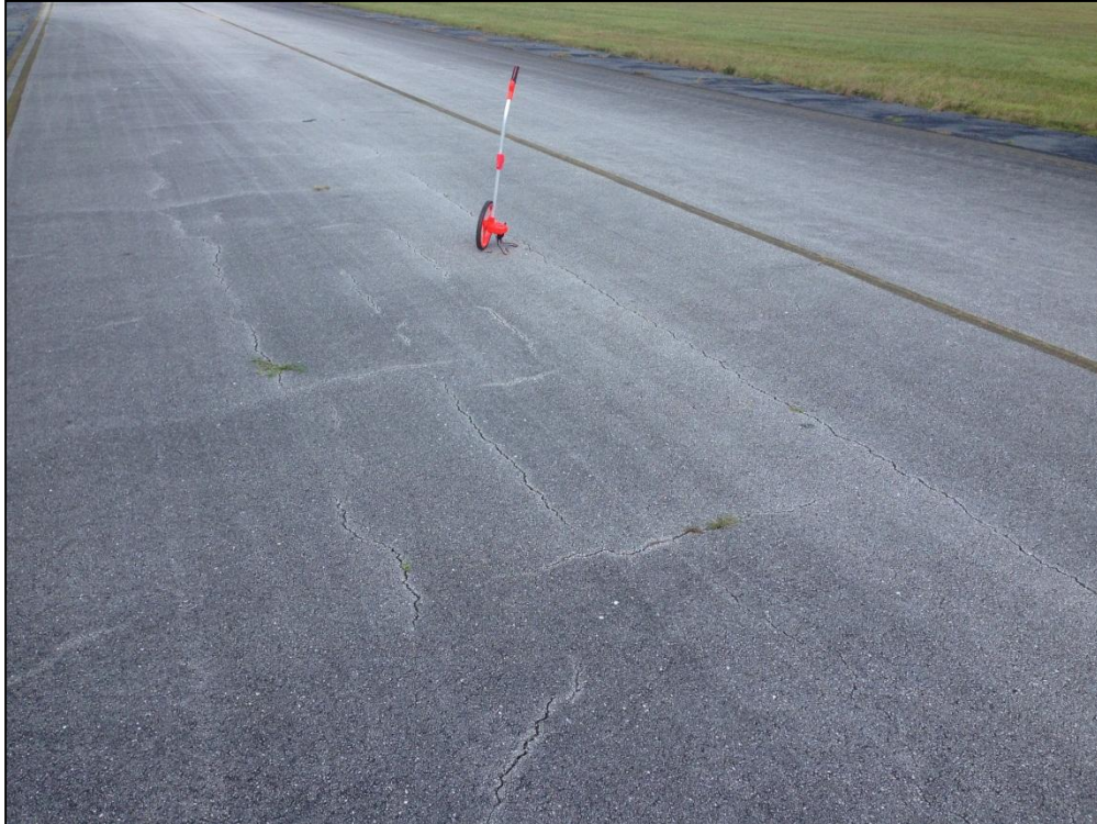
Taxiway B, Section 205, Sample Unit 131 – Low Severity (43) Block Cracking, Low Severity (57) Weathering
