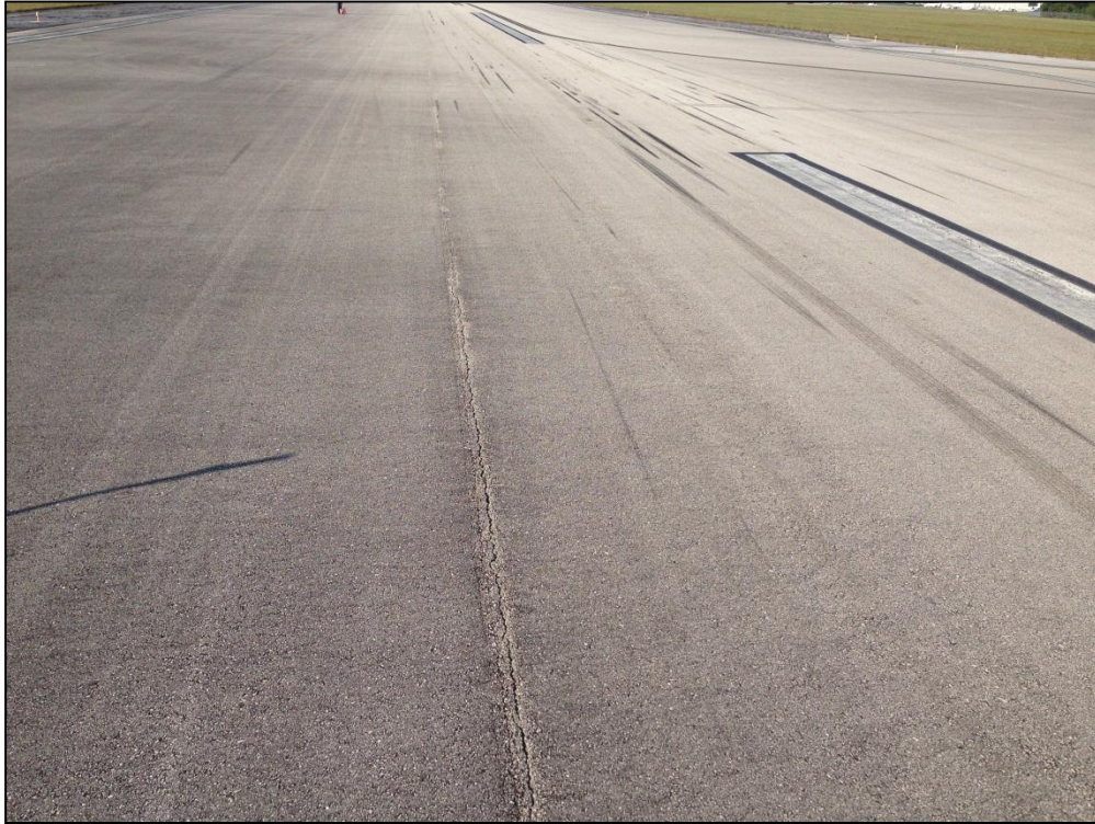
Runway 5-23, Section 6105, Sample Unit 335 – Low Severity (48) Longitudinal and Transverse Cracking, Low Severity (57) Weathering
