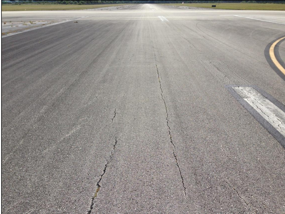
Runway 14-32, Section 6205, Sample Unit 343 – Low and Medium Severity (48) Longitudinal and Transverse Cracking, Low Severity (52) Raveling, Low Severity (57) Weathering
