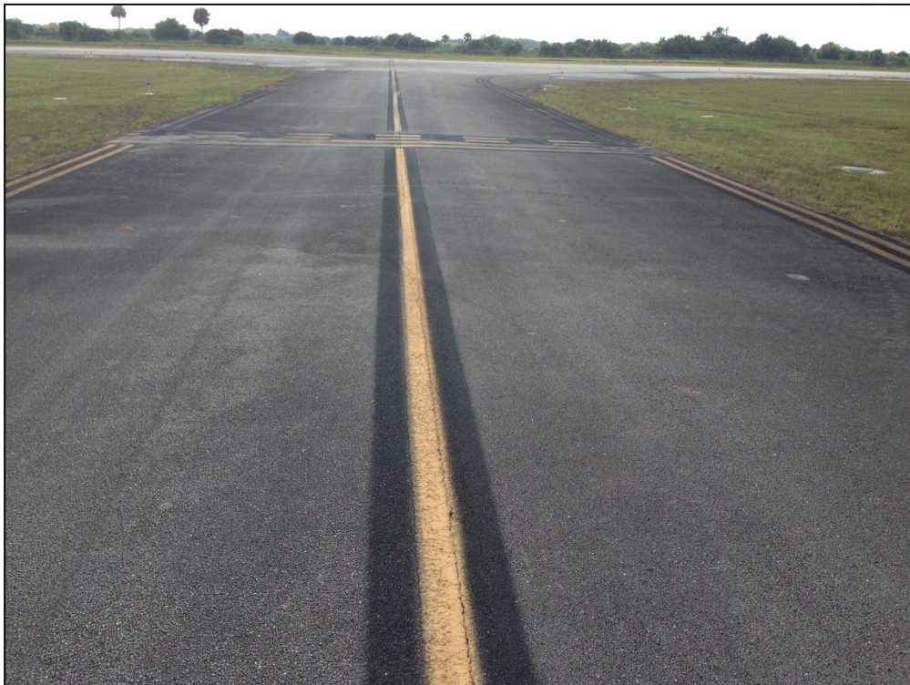
Taxiway D, Section 405, Sample Unit 102 – Low Severity (48) Longitudinal and Transverse Cracking, Low Severity (52) Raveling, Low Severity (57) Weathering
