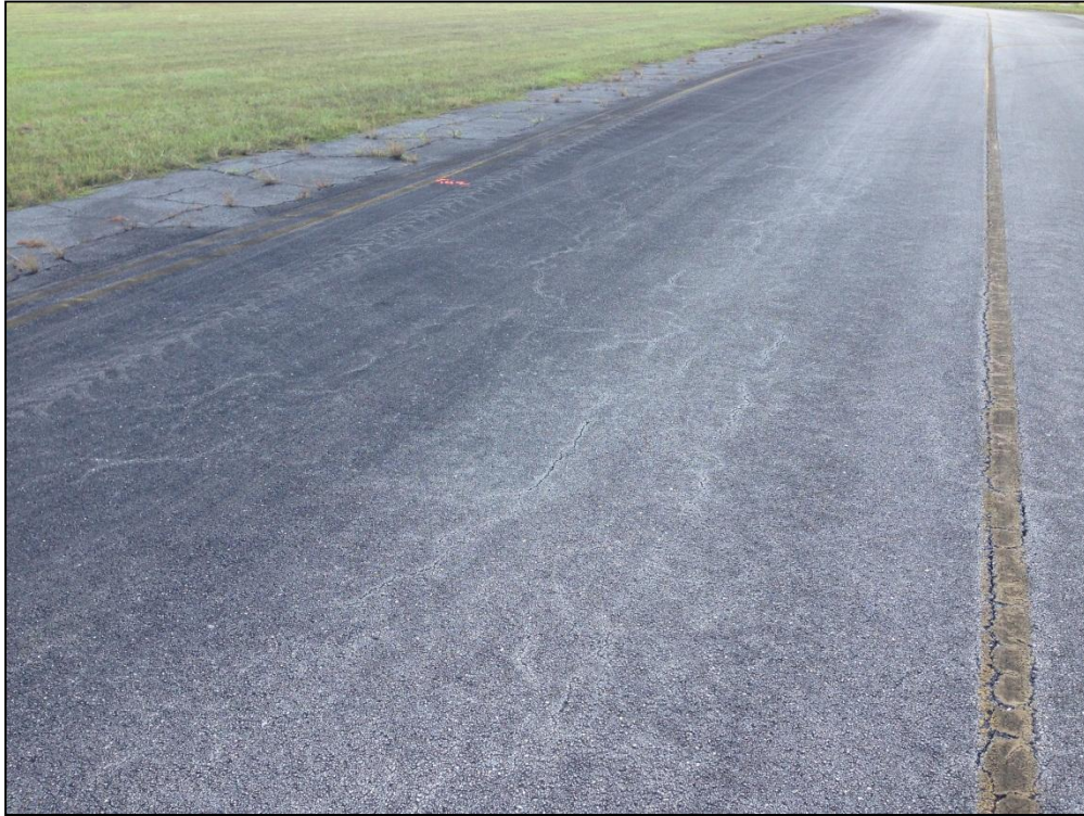
Taxiway B, Section 205, Sample Unit 142 – Low Severity (48) Longitudinal and Transverse Cracking, Low Severity (52) Raveling, Low Severity (57) Weathering
