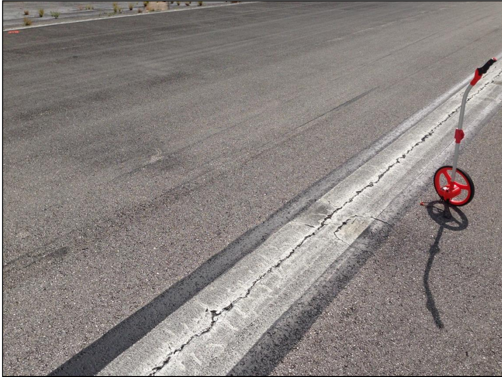
Runway 14-32, Section 6205, Sample Unit 319 – Low Severity (45) Depression, Medium Severity (48) Longitudinal and Transverse Cracking, Low Severity (57) Weathering
