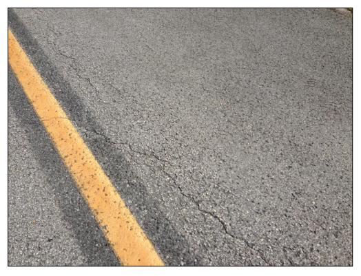
Taxiway T-Hang, Section 720, Sample Unit 100 – Low Severity (48) Longitudinal and Transverse Cracking, Medium Severity (52) Raveling
