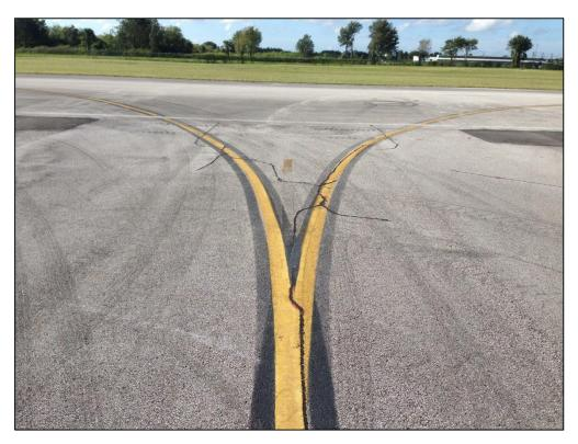
Taxiway A, Section 160, Sample Unit 300 – Low Severity (48) Longitudinal and Transverse Cracking, Low Severity (52) Raveling, Low Severity (57) Weathering, Low Severity (50) Patching
