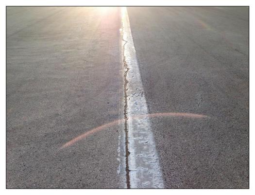
Runway 10-28, Section 6103, Sample Unit 296 – Low Severity (48) Longitudinal and Transverse Cracking, Low Severity (52) Raveling, Low Severity (57) Weathering, Low Severity (56) Swelling
