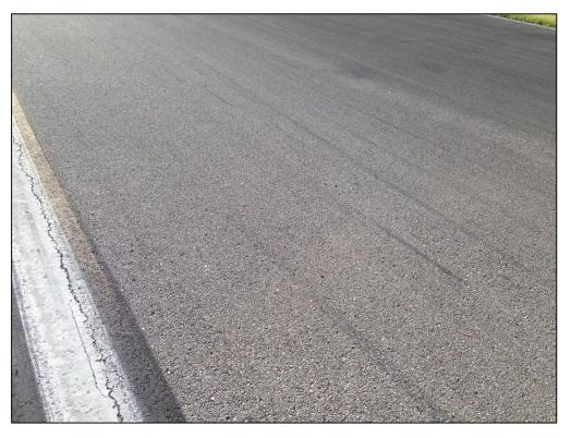
Runway 10-28, Section 6115, Sample Unit 342 – Low Severity (48) Longitudinal and Transverse Cracking, Low Severity (52) Raveling, Low Severity (57) Weathering
