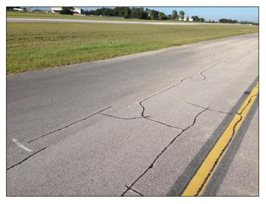
Taxiway A, Section 110, Sample Unit 130 – Low Severity (48) Longitudinal and Transverse Cracking, Low Severity (52) Raveling, Low Severity (57) Weathering
