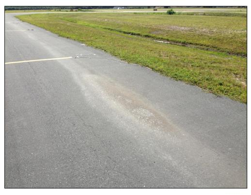
Apron, Section 4110, Sample Unit 105 – Low Severity (48) Longitudinal and Transverse Cracking, Low Severity (45) Depression
