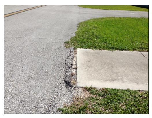
Taxiway T-Hang, Section 725, Sample Unit 400 – Low Severity (48) Longitudinal and Transverse Cracking, Low Severity (52) Raveling, Low Severity (57) Weathering, Medium Severity (54) Shoving
