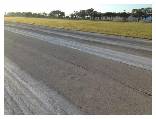
Runway 10-28, Section 6115, Sample Unit 301 – Low Severity (48) Longitudinal and Transverse Cracking, Low Severity (52) Raveling, Low Severity (57) Weathering, Low Severity (56) Swelling
