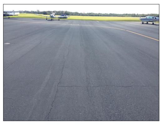
Apron, Section 4130, Sample Unit 209 - Low Severity (48) Longitudinal and Transverse Cracking
