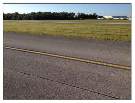
Taxiway A, Section 115, Sample Unit 135 – Low Severity (48) Longitudinal and Transverse Cracking, Low Severity (52) Raveling, Low Severity (57) Weathering
