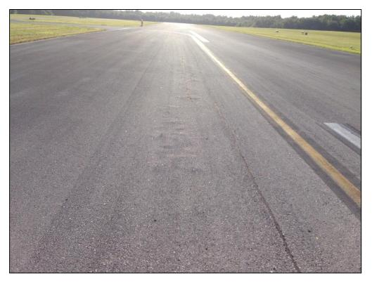
Runway 10-28, Section 6115, Sample Unit 356 – Low Severity (48) Longitudinal and Transverse Cracking, Low Severity (52) Raveling, Low Severity (57) Weathering, Low Severity (56) Swelling
