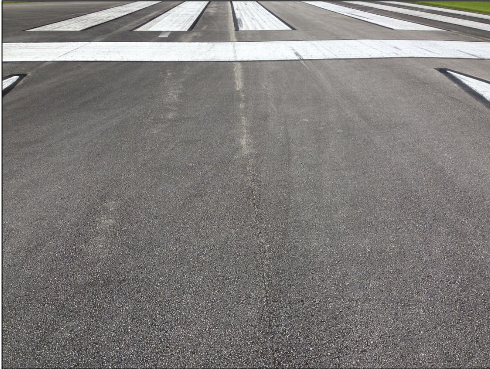
Runway 17-35, Section 6110, Sample Unit 180 – Low Severity (48) Longitudinal and Transverse Cracking, Low Severity (52) Raveling, Low Severity (57) Weathering, Low Severity (56) Swelling
