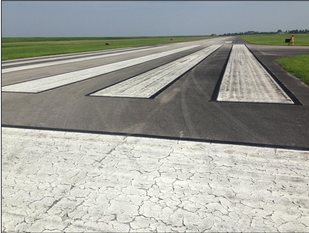
Runway 17-35, Section 6105, Sample Unit 101 – Low Severity (48) Longitudinal and Transverse Cracking, Low Severity (52) Raveling, Low Severity (57) Weathering
