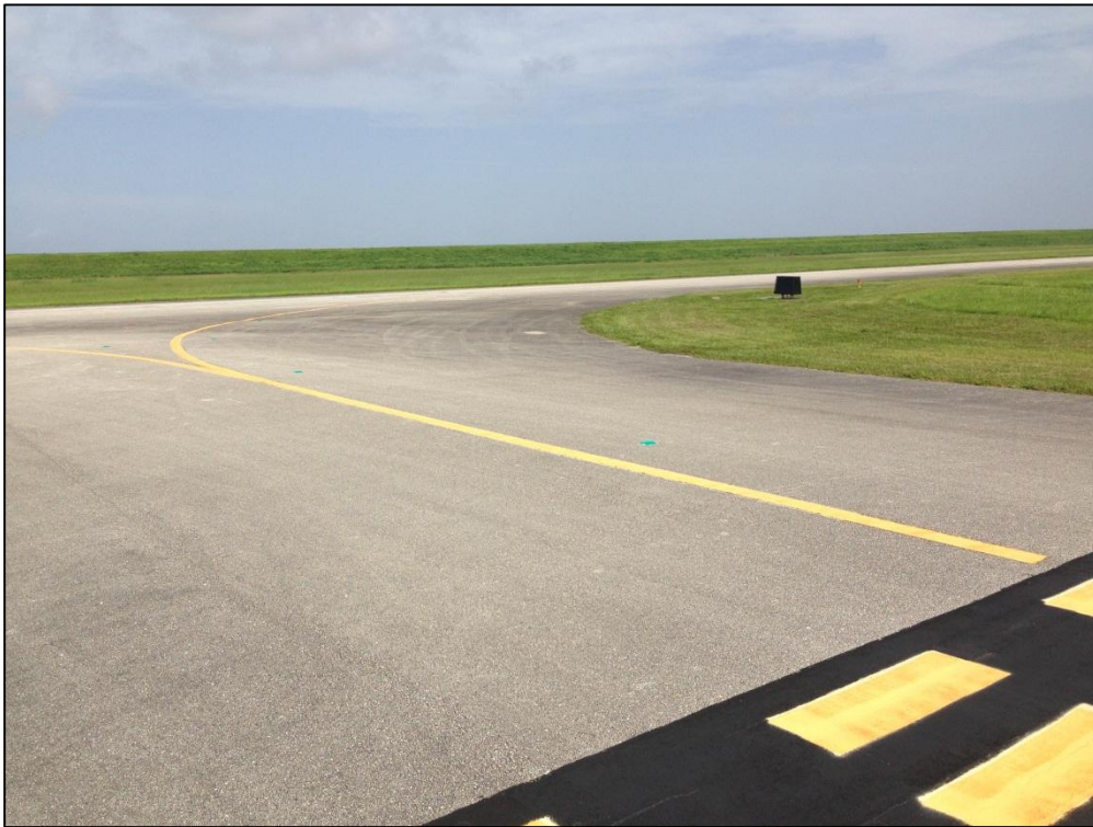
Taxiway Delta, Section 110, Sample Unit 100 – Low Severity (48) Longitudinal and Transverse Cracking, Low Severity (52) Raveling, Low Severity (57) Weathering
