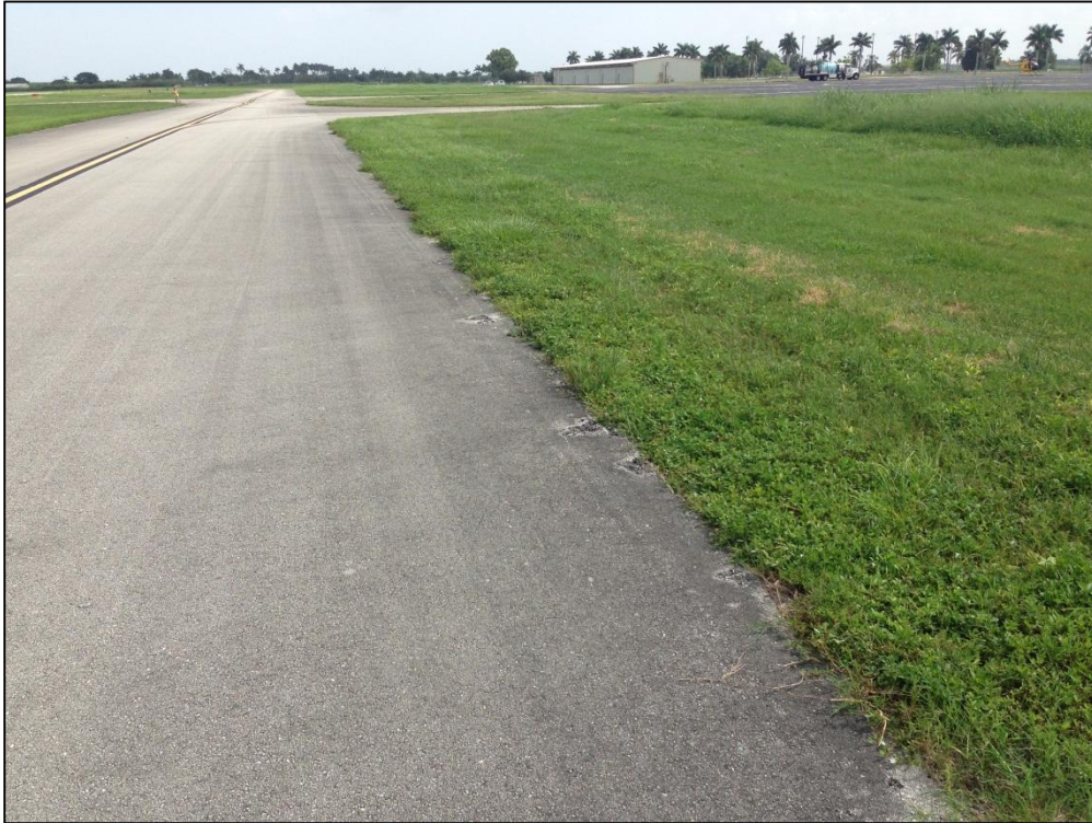
Taxiway Alpha, Section 105, Sample Unit 112 – Medium Severity (52) Raveling, Low Severity (57) Weathering
