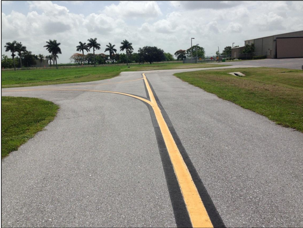
Apron T-Hangar, Section 4205, Sample Unit 101 – Low Severity (52) Raveling, Low Severity (57) Weathering
