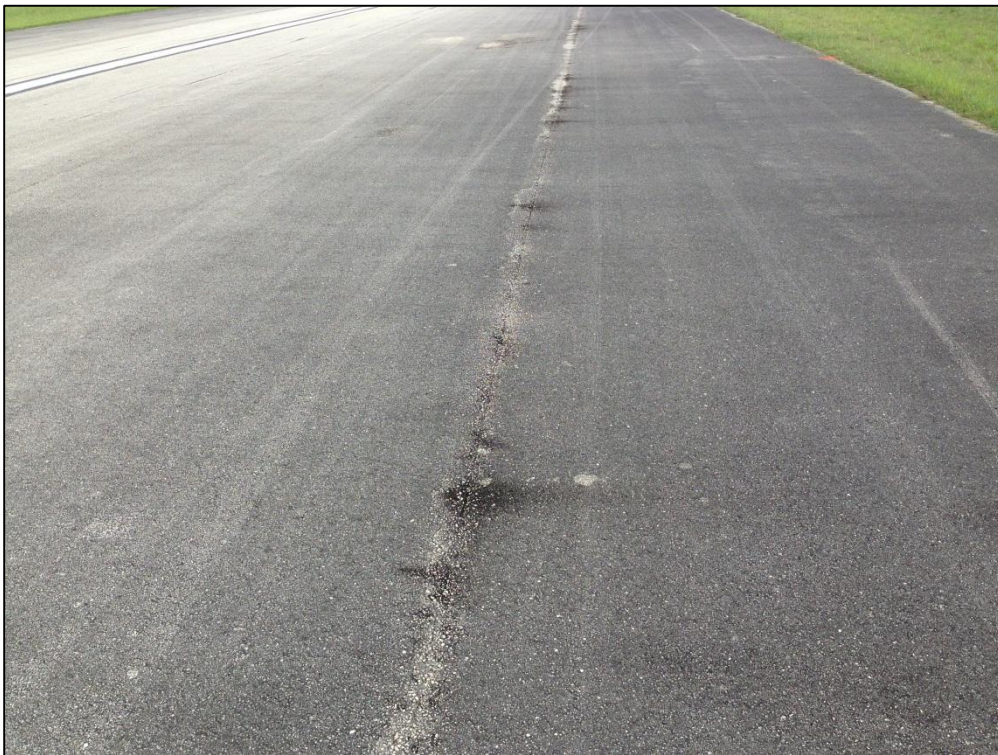
Runway 17-35, Section 6110, Sample Unit 131 – Low and Medium Severity (48) Longitudinal and Transverse Cracking, Low Severity (52) Raveling, Low Severity (57) Weathering, Low Severity (56) Swelling
