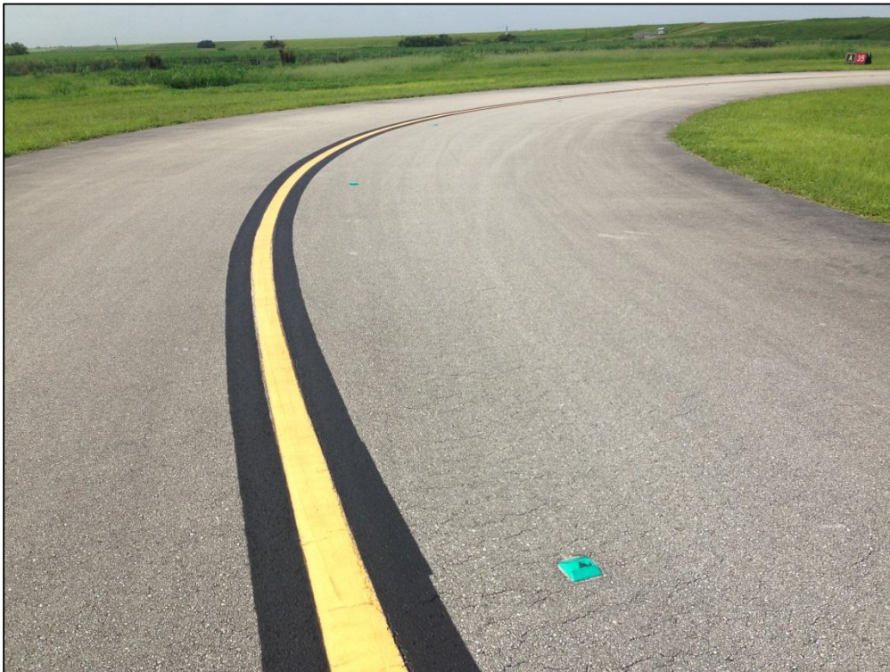
Taxiway Alpha, Section 105, Sample Unit 140 – Low Severity (48) Longitudinal and Transverse Cracking, Low Severity (52) Raveling, Low Severity (57) Weathering
