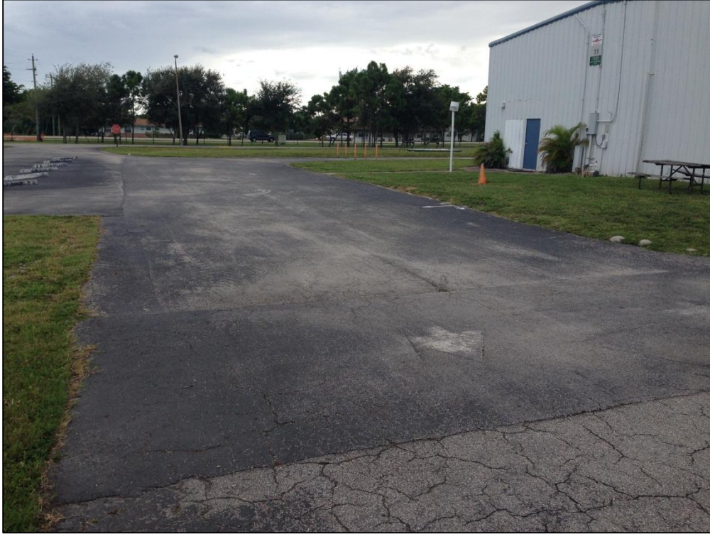
Apron Hang, Section 4315, Sample Unit 700 – Low Severity (43) Block Cracking, Low Severity (50) Patching, Low Severity (52) Raveling, Low Severity (57) Weathering
