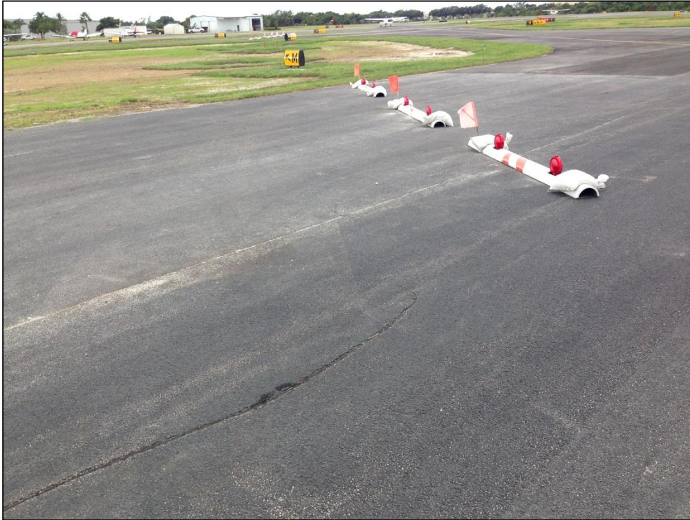
Runway 10-28, Section 6105, Sample Unit 124 – Low Severity (48) Longitudinal and Transverse Cracking, Low Severity (52) Raveling, Low Severity (57) Weathering
