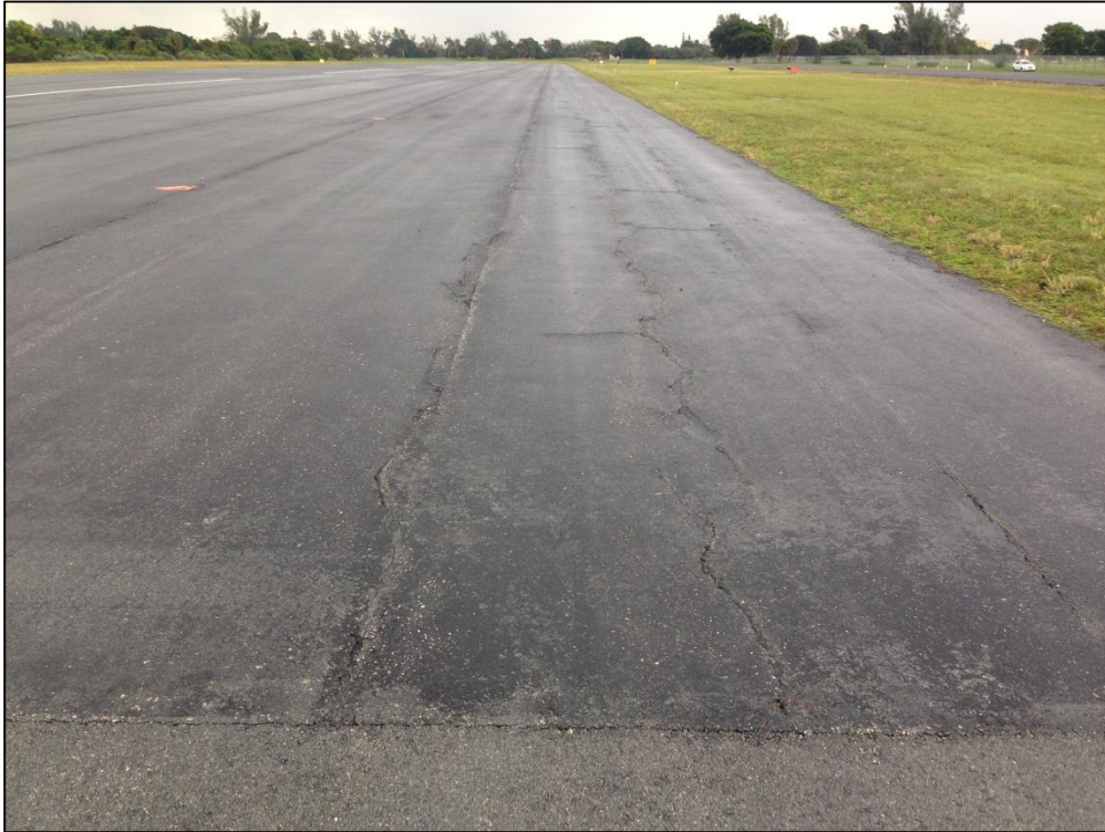
Runway 6-24, Section 6210, Sample Unit 556 – Low Severity (48) Longitudinal and Transverse Cracking, Low Severity (57) Weathering
