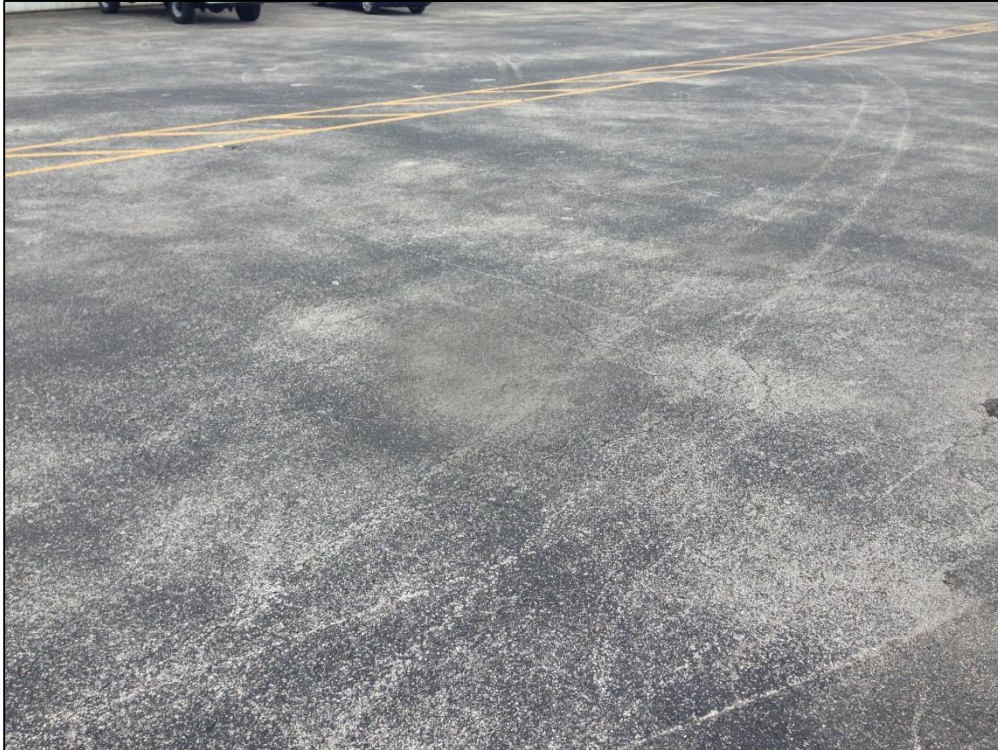
Apron S, Section 4125, Sample Unit 305 – Low Severity (45) Depression, Low Severity (43) Block Cracking, Low Severity (52) Raveling, Low Severity (57) Weathering
