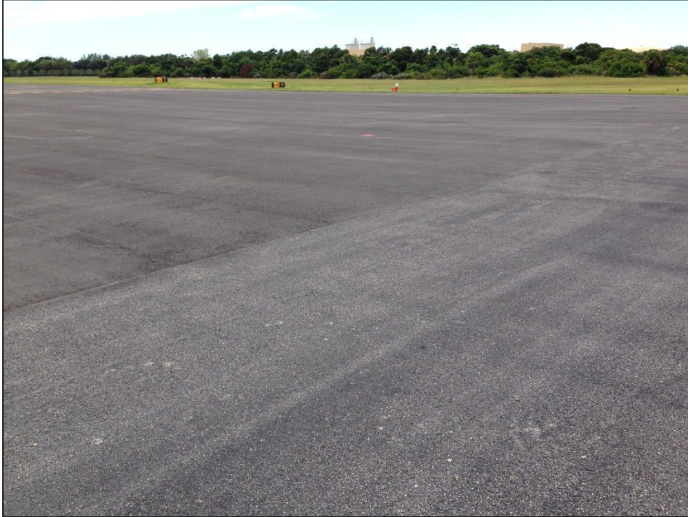
Runway 10-28, Section 6105, Sample Unit 102 – Low Severity (48) Longitudinal and Transverse Cracking, Low Severity (50) Patching, Low Severity (57) Weathering
