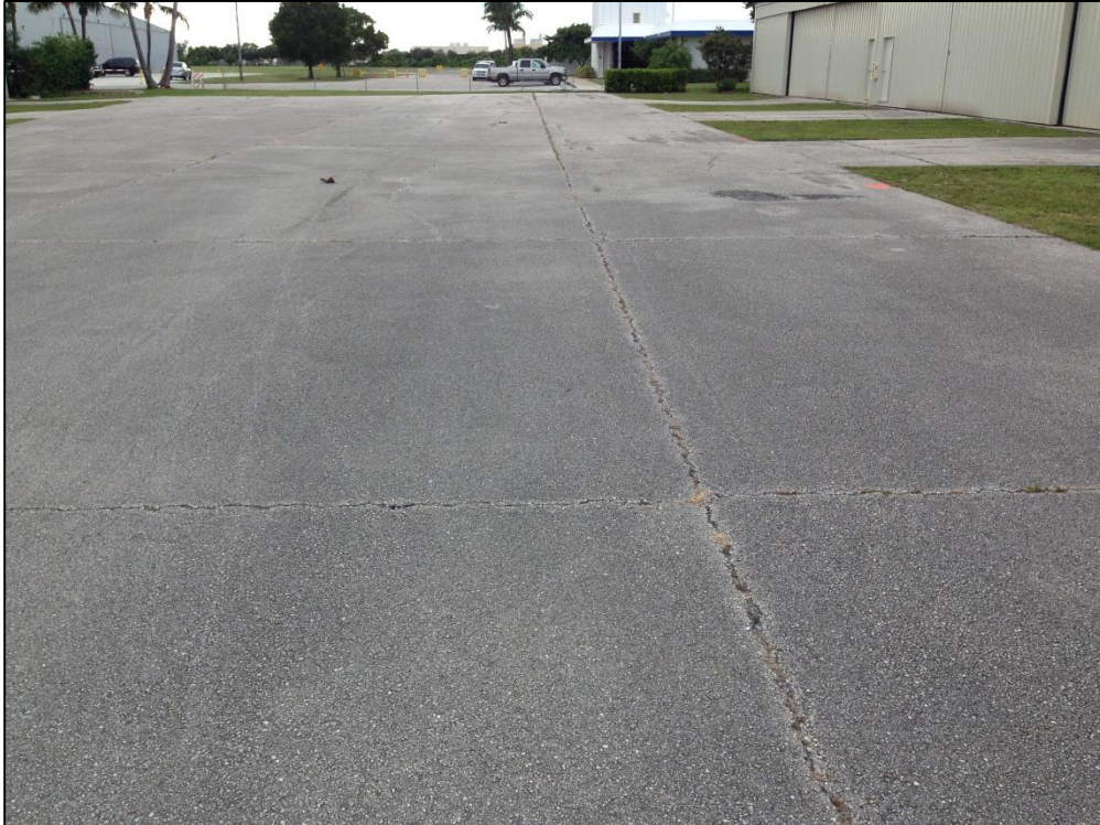
Apron Hang, Section 4320, Sample Unit 208 – Low Severity (47) Joint Reflection Cracking, Low Severity (57) Weathering
