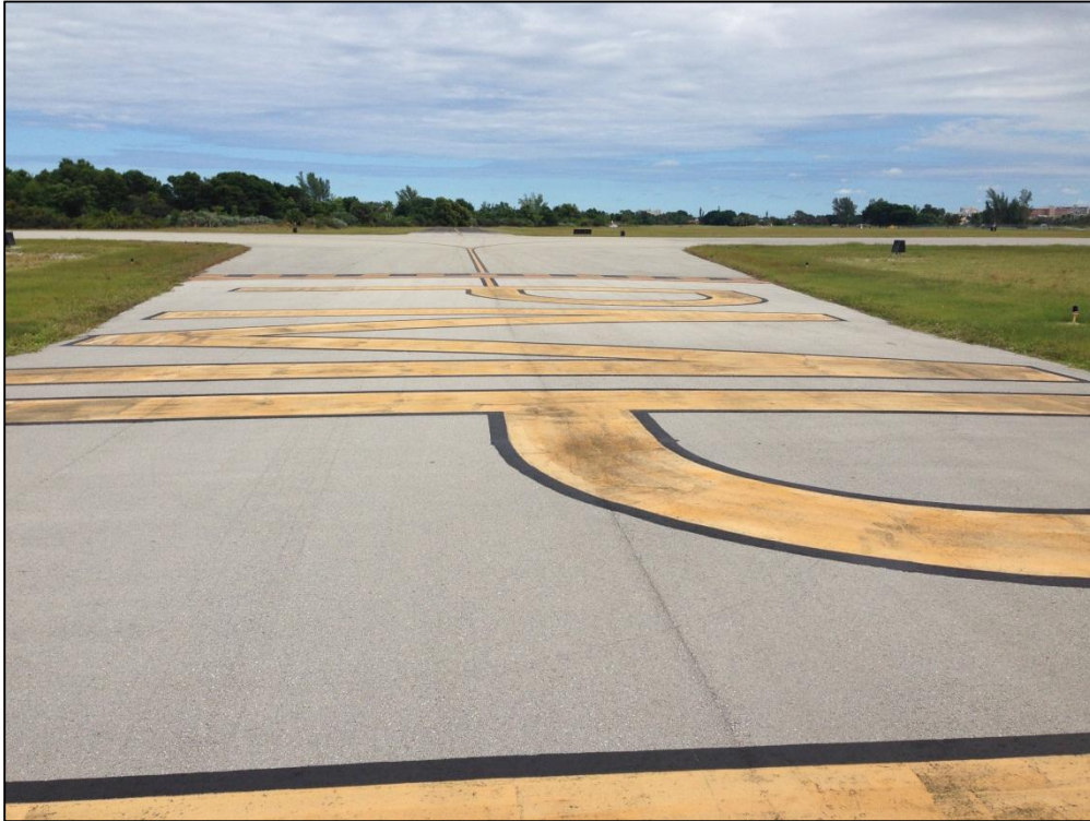
Taxiway F, Section 612, Sample Unit 616 – Low Severity (48) Longitudinal and Transverse Cracking, Low Severity (57) Weathering
