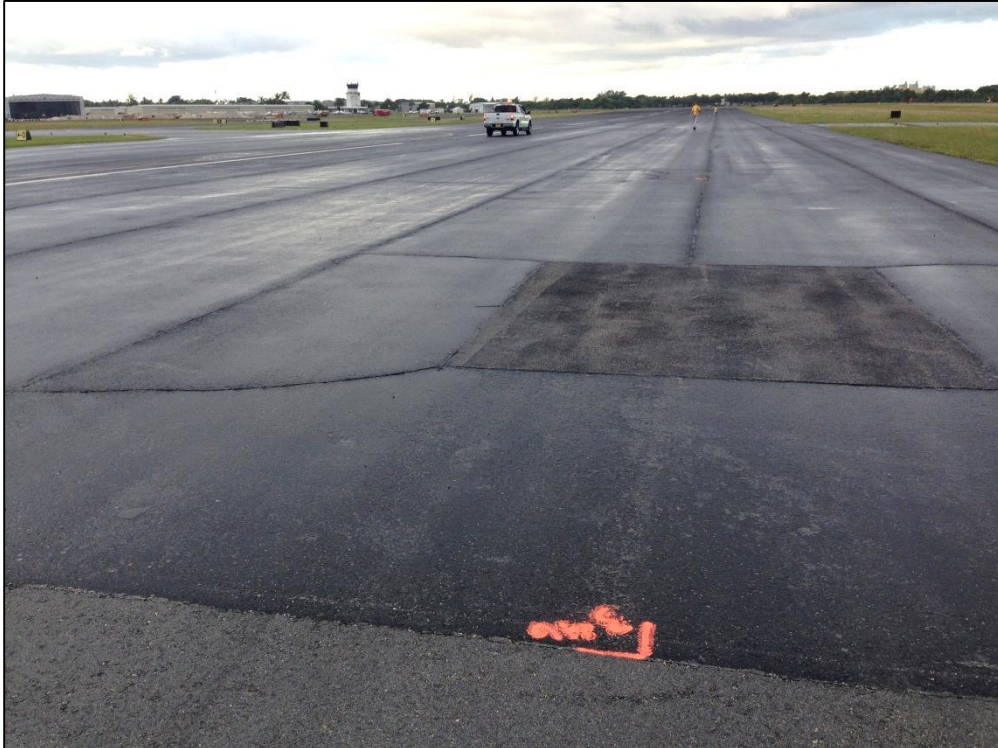
Runway 6-24, Section 6205, Sample Unit 346 – Low Severity (48) Longitudinal and Transverse Cracking, Low Severity (50) Patching, Low Severity (57) Weathering
