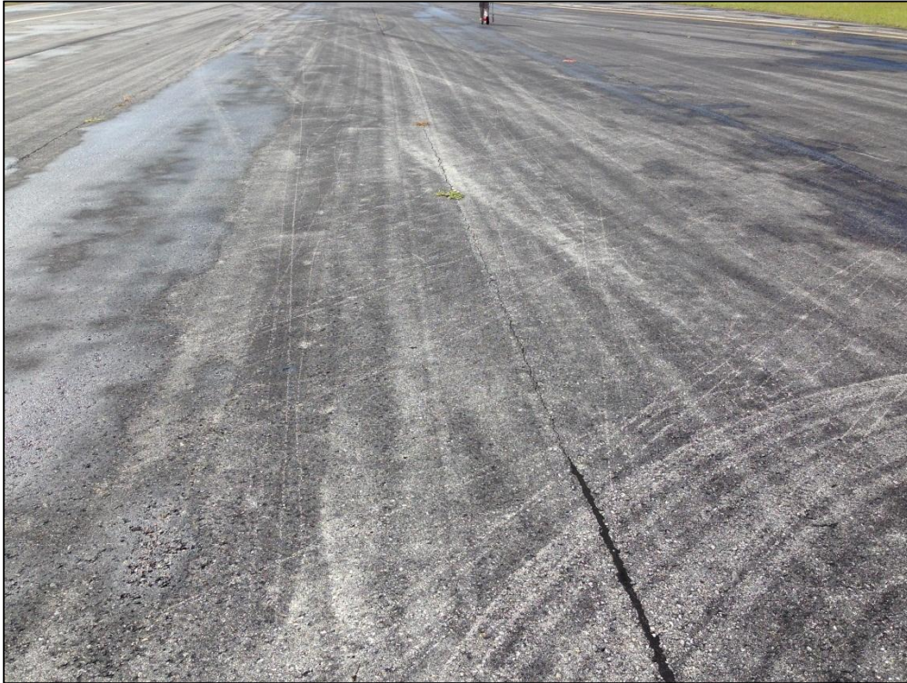
Apron N, Section 4205, Sample Unit 517 – Low Severity (48) Longitudinal and Transverse Cracking, Low Severity (57) Weathering
