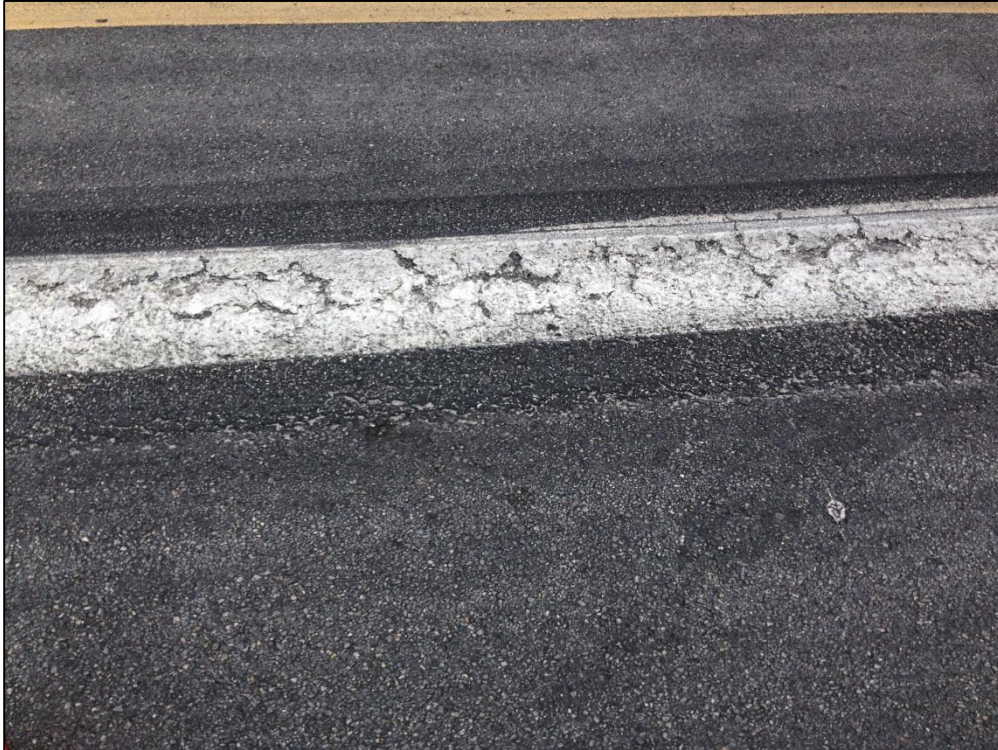
Runway 10-28, Section 6110, Sample Unit 110 – Low Severity (48) Longitudinal and Transverse Cracking, Low Severity (52) Raveling, Low Severity (57) Weathering
