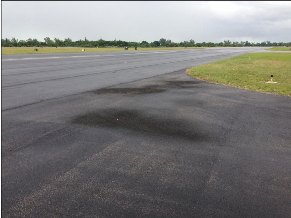
Taxiway C, Section 305, Sample Unit 300 – Low Severity (45) Depression, Low Severity (48) Longitudinal and Transverse Cracking, Low Severity (57) Weathering
