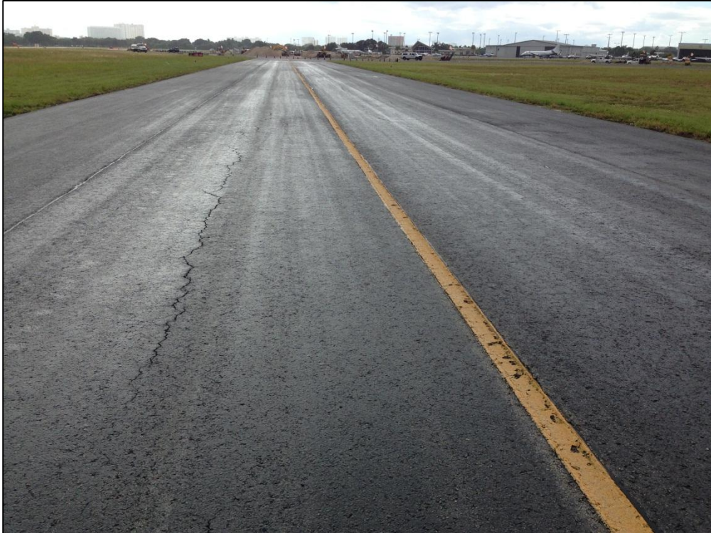
Taxiway D, Section 405, Sample Unit 420 – Low Severity (48) Longitudinal and Transverse Cracking, Low Severity (57) Weathering
