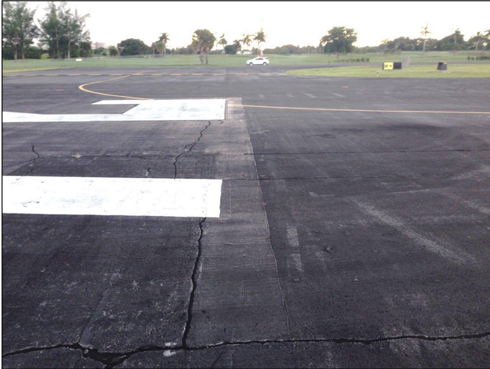
Runway 6-24, Section 6205, Sample Unit 378 – Low Severity (48) Longitudinal and Transverse Cracking, Low Severity (57) Weathering
