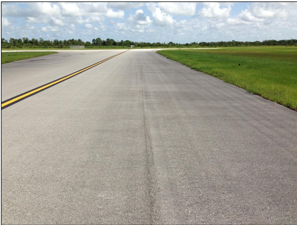
Taxiway Alpha, Section 420, Sample Unit 250 – Low Severity (48) Longitudinal and Transverse Cracking, Low Severity (57) Weathering
