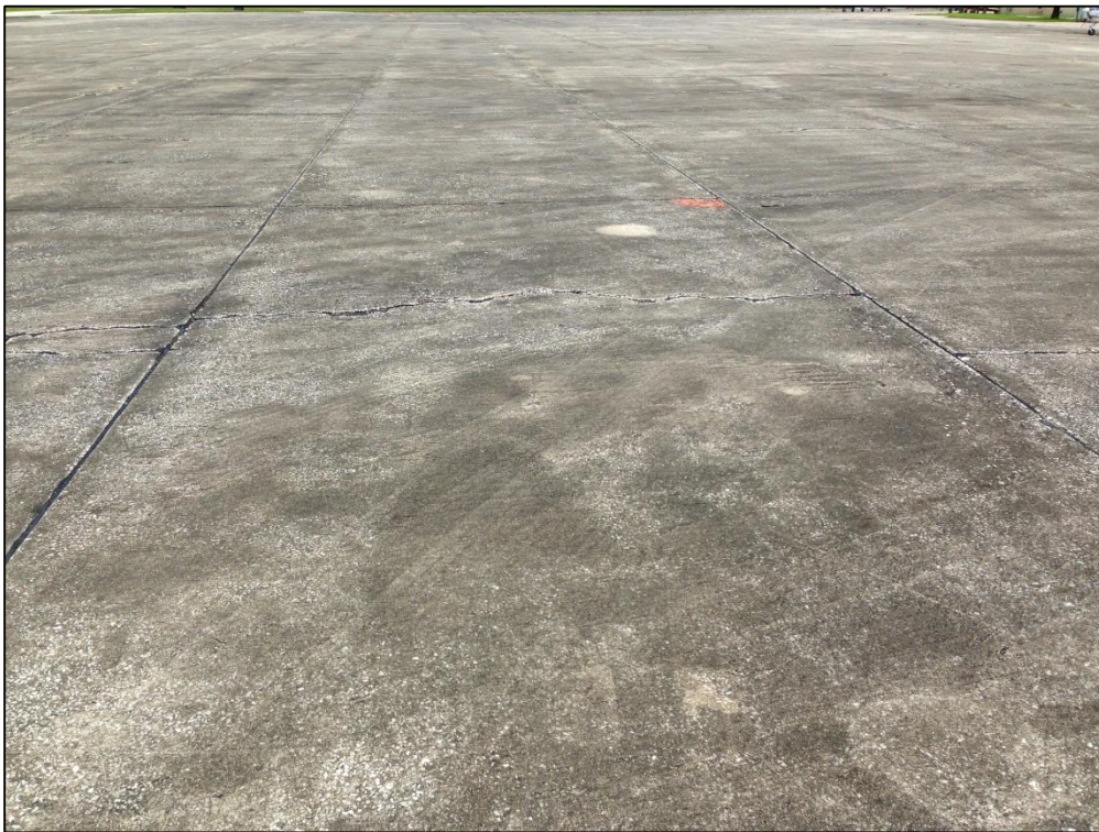
Apron West, Section 4105, Sample Unit 312 – Low and Medium Severity (63) Longitudinal, Transverse, Diagonal Cracking, Low Severity (65) Joint Seal Damage
