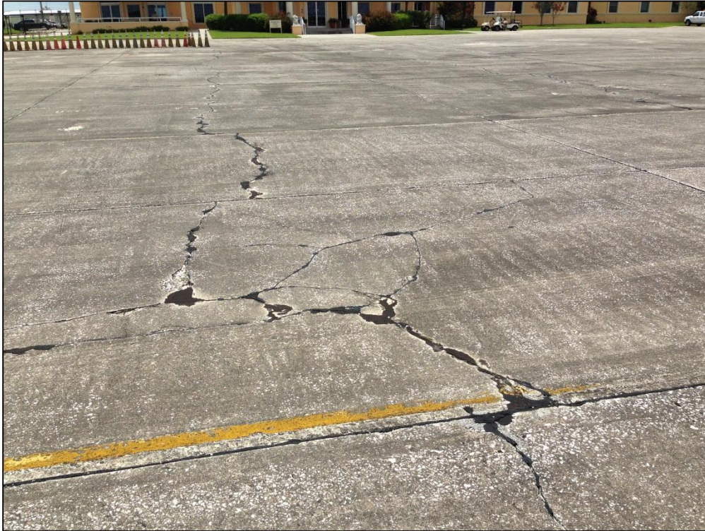
Apron West, Section 4105, Sample Unit 114 – Medium Severity (72) Shattered Slab, Medium Severity (63) Longitudinal, Transverse, Diagonal Cracking, Low Severity (65) Joint Seal Damage
