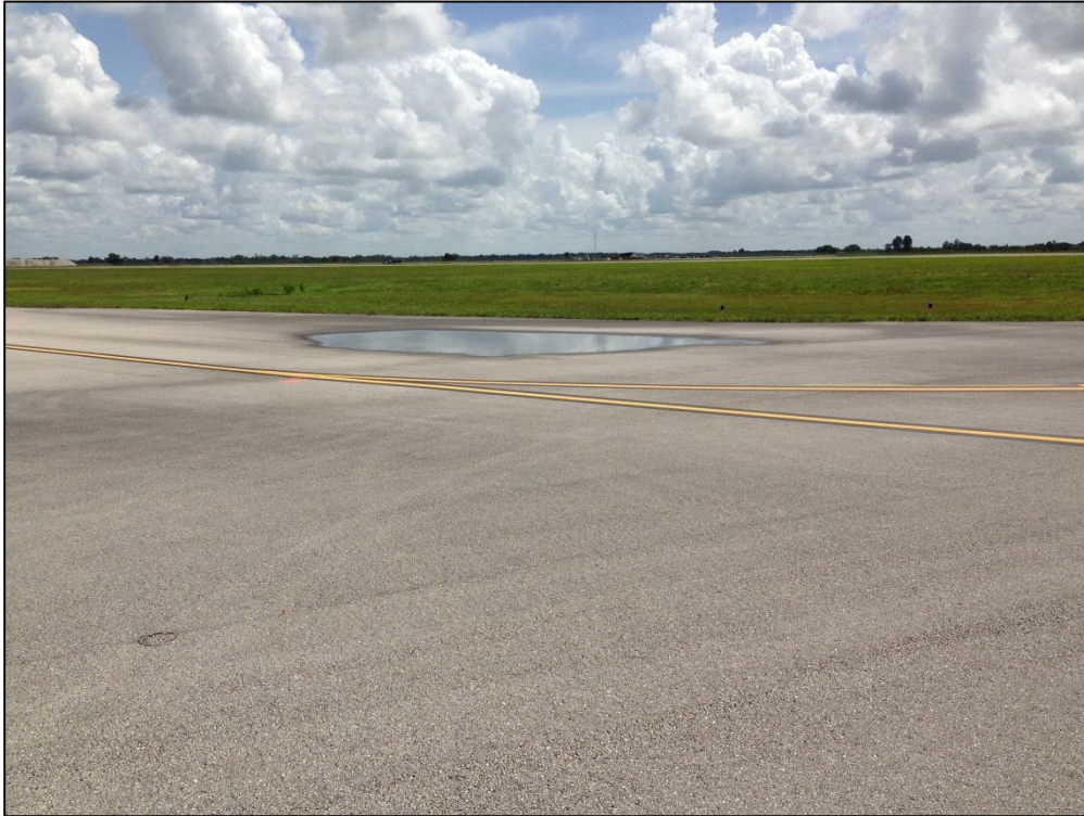
Taxiway A2, Section 110, Sample Unit 108 – Low Severity (57) Weathering, Low Severity (45) Depression
