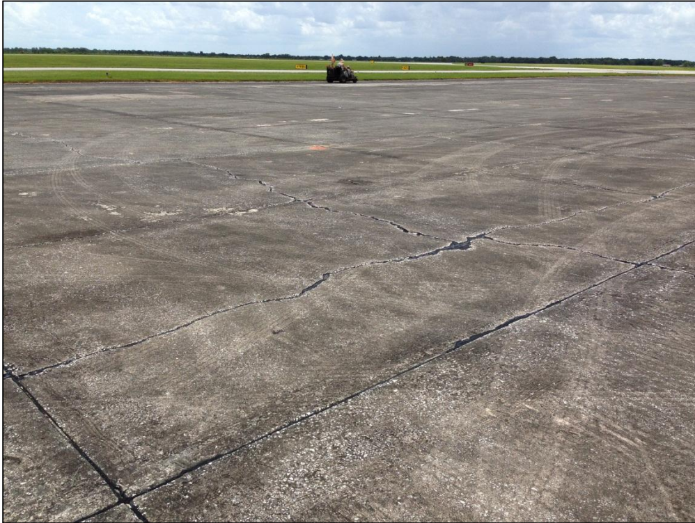
Apron West, Section 4105, Sample Unit 312 – Medium Severity (72) Shattered Slab, Low Severity (65) Joint Seal Damage
