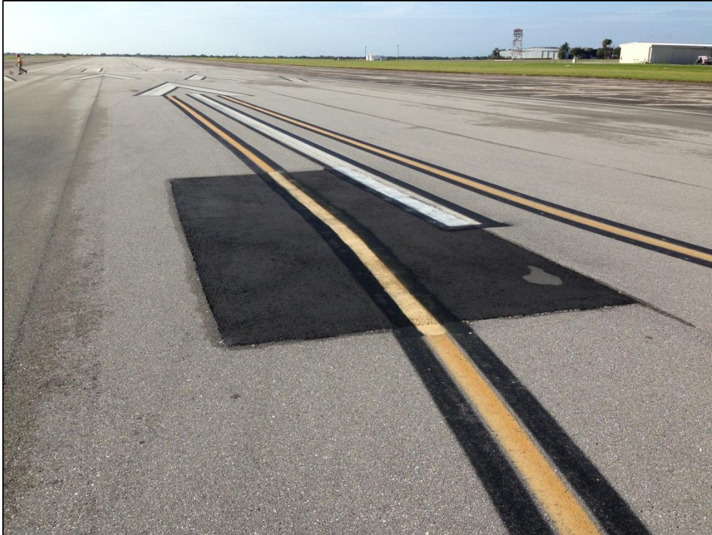
Runway 14-32, Section 6205, Sample Unit 198 –Low Severity (57) Weathering, Low Severity (50) Patch
