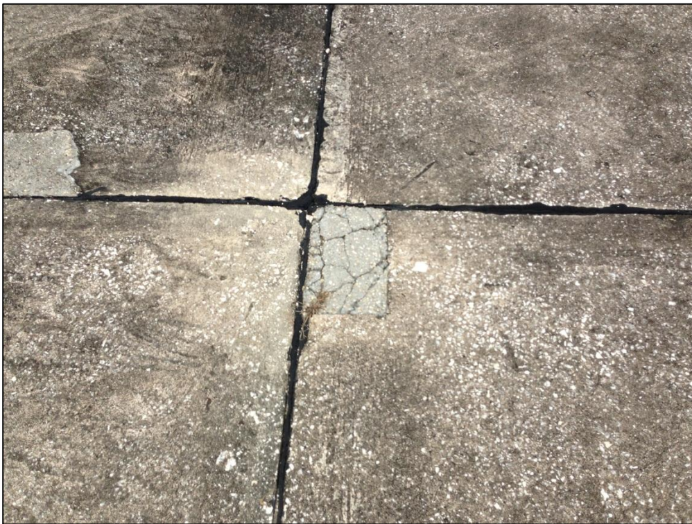
Apron West, Section 4105, Sample Unit 312 – Medium Severity (66) Patching, Low Severity (65) Joint Seal Damage
