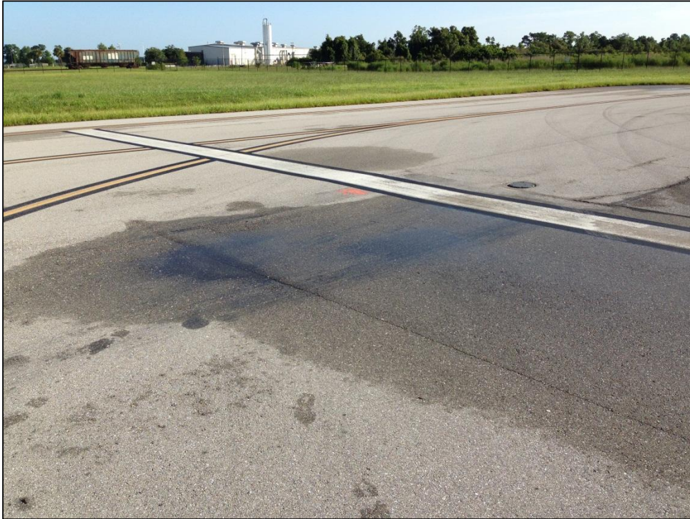
Runway 14-32, Section 6205, Sample Unit 198 – Low Severity (48) Longitudinal and Transverse Cracking, Low Severity (57) Weathering, Low Severity (45) Depression
