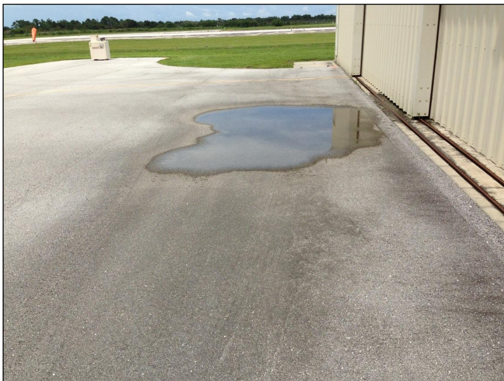
Apron West, Section 4115, Sample Unit 203 – Low Severity (48) Longitudinal and Transverse Cracking, Low Severity (52) Raveling, Low Severity (57) Weathering, Low Severity (45) Depression
