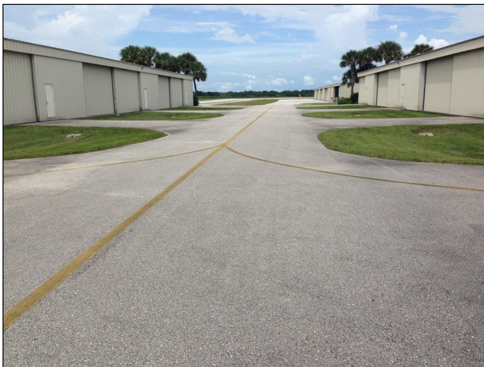
Taxiway T-Hangar, Section 505, Sample Unit 302 –Low and Medium Severity (57) Weathering
