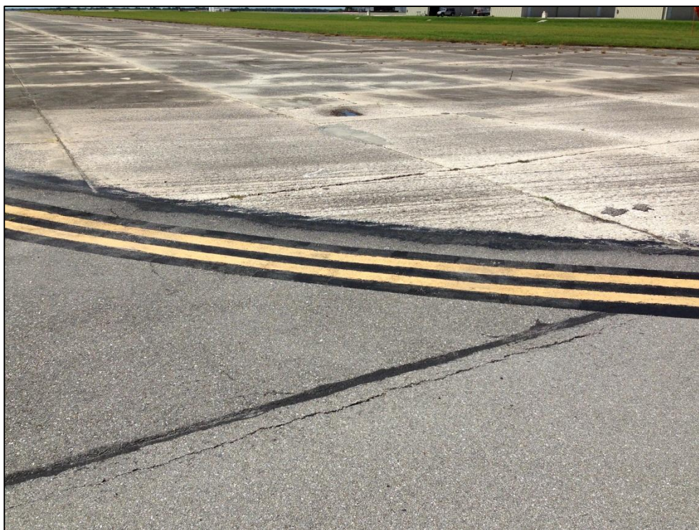
Taxiway Charlie, Section 305, Sample Unit 100 – Low Severity (57) Weathering, Low Severity (48) Longitudinal and Transverse Cracking
