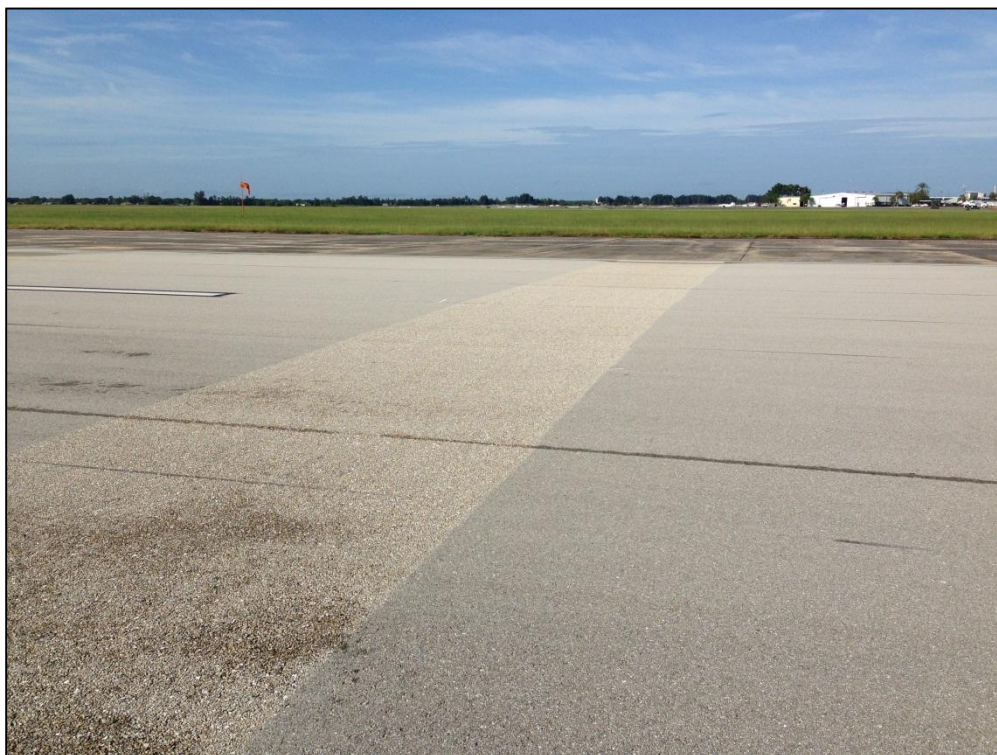
Runway 14-32, Section 6205, Sample Unit 149 – Low Severity (48) Longitudinal and Transverse Cracking, Low Severity (57) Weathering, Low Severity (52) Raveling
