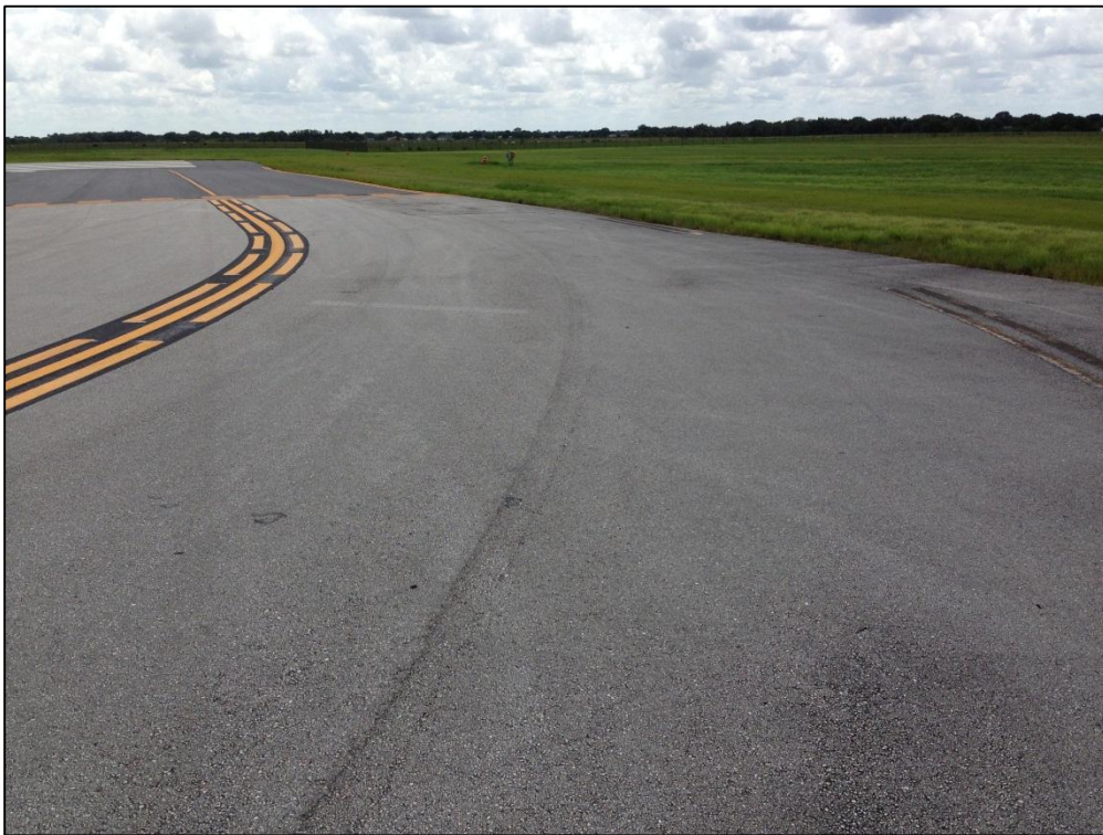
Taxiway A1, Section 605, Sample Unit 202 – Low Severity (57) Weathering, Low Severity (52) Raveling
