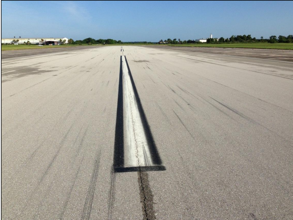
Runway 14-32, Section 6205, Sample Unit 177 – Low Severity (48) Longitudinal and Transverse Cracking, Low Severity (57) Weathering
