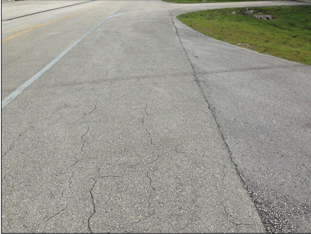
Taxiway T-Hangar, Section 505, Sample Unit 100 – Low Severity (48) Longitudinal and Transverse Cracking, Low Severity (57) Weathering, Low Severity (43) Block Cracking
