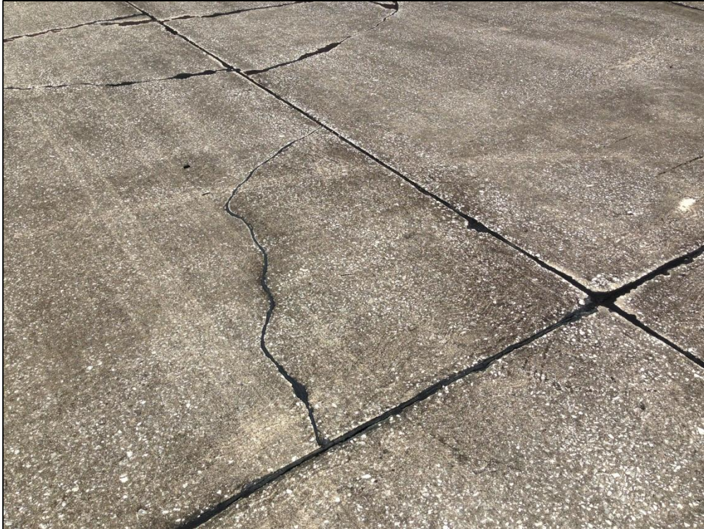
Apron West, Section 4105, Sample Unit 114 – Low Severity (62) Corner Break, Low Severity (70) Scaling, Map Cracking, Crazing, Low Severity (65) Joint Seal Damage
