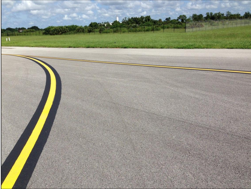
Apron RU, Section 415, Sample Unit 103 – Low Severity (57) Weathering
