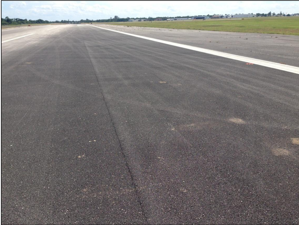
Runway 16-34, Section 6305, Sample Unit 390 – Low Severity (48) Longitudinal and Transverse Cracking, Low Severity (57) Weathering
