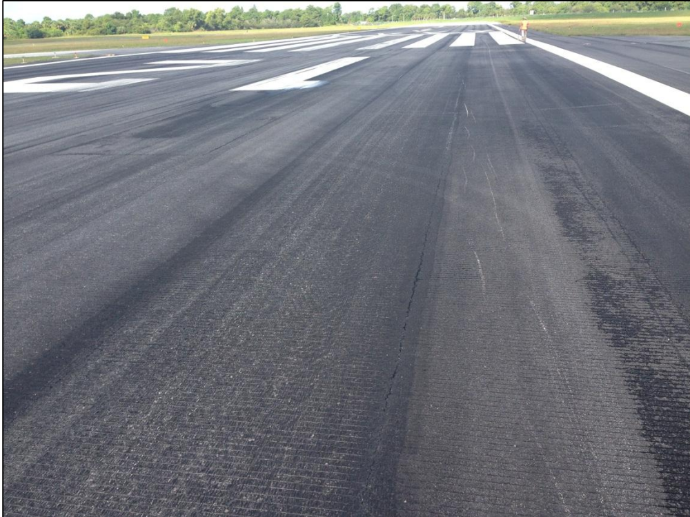
Runway 12-30, Section 6105, Sample Unit 301 – Low Severity (48) Longitudinal and Transverse Cracking, Low Severity (52) Raveling, Low Severity (57) Weathering
