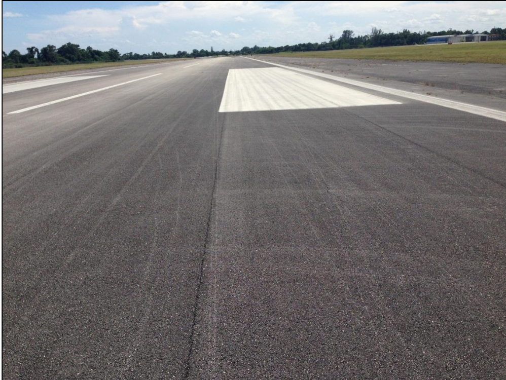
Runway 16-34, Section 6305, Sample Unit 341 – Low Severity (48) Longitudinal and Transverse Cracking, Low Severity (57) Weathering
