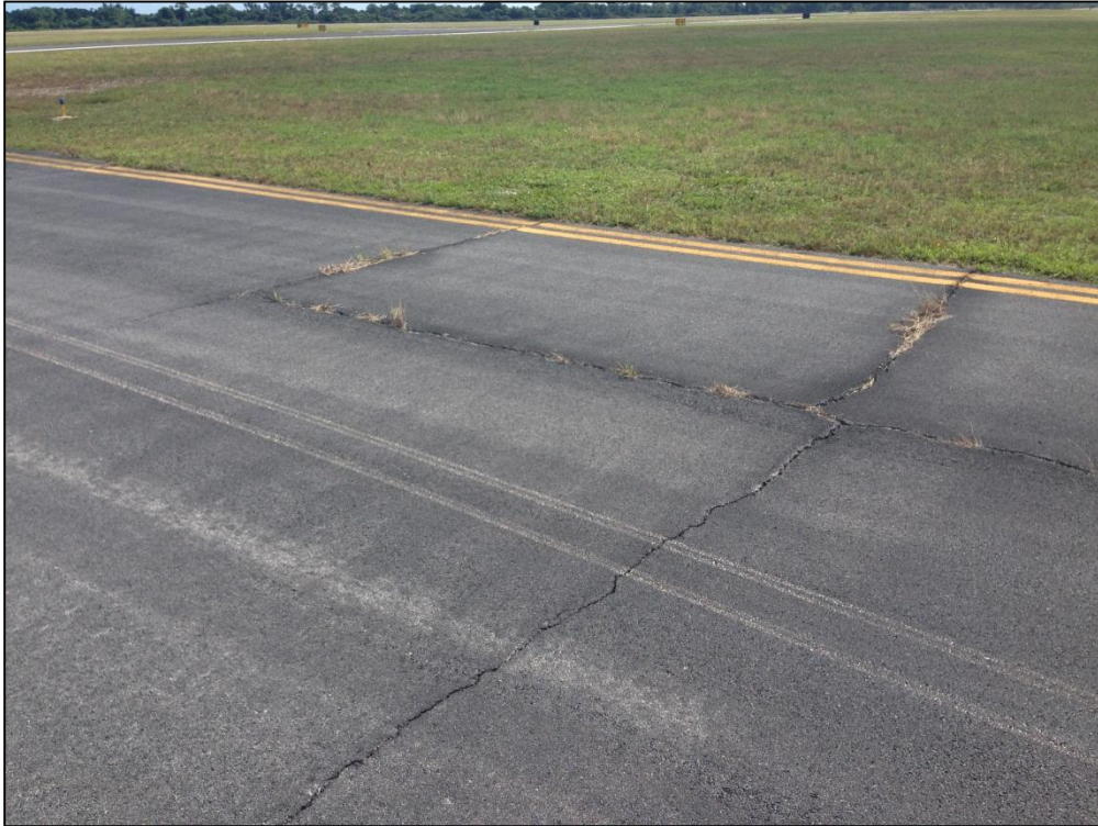
Taxiway B, Section 208, Sample Unit 200 – Medium Severity (43) Block Cracking, Low Severity (52) Raveling, Low Severity (57) Weathering
