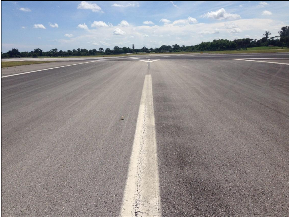
Runway 16-34, Section 6305, Sample Unit 310 – Low Severity (48) Longitudinal and Transverse Cracking, Low Severity (57) Weathering
