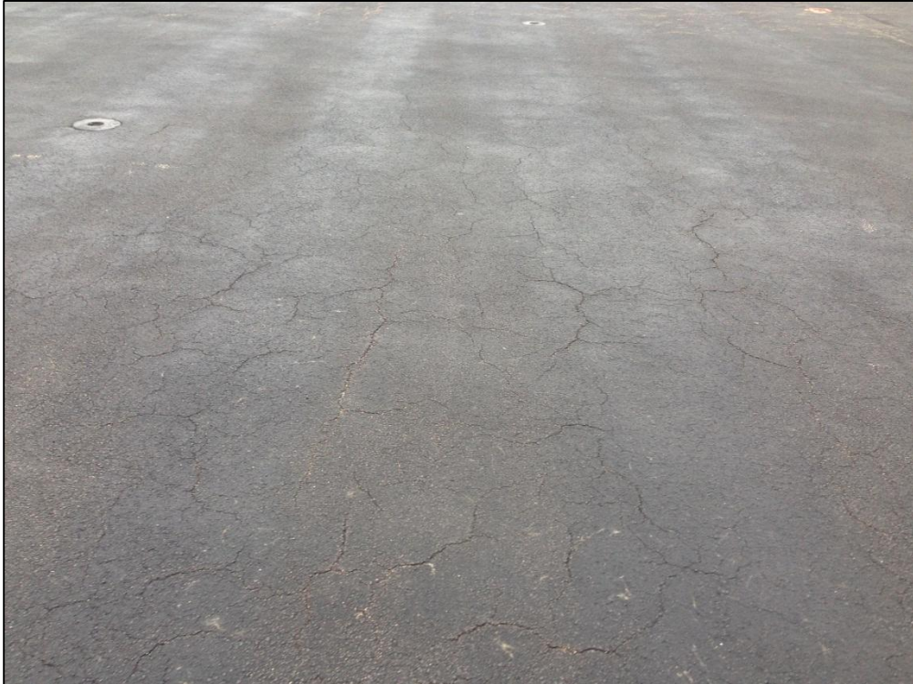
Apron E, Section 4205, Sample Unit 208 – Low Severity (43) Block Cracking, Low Severity (57) Weathering
