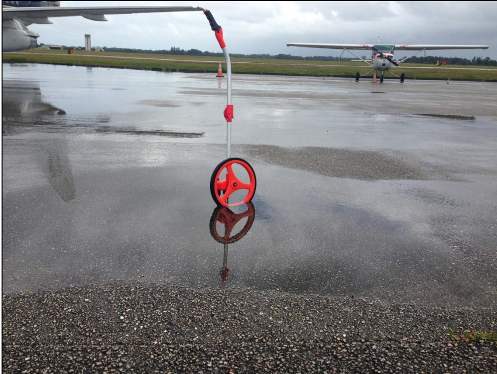
Apron W, Section 4120, Sample Unit 700 – High Severity (45) Depression, Low Severity (48) Longitudinal and Transverse Cracking, Low Severity (57) Weathering
