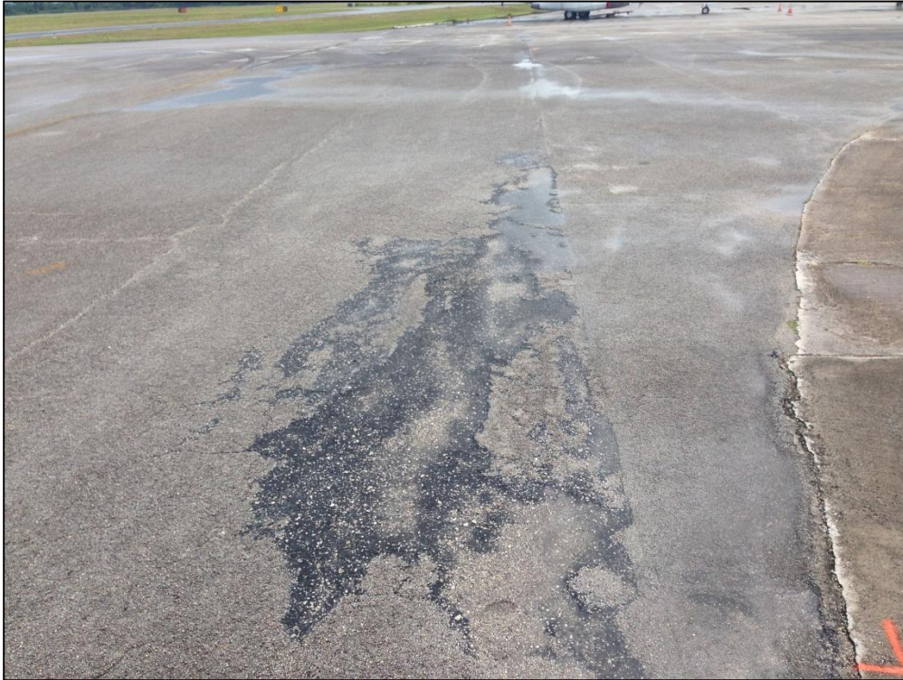
Apron W, Section 4105, Sample Unit 300 – Low Severity (43) Block Cracking, Low Severity (57) Weathering, High Severity (52) Raveling
