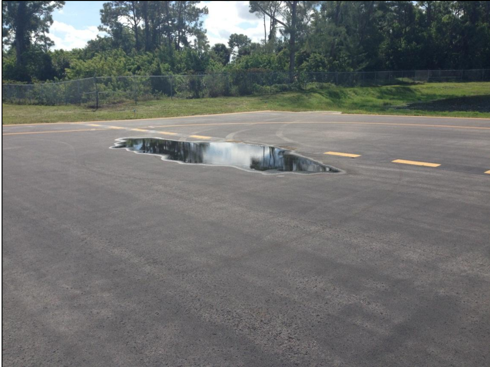
Taxiway D, Section 412, Sample Unit 101 – Low Severity (45) Depression, Low Severity (48) Longitudinal and Transverse Cracking, Low Severity (57) Weathering
