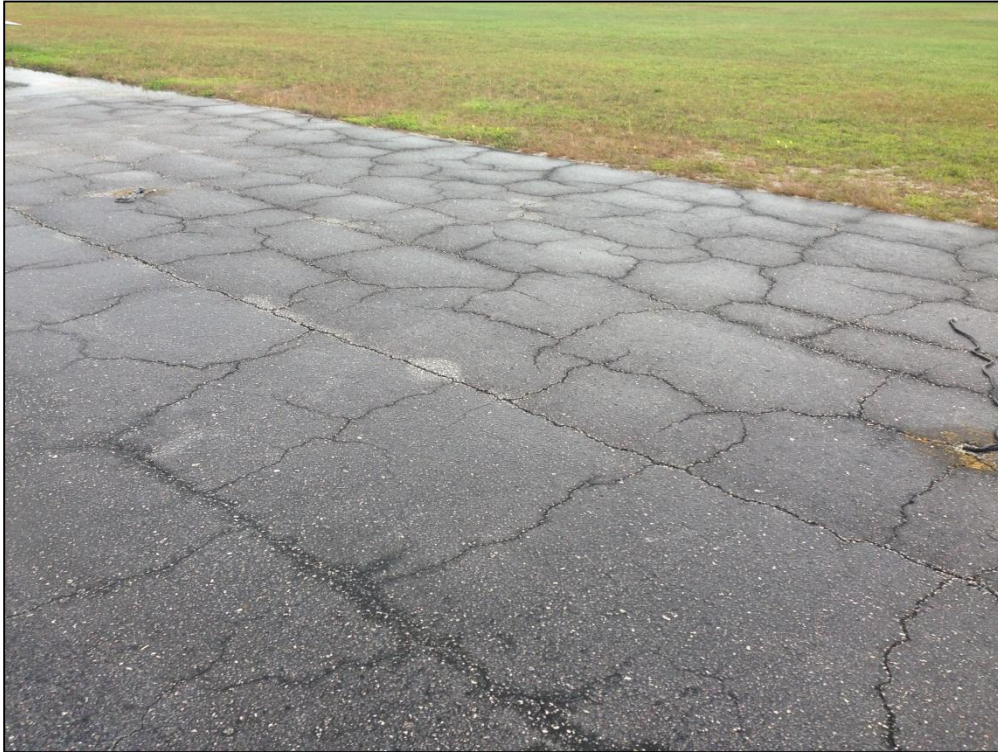
Apron E, Section 4235, Sample Unit 54 – Low Severity (43) Block Cracking, Low Severity (57) Weathering, Low Severity (52) Raveling
