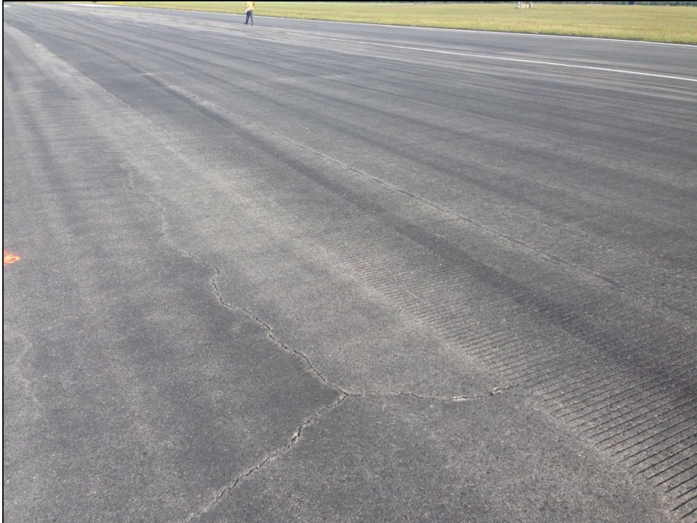
Runway 7-25, Section 6205, Sample Unit 315 – Low Severity (48) Longitudinal and Transverse Cracking, Low Severity (57) Weathering
