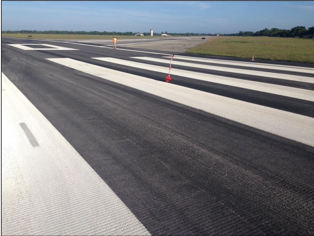
Runway 12-30, Section 6120, Sample Unit 400 – Low Severity (52) Raveling, Low Severity (57) Weathering
