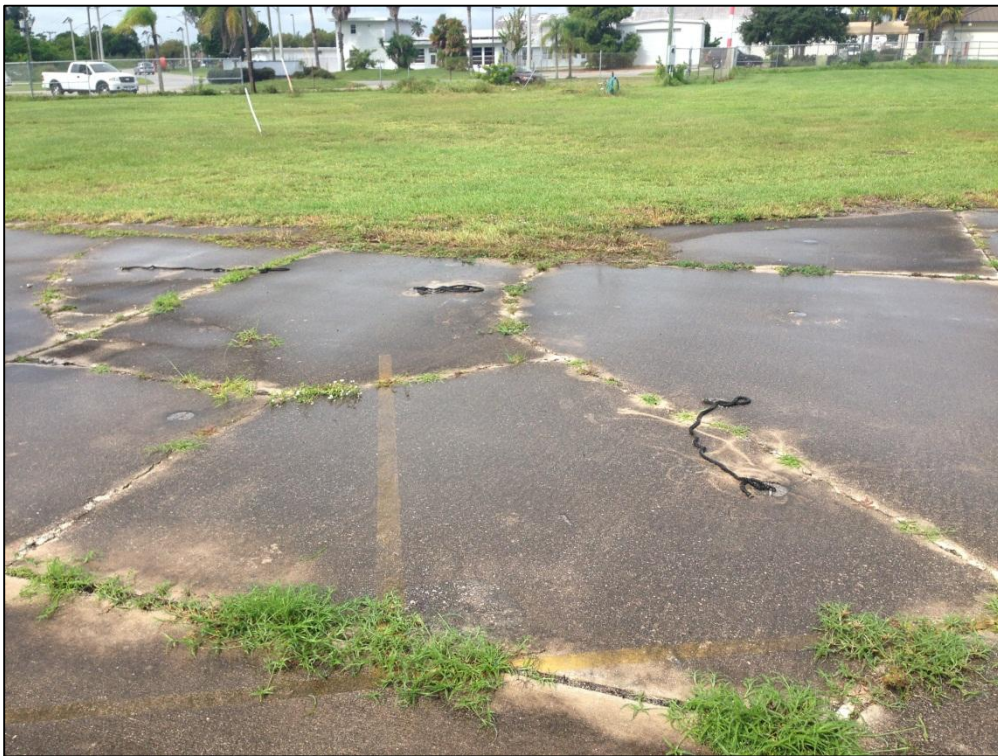
Apron W, Section 4110, Sample Unit 404 – High Severity (65) Joint Seal Damage, Medium Severity (72) Shattered Slab
