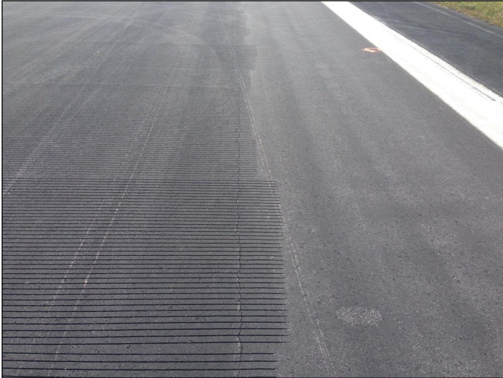
Runway 7-25, Section 6205, Sample Unit 354 – Low Severity (48) Longitudinal and Transverse Cracking, Low Severity (57) Weathering
