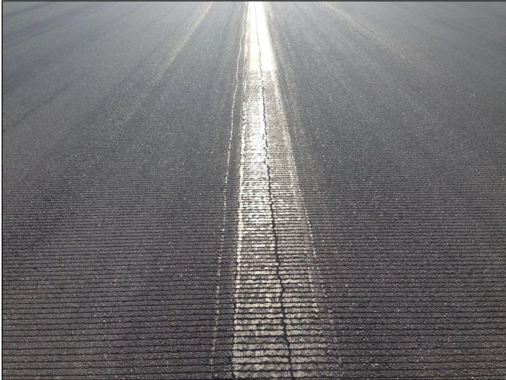
Runway 12-30, Section 6105, Sample Unit 357 – Low Severity (48) Longitudinal and Transverse Cracking, Low Severity (57) Weathering
