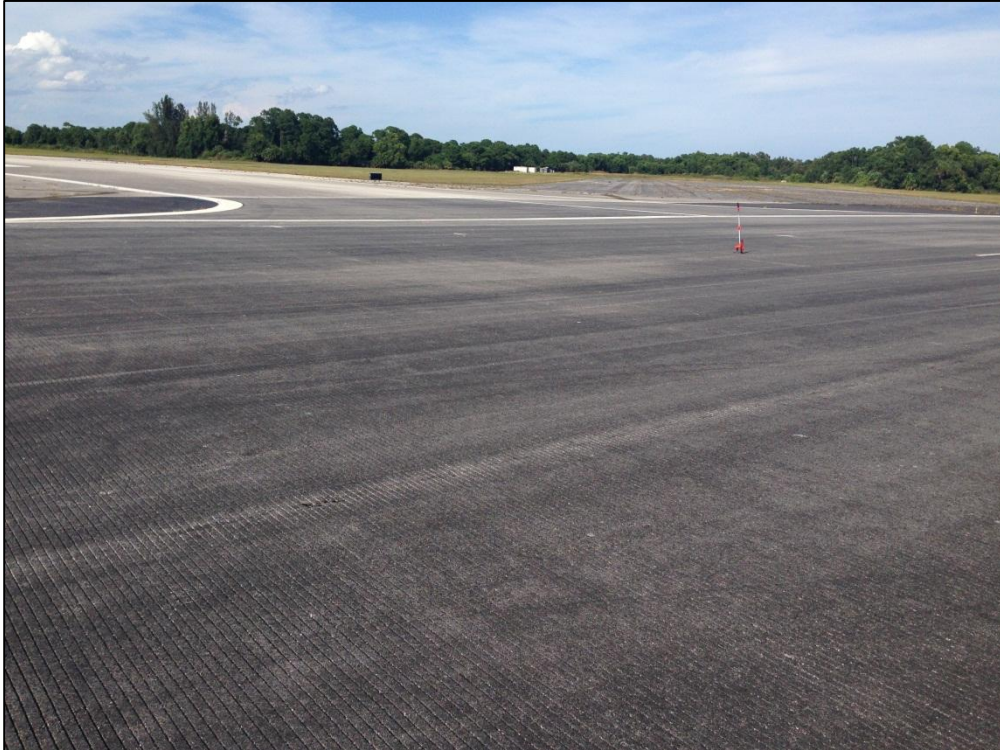
Runway 7-25, Section 6205, Sample Unit 368 – Low Severity (57) Weathering
