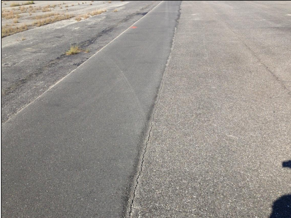
Apron N, Section 4105, Sample Unit 115 – Low Severity (48) Longitudinal and Transverse Cracking, Low Severity (52) Raveling, Medium Severity (57) Weathering, Low Severity (50) Patching
