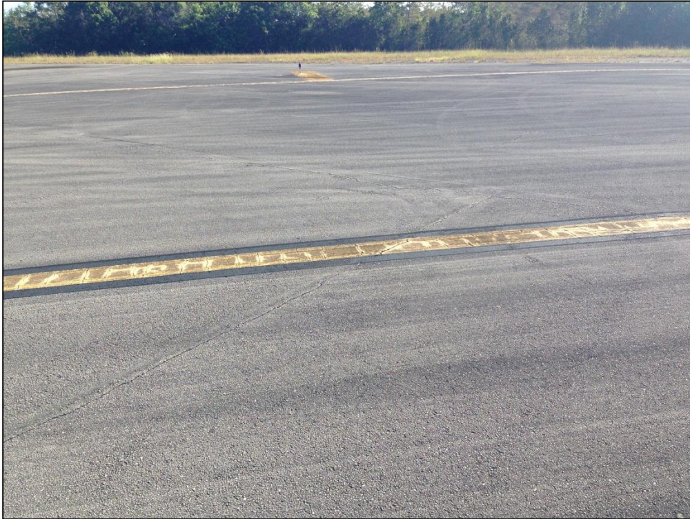
Taxiway B, Section 210, Sample Unit 100 – Low Severity (48) Longitudinal and Transverse Cracking, Low Severity (57) Weathering
