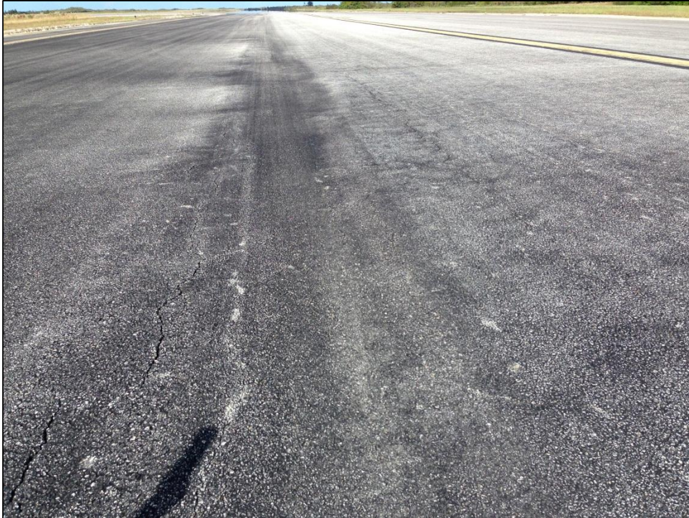
Taxiway A, Section 105, Sample Unit 237 – Low Severity (53) Rutting, Medium Severity (57) Weathering
