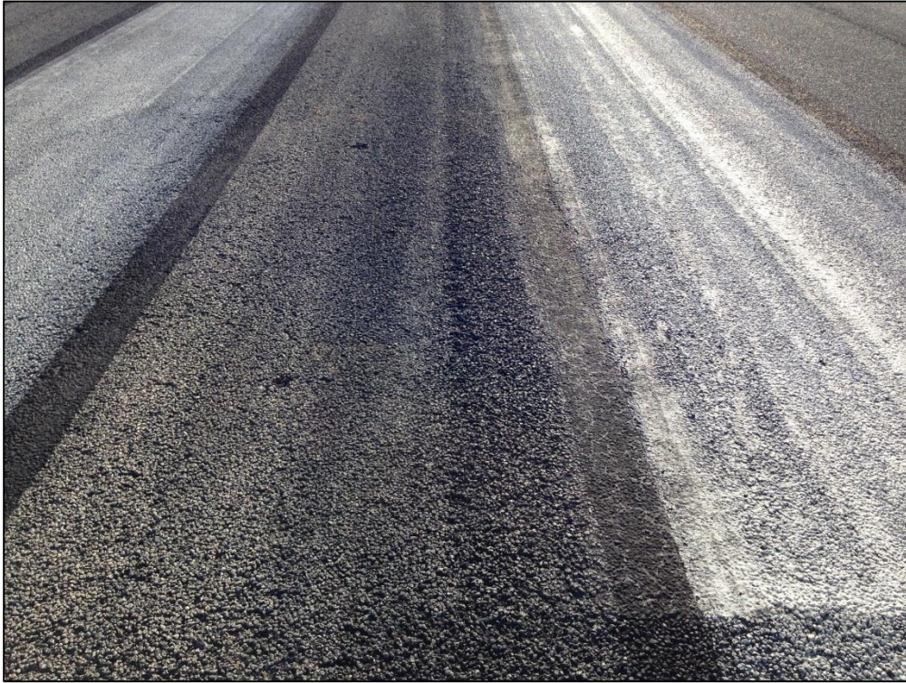
Runway 9-27, Section 6105, Sample Unit 403 – Medium Severity (57) Weathering, Low Severity (52) Raveling
