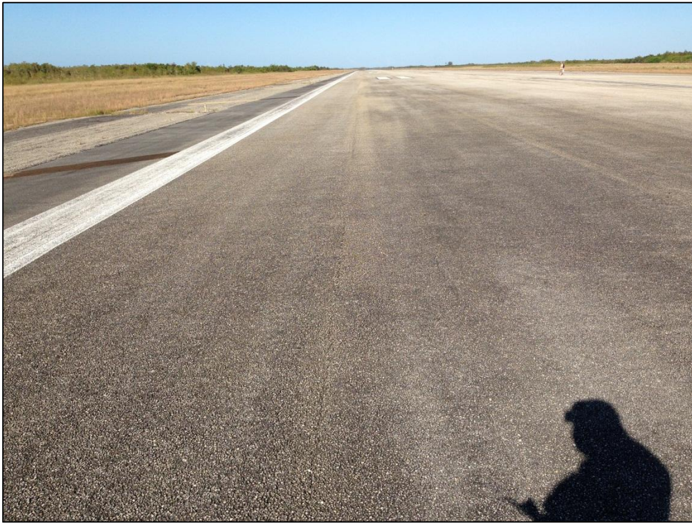
Runway 9-27, Section 6105, Sample Unit 592 – Low Severity (48) Longitudinal and Transverse Cracking, Medium Severity (57) Weathering, Low Severity (52) Raveling
