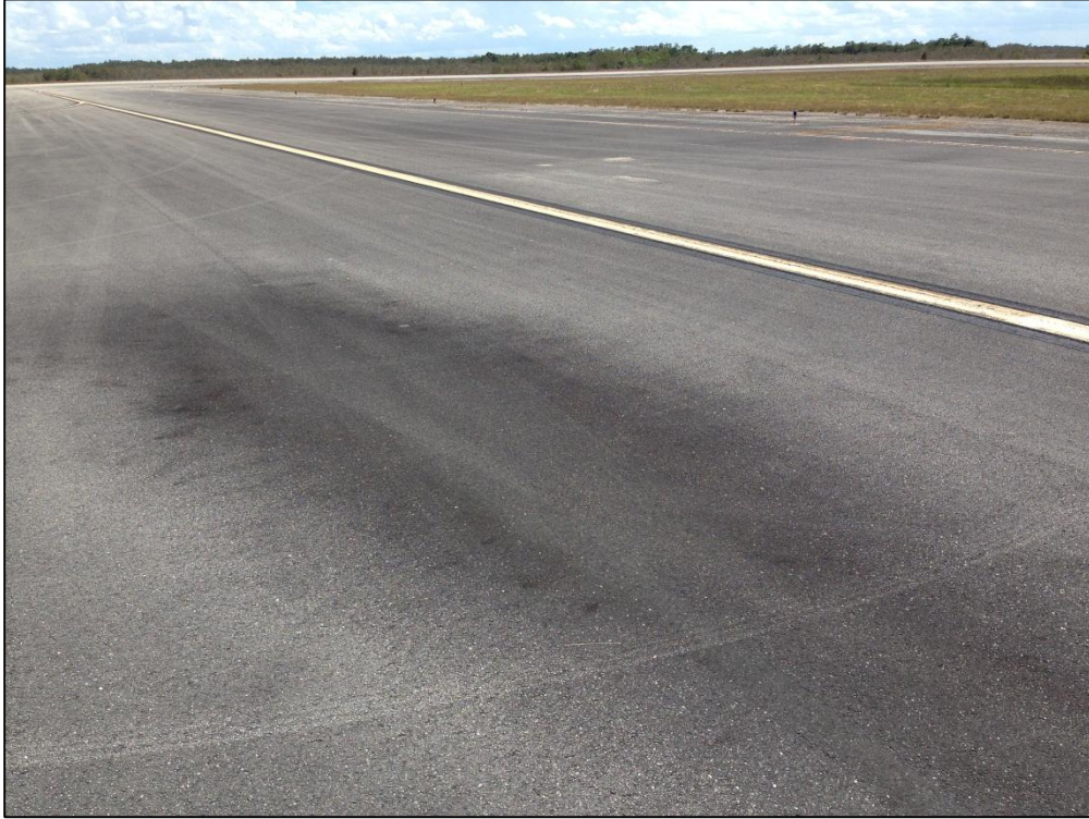
Taxiway A2, Section 130, Sample Unit 214 – Low Severity (45) Depression, Low Severity (57) Weathering
