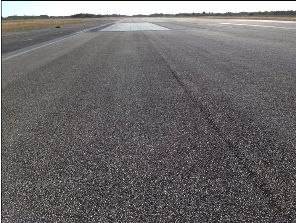
Runway 9-27, Section 6105, Sample Unit 192 – Low Severity (48) Longitudinal and Transverse Cracking, Medium Severity (57) Weathering, Low Severity (52) Raveling
