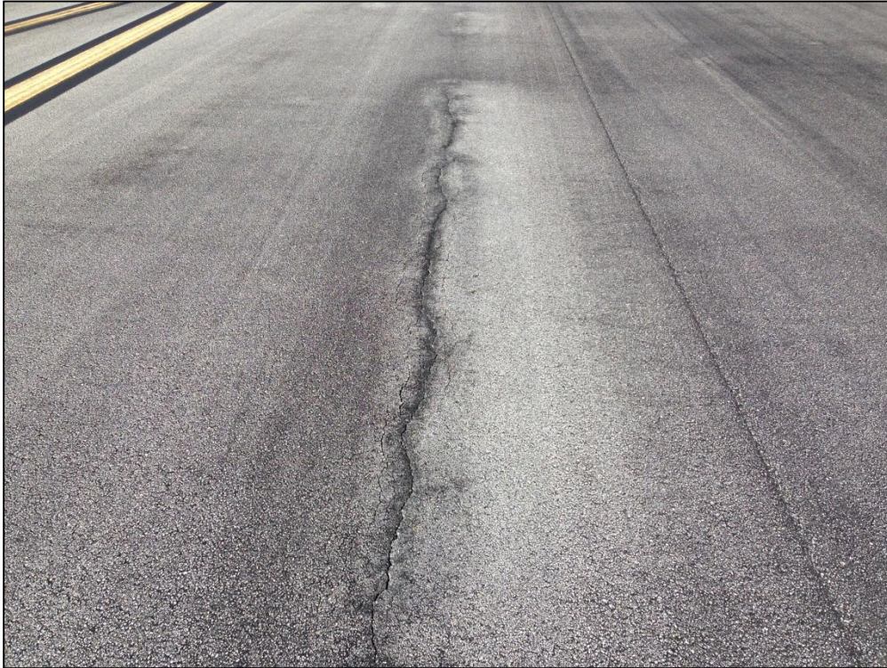
Taxiway A, Section 105, Sample Unit 261 – Low Severity (48) Longitudinal and Transverse Cracking, Medium Severity (56) Swelling, Medium Severity (57) Weathering
