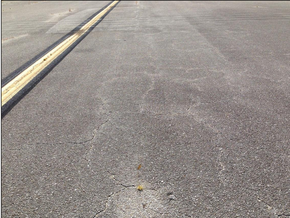
Taxiway A6, Section 170, Sample Unit 608 – Low Severity (48) Longitudinal and Transverse Cracking, Low Severity (43) Block Cracking, Medium Severity (57) Weathering
