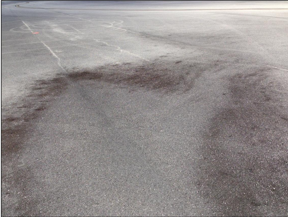
Taxiway A4, Section 150, Sample Unit 435 – Low Severity (45) Depression, Low Severity (48) Longitudinal and Transverse Cracking, Medium Severity (57) Weathering
