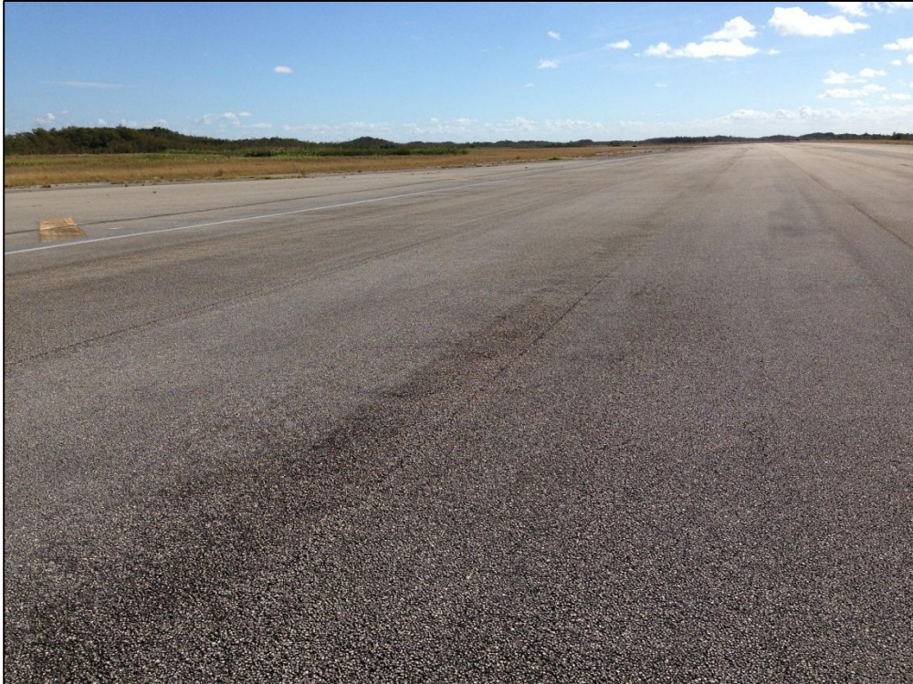
Runway 9-27, Section 6105, Sample Unit 168 – Low Severity (48) Longitudinal and Transverse Cracking, Medium Severity (57) Weathering, Low Severity (52) Raveling, Low Severity (56) Swelling
