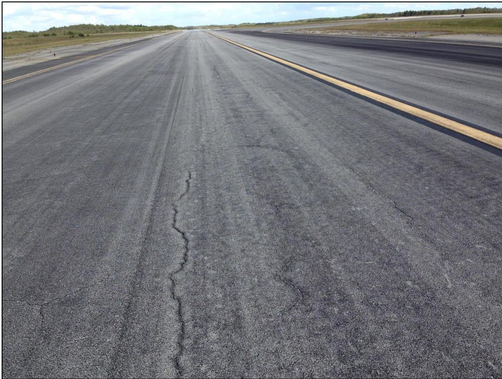
Taxiway A, Section 105, Sample Unit 159 – Low Severity (43) Block Cracking, Low Severity (56) Swelling, Low Severity (57) Weathering
