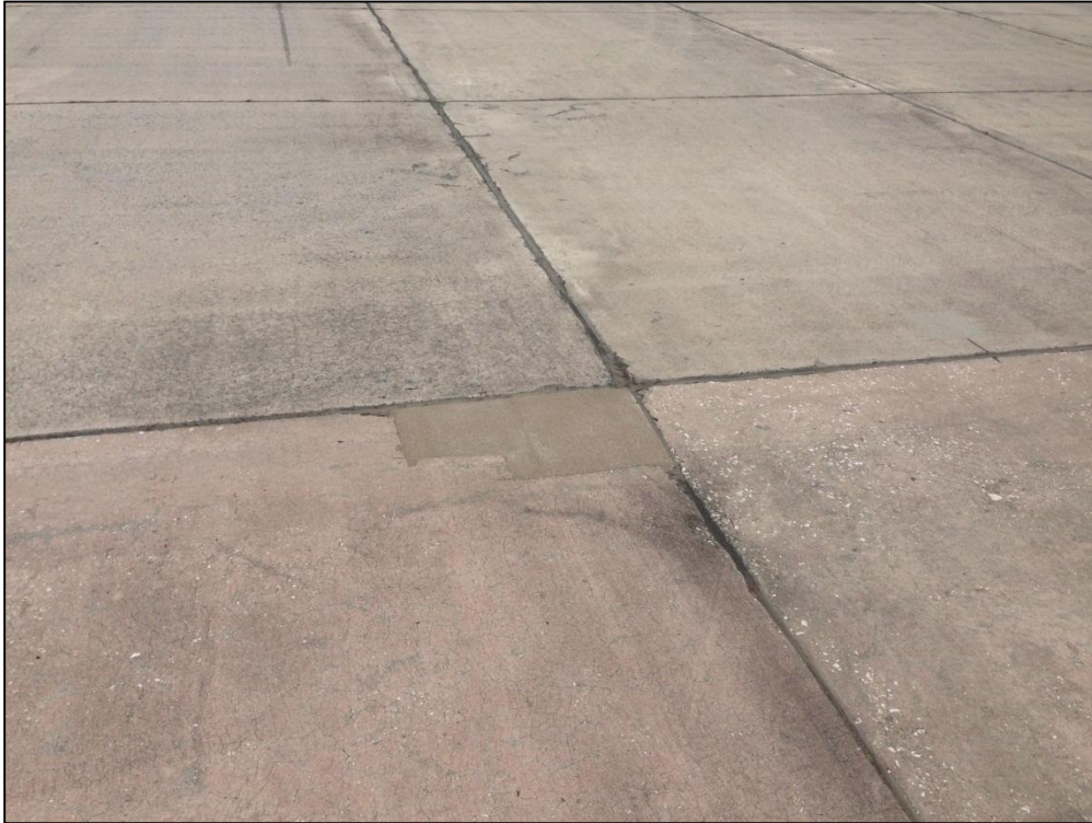
Runway 18L-36R, Section 6235, Sample Unit 384 – Low Severity (70) Map Cracking, Low Severity (66) Patching
