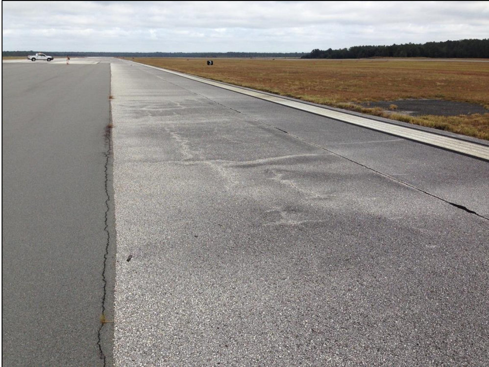
Runway 9L-27R, Section 6420, Sample Unit 709 – Low Severity (43) Block Cracking, Low Severity (48) Longitudinal and Transverse Cracking, Low Severity (52) Raveling, Low Severity (52) Swelling, Low Severity (57) Weathering
