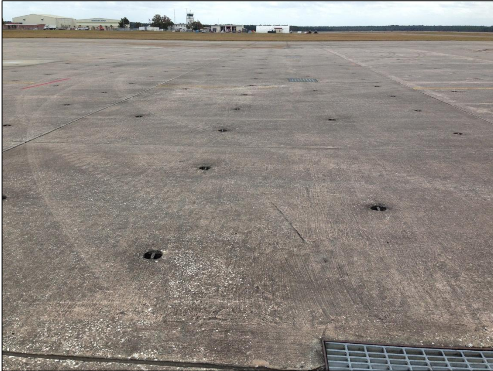
Apron West, Section 4210, Sample Unit 253 –Low Severity (70) Map Cracking
