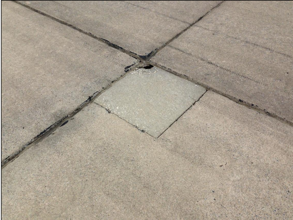
Runway 9L-27R, Section 6410, Sample Unit 702 – Low Severity (70) Map Cracking, Medium Severity (66) Small Patching
