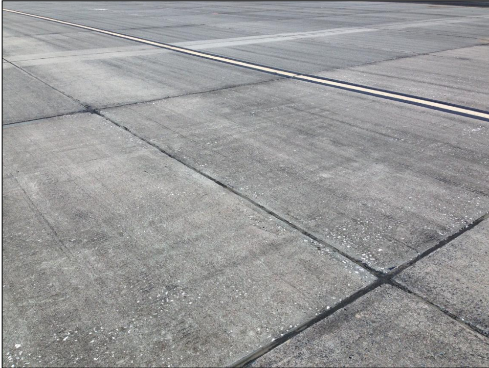
Taxiway A4, Section 805, Sample Unit 501 – Low Severity (70) Map Cracking
