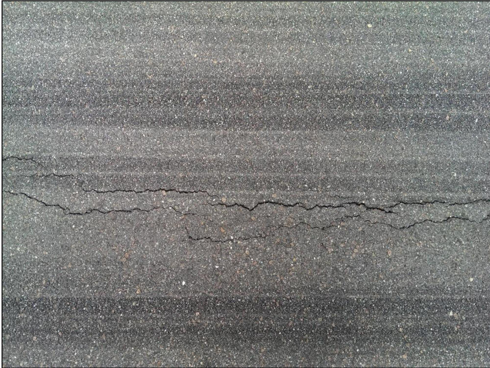
Runway 9L-27R, Section 6414, Sample Unit 511 – Low Severity (41) Alligator Cracking
