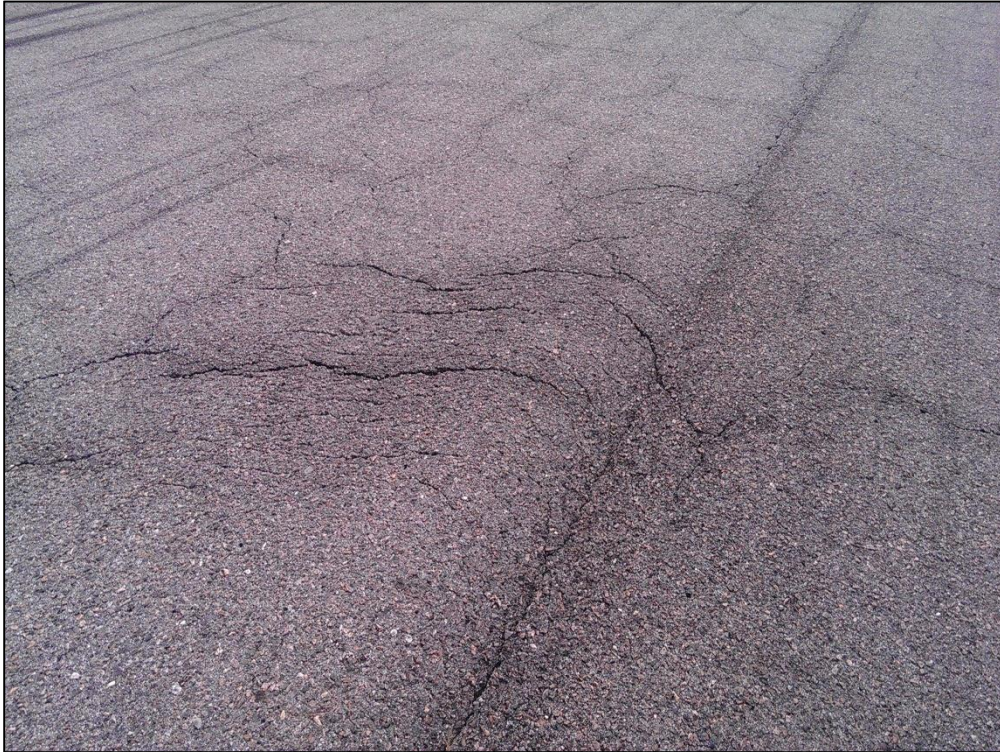
Runway 18R-36L, Section 6115, Sample Unit 313 – (55) Slippage Cracking, Low Severity (52) Raveling, Low Severity (57) Weathering
