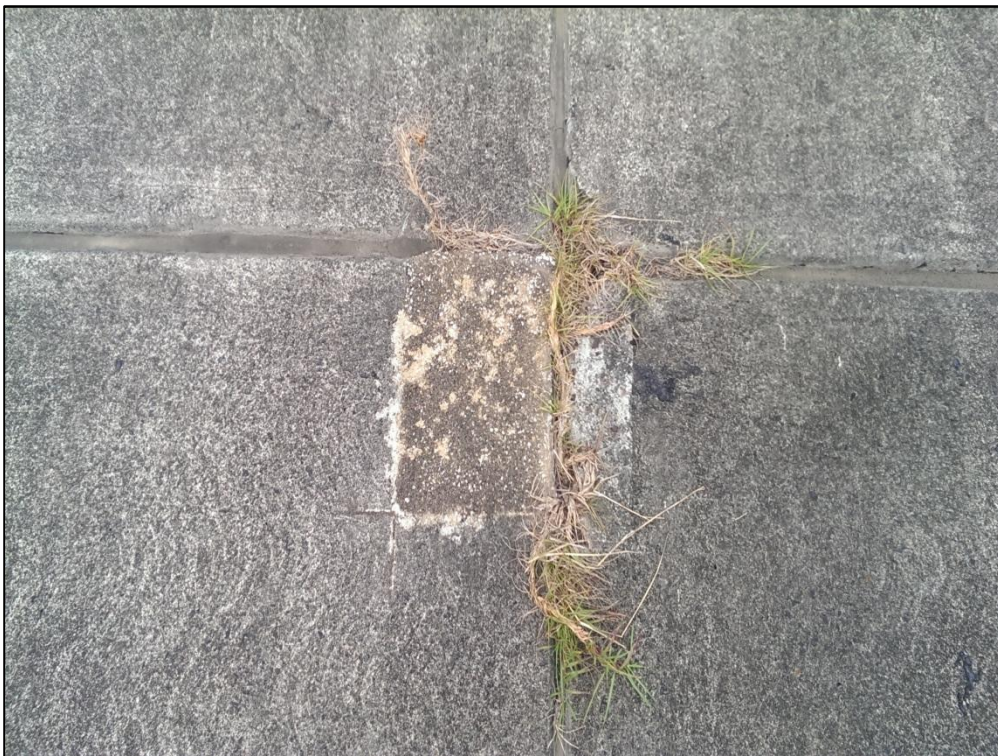
Taxiway B, Section 205, Sample Unit 148 – Low Severity (70) Map Cracking, Low Severity (66) Small Patching
