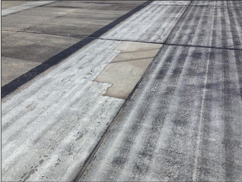
Runway 18R-36L, Section 6110, Sample Unit 101 – Low Severity (67) Large Patching, Low Severity (70) Map Cracking
