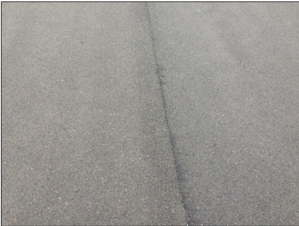
Runway 9R-27L, Section 6320, Sample Unit 741 – Low Severity (48) Longitudinal and Transverse Cracking
