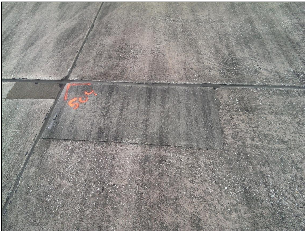
Runway 9R-27L, Section 6305, Sample Unit 504 – Low Severity (70) Map Cracking, Low Severity (66) Small Patching
