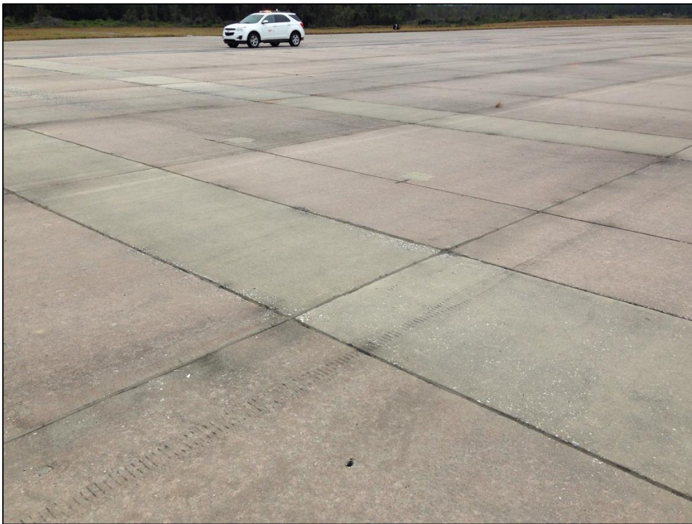
Runway 18L-36R, Section 6240, Sample Unit 797 – Low Severity (70) Map Cracking, Low Severity (66) Small Patching, Low Severity (67) Large Patching
