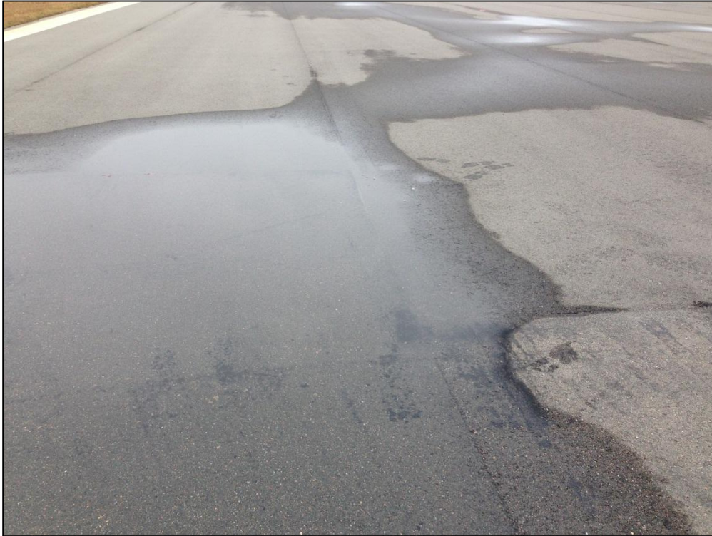
Runway 9R-27L, Section 6320, Sample Unit 154 – Low Severity (48) Longitudinal and Transverse Cracking, Low Severity (45) Depression
