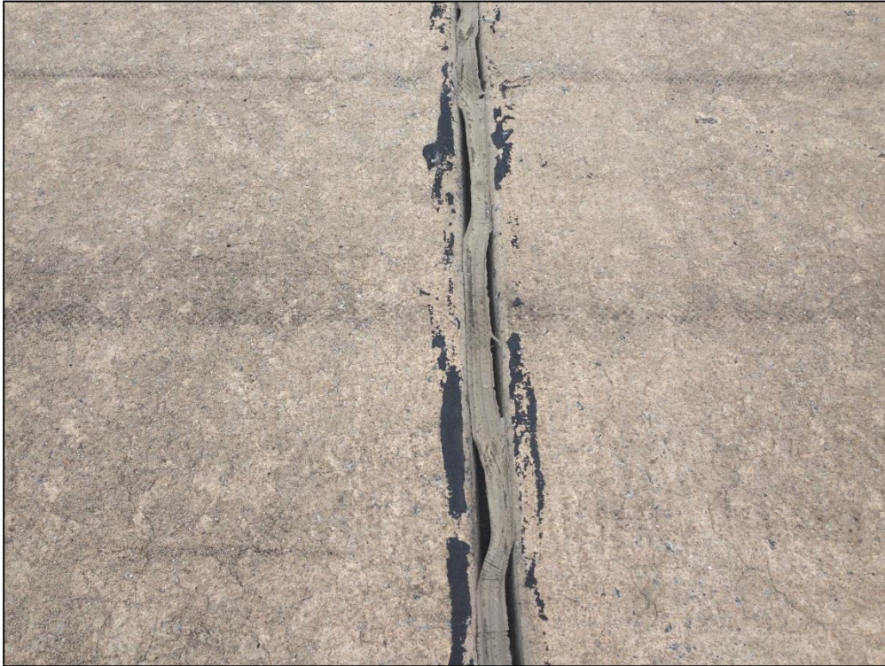
Runway 9L-27R, Section 6410, Sample Unit 105 – Medium Severity (65) Joint Seal Damage, Low Severity (70) Map Cracking
