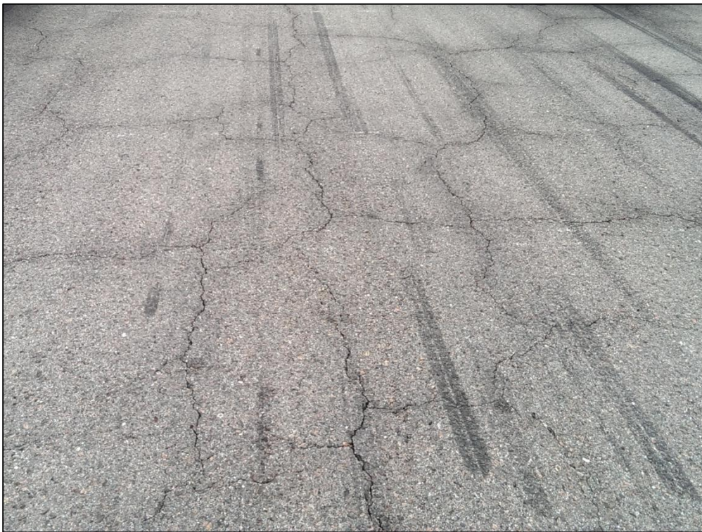
Runway 18R-36L, Section 6115, Sample Unit 369 – Low Severity (43) Block Cracking, Low Severity (52) Raveling, Low Severity (57) Weathering
