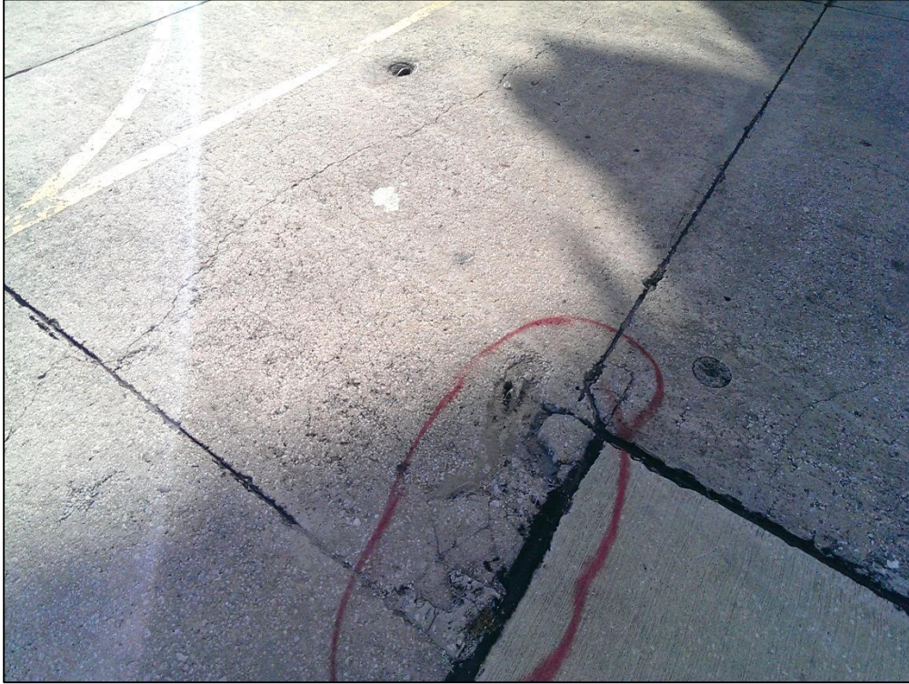
Apron North, Section 4110, Sample Unit 407 – Medium Severity (70) Map Cracking, Low Severity (63) Longitudinal, Transverse, and Diagonal Cracking, High Severity (75) Corner Spalling
