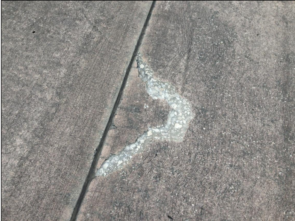
Taxiway A, Section 105, Sample Unit 302 – Low Severity (70) Map Cracking, High Severity (74) Joint Spalling
