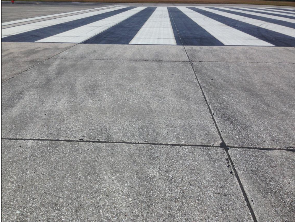
Runway 9R-27L, Section 6340, Sample Unit 183 – Low Severity (70) Map Cracking
