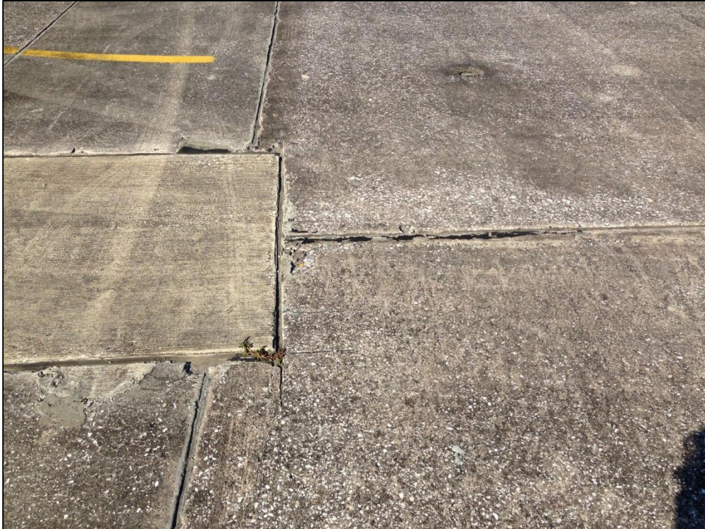
Apron North, Section 4120, Sample Unit 288 – Low Severity (65) Joint Seal Damage, Low Severity (70) Map Cracking, Low Severity (66) Small Patching
