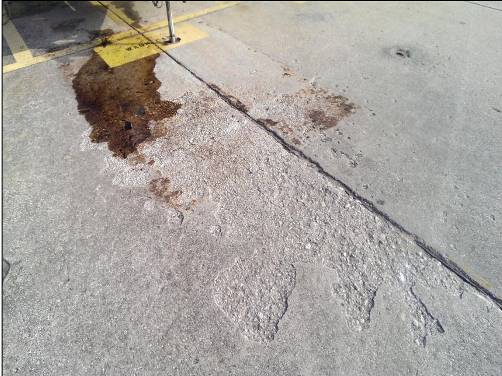
Apron North, Section 4110, Sample Unit 411 – High Severity (70) Map Cracking, Low Severity (65) Joint Seal Damage
