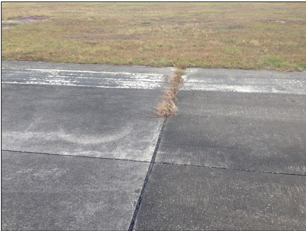
Runway 18R-36L, Section 6130, Sample Unit 474 – Medium Severity (65) Joint Seal Damage
