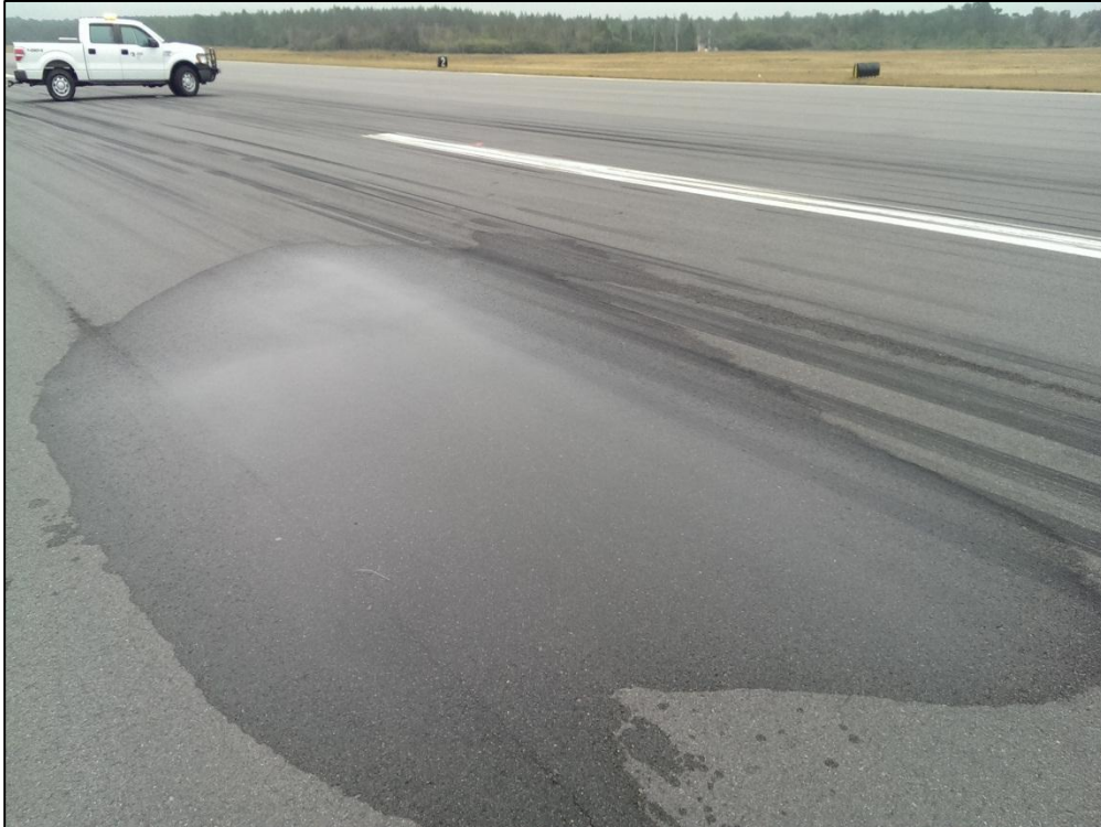
Runway 9R-27L, Section 6315, Sample Unit 359 – Low Severity (48) Longitudinal and Transverse Cracking, Low Severity (45) Depression
