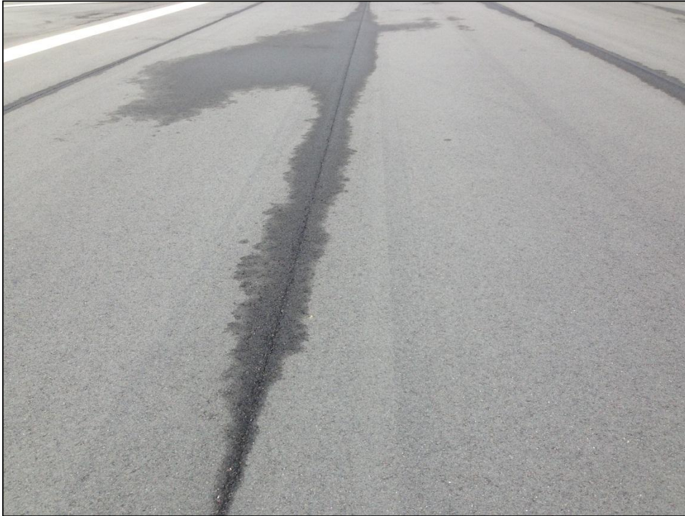
Runway 18L-36R, Section 6220, Sample Unit 773 – Low Severity (48) Longitudinal and Transverse Cracking
