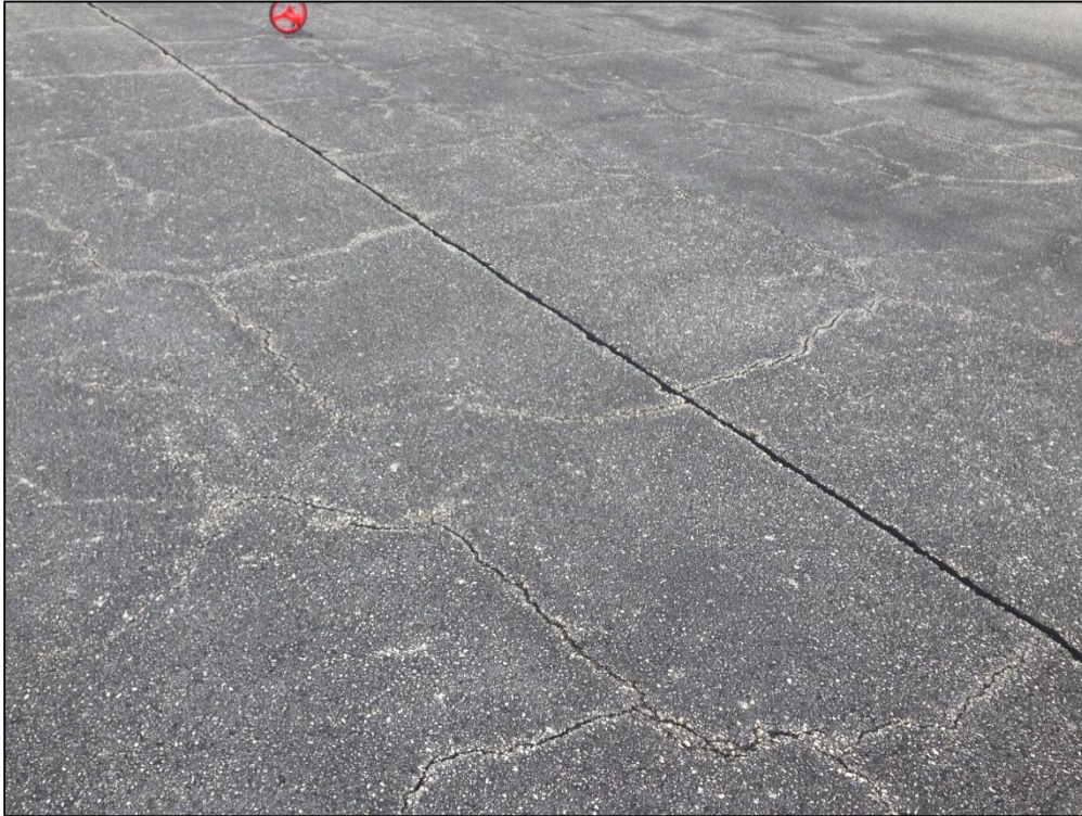
Runway 9L-27R, Section 6420, Sample Unit 126 – Low Severity (43) Block Cracking, Low Severity (52) Raveling, Low Severity (52) Swelling, Low Severity (57) Weathering
