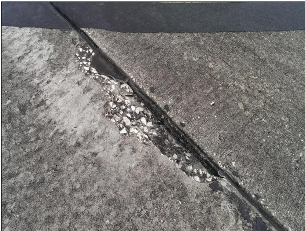
Apron West, Section 4250, Sample Unit 453 – Low Severity (70) Map Cracking, Low Severity (74) Joint Spalling
