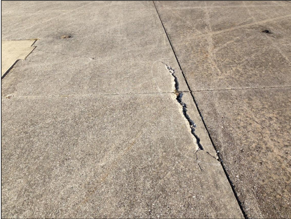
Apron North, Section 4110, Sample Unit 211 – Low Severity (70) Map Cracking, Medium Severity (62) Corner Break, Low Severity (67) Large Patching
