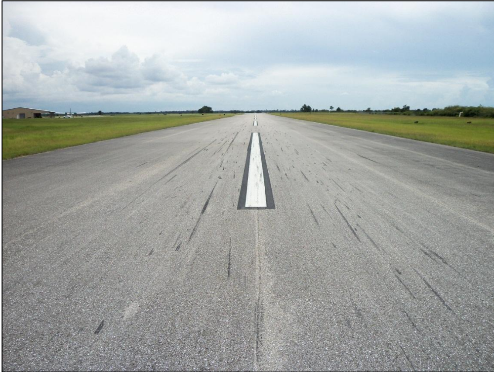
Runway 17-35, Section 6205, Sample Unit 170 – Low Severity (48) Longitudinal and Transverse Cracking, Low Severity (57) Weathering, Low Severity (52) Raveling
