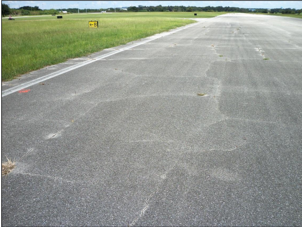
Runway 6-24, Section 6105, Sample Unit 145 – Medium Severity (57) Weathering, Low Severity (52) Raveling, Low Severity (43) Block Cracking
