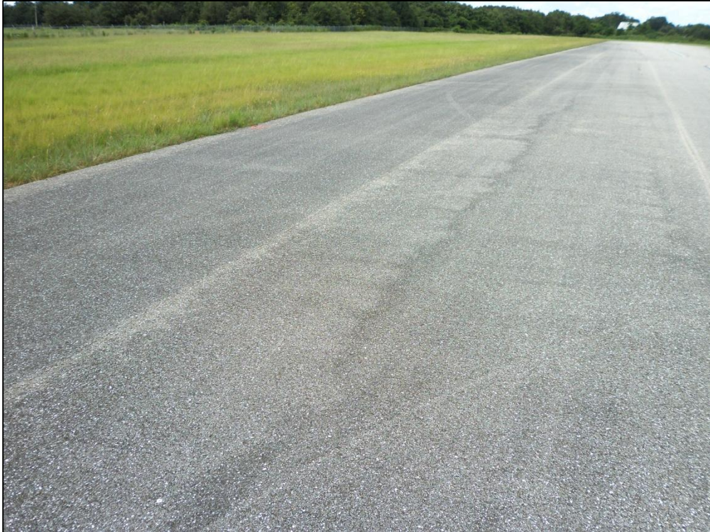
Runway 17-35, Section 6205, Sample Unit 166 – Low Severity (57) Weathering, Low Severity (52) Raveling, Low Severity (56) Swelling
