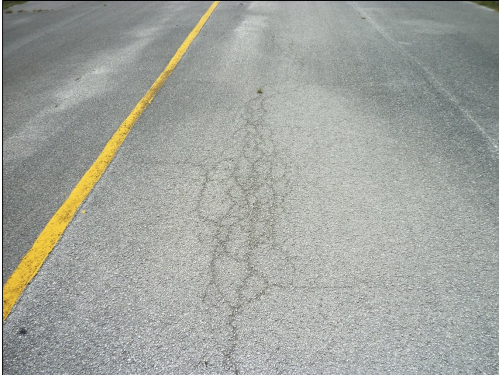
Taxiway A, Section 105, Sample Unit 104 – Medium Severity (52) Raveling, Low Severity (41) Alligator Cracking
