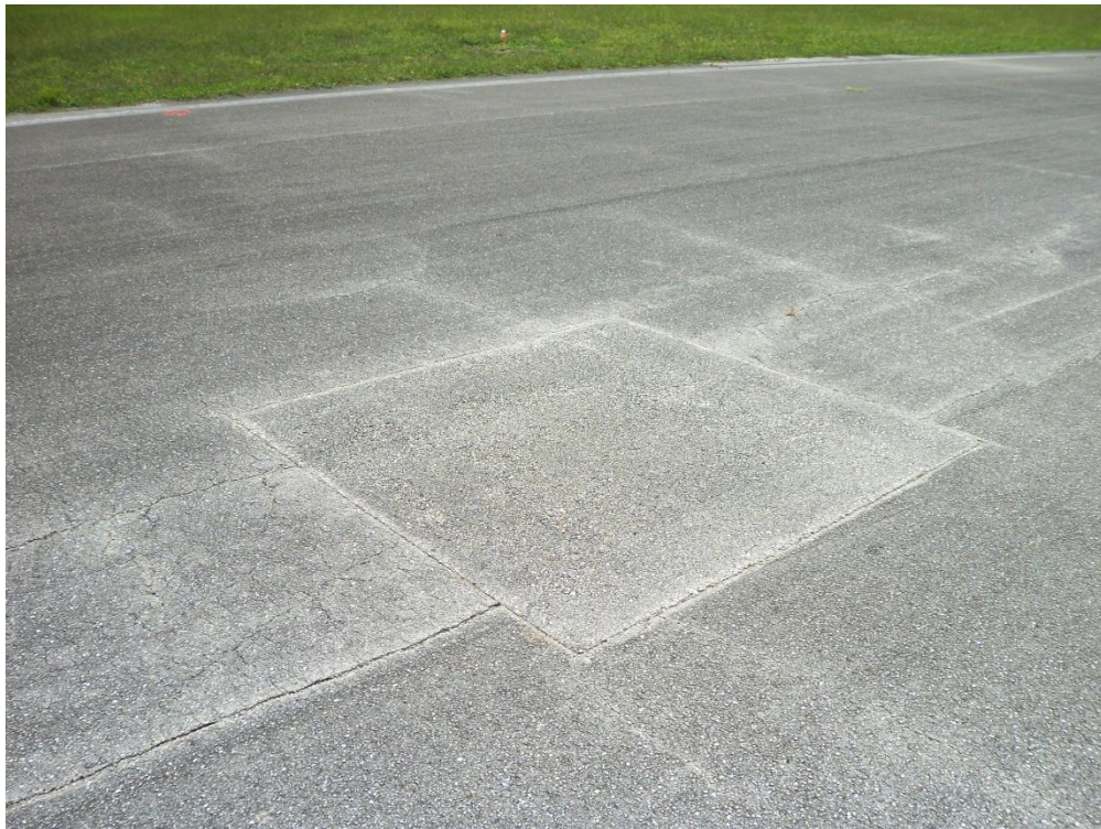
Runway 6-24, Section 6105, Sample Unit 154 – Low Severity (48) Longitudinal and Transverse Cracking, Medium Severity (57) Weathering, Low Severity (52) Raveling, Low Severity (50) Patching
