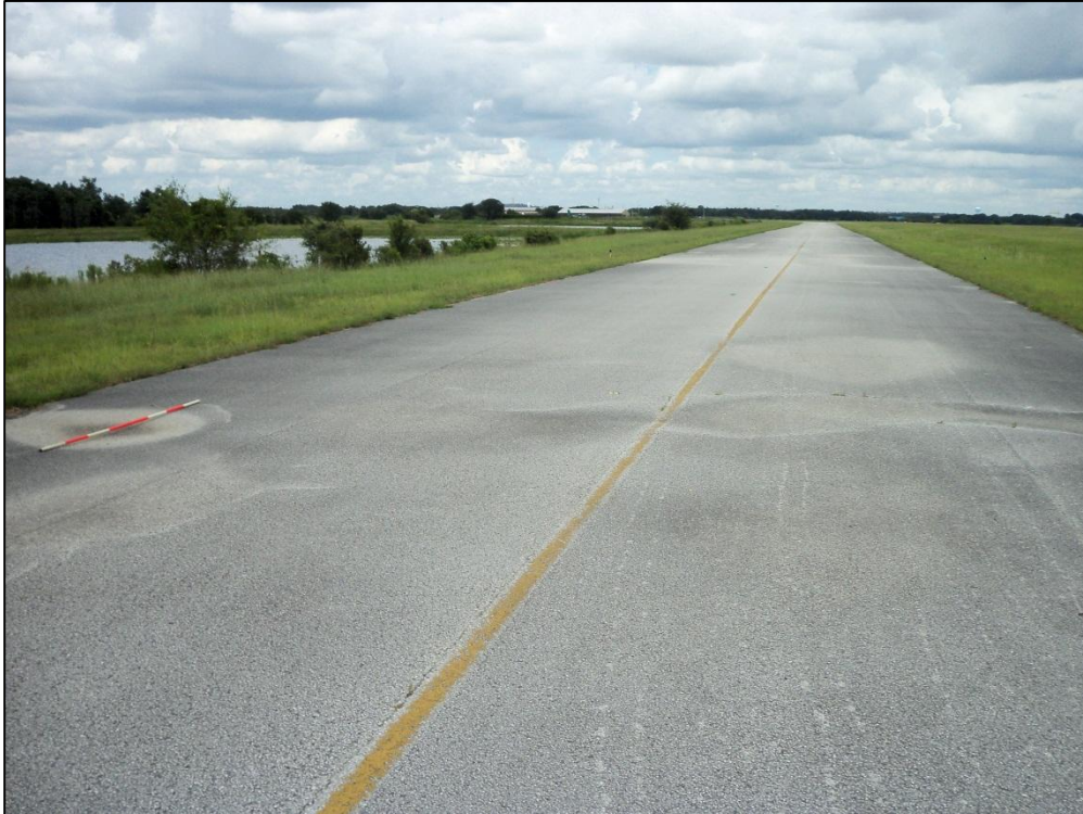
Taxiway D, Section 410, Sample Unit 102 – Low Severity (48) Longitudinal and Transverse Cracking, Low Severity (52) Raveling, Medium Severity (57) Weathering, Low, Medium, and High Severity (45) Depression
