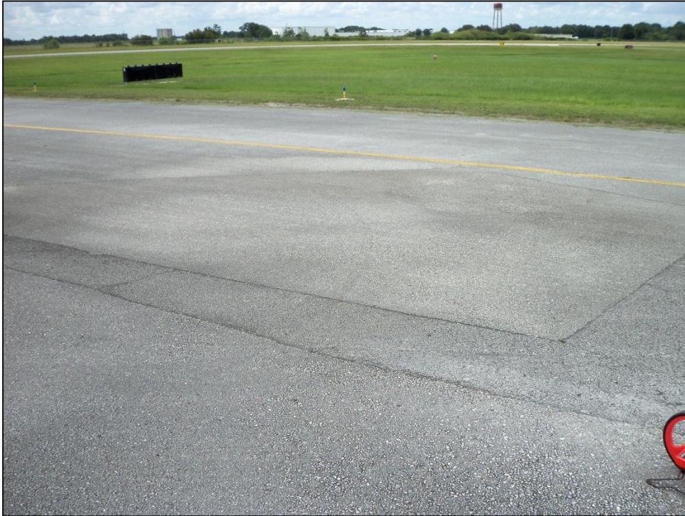
Taxiway A, Section 105, Sample Unit 118 – Low Severity (52) Raveling, Medium Severity (57) Weathering, Low Severity (50) Patching
