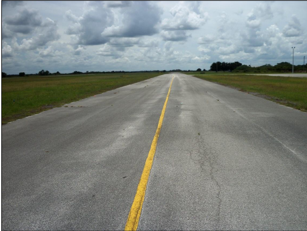
Taxiway A, Section 105, Sample Unit 104 – Low Severity (48) Longitudinal and Transverse Cracking, Medium Severity (52) Raveling, Low Severity (41) Alligator Cracking
