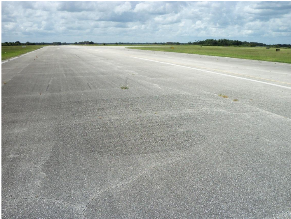
Runway 6-24, Section 6105, Sample Unit 149 – Low Severity (48) Longitudinal and Transverse Cracking, Medium Severity (57) Weathering, Low and Medium Severity (52) Raveling
