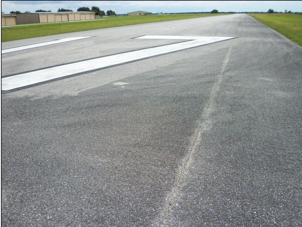
Runway 17-35, Section 6205, Sample Unit 179 – Low Severity (48) Longitudinal and Transverse Cracking, Low Severity (57) Weathering, Low Severity (52) Raveling
