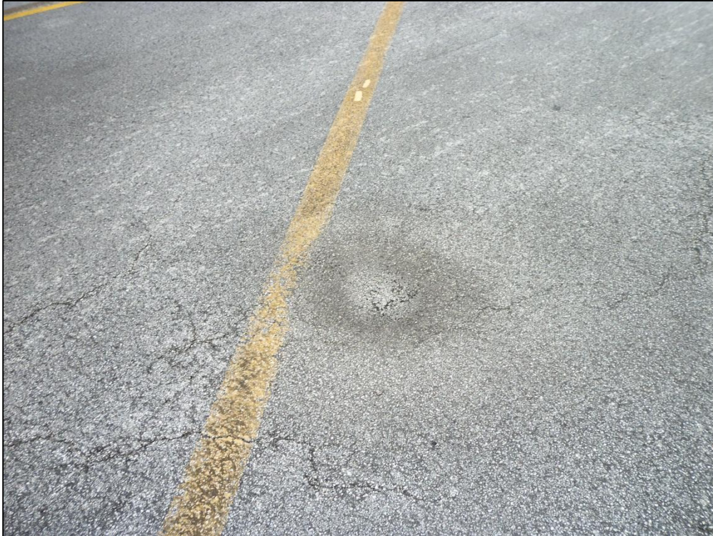
Taxiway A, Section 105, Sample Unit 118 – Low Severity (48) Longitudinal and Transverse Cracking, Low Severity (52) Raveling, Medium Severity (57) Weathering, High Severity (45) Depression
