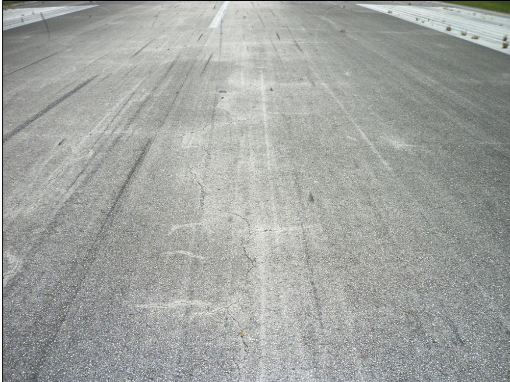
Runway 6-24, Section 6105, Sample Unit 121 – Low Severity (48) Longitudinal and Transverse Cracking, Medium Severity (57) Weathering, Low Severity (52) Raveling
