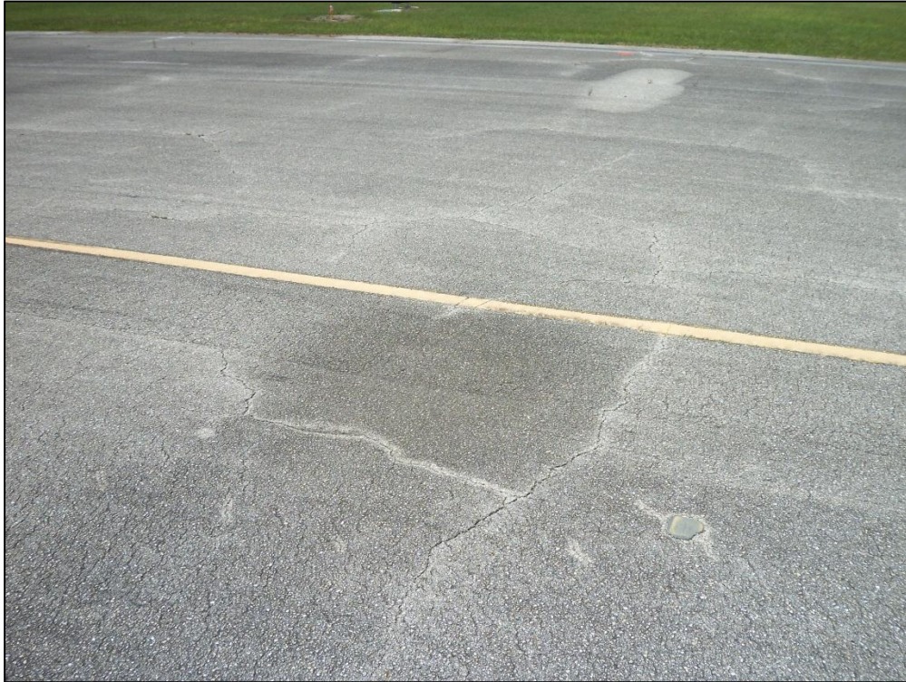
Runway 6-24, Section 6105, Sample Unit 154 – Low Severity (48) Longitudinal and Transverse Cracking, Medium Severity (57) Weathering, Low Severity (52) Raveling, Medium Severity (45) Depression
