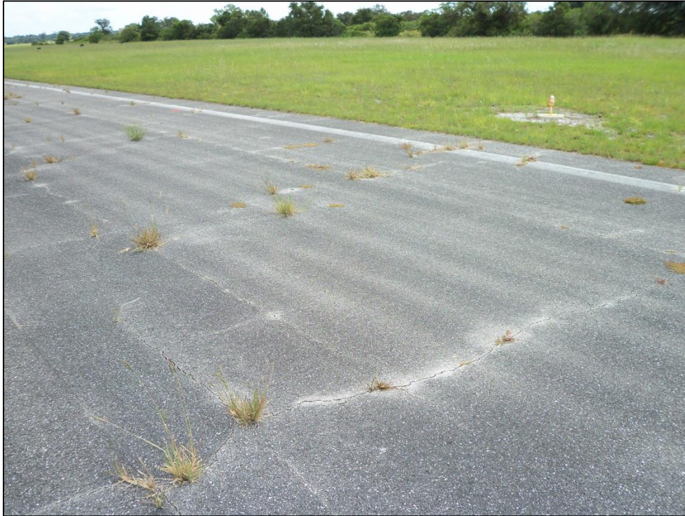
Runway 6-24, Section 6105, Sample Unit 107 – Medium Severity (57) Weathering, Low Severity (52) Raveling, Low Severity (43) Block Cracking
