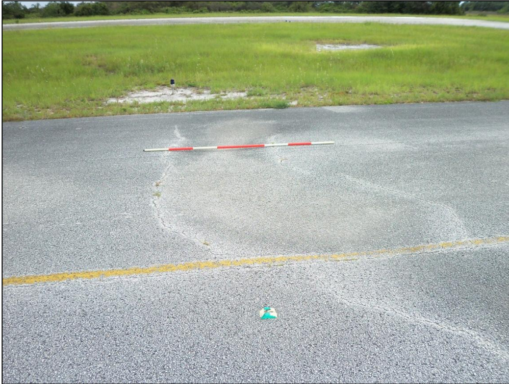
Taxiway D, Section 410, Sample Unit 102 – Low Severity (48) Longitudinal and Transverse Cracking, Low Severity (52) Raveling, Medium Severity (57) Weathering, High Severity (45) Depression
