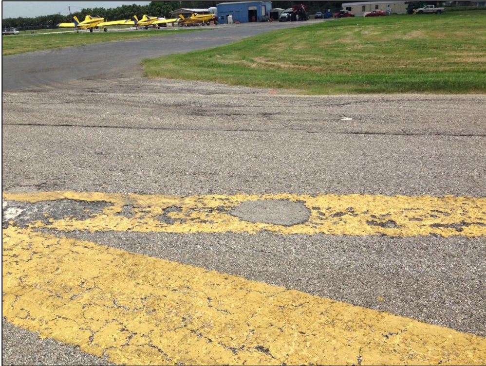
Runway 9-27, Section 6105, Sample Unit 101 – Medium and High Severity (48) Longitudinal and Transverse Cracking, Medium and High Severity (52) Raveling, High Severity (50) Patching
