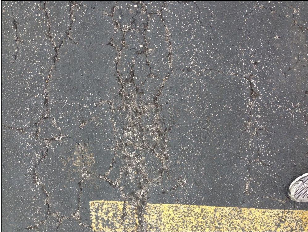
Taxiway, Section 105, Sample Unit 100 – High Severity (52) Raveling, High Severity (41) Alligator Cracking
