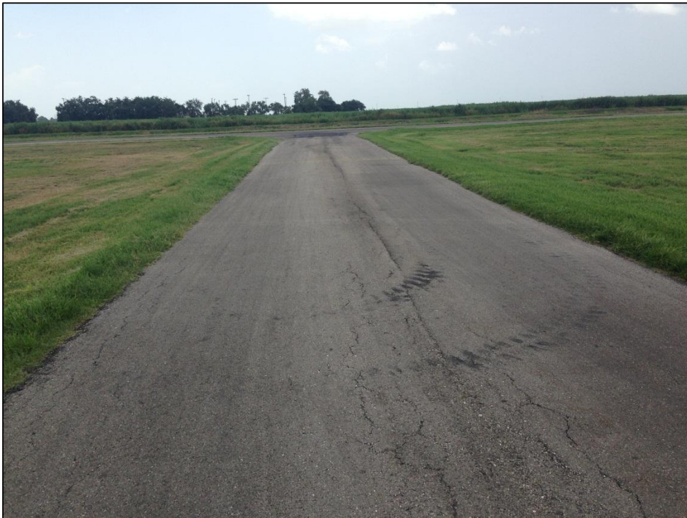
Taxiway, Section 115, Sample Unit 100 – Low Severity (48) Longitudinal and Transverse Cracking, Low and Medium Severity (52) Raveling, Low and Medium Severity (41) Alligator Cracking
