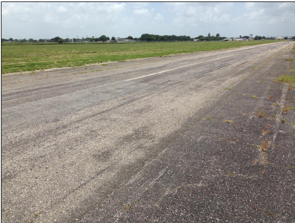
Runway 9-27, Section 6105, Sample Unit 129 – Medium Severity (48) Longitudinal and Transverse Cracking, Medium and High Severity (52) Raveling, Medium Severity (43) Block Cracking
