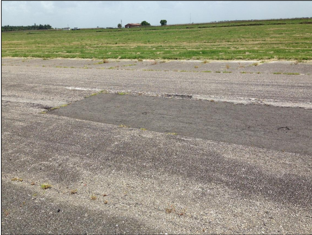
Runway 9-27, Section 6105, Sample Unit 129 – Medium Severity (48) Longitudinal and Transverse Cracking, Medium and High Severity (52) Raveling, High Severity (50) Patching
