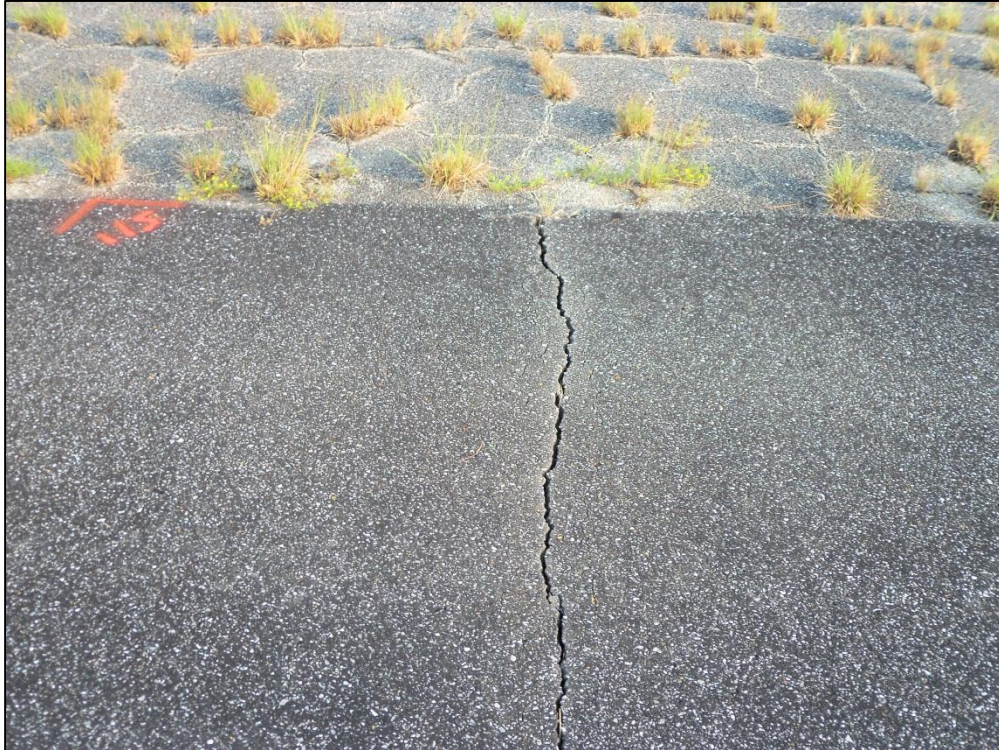
Runway 5-23, Section 6105, Sample Unit 115 – Medium Severity (48) Longitudinal and Transverse Cracking, Low Severity (52) Raveling, Low Severity (57) Weathering
