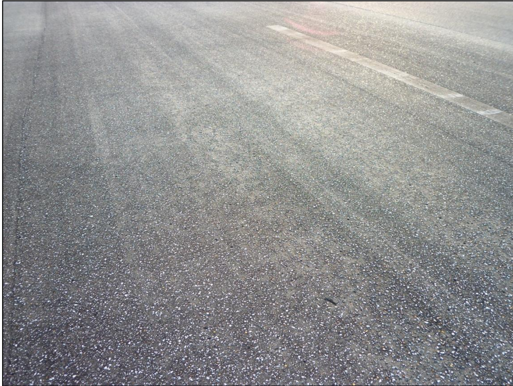
Runway 5-23, Section 6105, Sample Unit 115 - Medium Severity (57) Weathering
