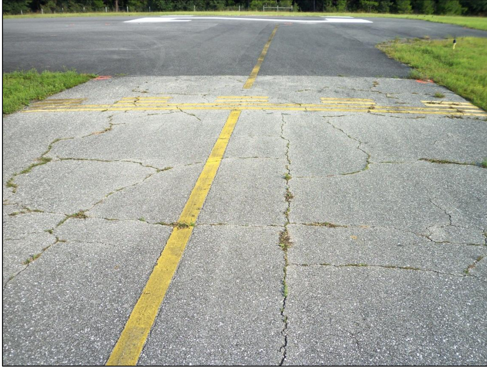
Taxiway A, Section 105, Sample Unit 101 – Low Severity (43) Block Cracking, Low Severity (52) Raveling, Low Severity (57) Weathering
