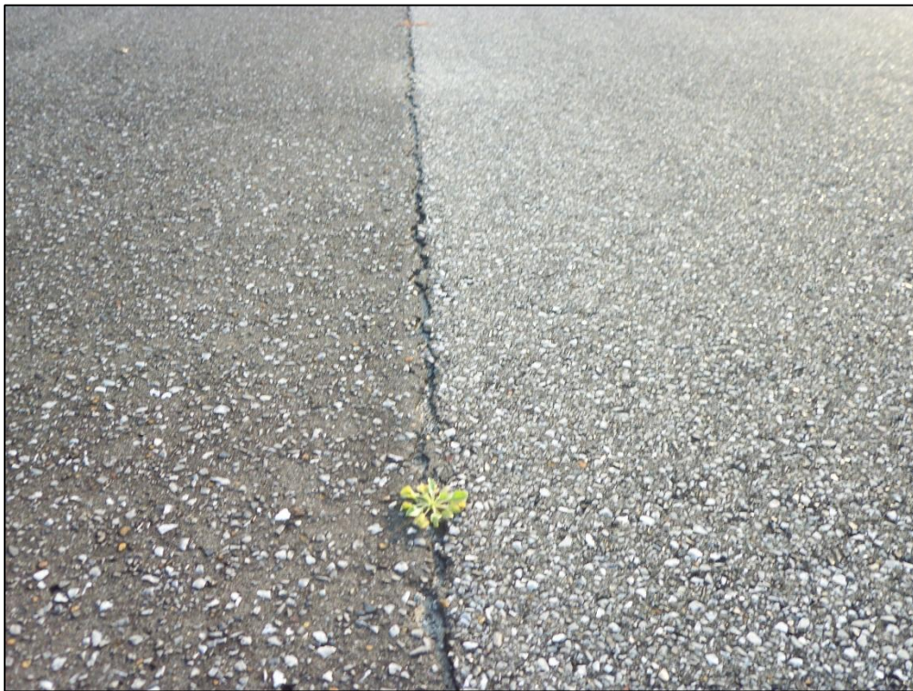
Runway 5-23, Section 6105, Sample Unit 145 - Medium Severity (48) Longitudinal and Transverse Cracking
