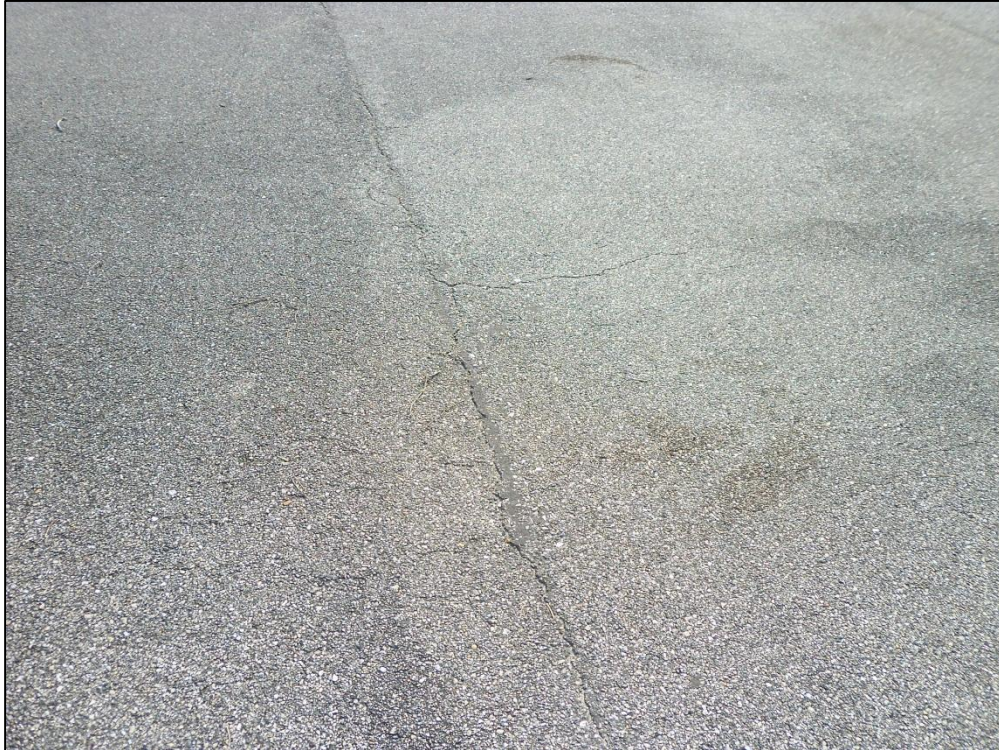
Apron, Section 4120, Sample Unit 501 – Low Severity (48) Longitudinal and Transverse Cracking, Low Severity (52) Raveling, Low Severity (57) Weathering
