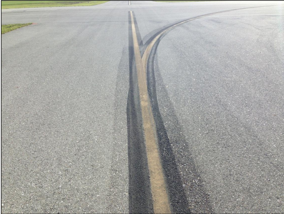
Taxiway to Hangar, Section 510, Sample Unit 100 – Low Severity (52) Raveling
