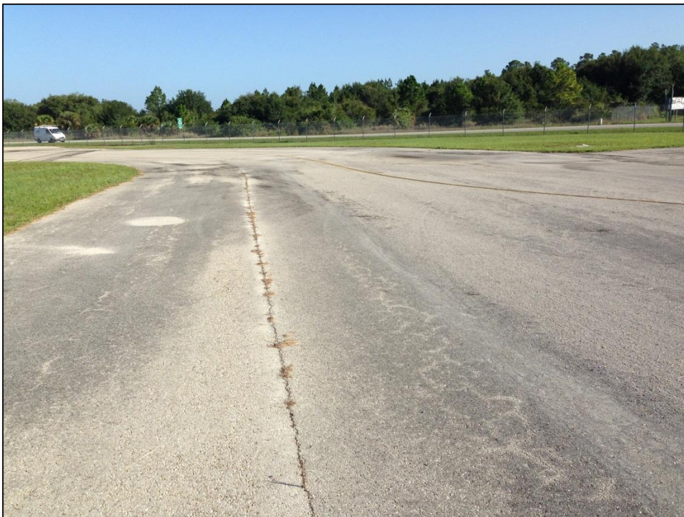
Northwest Apron, Section 4160, Sample Unit 104 – Low Severity (48) Longitudinal and Transverse Cracking, Medium Severity (52) Raveling, Low Severity (43) Block Cracking
