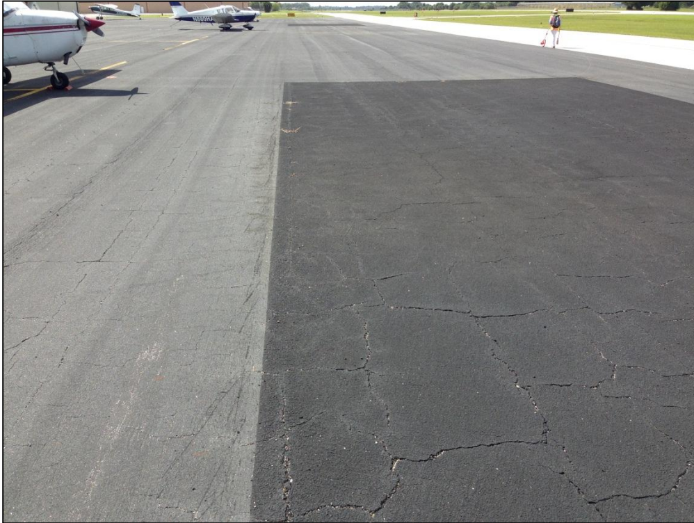
Apron North, Section 4110, Sample Unit 200 – Low Severity (43) Block Cracking, Medium Severity (52) Raveling, Low Severity (57) Weathering
