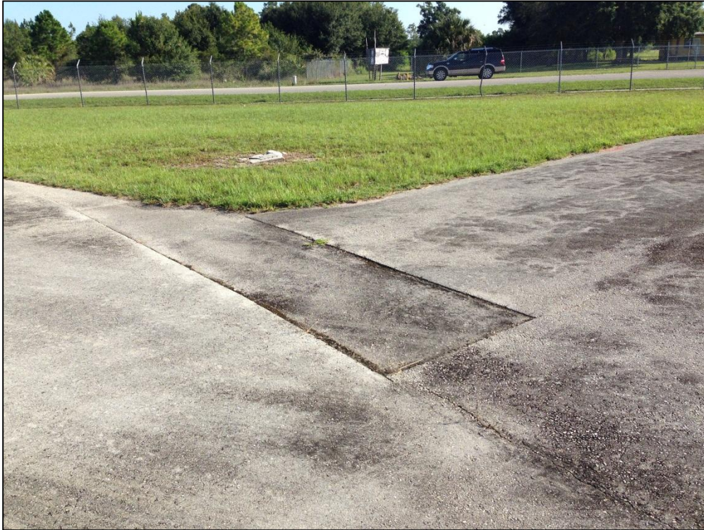
Northwest Apron, Section 4160, Sample Unit 104 – Low Severity (48) Longitudinal and Transverse Cracking, Medium Severity (52) Raveling, Medium Severity (50) Patching, Low Severity (43) Block Cracking
