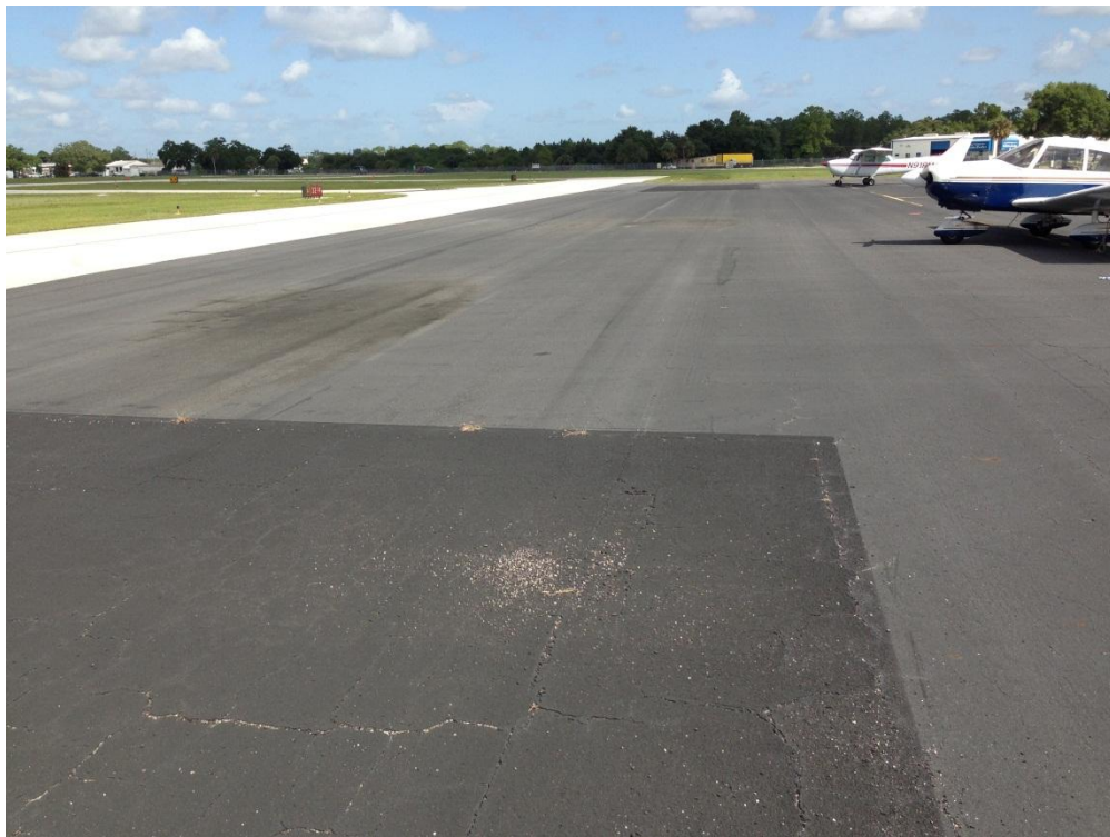
Apron North, Section 4110, Sample Unit 202 – Low Severity (43) Block Cracking, Low Severity (52) Raveling, Low Severity (57) Weathering, Low Severity (45) Depression
