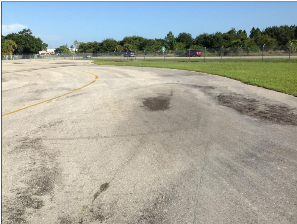
Northwest Apron, Section 4160, Sample Unit 104 – Low Severity (48) Longitudinal and Transverse Cracking, Medium Severity (52) Raveling, Medium Severity (45) Depression
