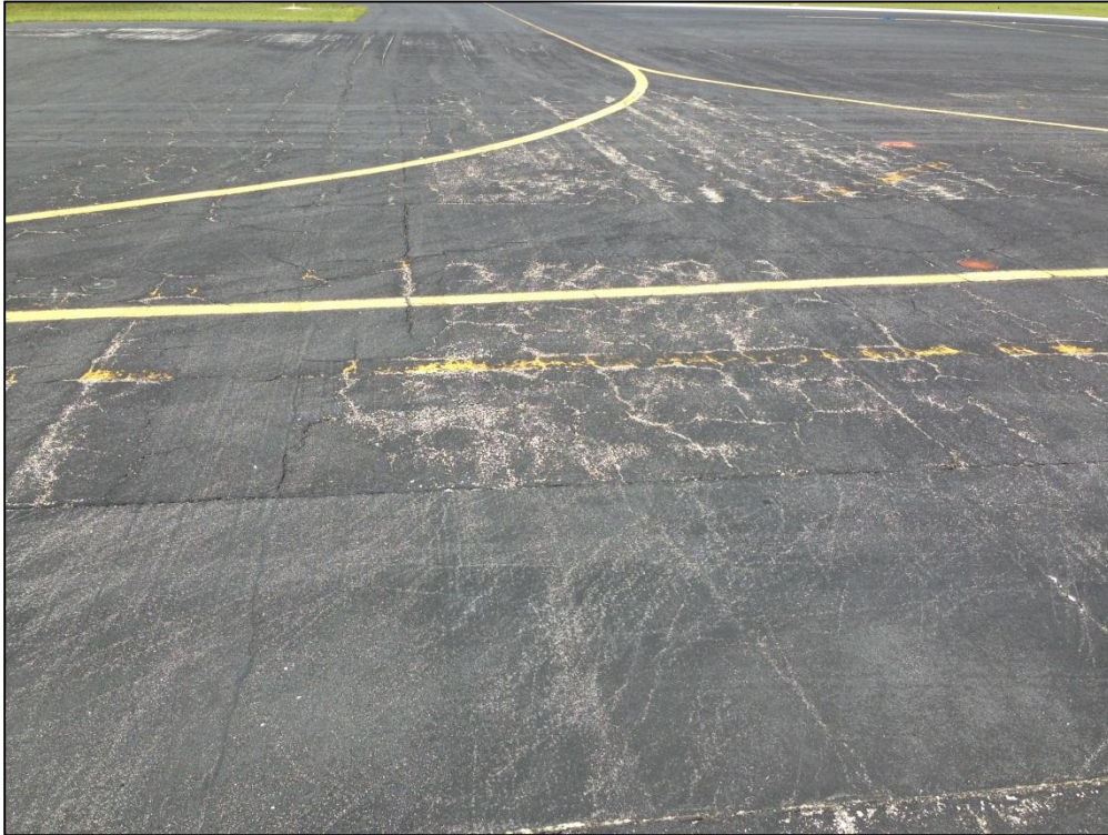
Apron North, Section 4110, Sample Unit 505 – Low and Medium Severity (43) Block Cracking, Low Severity (52) Raveling
