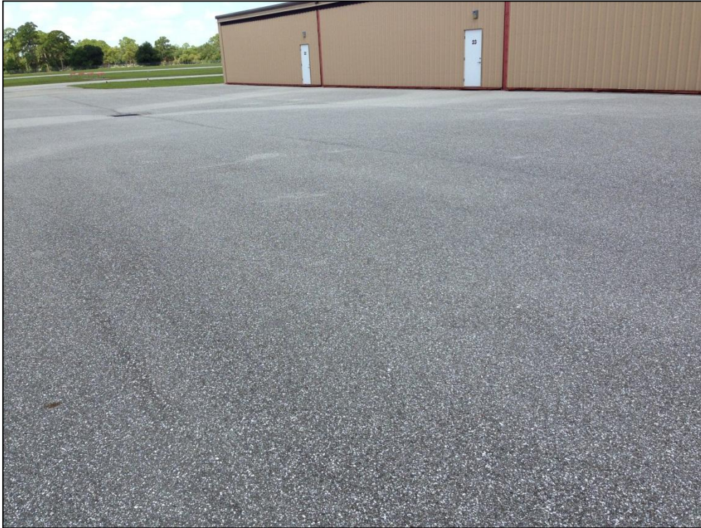
Apron T-Hangar, Section 4305, Sample Unit 202 – Low Severity (48) Longitudinal and Transverse Cracking, Medium Severity (57) Weathering
