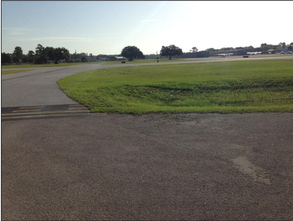
Taxiway to Hangar, Section 505, Sample Unit 102 – Low Severity (48) Longitudinal and Transverse Cracking, Medium and High Severity (52) Raveling
