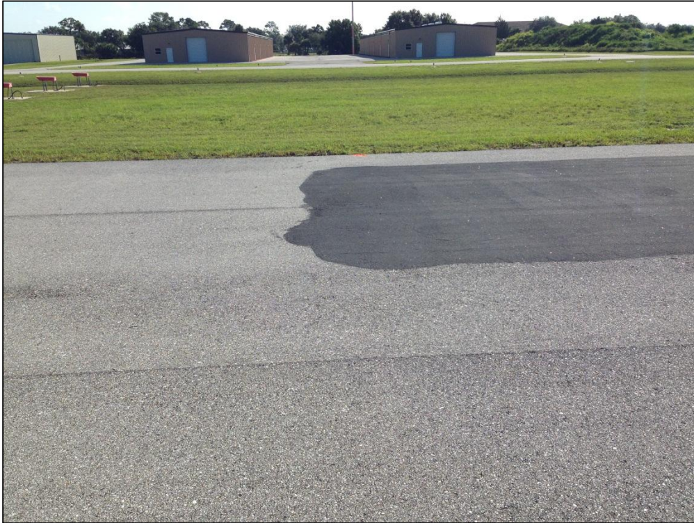
Runway 14-32, Section 6105, Sample Unit 115 – Low Severity (48) Longitudinal and Transverse Cracking, Low Severity (52) Raveling, Low Severity (57) Weathering
