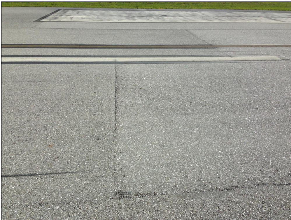
Runway 14-32, Section 6105, Sample Unit 143 – Low Severity (48) Longitudinal and Transverse Cracking, Low Severity (57) Weathering
