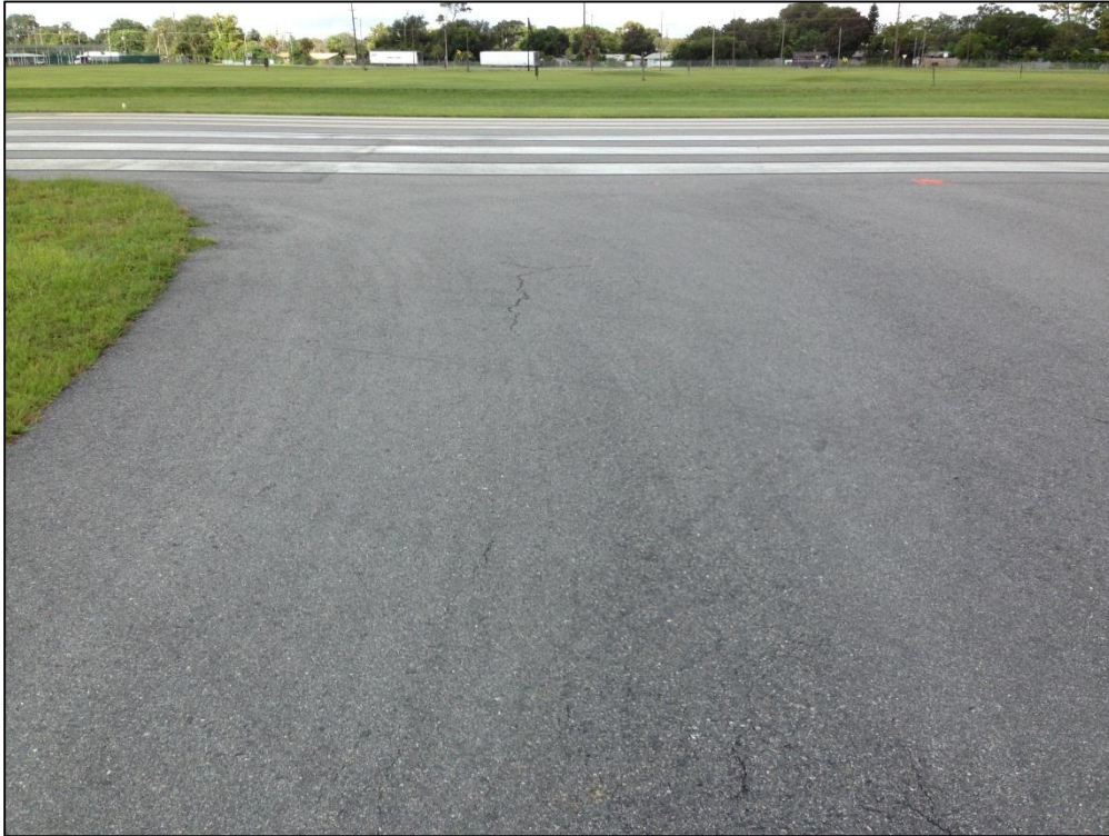
Taxiway A, Section 105, Sample Unit 100 – Low Severity (57) Weathering, Low Severity (48) Longitudinal and Transverse Cracking
