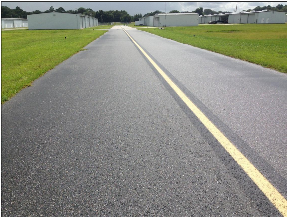
Taxiway C, Section 310, Sample Unit 101 – Low Severity (57) Weathering
