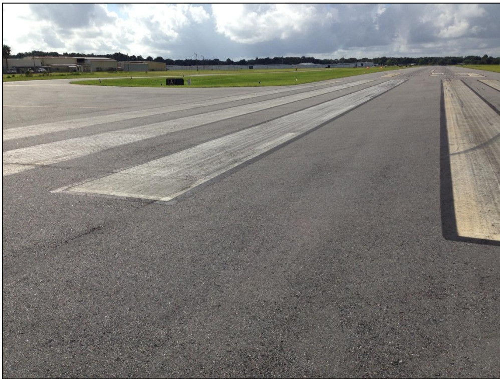
Runway 15-23, Section 6105, Sample Unit 100 – Low Severity (57) Weathering
