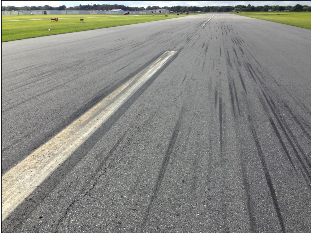
Runway 15-23, Section 6105, Sample Unit 105 – Low Severity (57) Weathering, Low Severity (48) Longitudinal and Transverse Cracking
