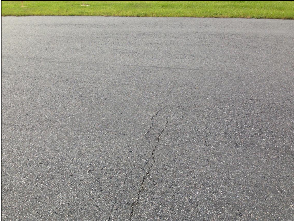
Runway 15-23, Section 6105, Sample Unit 129 – Low Severity (57) Weathering, Low Severity (48) Longitudinal and Transverse Cracking, Low Severity (56) Swelling
