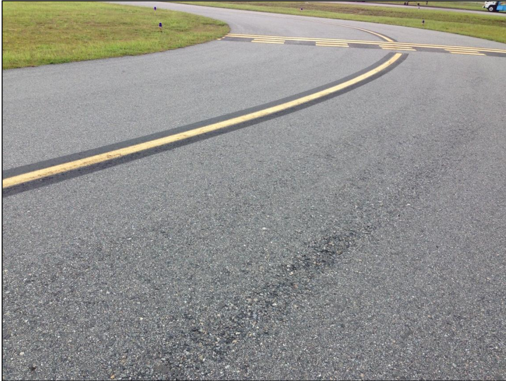
Taxiway A, Section 110, Sample Unit 100 – Low Severity (57) Weathering, Low Severity (52) Raveling
