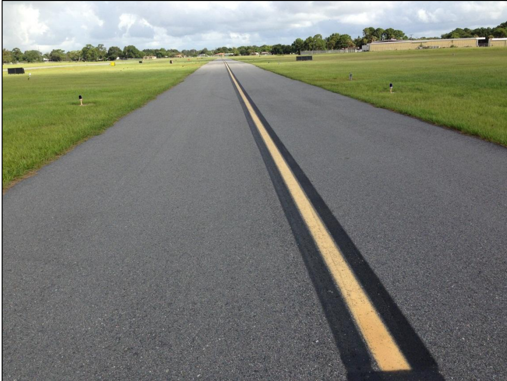
Taxiway A, Section 105, Sample Unit 110 – Low Severity (57) Weathering
