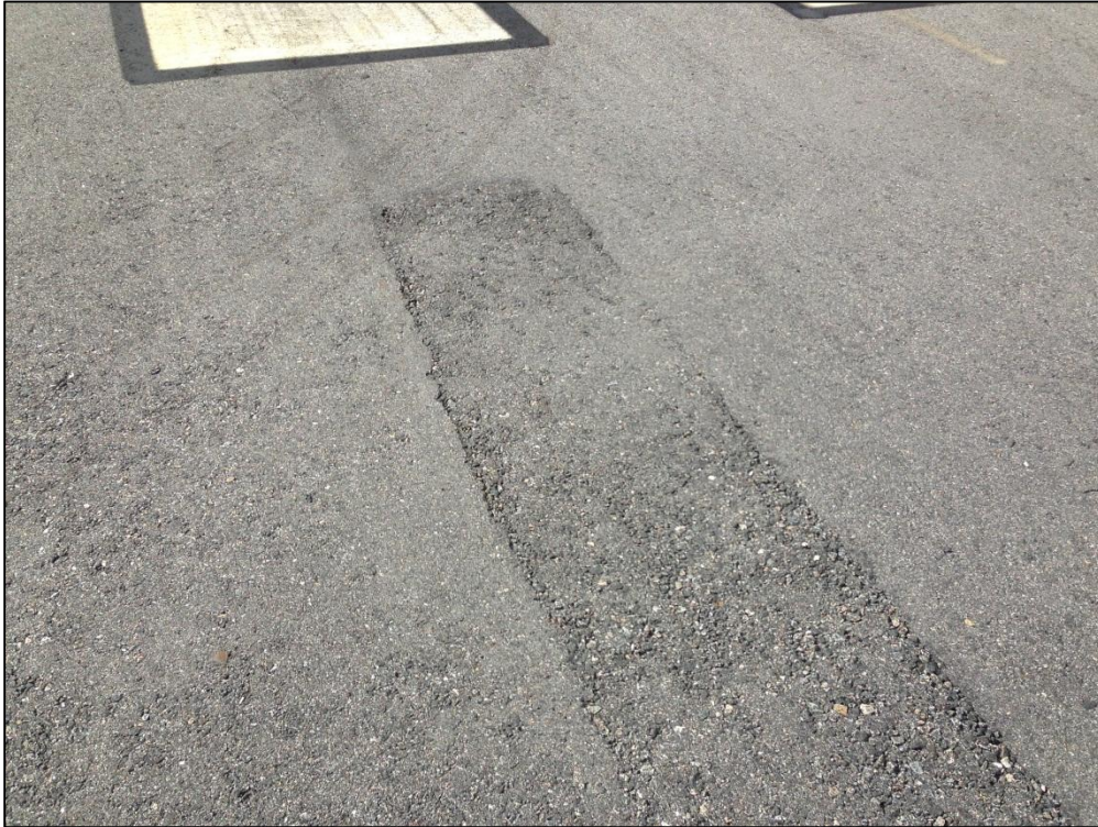
Runway 15-23, Section 6105, Sample Unit 100 – Low Severity (57) Weathering, Low Severity (52) Raveling
