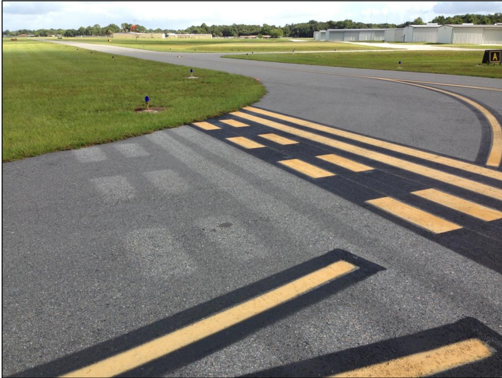
Taxiway B, Section 205, Sample Unit 100 – Low Severity (57) Weathering
