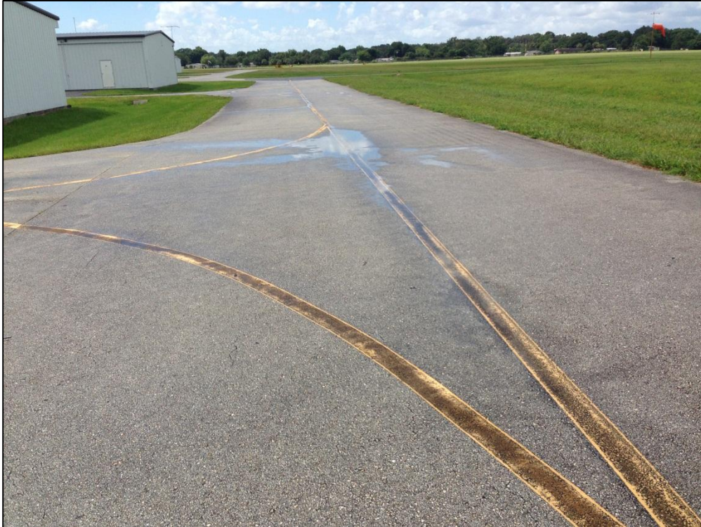
Apron T-Hangar, Section 4205, Sample Unit 102 – Low Severity (45) Depression, Low Severity (57) Weathering, Low Severity (52) Raveling
