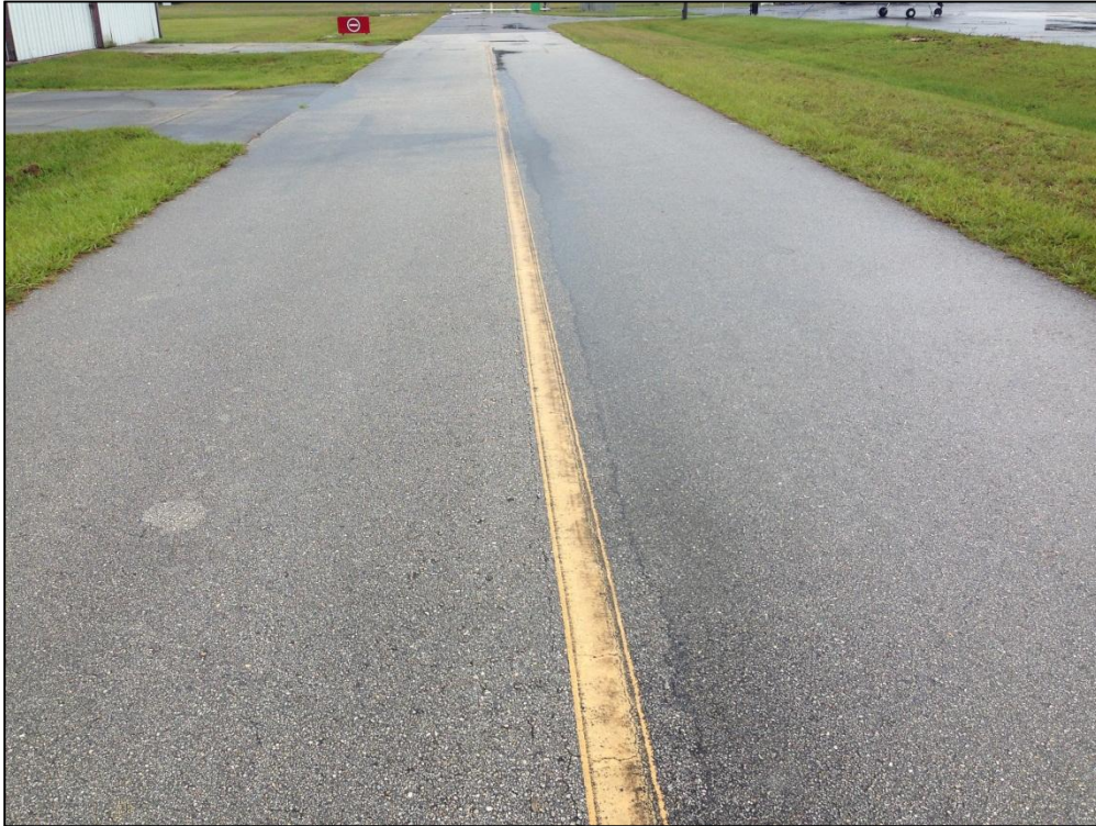
Apron T-Hangar, Section 4210, Sample Unit 501 – Low Severity (57) Weathering, Low Severity (48) Longitudinal and Transverse Cracking
