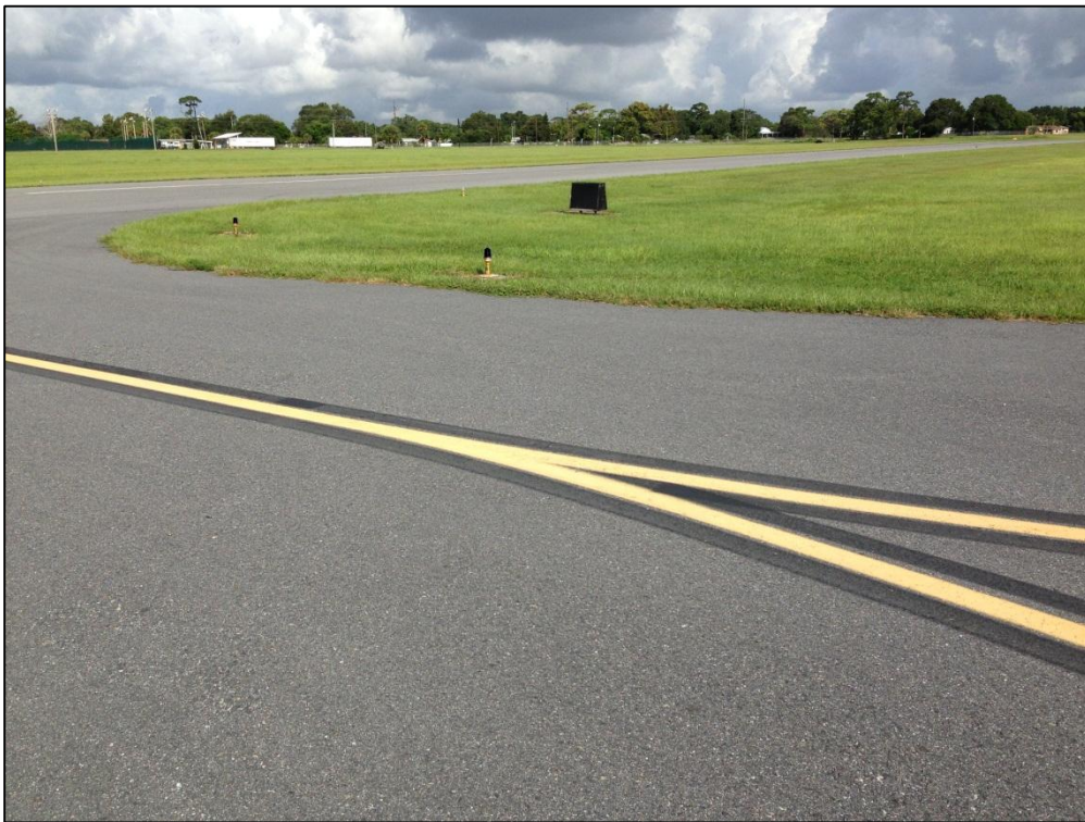
Taxiway D, Section 405, Sample Unit 100 – Low Severity (57) Weathering
