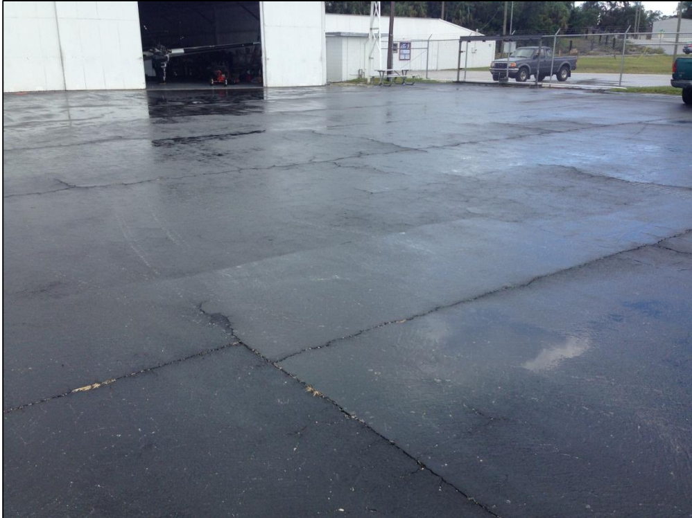
Apron, Section 4107, Sample Unit 203 – Low Severity (57) Weathering, Low Severity (48) Longitudinal and Transverse Cracking
