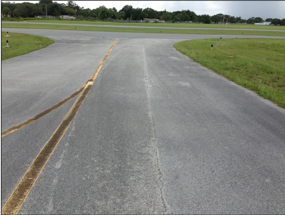
Taxiway AP, Section 115, Sample Unit 115 – Low Severity (57) Weathering, Low Severity (48) Longitudinal and Transverse Cracking
