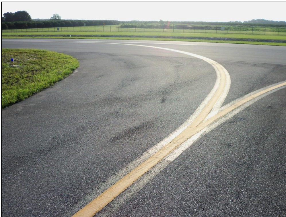
Apron Term, Section 4105, Sample Unit 100 – Low Severity (57) Weathering, Low Severity (52) Raveling
