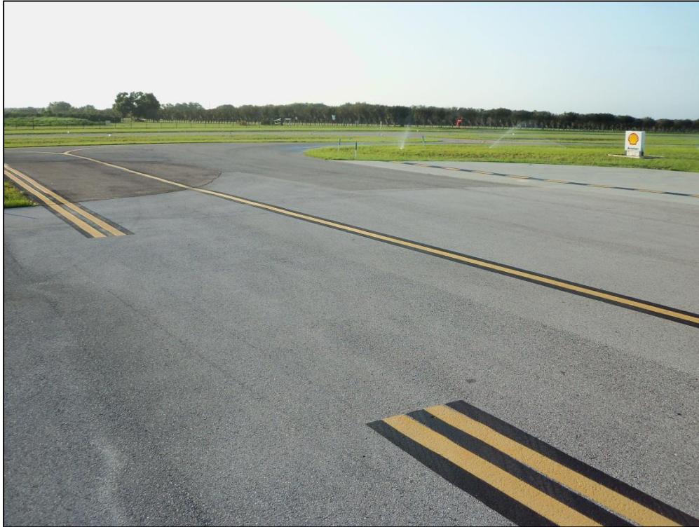
Apron Term, Section 4110, Sample Unit 301 – Low Severity (57) Weathering, Low Severity (52) Raveling
