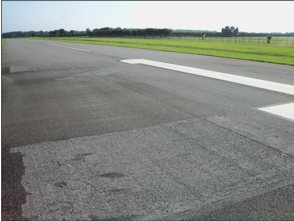
Runway 01-19, Section 6105, Sample Unit 202 – Low Severity (57) Weathering, Low and Medium Severity (52) Raveling
