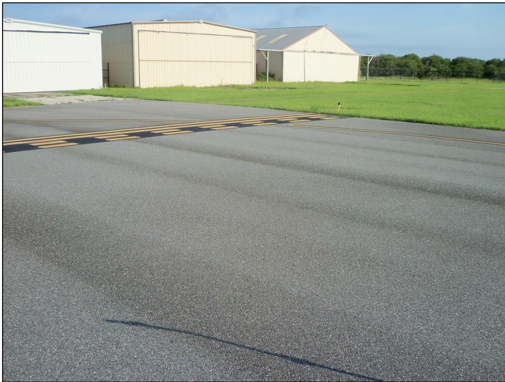
Apron T-Hangar, Section 4205, Sample Unit 102 – Low Severity (57) Weathering, Low Severity (52) Raveling
