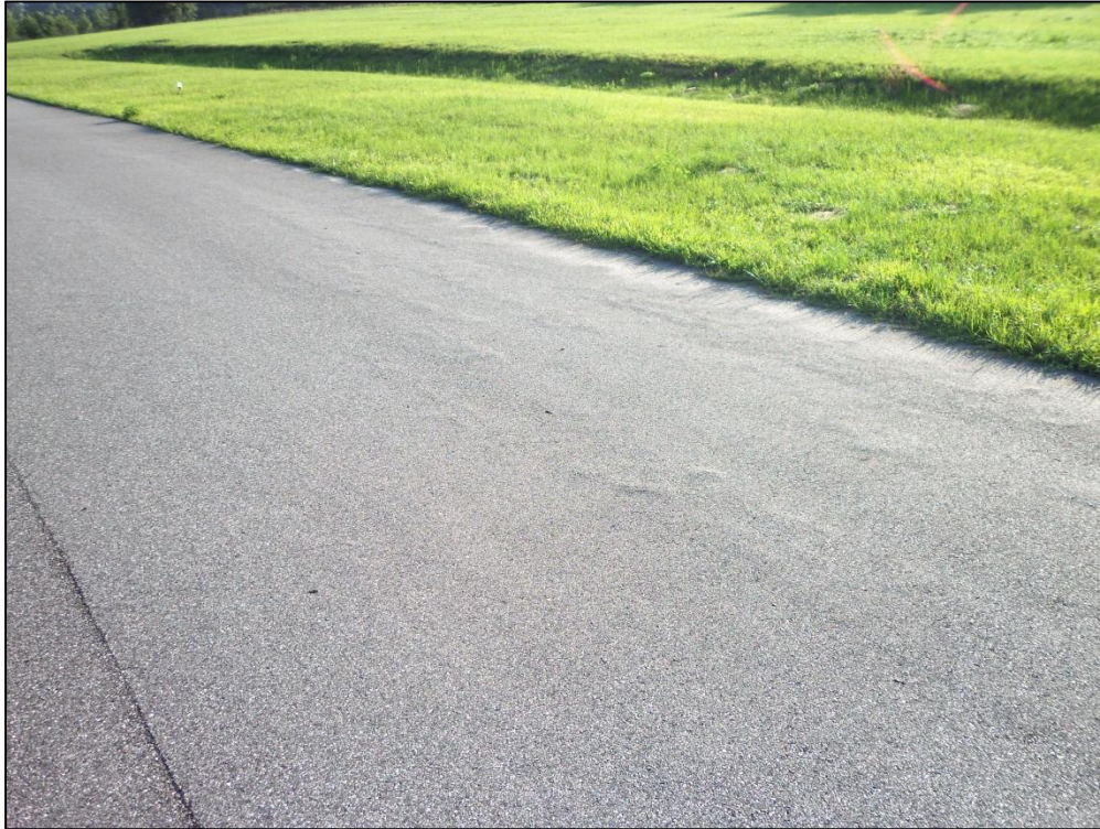
Runway 01-19, Section 6105, Sample Unit 222 – Low Severity (57) Weathering, Low Severity (48) Longitudinal and Transverse Cracking, Low Severity (56) Swelling
