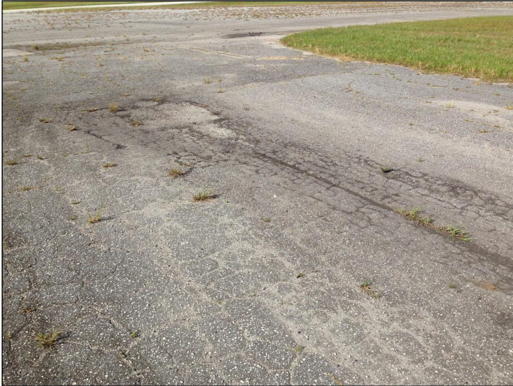
Taxiway C, Section 305, Sample Unit 300 – Low Severity (41) Alligator Cracking, Low Severity (52) Raveling, Low Severity (53) Rutting, Low Severity (57) Weathering
