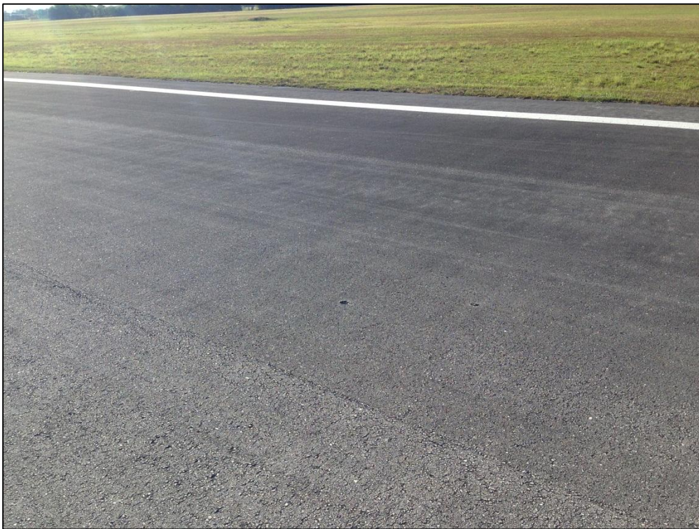
Runway 10-28, Section 6305, Sample Unit 514 – Low Severity (57) Weathering
