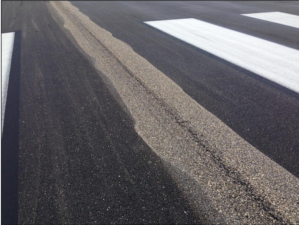
Runway 5-23, Section 6205, Sample Unit 377 – Low Severity (48) Longitudinal and Transverse Cracking, Low Severity (52) Raveling, Low Severity (57) Weathering
