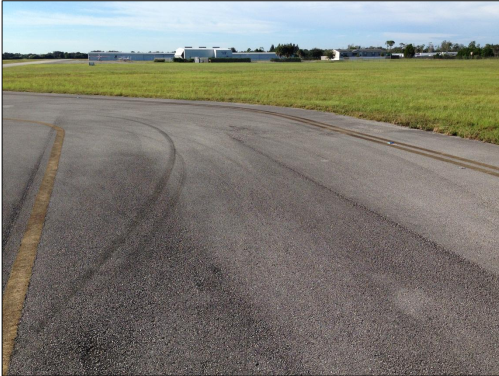
Runway 10-28, Section 6305, Sample Unit 502 – Low Severity (52) Raveling, Low Severity (57) Weathering
