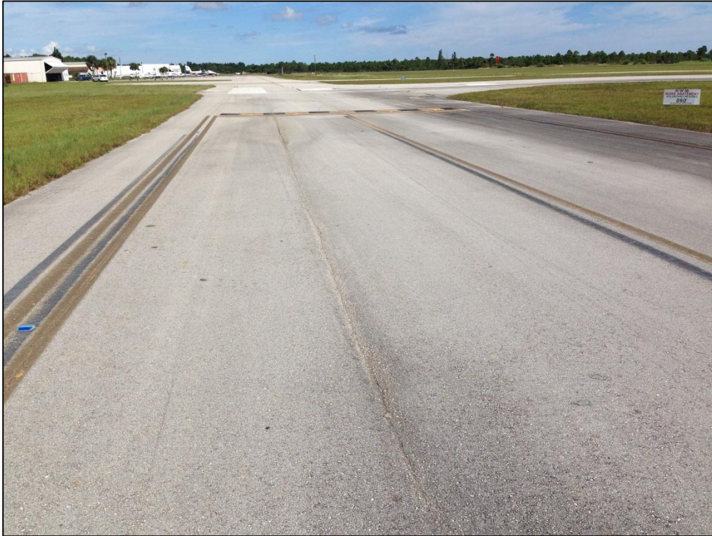
Taxiway A, Section 425, Sample Unit 99 – Low Severity (45) Depression, Low Severity (48) Longitudinal and Transverse Cracking, Low Severity (52) Raveling, Low Severity (57) Weathering
