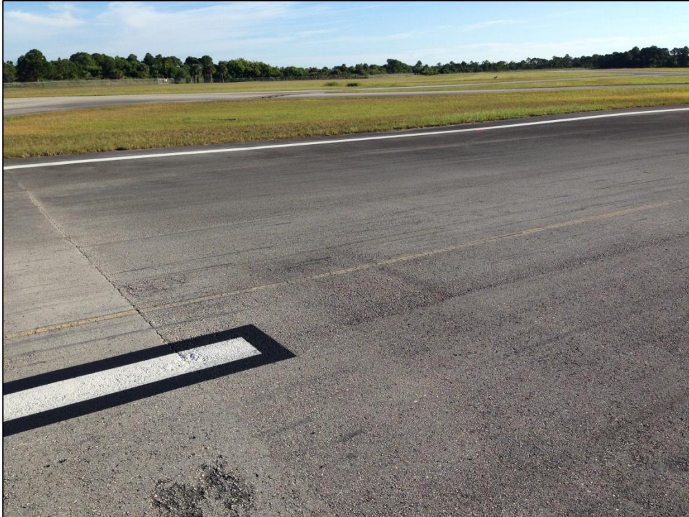
Runway 10-28, Section 6305, Sample Unit 534 – Low Severity (48) Longitudinal and Transverse Cracking, Low Severity (52) Raveling, Low Severity (57) Weathering
