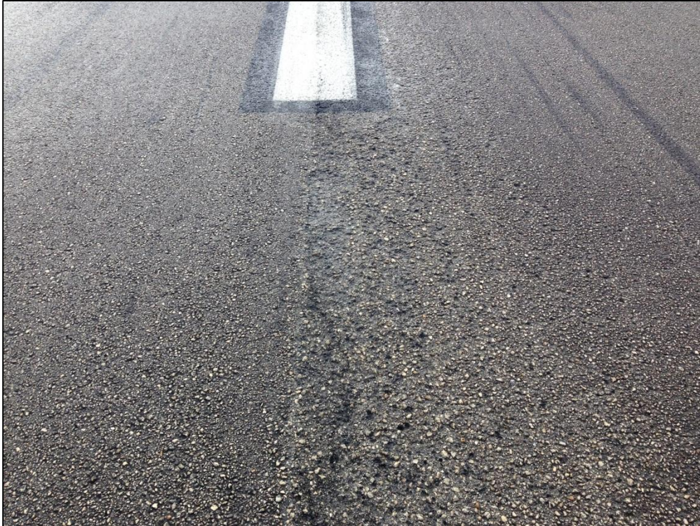
Runway 5-23, Section 6205, Sample Unit 314 – Low Severity (52) Raveling, Low Severity (57) Weathering
