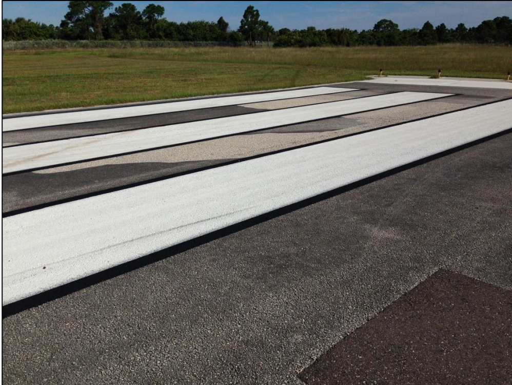
Runway 5-23, Section 6205, Sample Unit 379 – Low Severity (50) Patching, Low Severity (52) Raveling, Low Severity (57) Weathering
