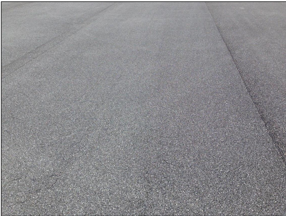
Apron W, Section 5105, Sample Unit 431 – Low Severity (48) Longitudinal and Transverse Cracking, Low Severity (57) Weathering
