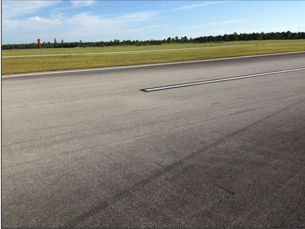
Runway 10-28, Section 6305, Sample Unit 502 – Low Severity (48) Longitudinal and Transverse Cracking, Low Severity (57) Weathering
