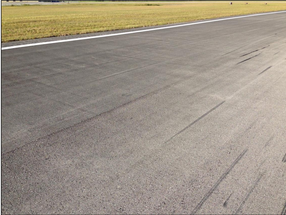
Runway 10-28, Section 6315, Sample Unit 554 – Low Severity (57) Weathering
