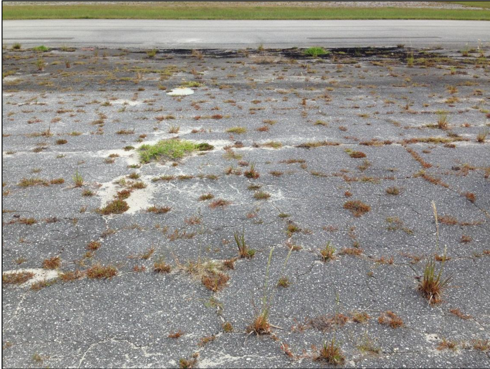
Apron W, Section 5115, Sample Unit 435 – Medium Severity (43) Block Cracking, Medium Severity (52) Raveling
