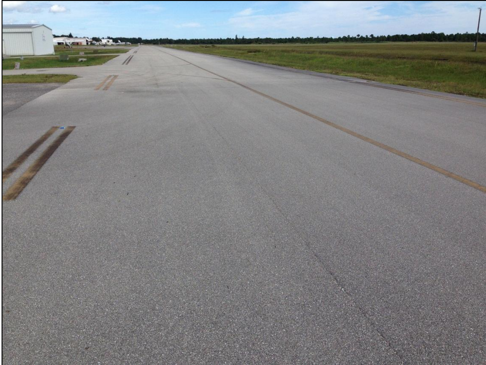
Taxiway A, Section 405, Sample Unit 108 – Low Severity (48) Longitudinal and Transverse Cracking, Low Severity (57) Weathering
