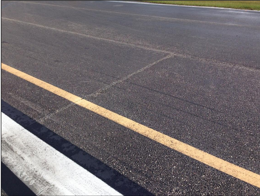
Runway 5-23, Section 6205, Sample Unit 307 – Low Severity (48) Longitudinal and Transverse Cracking, Low Severity (57) Weathering
