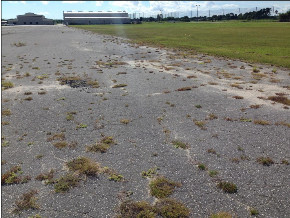
Apron SE, Section 5605, Sample Unit 101 – Low Severity (43) Block Cracking, Low, Medium, and High Severity (52) Raveling
