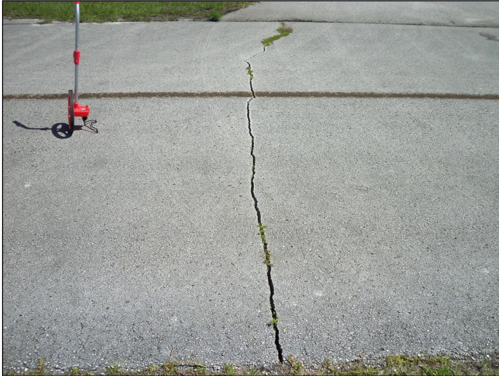
Apron Hangar, Section 4220, Sample Unit 300 – High Severity (48) Longitudinal and Transverse Cracking, Low and Medium Severity (52) Raveling, Low Severity (57) Weathering
