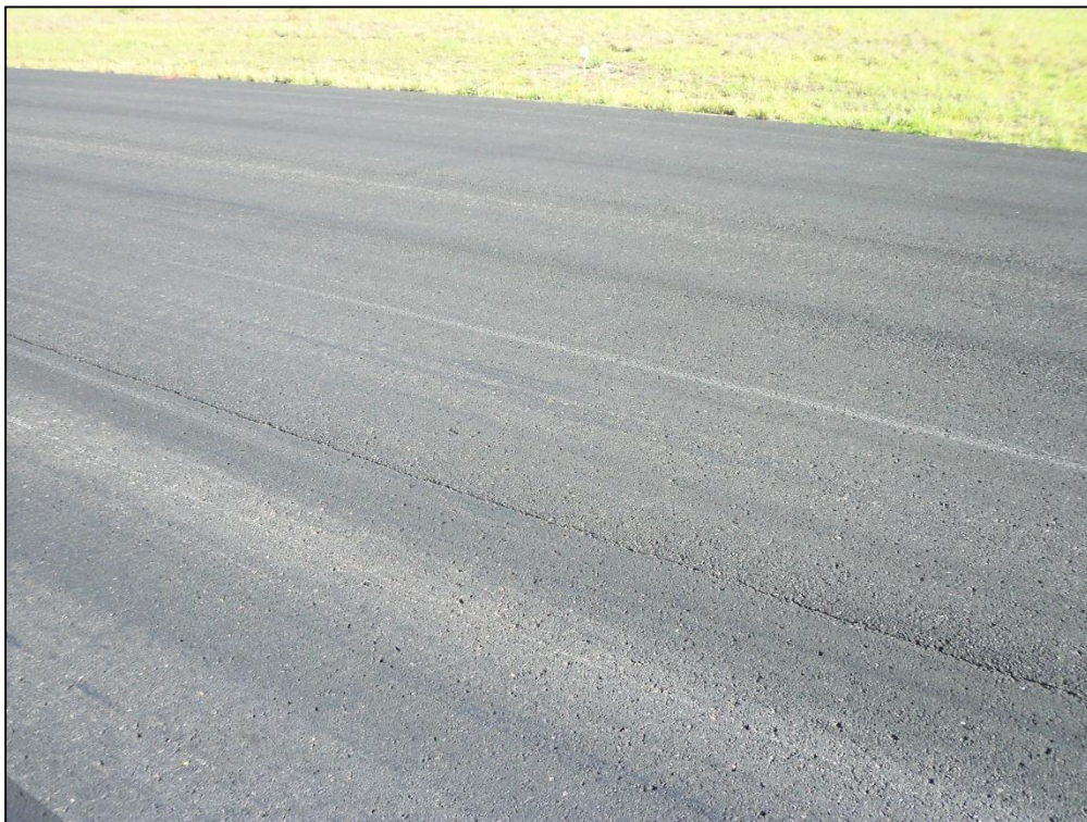
Runway 10-28, Section 6105, Sample Unit 157 – Low Severity (48) Longitudinal and Transverse Cracking, Low Severity (52) Raveling
