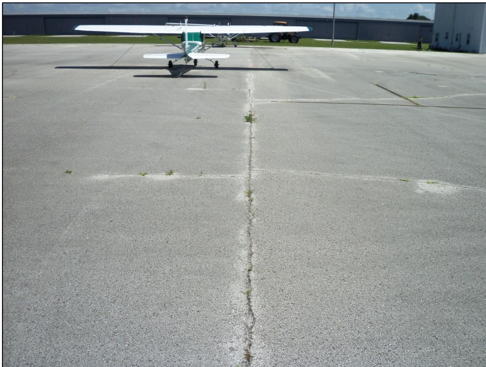
Apron, Section 4105, Sample Unit 204 – Low and Medium Severity (48) Longitudinal and Transverse Cracking, Low and Medium Severity (52) Raveling, Low Severity (57) Weathering
