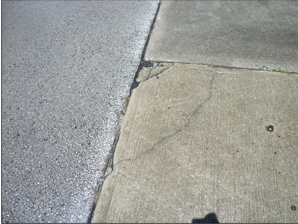
Apron Hangar, Section 4230, Sample Unit 401 – Medium Severity (65) Joint Seal Damage, Medium Severity (62) Corner Break
