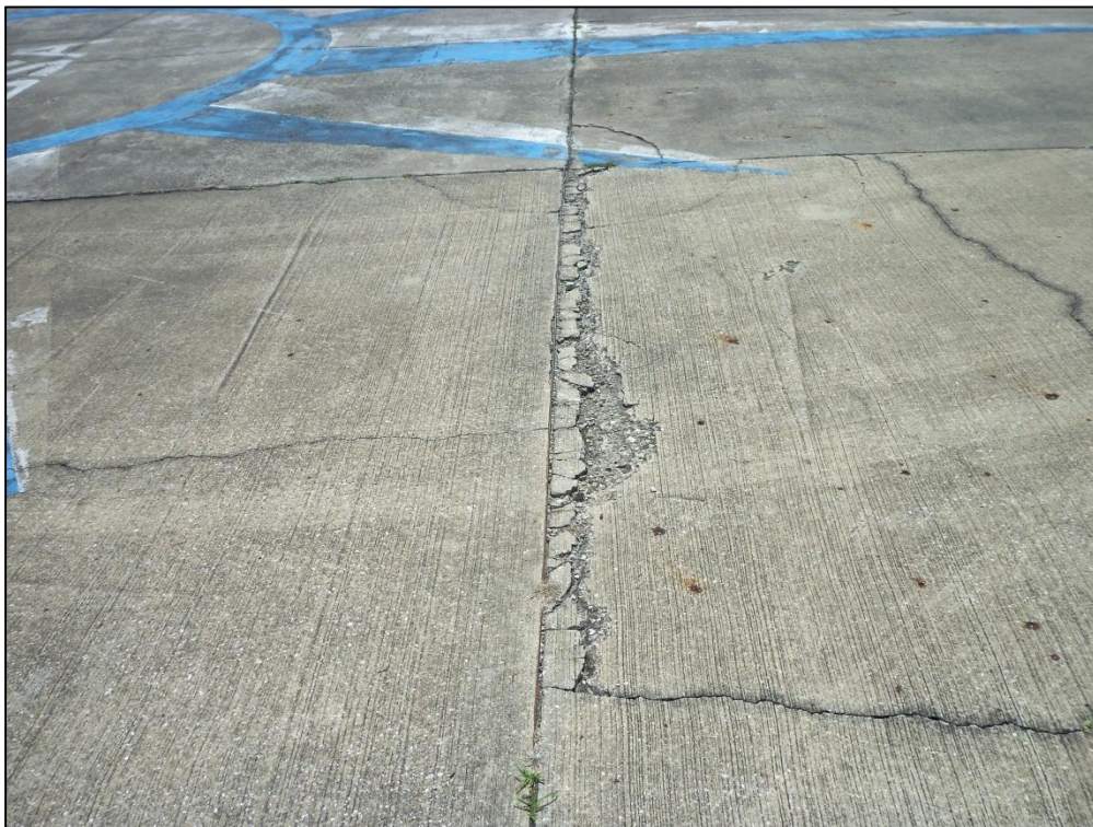
Apron Hangar, Section 4230, Sample Unit 401 – Medium Severity (65) Joint Seal Damage, High Severity (74) Joint Spalling, Low Severity (63) Longitudinal, Transverse, Diagonal Cracking, Low Severity (62) Corner Break
