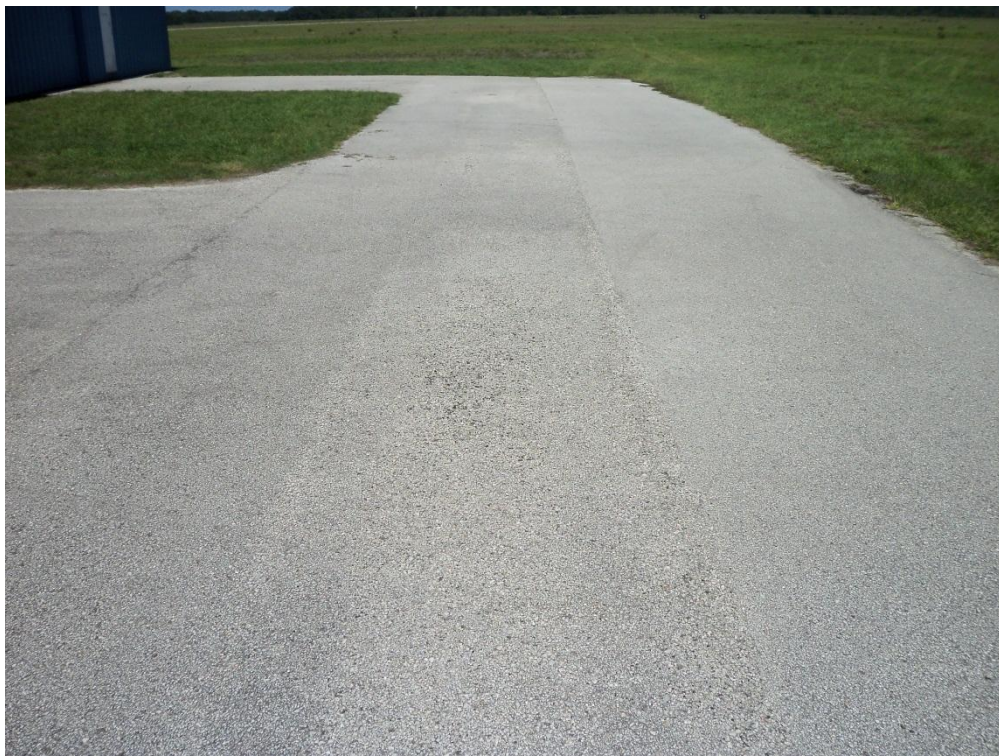
Apron Hangar, Section 4210, Sample Unit 100 – Low Severity (48) Longitudinal and Transverse Cracking, Low and Medium Severity (52) Raveling, Low Severity (57) Weathering
