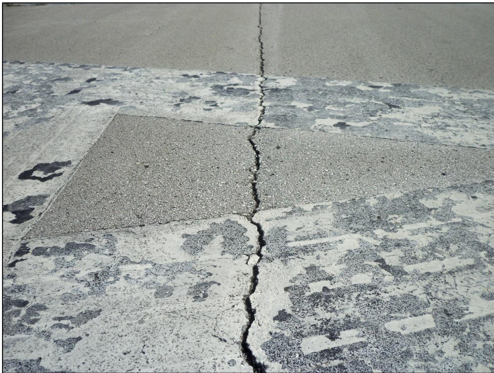
Taxiway East, Section 110, Sample Unit 113 – Medium Severity (48) Longitudinal and Transverse Cracking, Low Severity (52) Raveling, Low Severity (57) Weathering
