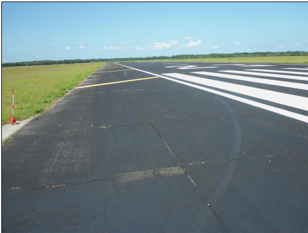
Taxiway East, Section 115, Sample Unit 135 – Low Severity (63) Longitudinal, Transverse, Diagonal Cracking, Low Severity (65) Joint Seal Damage
