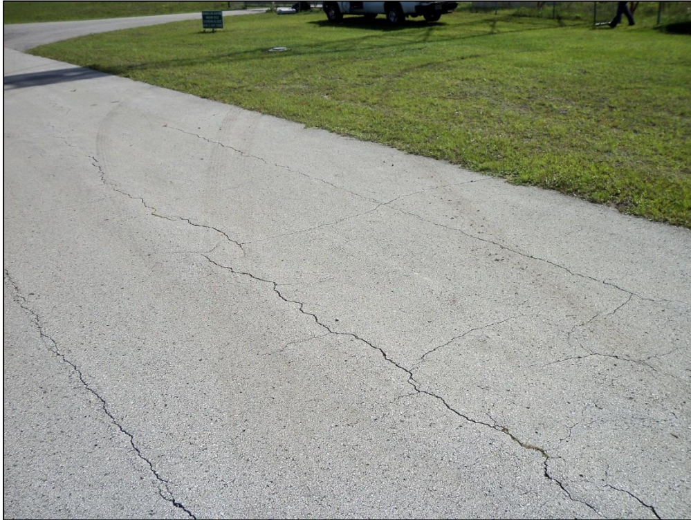
Taxiway East, Section 110, Sample Unit 113 – Low Severity (48) Longitudinal and Transverse Cracking, Low Severity (52) Raveling, Low Severity (57) Weathering, Low Severity (43) Block Cracking
