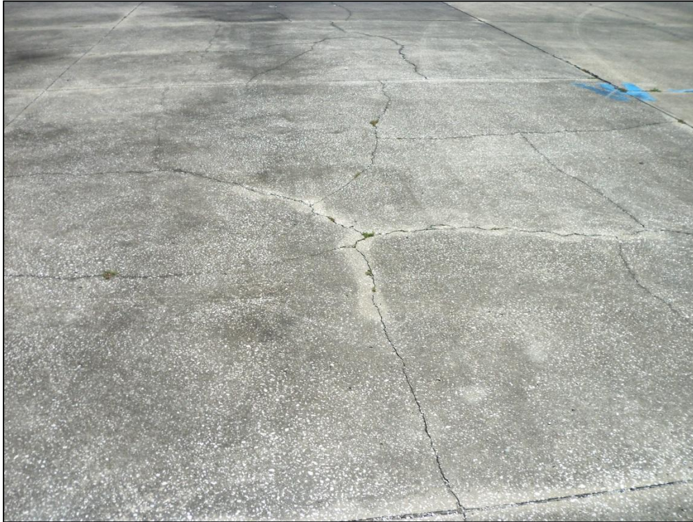
Apron Hangar, Section 4230, Sample Unit 401 – Medium Severity (65) Joint Seal Damage, Low Severity (72) Shattered Slab
