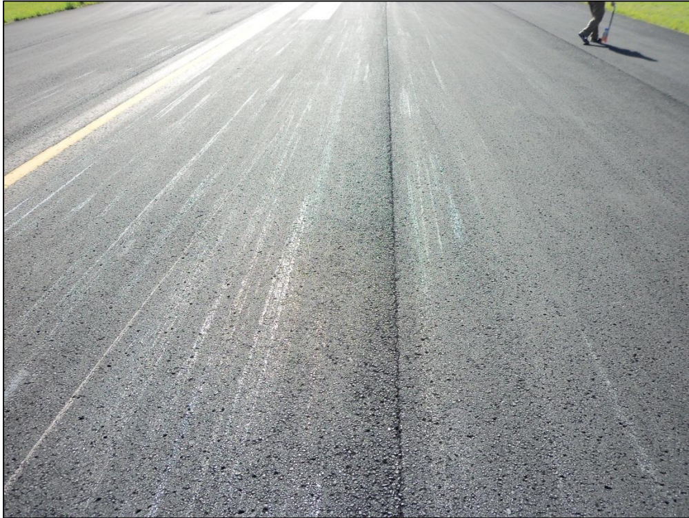
Runway 10-28, Section 6105, Sample Unit 105 – Low Severity (48) Longitudinal and Transverse Cracking, Low Severity (52) Raveling
