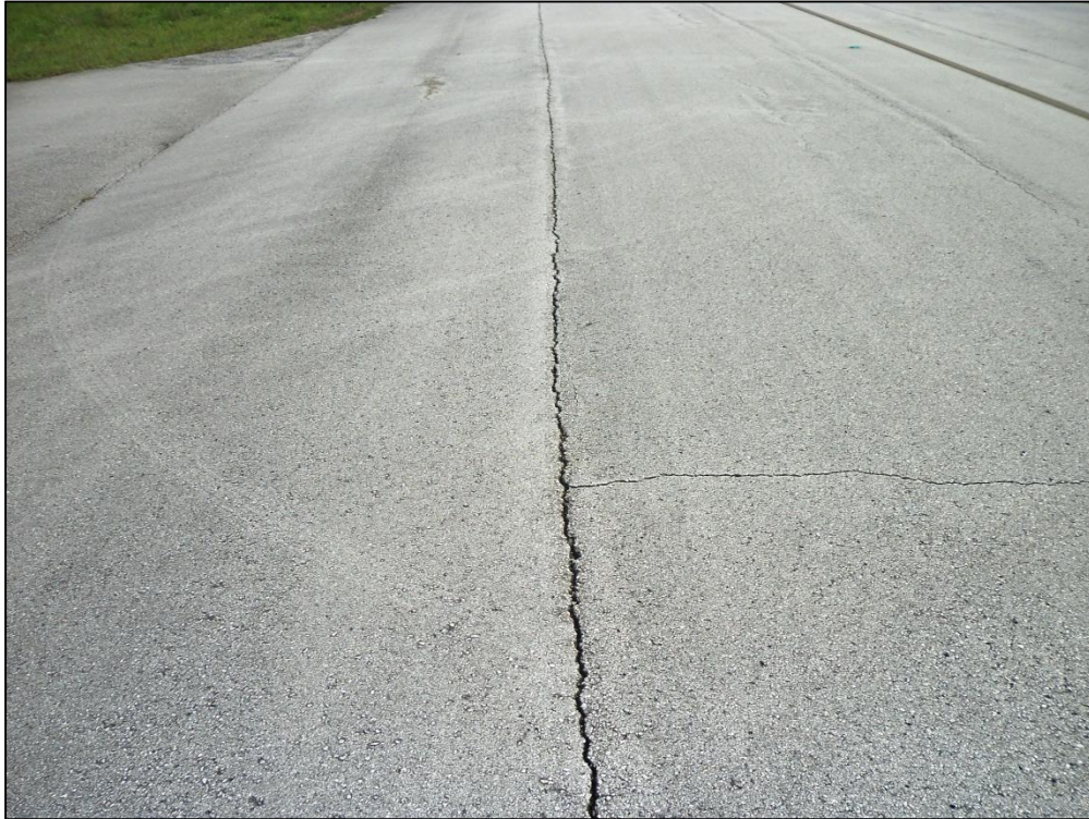
Taxiway East, Section 110, Sample Unit 105 – Low and Medium Severity (48) Longitudinal and Transverse Cracking, Low Severity (52) Raveling, Low Severity (57) Weathering
