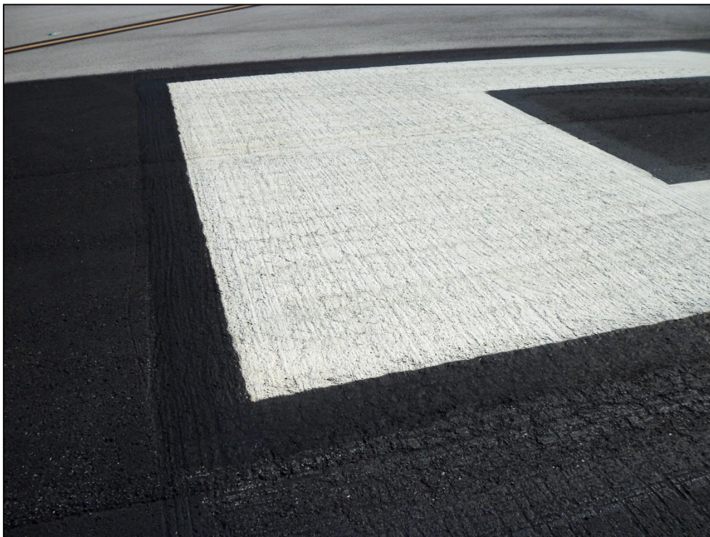
Runway 10-28, Section 6105, Sample Unit 101 –Low Severity (52) Raveling
