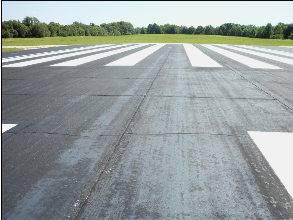
Runway 5-23, Section 6215, Sample Unit 195 – Low Severity (63) Longitudinal, Transverse, Diagonal Cracking
