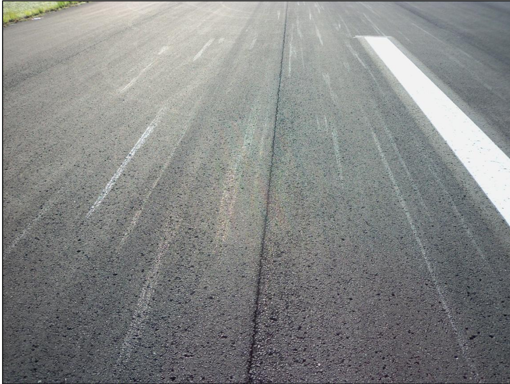
Runway 10-28, Section 6105, Sample Unit 185 – Low Severity (48) Longitudinal and Transverse Cracking, Low Severity (52) Raveling
