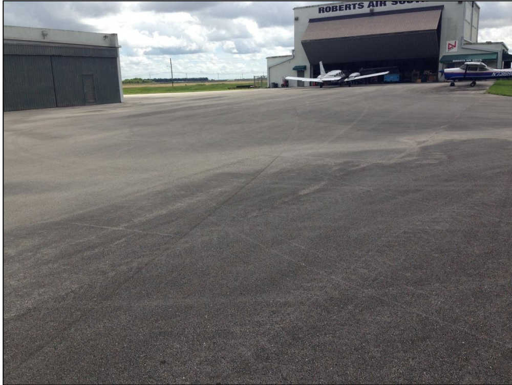
Apron NE, Section 4305, Sample Unit 204 – Low Severity (48) Longitudinal and Transverse Cracking, Low Severity (57) Weathering
