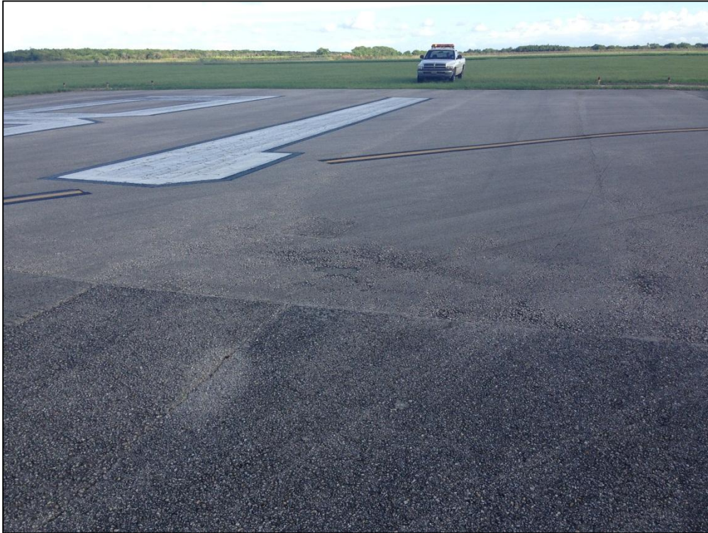
Runway 18-36, Section 6110, Sample Unit 576 – Low Severity (48) Longitudinal and Transverse Cracking, Medium Severity (57) Weathering, Low Severity (52) Raveling
