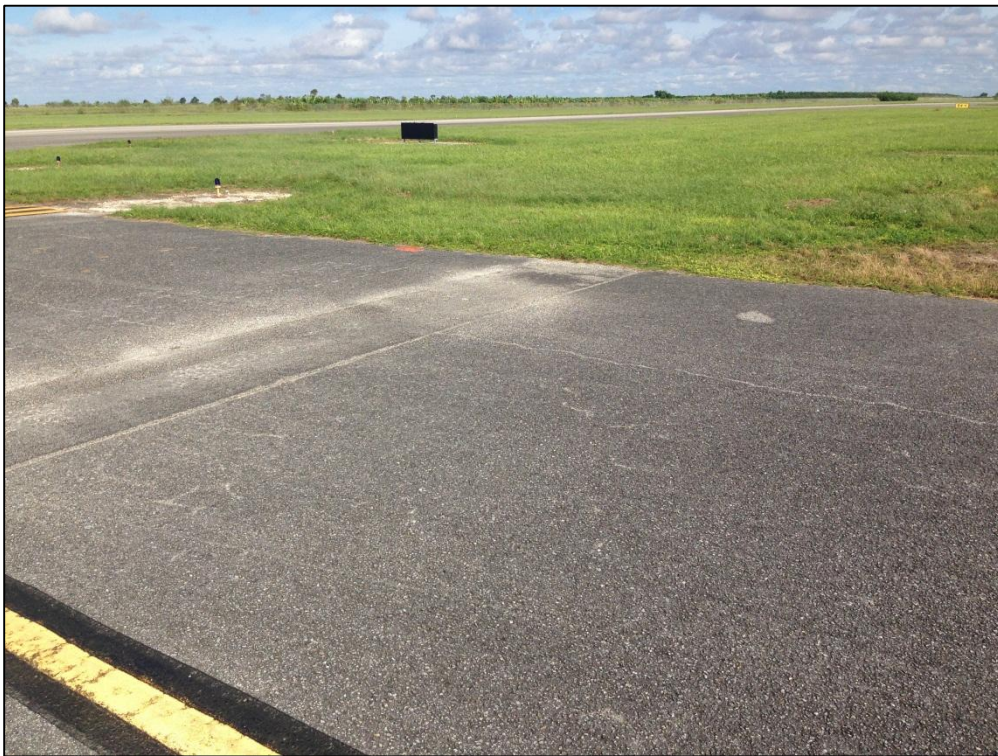
Taxiway B3, Section 130, Sample Unit 302 – Low Severity (48) Longitudinal and Transverse Cracking, Low Severity (52) Raveling, Low Severity (50) Patching
