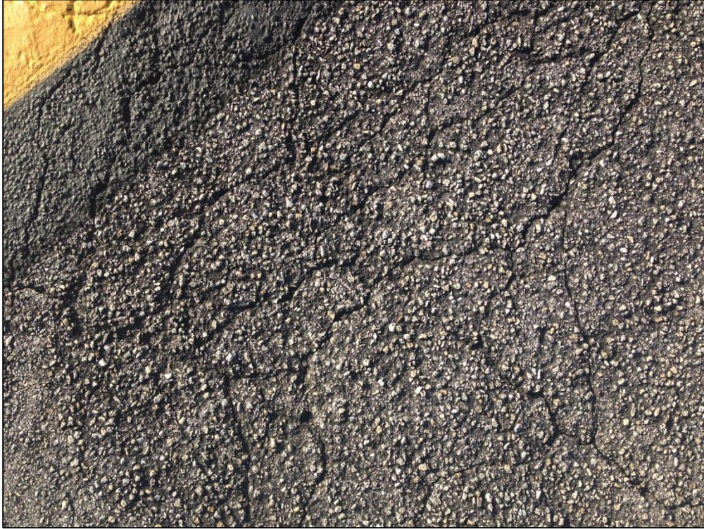
Taxiway A1, Section 230, Sample Unit 100 – Low Severity (41) Alligator Cracking
