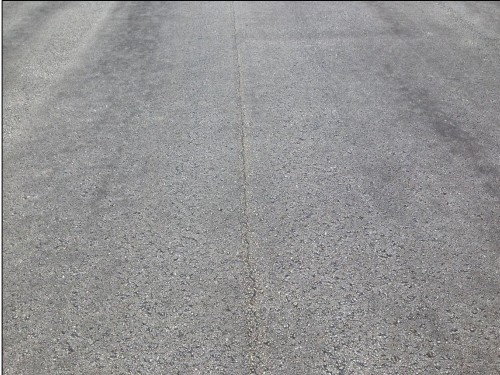
Runway 10-28, Section 6205, Sample Unit 149 – Low Severity (48) Longitudinal and Transverse Cracking, Low Severity (57) Weathering
