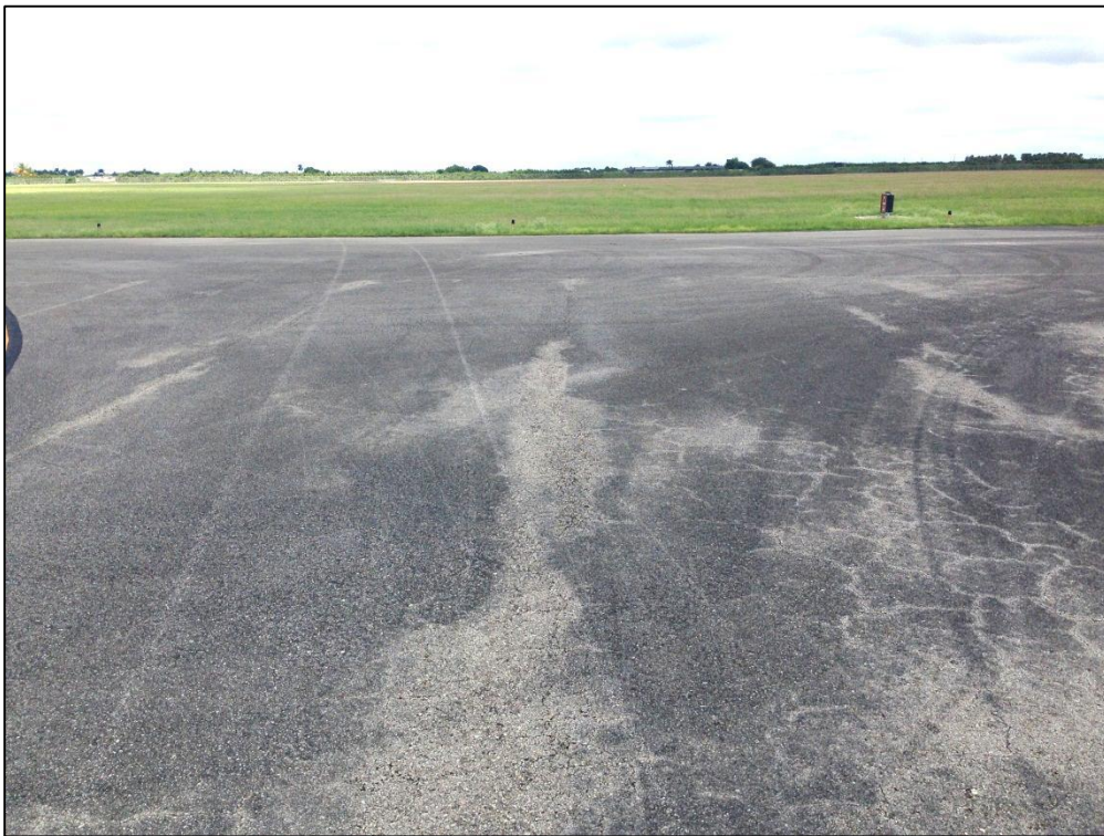
Taxiway AP, Section 305, Sample Unit 100 – Low Severity (48) Longitudinal and Transverse Cracking, Low and Medium Severity (52) Raveling, Low Severity (43) Block Cracking
