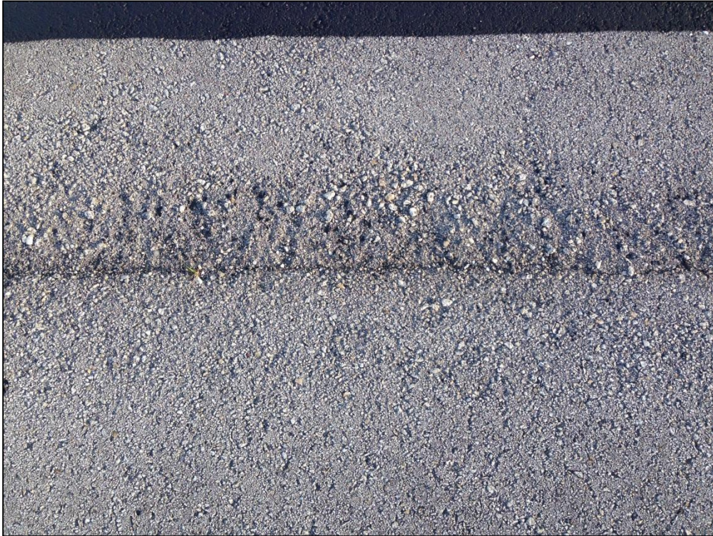
Runway 10-28, Section 6205, Sample Unit 159 – Low Severity (48) Longitudinal and Transverse Cracking, Medium Severity (52) Raveling
