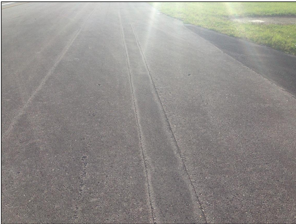
Runway 10-28, Section 6205, Sample Unit 131 – Low Severity (48) Longitudinal and Transverse Cracking, Low Severity (57) Weathering, Low Severity (50) Patching
