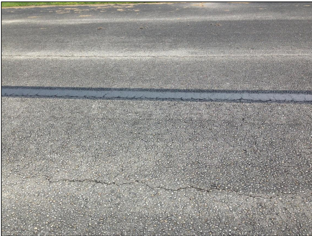
Taxiway B, Section 180, Sample Unit 801 – Low Severity (48) Longitudinal and Transverse Cracking, Low Severity (57) Weathering, Low Severity (52) Raveling
