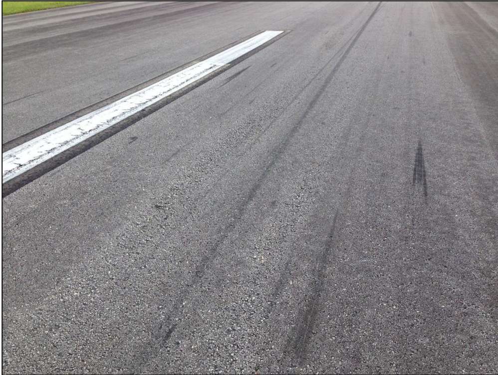
Runway 10-28, Section 6205, Sample Unit 149 – Low Severity (52) Raveling, Low Severity (57) Weathering
