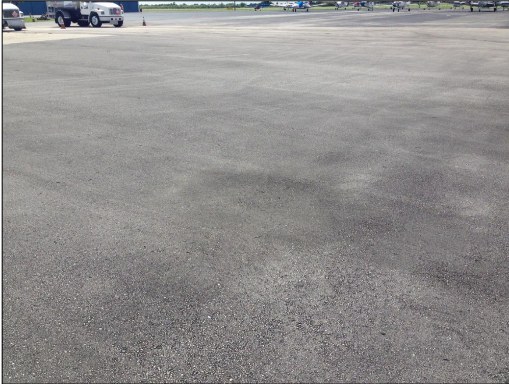
Apron NW, Section 4110, Sample Unit 200 – Low Severity (45) Depression, Low Severity (57) Weathering
