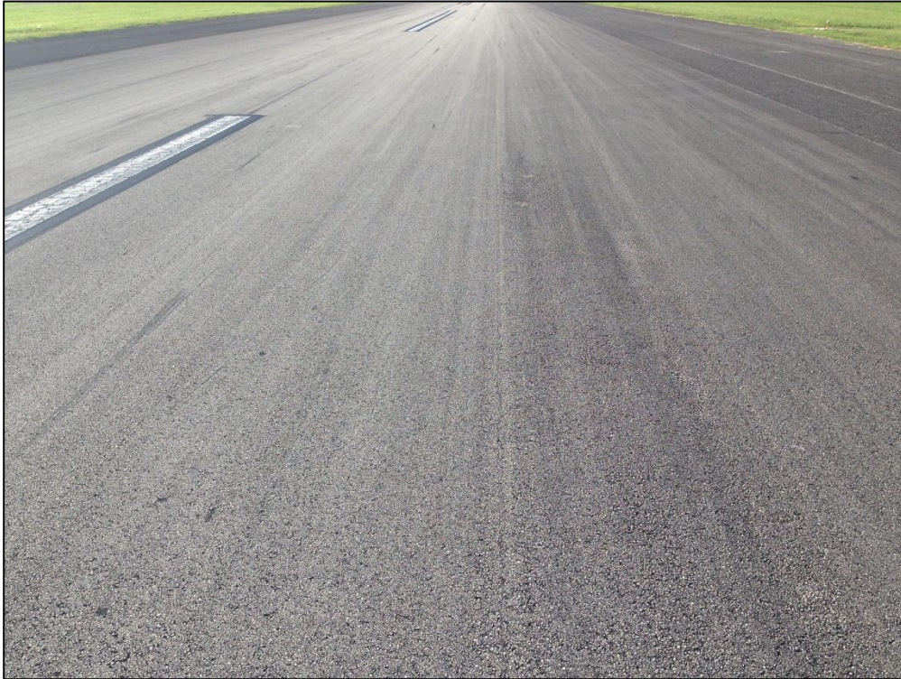
Runway 18-36, Section 6105, Sample Unit 329 – Low Severity (57) Weathering
