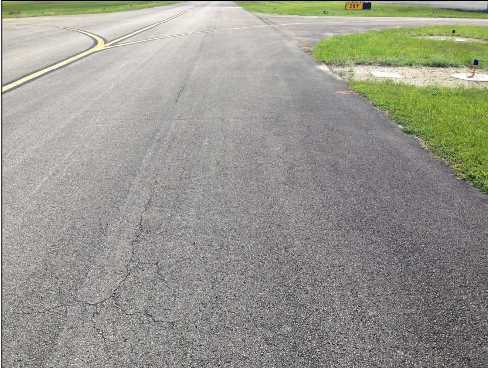
Taxiway A, Section 215, Sample Unit 117 – Low Severity (43) Block Cracking, Medium Severity (57) Weathering
