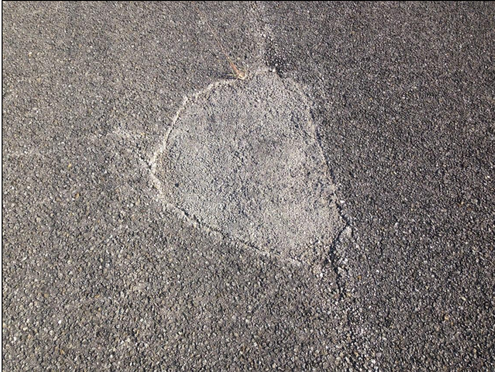
Runway 18-36, Section 6110, Sample Unit 560 – Low Severity (48) Longitudinal and Transverse Cracking, Medium Severity (57) Weathering, Low Severity (52) Raveling, Medium Severity (50) Patching
