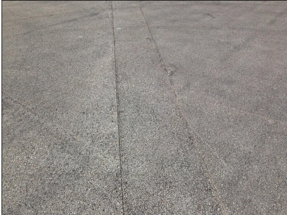
Apron NE, Section 4205, Sample Unit 403 – Low Severity (48) Longitudinal and Transverse Cracking, Medium Severity (57) Weathering, Low Severity (50) Patching
