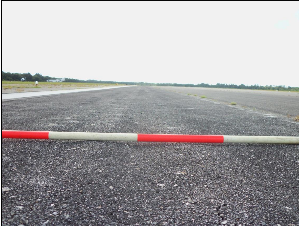
Runway 11-29, Section 6105, Sample Unit 164 – Low Severity (52) Raveling, Low Severity (57) Weathering, Low and Medium Severity (56) Swelling
