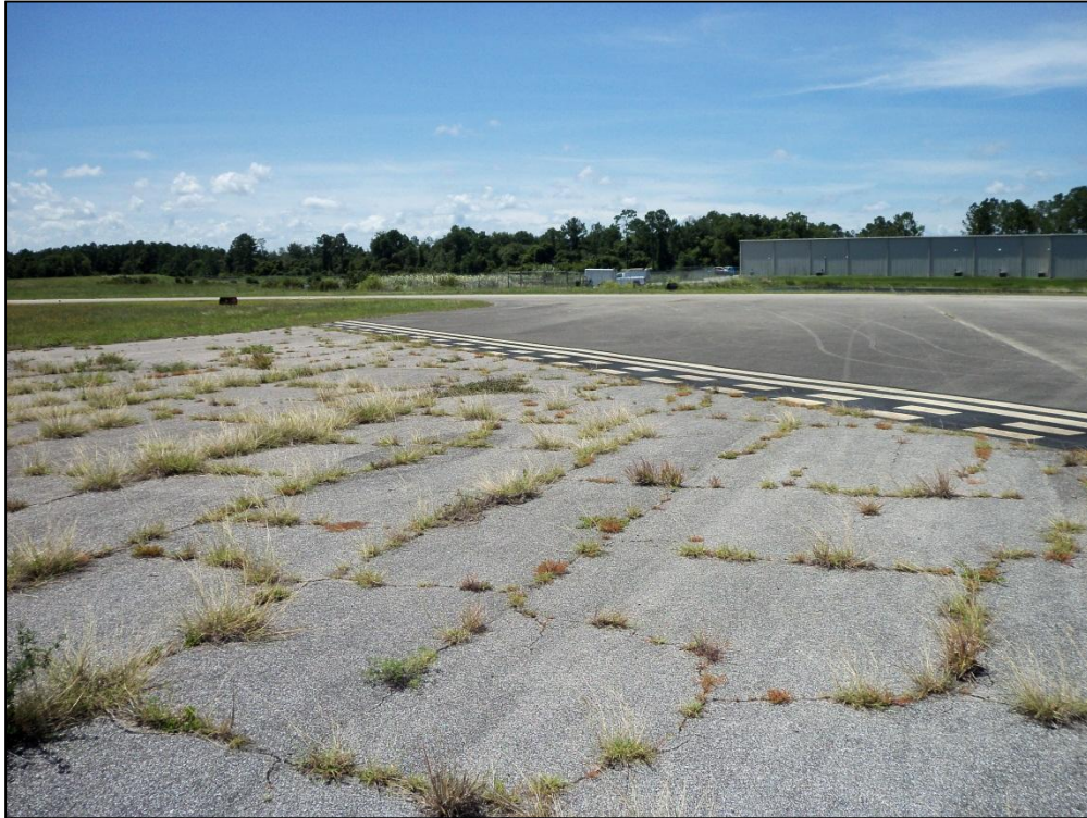
Apron Run-Up 11, Section 5103, Sample Unit 602 – Low Severity (52) Raveling, Low Severity (57) Weathering, Medium Severity (43) Block Cracking
