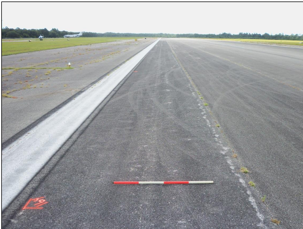
Runway 11-29, Section 6105, Sample Unit 164 – Low and Medium Severity (48) Longitudinal and Transverse Cracking, Low Severity (52) Raveling, Low Severity (57) Weathering, Low and Medium Severity (56) Swelling
