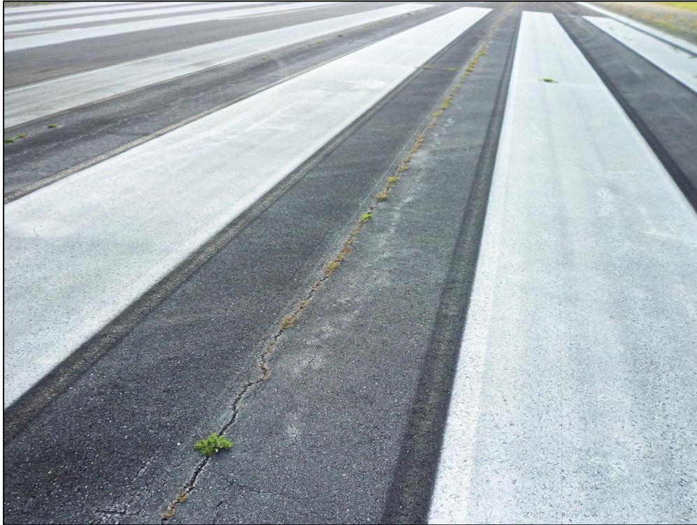
Runway 11-29, Section 6105, Sample Unit 199 – Low and Medium Severity (48) Longitudinal and Transverse Cracking, Low Severity (52) Raveling, Low Severity (57) Weathering, Low Severity (56) Swelling
