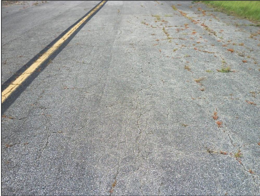
Taxiway Delta, Section 405, Sample Unit 101 – Low Severity (52) Raveling, Low Severity (57) Weathering, Low and Medium Severity (43) Block Cracking, Low Severity (41) Alligator Cracking
