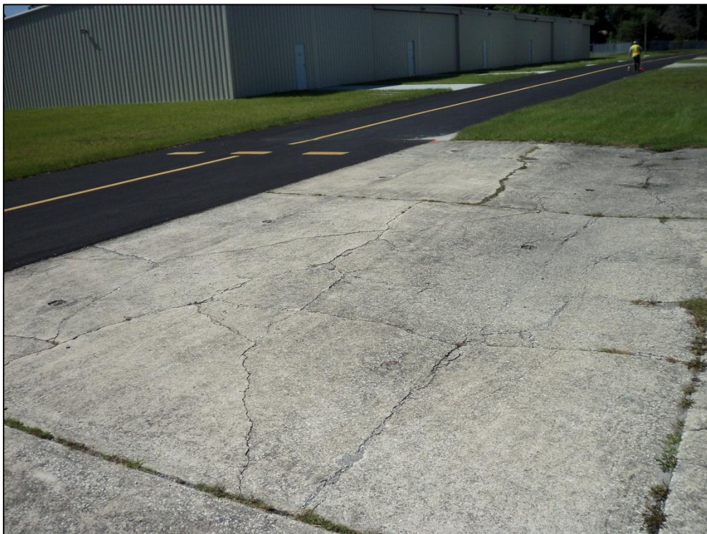
Apron, Section 4105, Sample Unit 101 – High Severity (72) Shattered Slab
