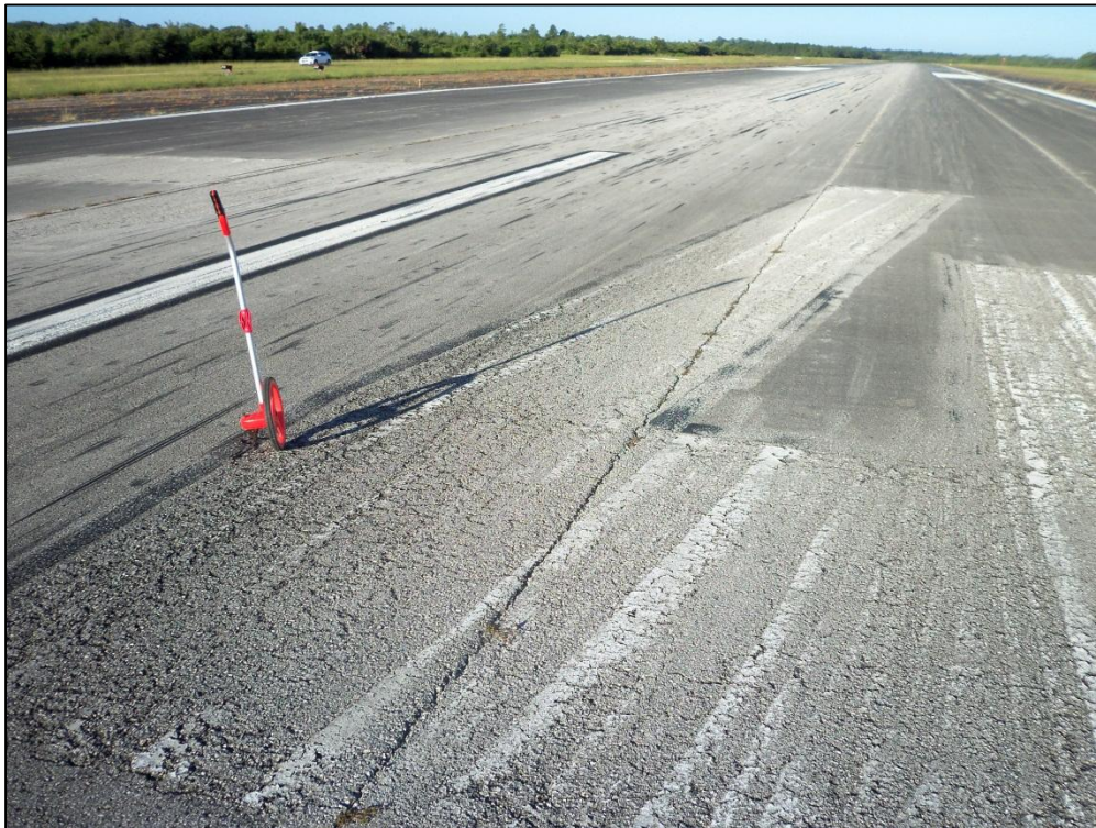
Runway 6-24, Section 6205, Sample Unit 188 – Low and Medium Severity (48) Longitudinal and Transverse Cracking, Low and High Severity (52) Raveling
