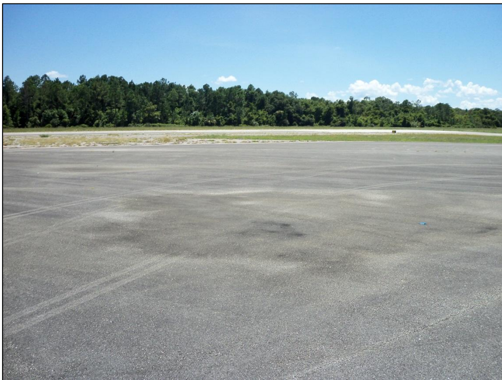
Apron Run-Up 11, Section 5105, Sample Unit 301 – Low Severity (48) Longitudinal and Transverse Cracking, Low Severity (52) Raveling, Low Severity (57) Weathering, Low Severity (45) Depression
