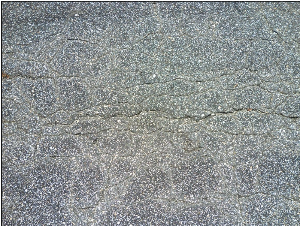
Taxiway Delta, Section 405, Sample Unit 101 – Low Severity (52) Raveling, Low Severity (57) Weathering, Low Severity (41) Alligator Cracking
