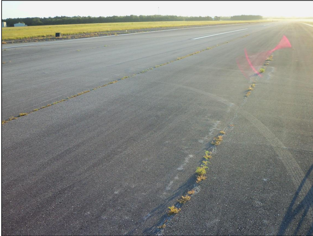
Runway 6-24, Section 6205, Sample Unit 145 – Low and Medium Severity (48) Longitudinal and Transverse Cracking, Low Severity (52) Raveling, Low Severity (57) Weathering, Low Severity (56) Swelling
