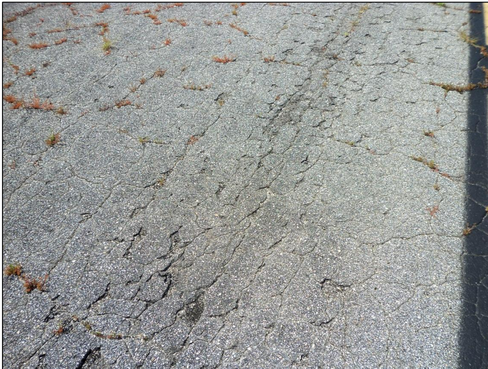
Taxiway D, Section 405, Sample Unit 103 – Low Severity (52) Raveling, Low Severity (57) Weathering, Medium Severity (43) Block Cracking, Medium Severity (41) Alligator Cracking
