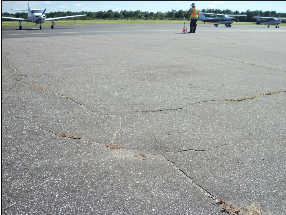
Apron, Section 4115, Sample Unit 401 – Low Severity (57) Weathering, Medium Severity (43) Block Cracking, Low Severity (45) Depression
