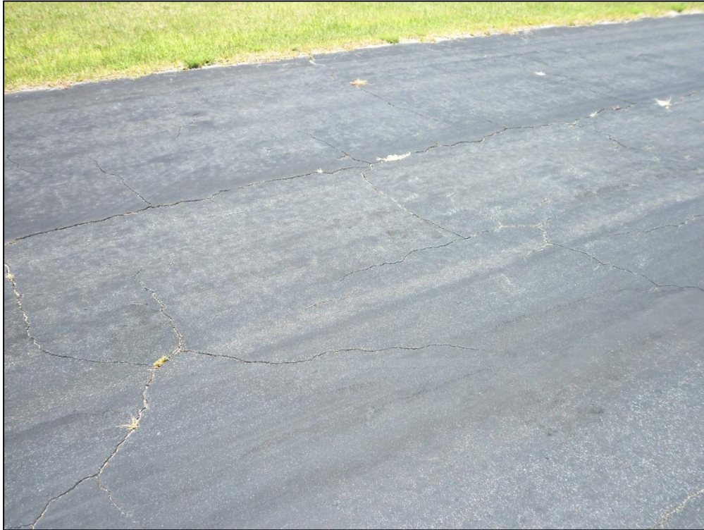
Taxiway Alpha, Section 105, Sample Unit 129 – Low and Medium Severity (43) Block Cracking
