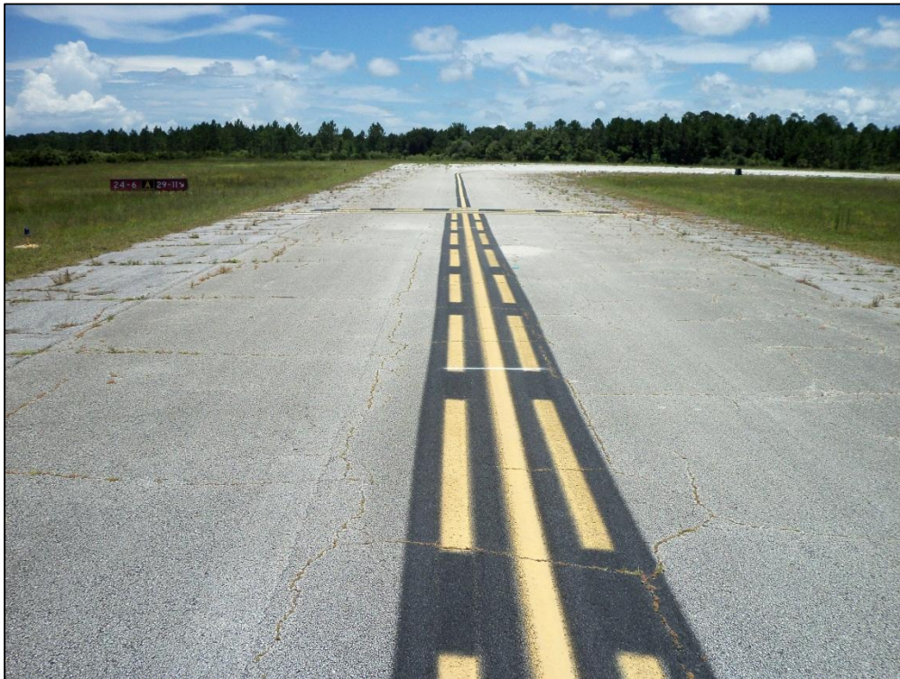
Taxiway Alpha, Section 110, Sample Unit 148 – Low Severity (52) Raveling, Medium Severity (57) Weathering, Medium Severity (43) Block Cracking
