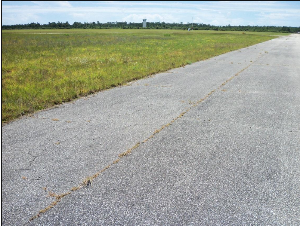
Taxiway Charlie, Section 315, Sample Unit 111 – Low and Medium Severity (48) Longitudinal and Transverse Cracking, Low Severity (52) Raveling, Low Severity (57) Weathering, Low Severity (43) Block Cracking
