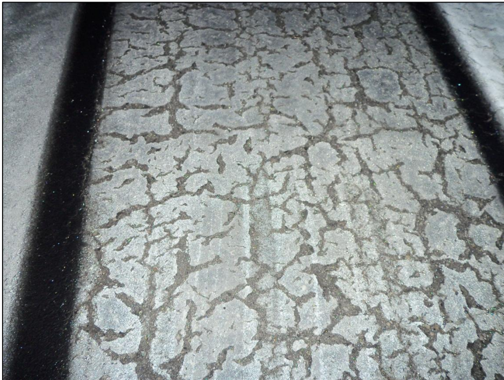
Runway 6-24, Section 6205, Sample Unit 100 – Medium Severity (52) Raveling
