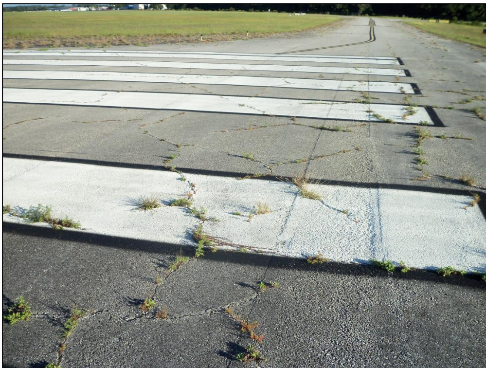
Runway 6-24, Section 6205, Sample Unit 199– Low and Medium Severity (48) Longitudinal and Transverse Cracking, Low and Medium Severity (52) Raveling, Low Severity (43) Block Cracking
