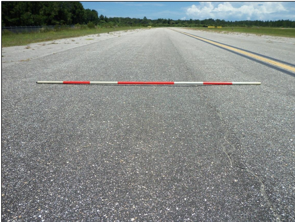
Taxiway Alpha, Section 105, Sample Unit 141 – Low Severity (57) Weathering, Low Severity (52) Raveling, Low Severity (43) Block Cracking, Low Severity (53) Rutting
