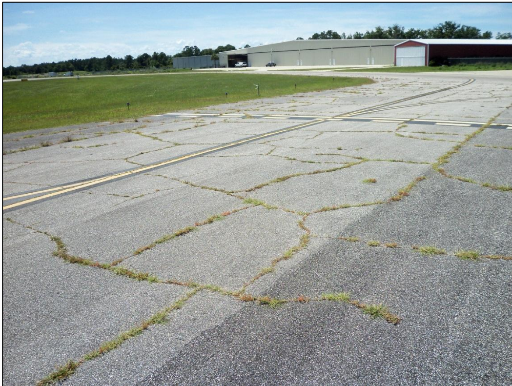
Taxiway Charlie, Section 307, Sample Unit 104 – Low Severity (52) Raveling, Low Severity (57) Weathering, Medium Severity (43) Block Cracking
