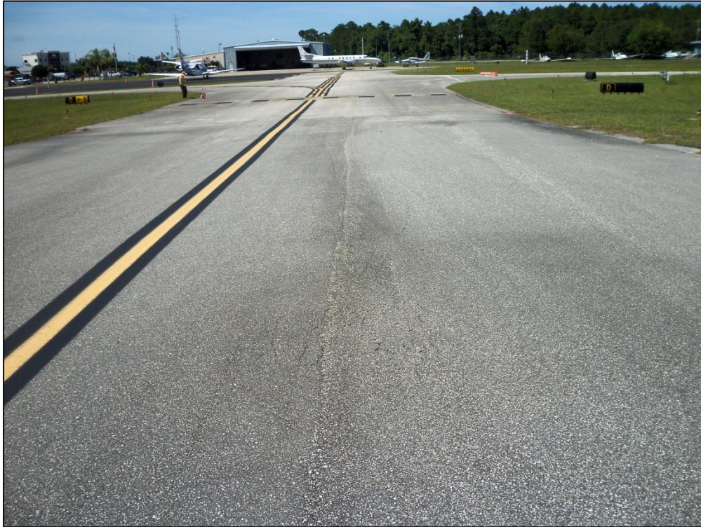
Taxiway Delta, Section 414, Sample Unit 100 – Low Severity (48) Longitudinal and Transverse Cracking, Low Severity (57) Weathering, Low Severity (53) Rutting
