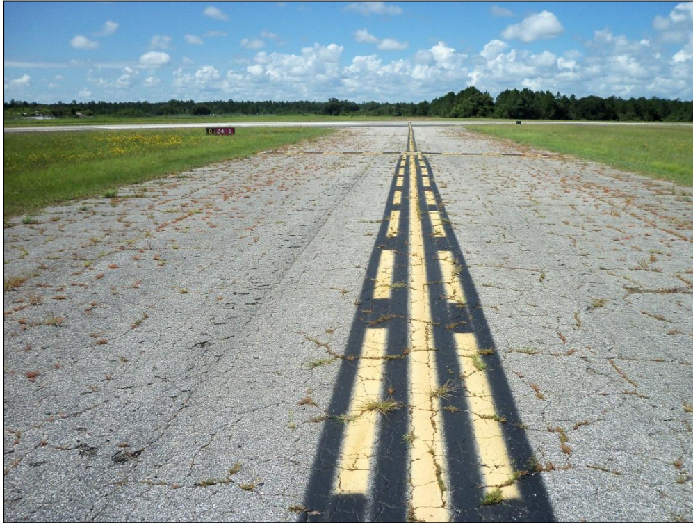
Taxiway Delta, Section 405, Sample Unit 103 – Medium Severity (52) Raveling, Medium Severity (43) Block Cracking, Medium Severity (41) Alligator Cracking
