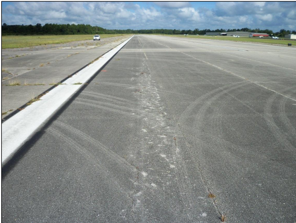
Runway 11-29, Section 6105, Sample Unit 153 – Low and Medium Severity (48) Longitudinal and Transverse Cracking, Low Severity (52) Raveling, Low Severity (57) Weathering, Low Severity (56) Swelling
