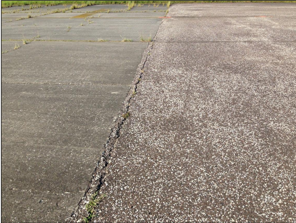
Taxiway B, Section 245, Sample Unit 134 – Medium Severity (52) Raveling, Low Severity (54) Shoving
