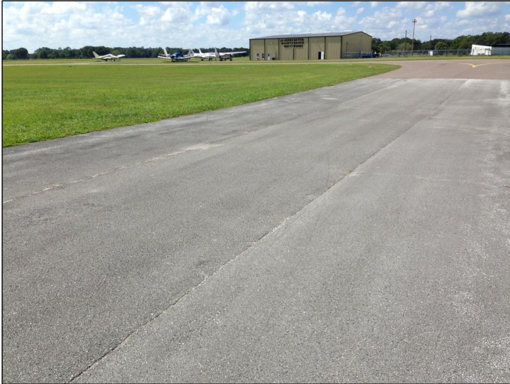
Taxiway C-1, Section 505, Sample Unit 101 – Low Severity (48) Longitudinal and Transverse Cracking, Low Severity (52) Raveling, Low Severity (57) Weathering
