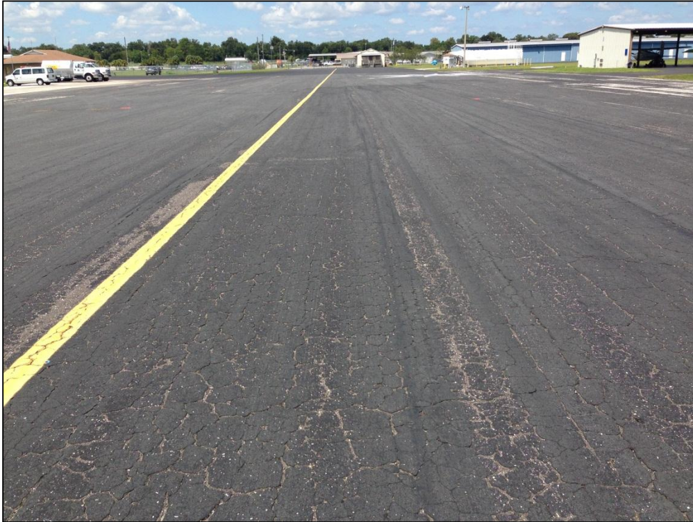
Taxiway B, Section 205, Sample Unit 108 – Medium Severity (43) Block Cracking, Medium Severity (52) Raveling
