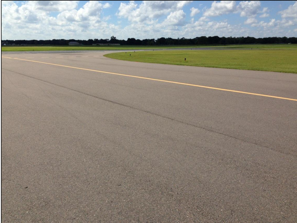
Taxiway C, Section 320, Sample Unit 101 – Low Severity (48) Longitudinal and Transverse Cracking, Low Severity (57) Weathering
