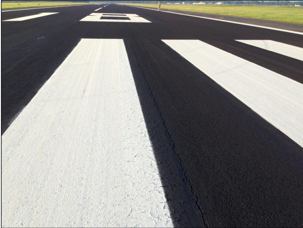
Runway 18-36, Section 6205, Sample Unit 390 – Low Severity (48) Longitudinal and Transverse Cracking, Low Severity (52) Raveling, Low Severity (57) Weathering
