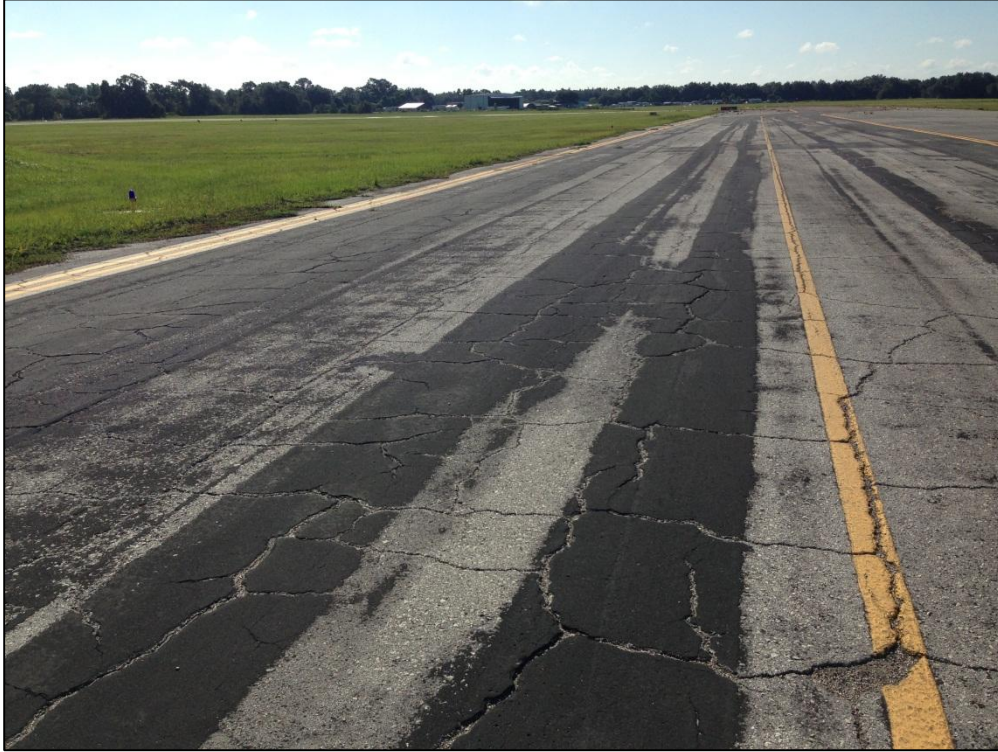
Taxiway B, Section 220, Sample Unit 219 – High Severity (43) Block Cracking, Medium Severity (52) Raveling
