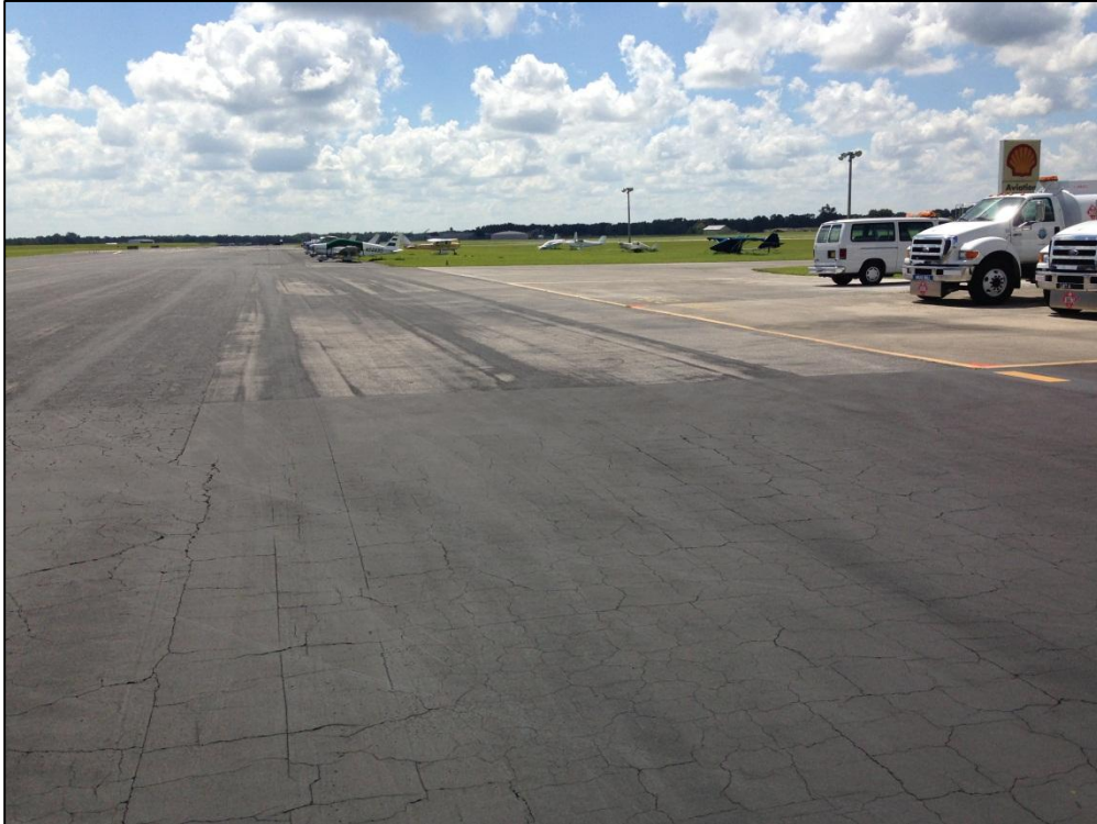
Apron NE, Section 5105, Sample Unit 200 – Low Severity (43) Block Cracking, Low Severity (52) Raveling, Low Severity (57) Weathering
