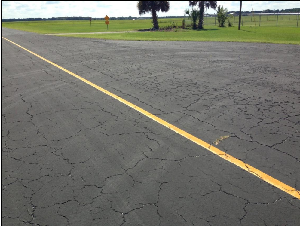
Apron TW D, Section 5205, Sample Unit 201 – Low Severity (43) Block Cracking, Low Severity (52) Raveling, Low Severity (57) Weathering
