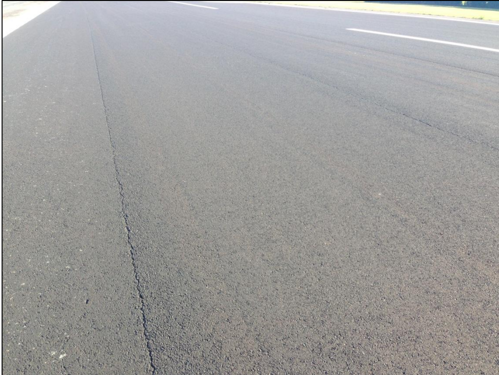
Runway 18-36, Section 6205, Sample Unit 320 – Low Severity (48) Longitudinal and Transverse Cracking, Low Severity (57) Weathering
