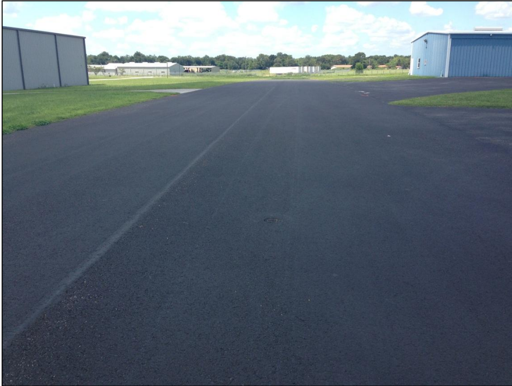
Taxiway E, Section 610, Sample Unit 104 – Low Severity (57) Weathering
