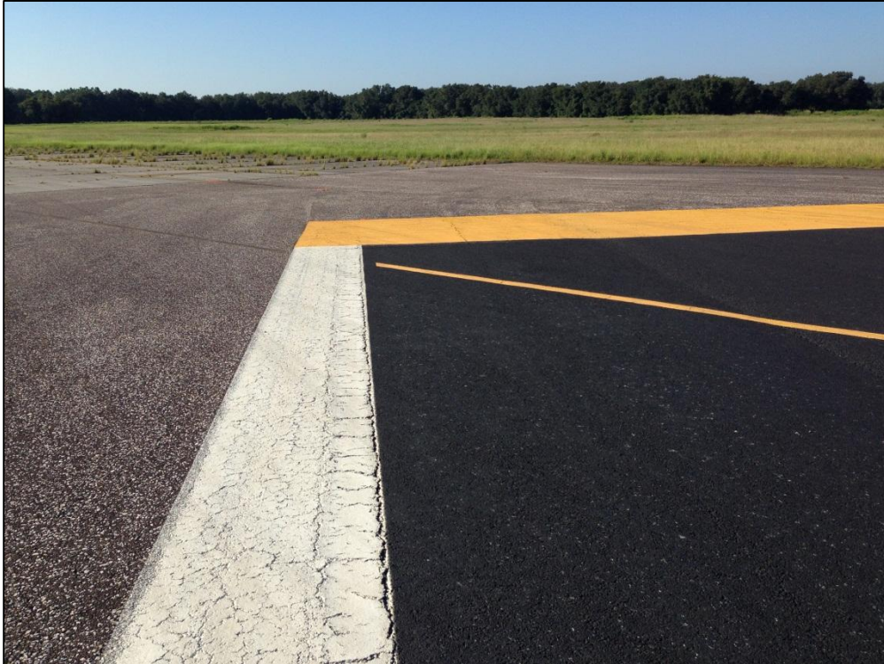
Runway 18-36, Section 6205, Sample Unit 299 – Low Severity (52) Raveling, Low Severity (57) Weathering
