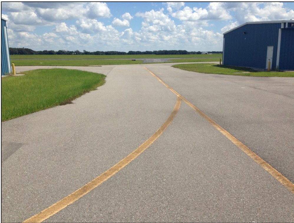
Apron T-Hang3, Section 5510, Sample Unit 102 – Low Severity (45) Depression, Low Severity (57) Weathering
