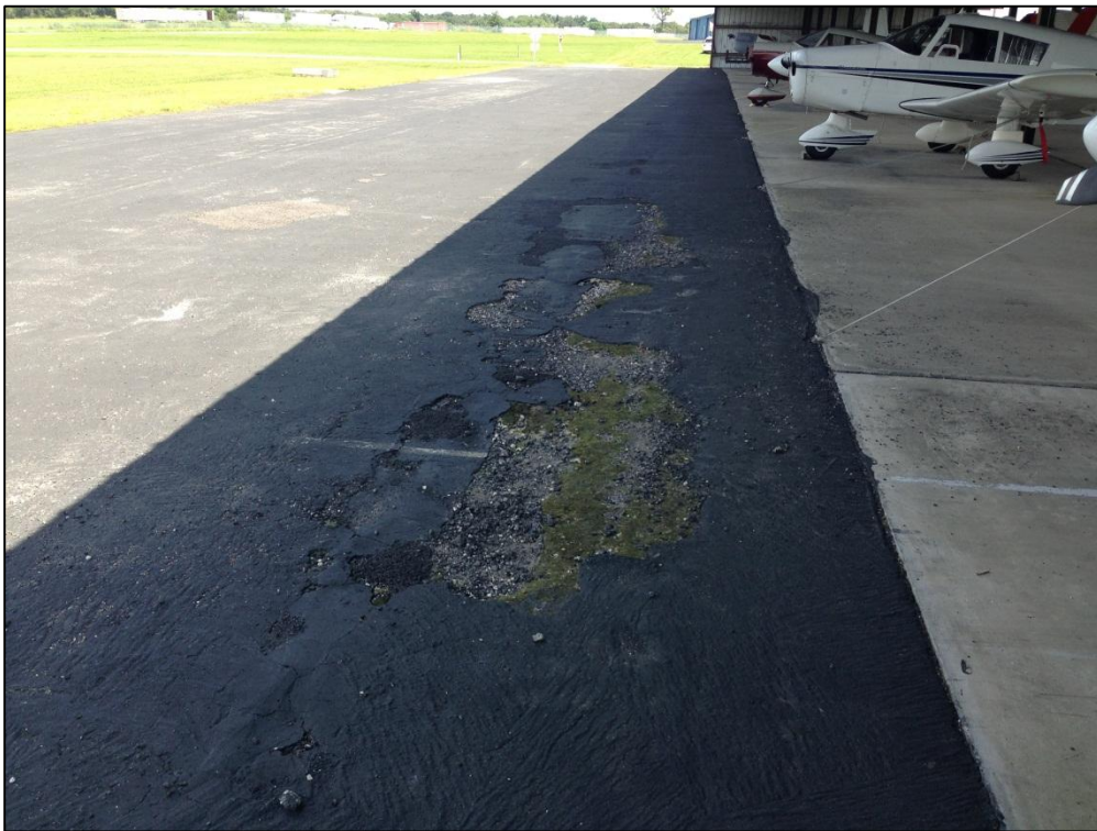
Apron T-Hang, Section 5305, Sample Unit 400 – High Severity (52) Raveling
