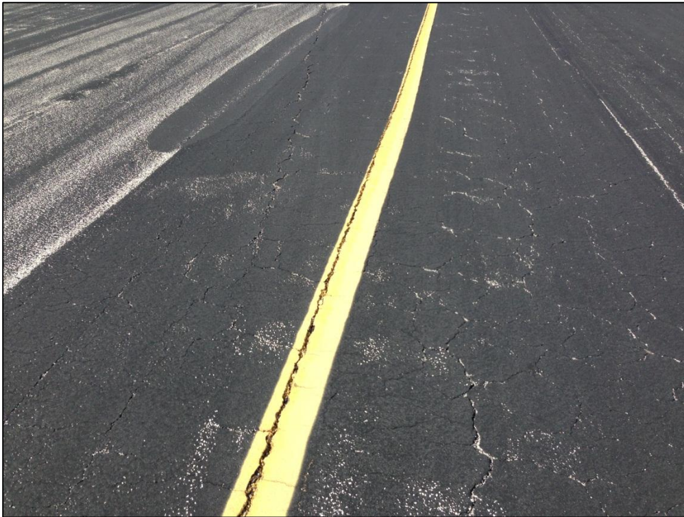
Taxiway A, Section 105, Sample Unit 149 – Low and Medium Severity (48) Longitudinal and Transverse Cracking, Low Severity (52) Raveling, Low Severity (57) Weathering
