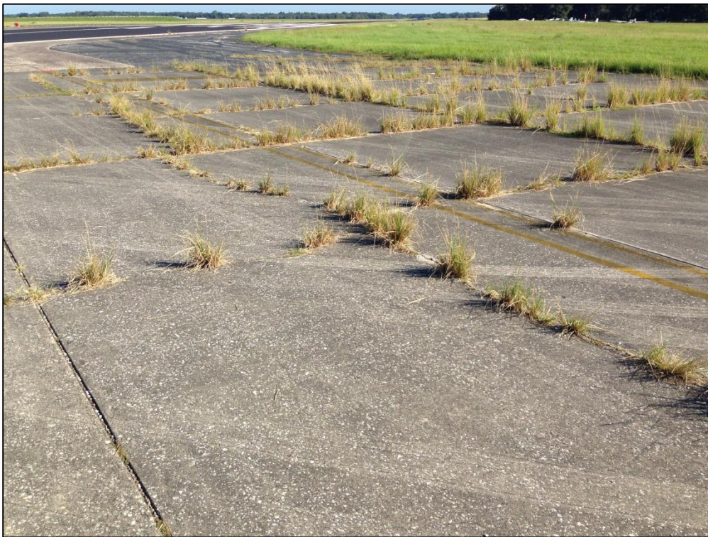
Taxiway B, Section 230, Sample Unit 135 – Medium Severity (72) Shattered Slab
