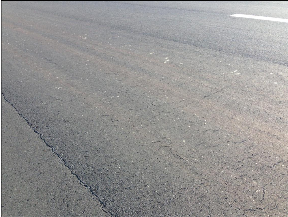
Runway 18-36, Section 6205, Sample Unit 313 – Low Severity (48) Longitudinal and Transverse Cracking, Low Severity (57) Weathering, Check Cracking
