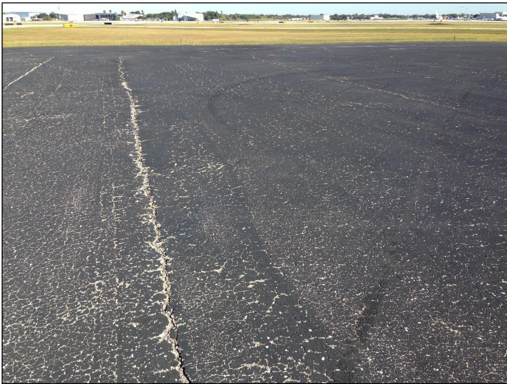
Apron Commercial, Section 4110, Sample Unit 708 – Low and Medium Severity (48) Longitudinal and Transverse Cracking, Medium Severity (52) Raveling
