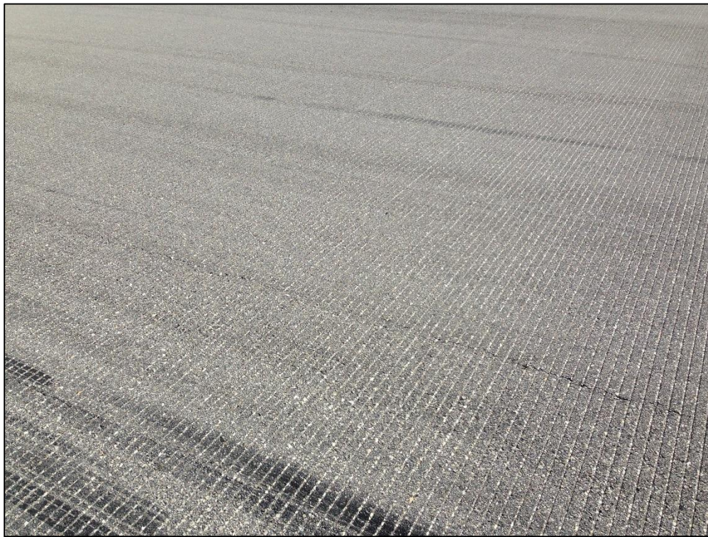
Runway 5-23, Section 6105, Sample Unit 331 – Low Severity (48) Longitudinal and Transverse Cracking, Low Severity (57) Weathering
