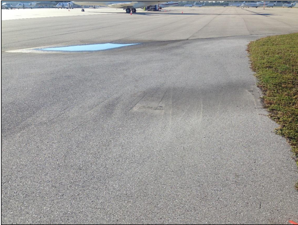
Taxiway Alpha, Section 165, Sample Unit 151 – Low Severity (45) Depression, Low Severity (57) Weathering
