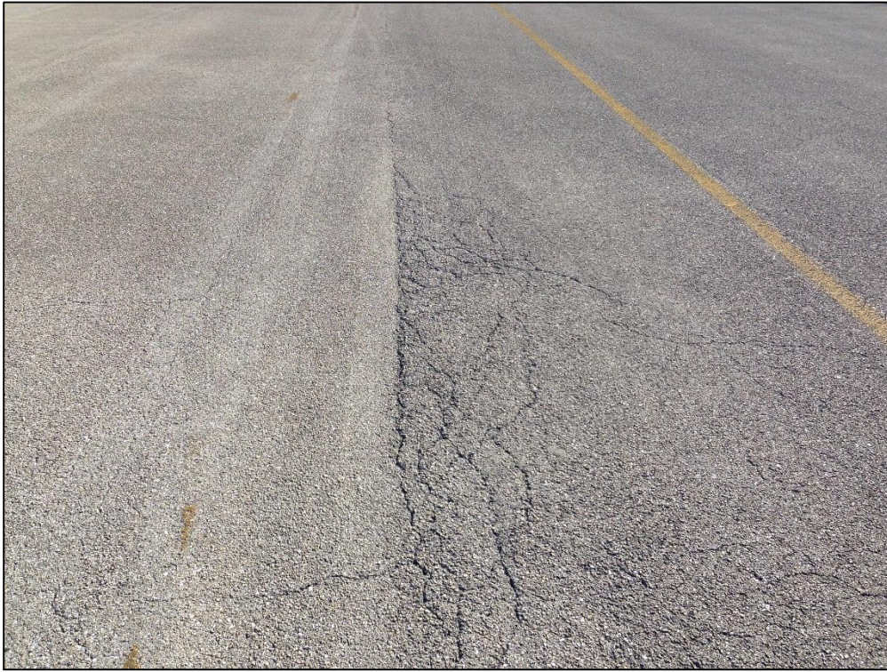
Apron GA, Section 4290, Sample Unit 254 – Low Severity (41) Alligator Cracking, Low Severity (52) Raveling, Medium Severity (52) Raveling
