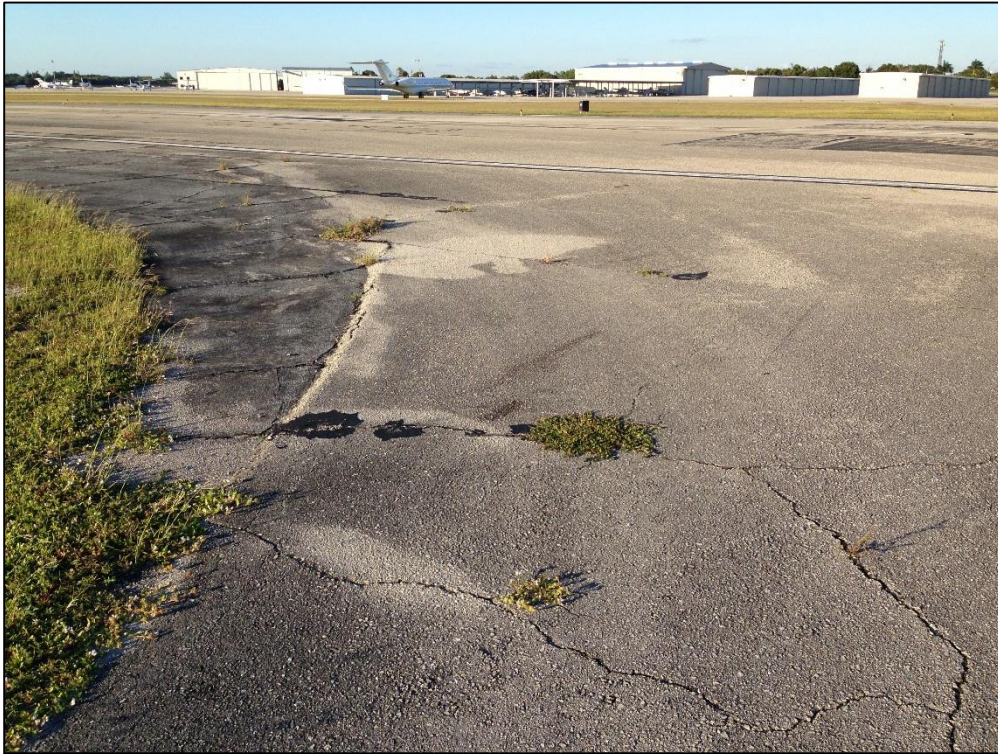
Taxiway Charlie, Section 310, Sample Unit 100 – Low Severity (43) Block Cracking, Low Severity (48) Longitudinal and Transverse Cracking, Low Severity (52) Raveling, Medium Severity (52) Raveling
