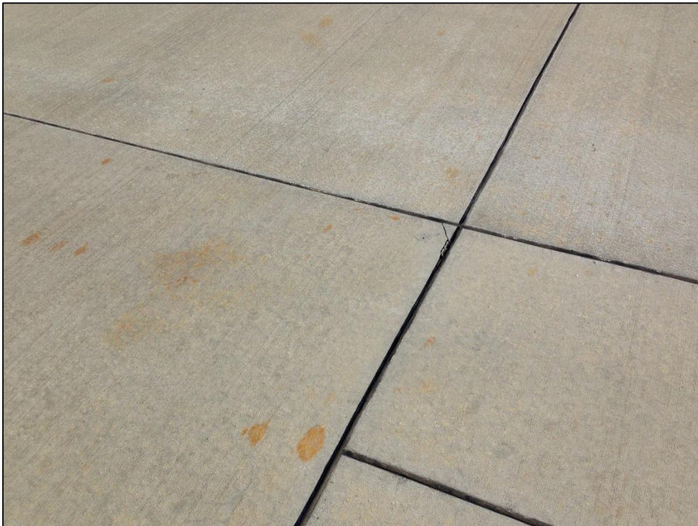
Apron GA, Section 4209, Sample Unit 655 – Low Severity (75) Corner Spalling
