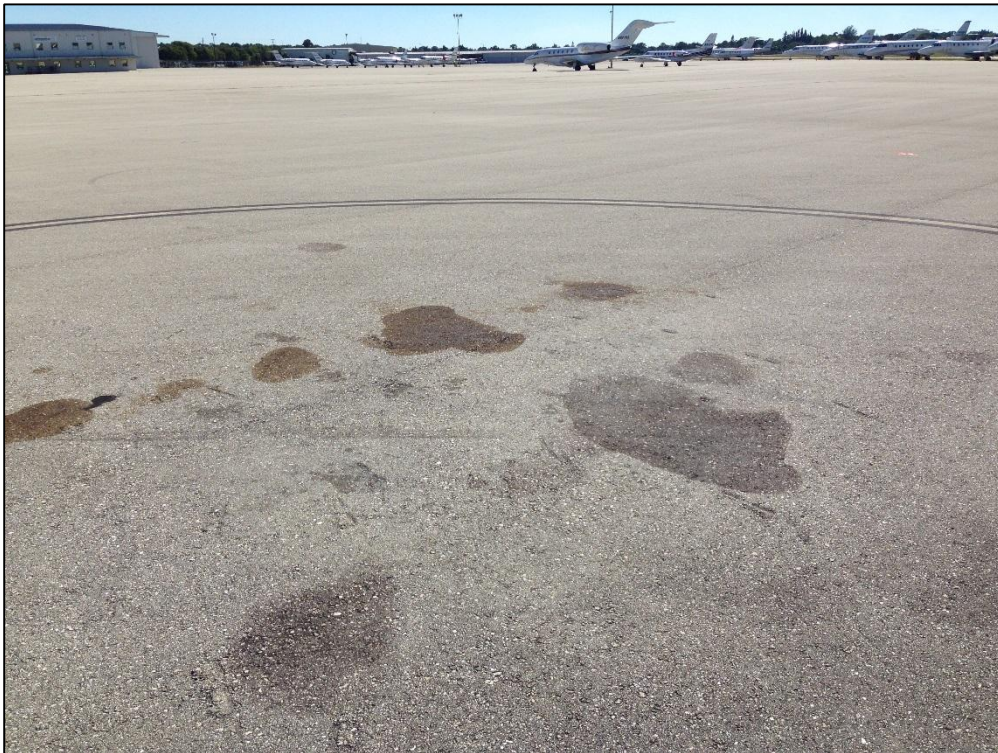
Apron GA, Section 4212, Sample Unit 152 – (49) Oil Spillage, Low Severity (57) Weathering
