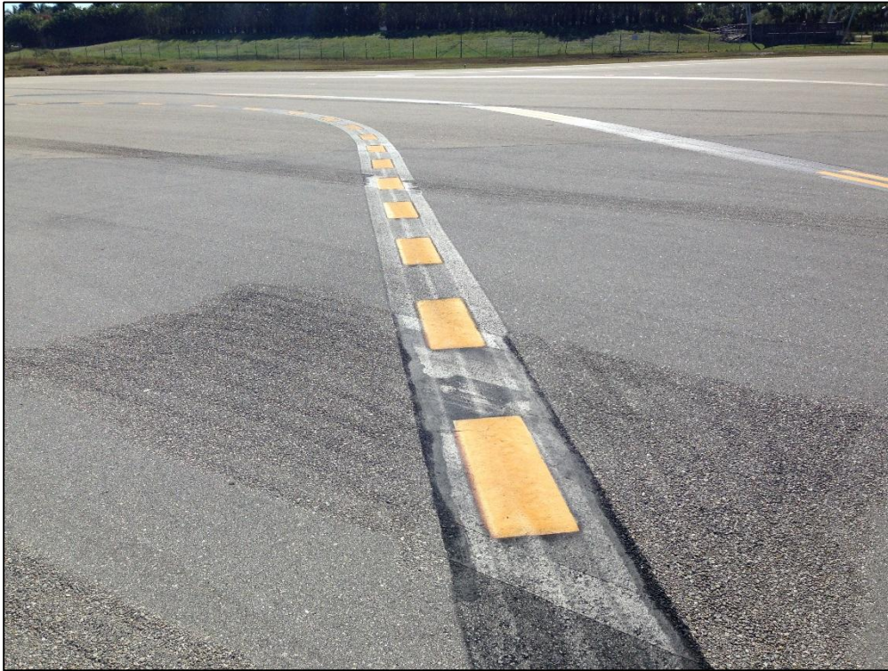
Taxiway A1, Section 105, Sample Unit 582 – Low Severity (52) Raveling, Low Severity (57) Weathering
