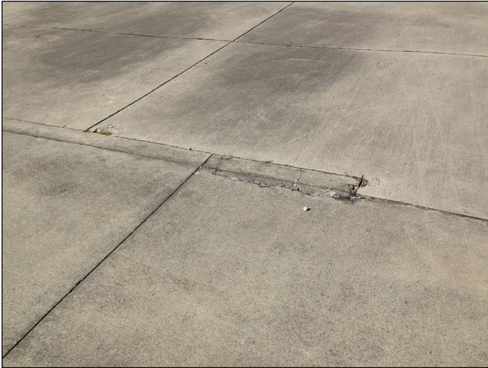
Apron GA, Section 4285, Sample Unit 202 – High Severity (65) Joint Seal Damage, High Severity (66) Small Patching
