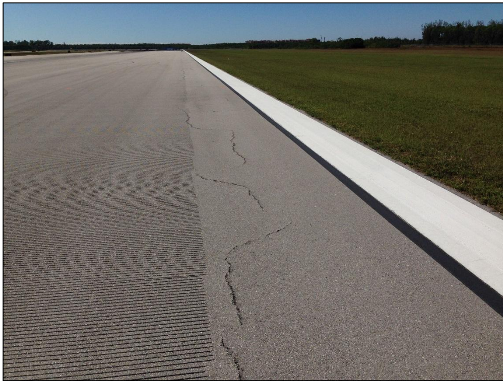
Runway 5-23, Section 6110, Sample Unit 144 – Low Severity (48) Longitudinal and Transverse Cracking, Low Severity (57) Weathering
