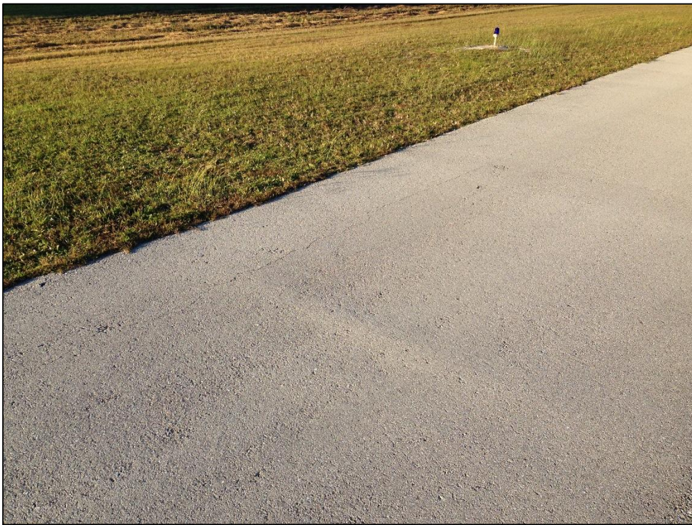
Taxiway Delta, Section 410, Sample Unit 102 – Low Severity (48) Longitudinal and Transverse Cracking, Low Severity (57) Weathering
