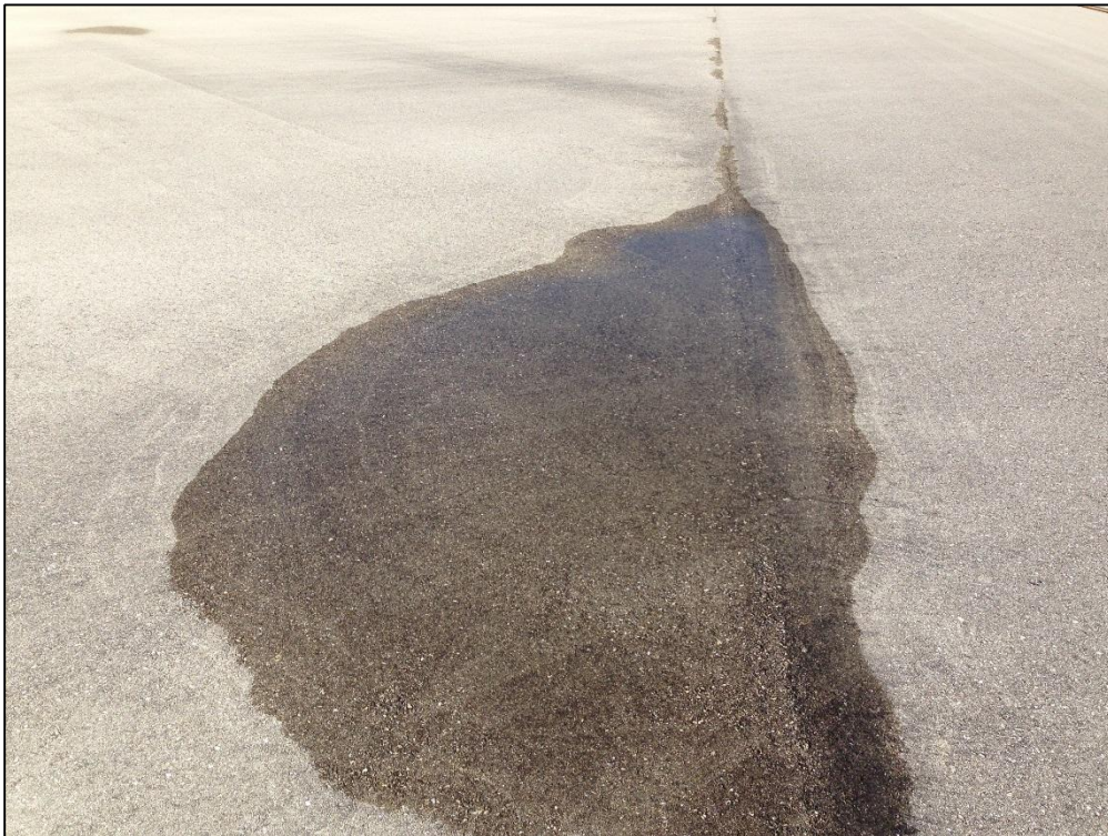
Taxiway A2, Section 106, Sample Unit 103 – Low Severity (45) Depression, Low Severity (57) Weathering
