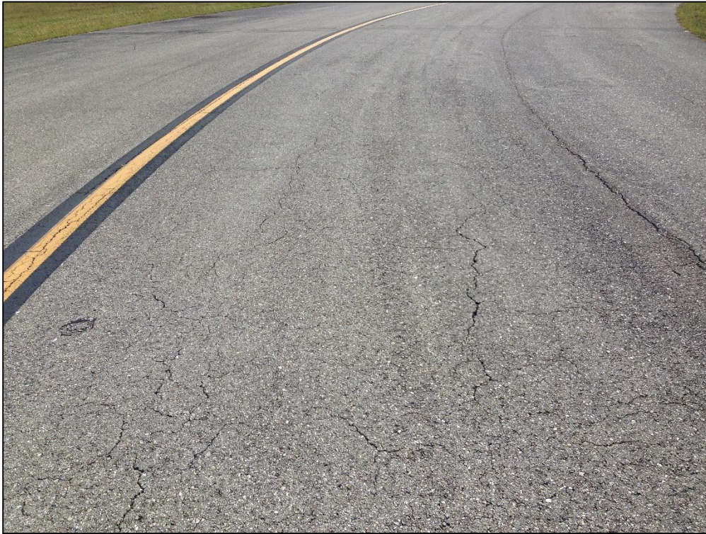
Taxiway Bravo, Section 205, Sample Unit 125 – Low Severity (43) Block Cracking, Low and Medium Severity (48) Longitudinal and Transverse Cracking, Low Severity (52) Raveling, Low Severity (56) Swelling
