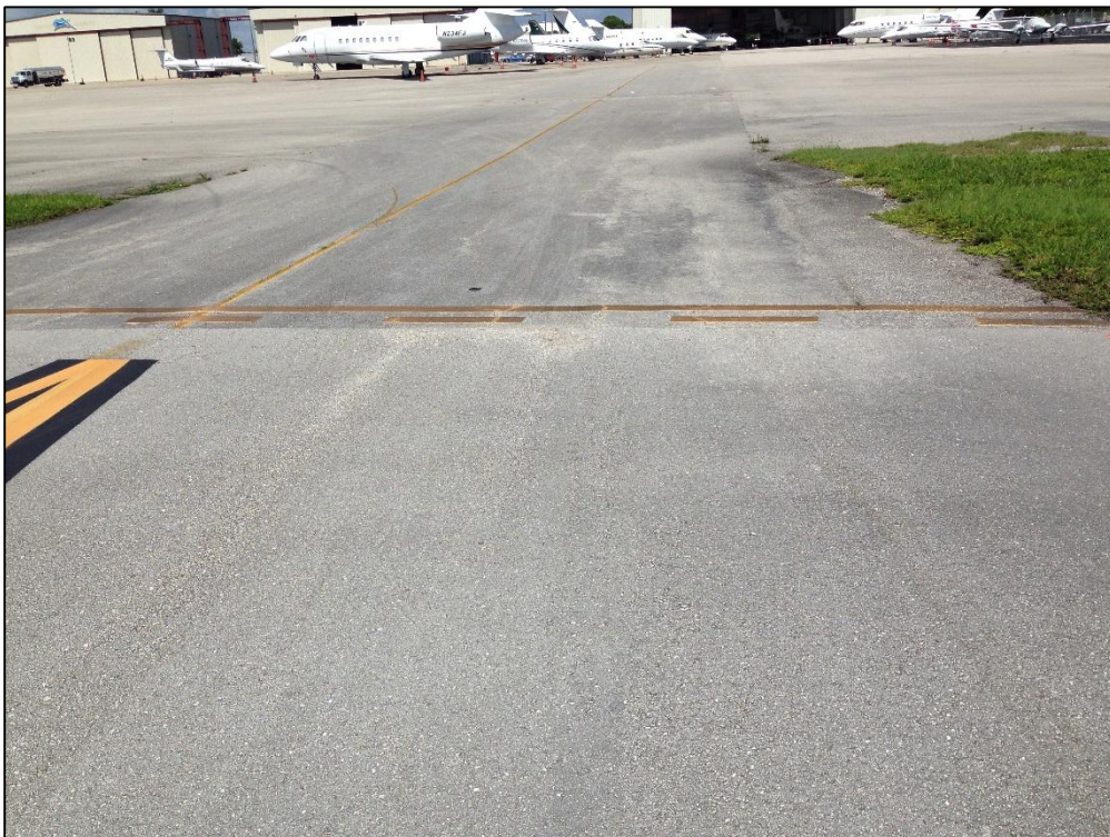
Taxiway Connector, Section 225, Sample Unit 803 – Low Severity (57) Weathering, Medium Severity (57) Weathering
