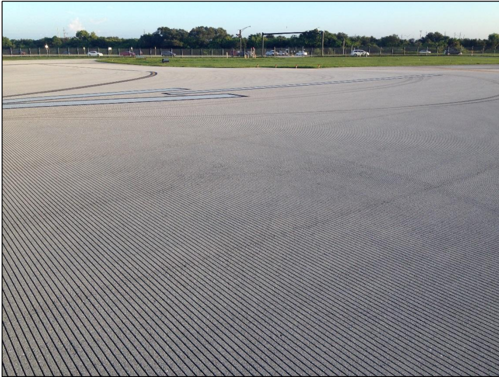
Runway 5-23, Section 6107, Sample Unit 409 – Low Severity (57) Weathering
