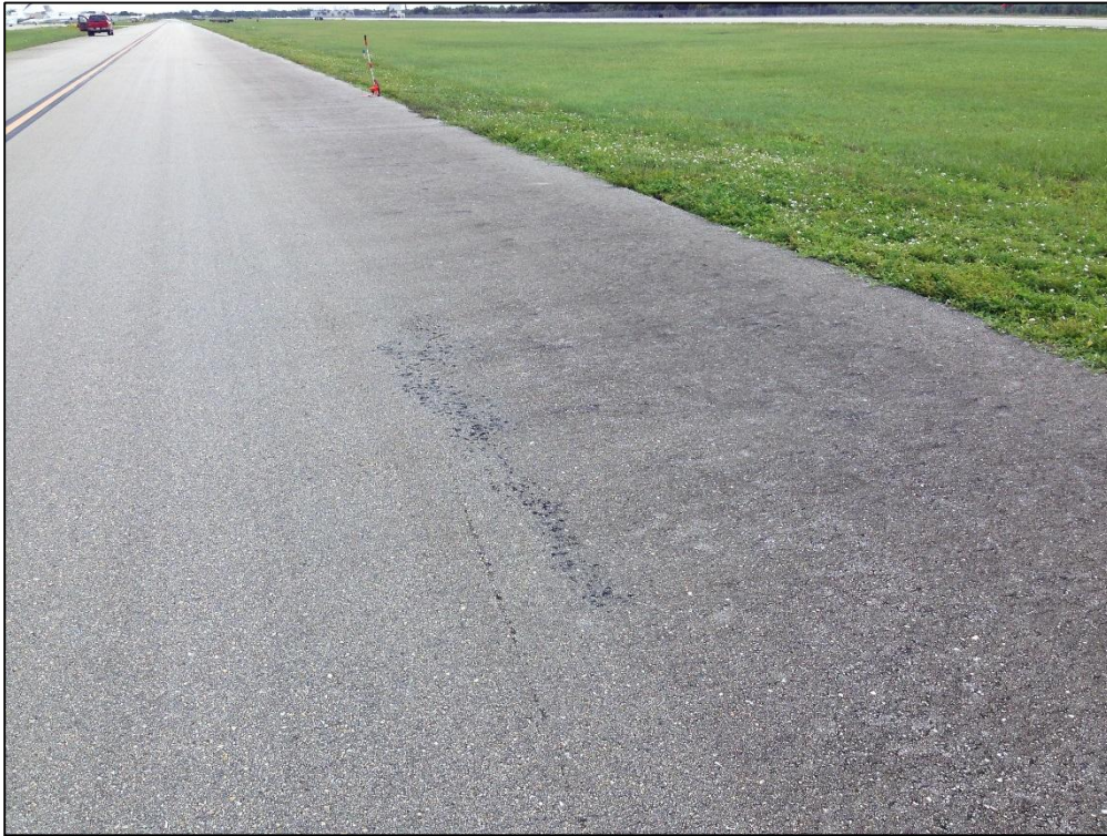
Taxiway Papa, Section 105, Sample Unit 105 – (42) Bleeding, Low Severity (57) Weathering
