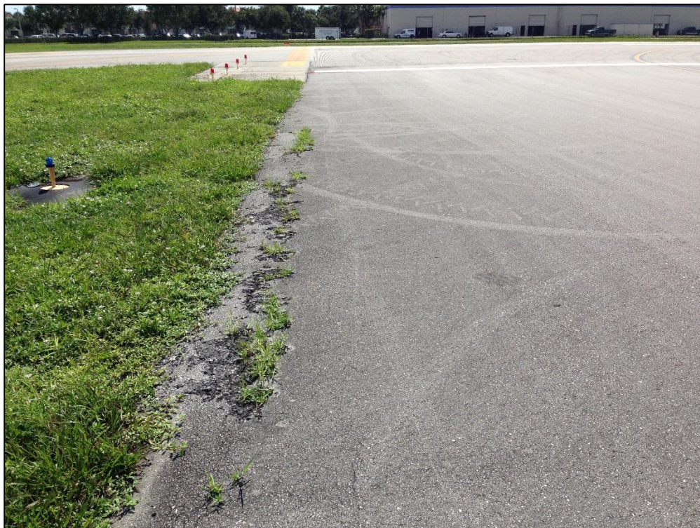
Taxiway Papa, Section 131, Sample Unit 100 – Low Severity (52) Raveling, Medium Severity (52) Raveling, Low Severity (57) Weathering
