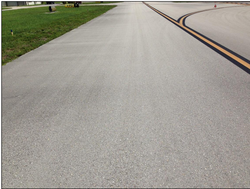
Taxiway Papa, Section 105, Sample Unit 150 – Low Severity (57) Weathering
