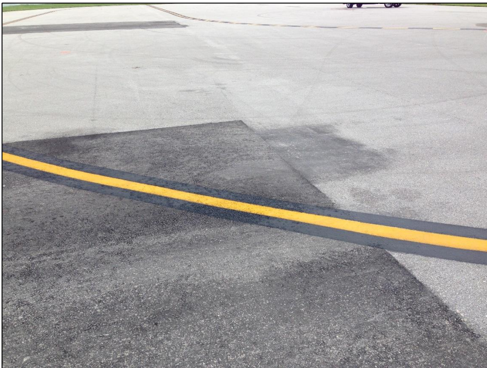
Apron Run-Up, Section 5115, Sample Unit 201 – Low Severity (50) Patching, Low Severity (57) Weathering
