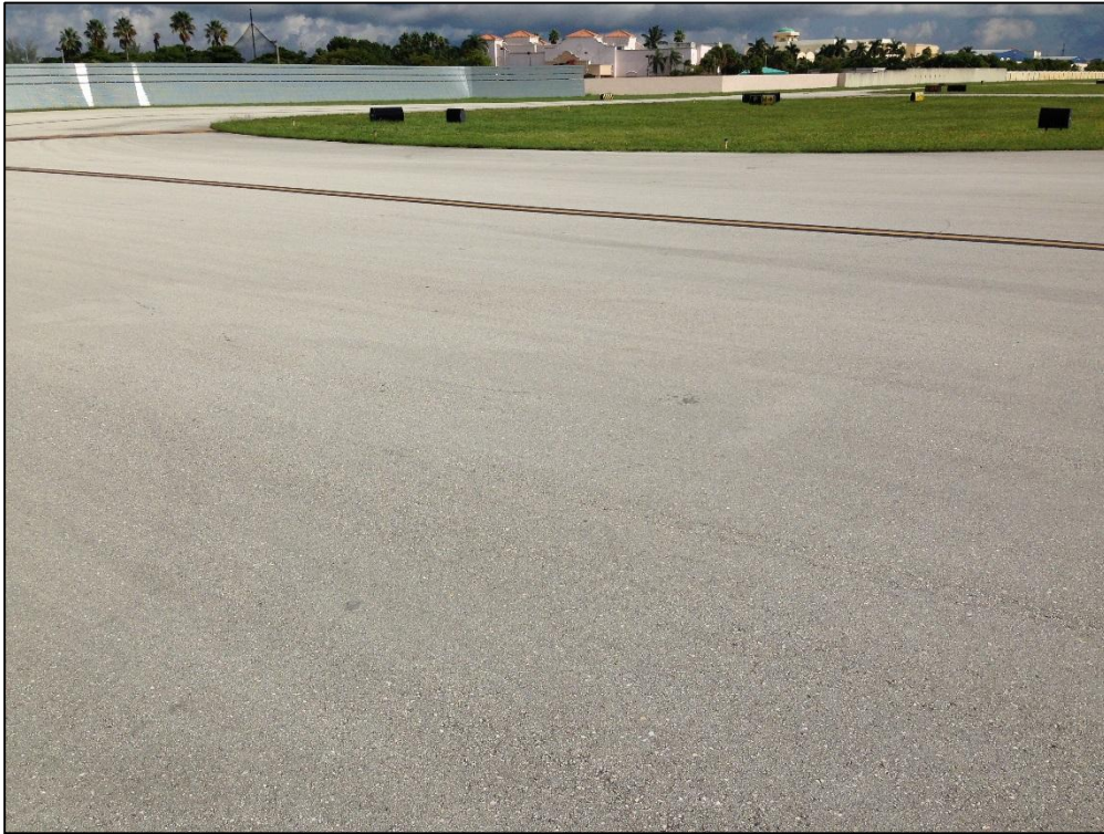
Taxiway Papa, Section 112, Sample Unit 100 – Low Severity (57) Weathering
