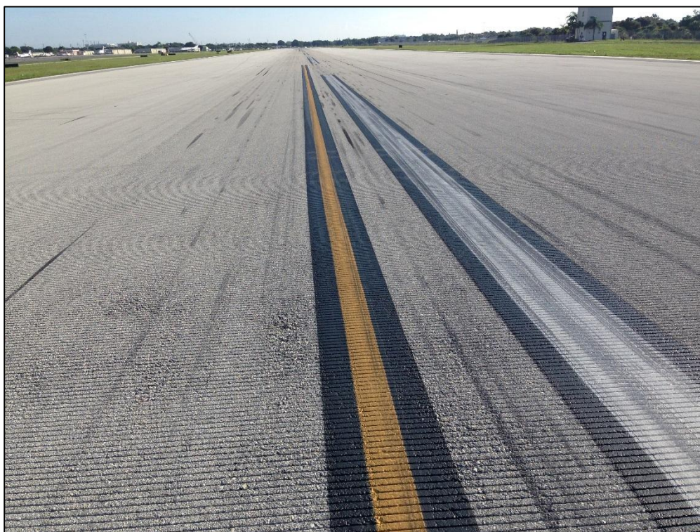
Runway 5-23, Section 6105, Sample Unit 350 – Low Severity (52) Raveling, Low Severity (57) Weathering
