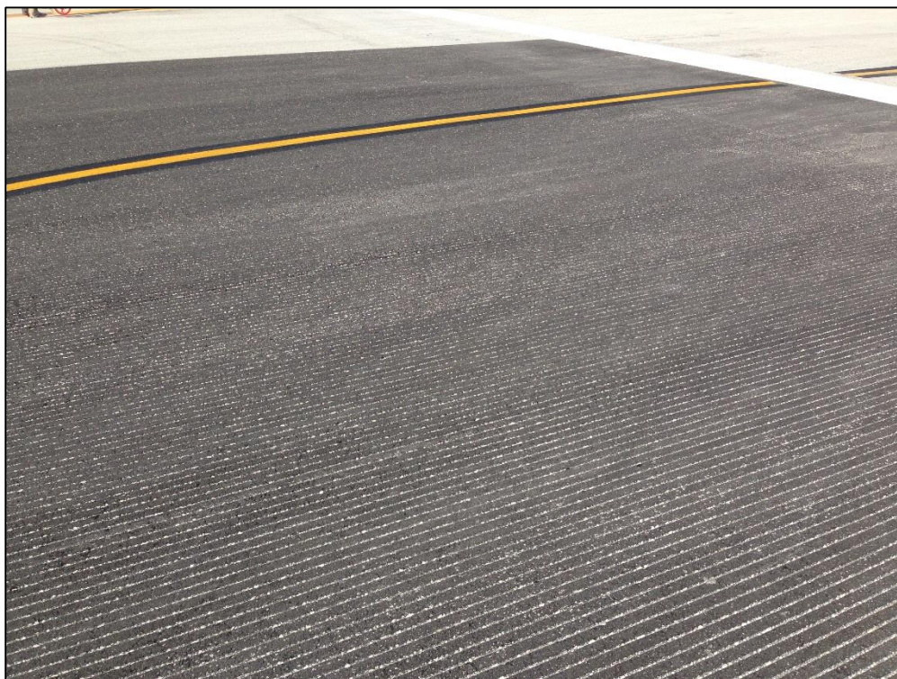
Runway 5-23, Section 6111, Sample Unit 84 – Low Severity (50) Patching, Low Severity (57) Weathering
