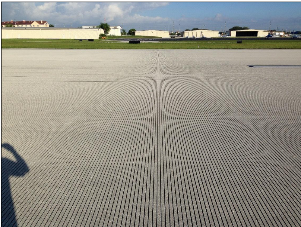
Runway 5-23, Section 6105, Sample Unit 357 – Low Severity (57) Weathering
