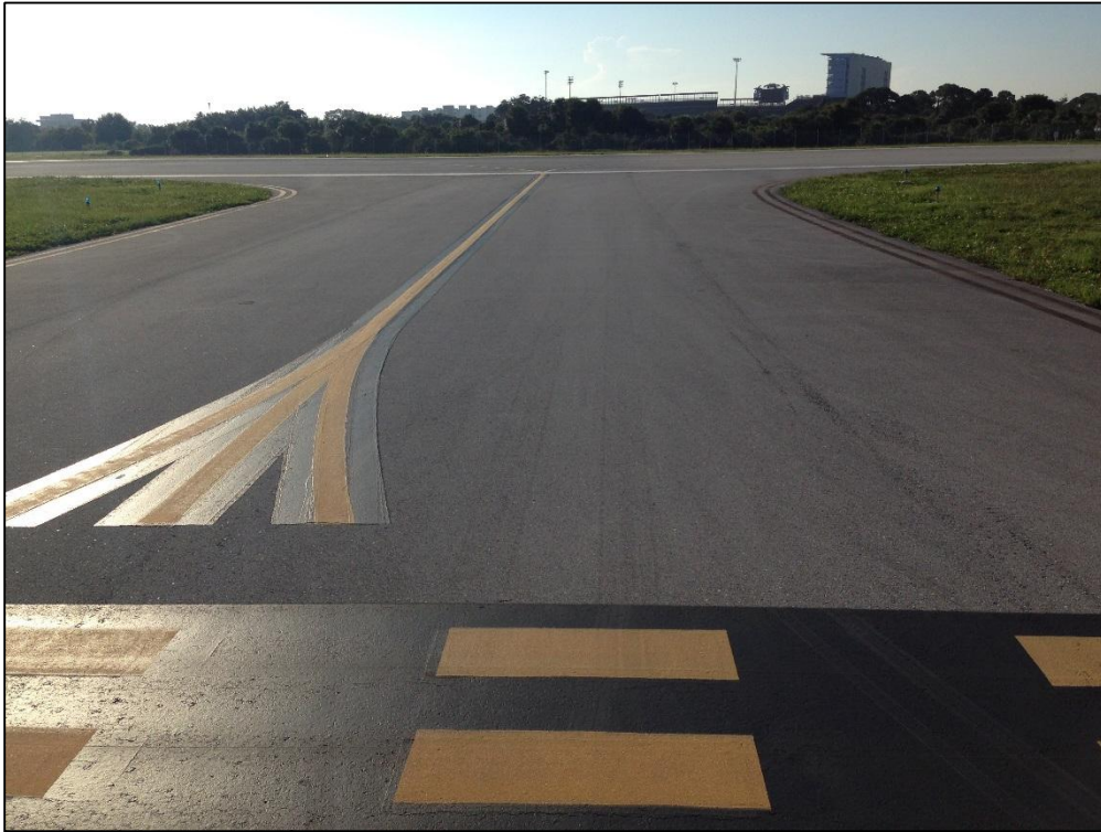
Taxiway Charlie, Section 120, Sample Unit 300 – Low Severity (57) Weathering
