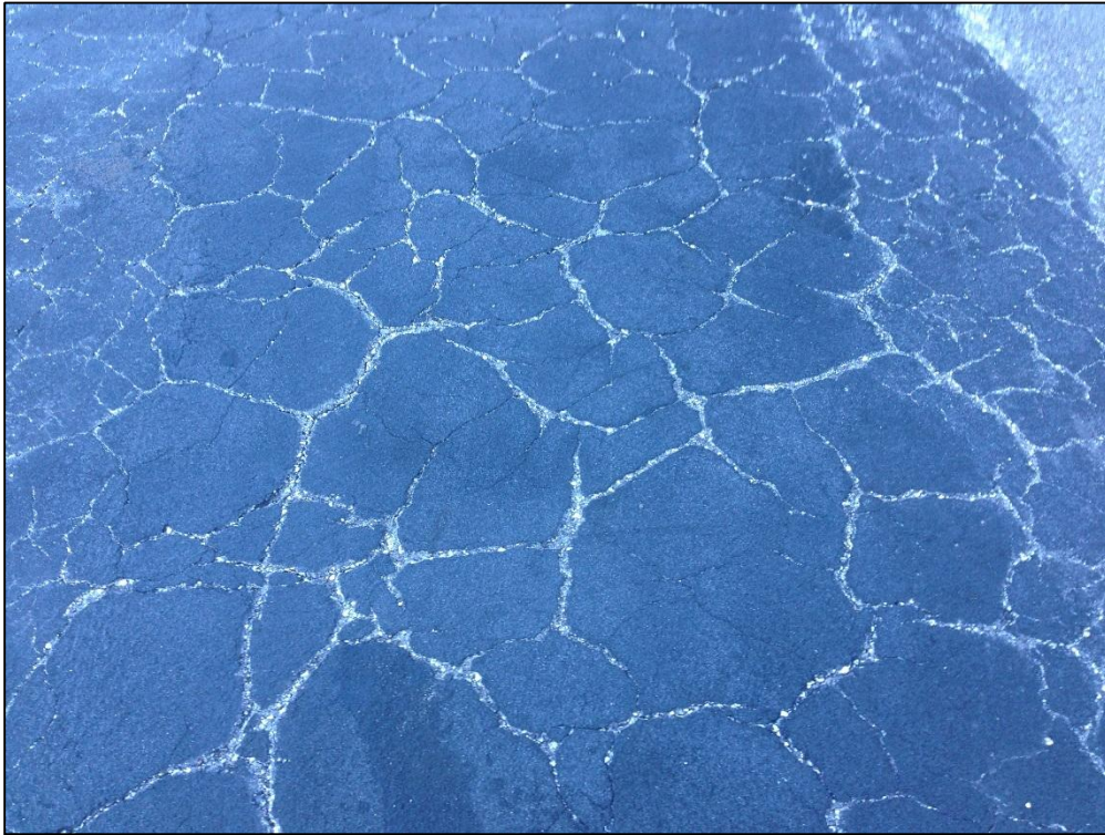
Apron North, Section 4505, Sample Unit 400 – Low Severity (43) Block Cracking, Low Severity (52) Raveling
