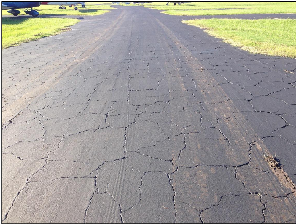
Apron Center, Section 4410, Sample Unit 304 – Low Severity (43) Block Cracking, Low Severity (57) Weathering
