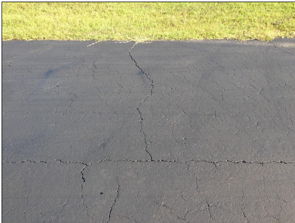
Taxiway Alpha, Section 130, Sample Unit 101 – Low Severity (43) Block Cracking, Low Severity (57) Weathering
