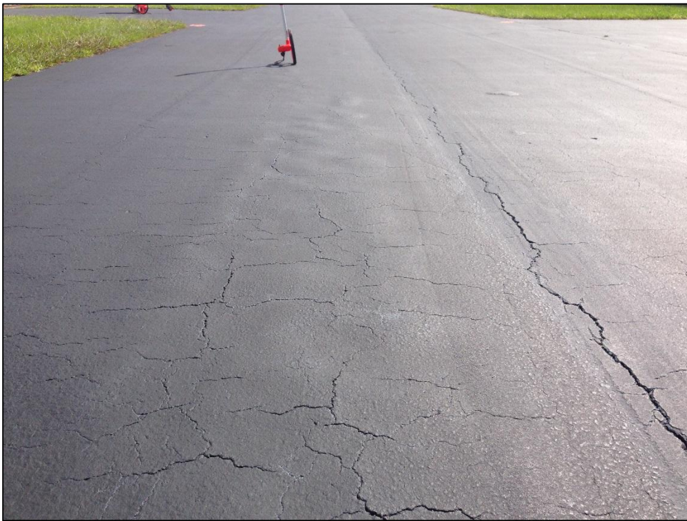
Apron T-Hangar 3, Section 4205, Sample Unit 101 – Low Severity (48) Longitudinal and Transverse Cracking, Low Severity (56) Swelling, Medium Severity (57) Weathering
