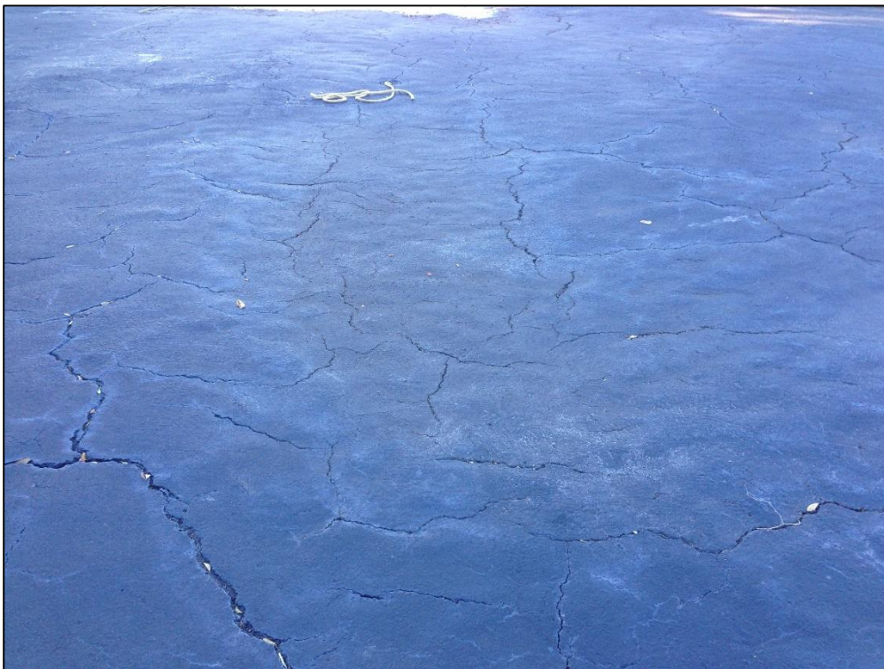
Apron Center, Section 4405, Sample Unit 501 – Low Severity (43) Block Cracking, Low Severity (48) Longitudinal and Transverse Cracking, Medium Severity (48) Longitudinal and Transverse Cracking, Low Severity (57) Weathering
