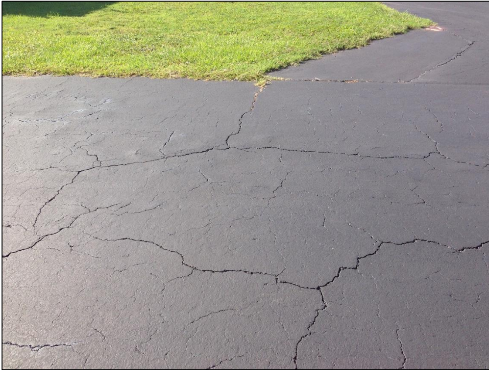
Apron T-Hangar 1, Section 4305, Sample Unit 600 – Low Severity (43) Block Cracking, Low Severity (48) Longitudinal and Transverse Cracking, Medium Severity (57) Weathering
