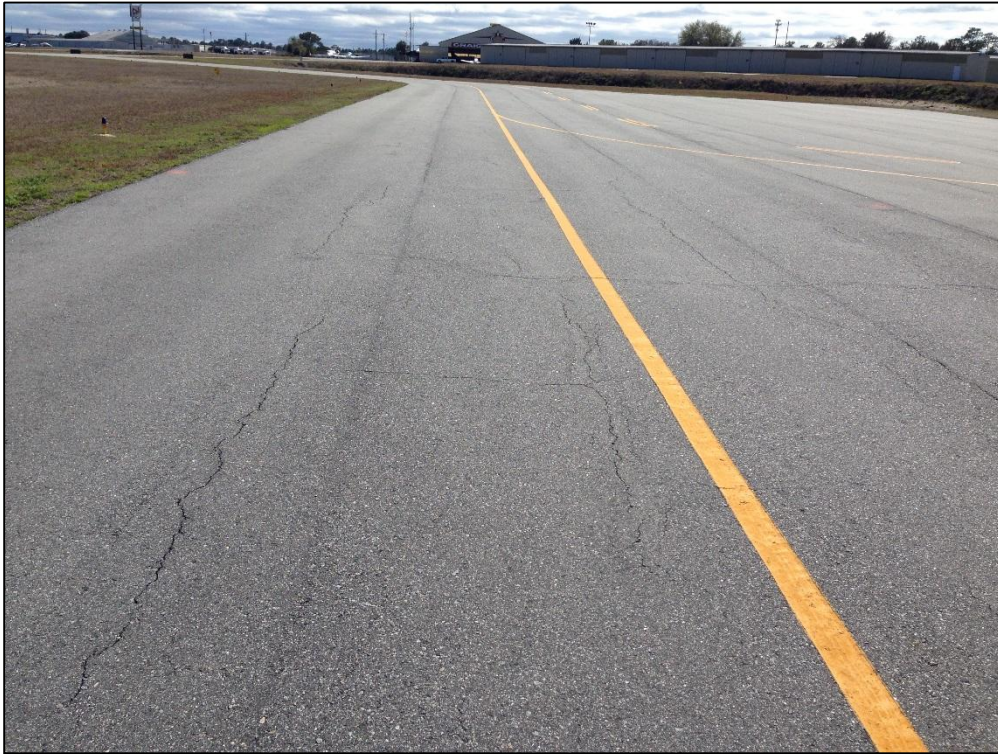
Taxiway Alpha, Section 105, Sample Unit 161 – Low Severity (48) Longitudinal and Transverse Cracking, Low Severity (52) Raveling, Low Severity (56) Swelling
