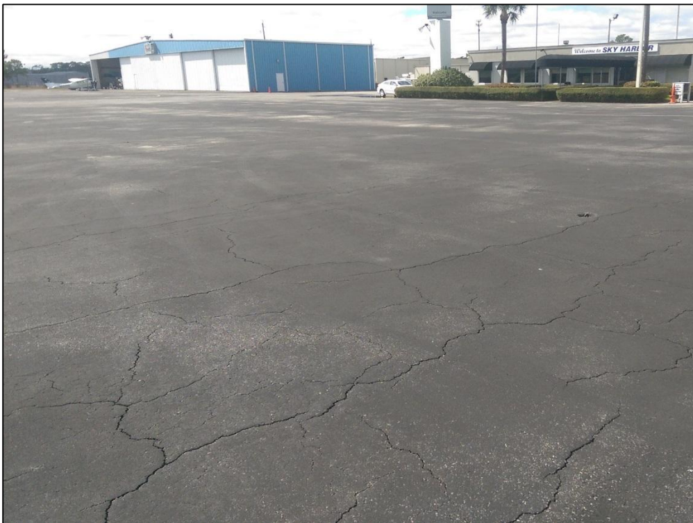
Apron South, Section 4105, Sample Unit 404 – Low Severity (43) Block Cracking, Low Severity (52) Raveling, Low Severity (57) Weathering
