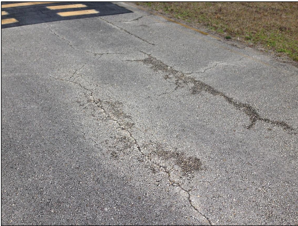
Taxiway Foxtrot, Section 605, Sample Unit 601 – Low Severity (48) Longitudinal and Transverse Cracking, Low Severity (52) Raveling, Medium Severity (52) Raveling
