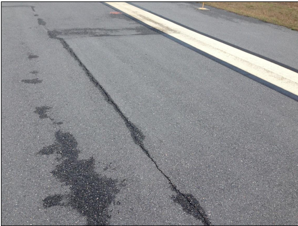
Runway 5-23, Section 6105, Sample Unit 168 – Low Severity (48) Longitudinal and Transverse Cracking, Low Severity (57) Weathering
