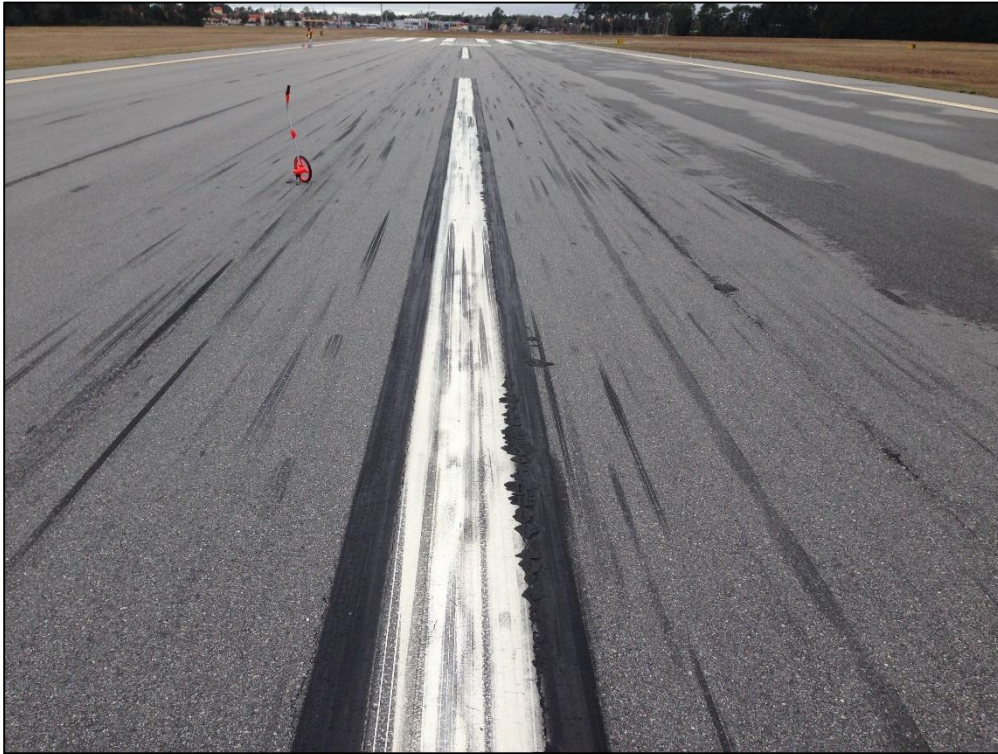
Runway 5-23, Section 6105, Sample Unit 112 – (42) Bleeding, Low Severity (48) Longitudinal and Transverse Cracking, Low Severity (57) Weathering
