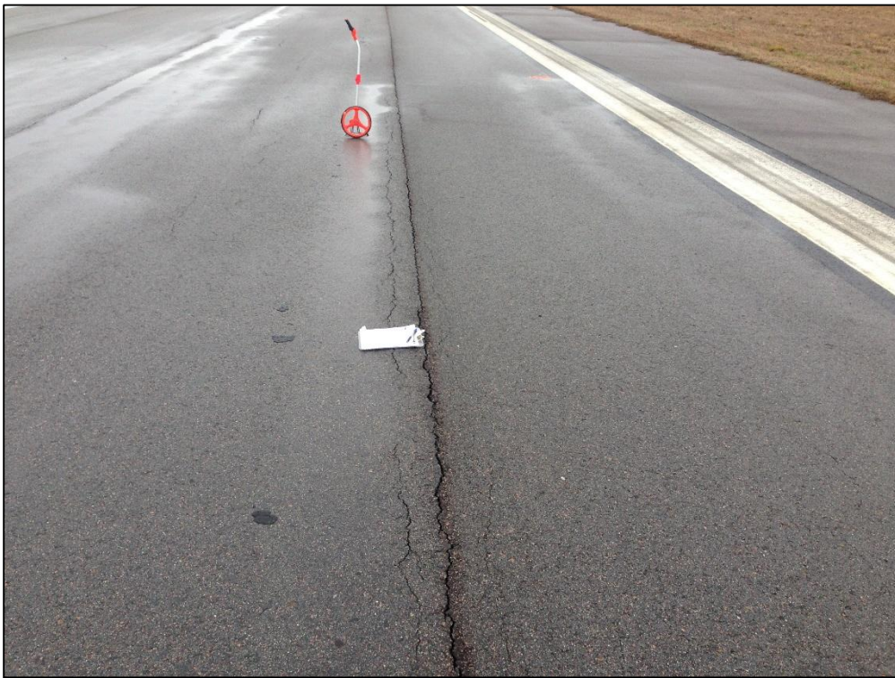
Runway 14-32, Section 6210, Sample Unit 174 – (42) Bleeding, Low and Medium Severity (48) Longitudinal and Transverse Cracking, Low Severity (52) Raveling, Low Severity (56) Swelling, Low Severity (57) Weathering
