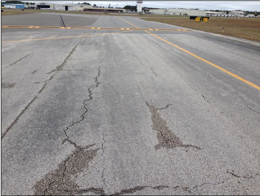
Taxiway Charlie, Section 305, Sample Unit 304 – Low Severity (48) Longitudinal and Transverse Cracking, Low Severity (52) Raveling, Low Severity (56) Swelling
