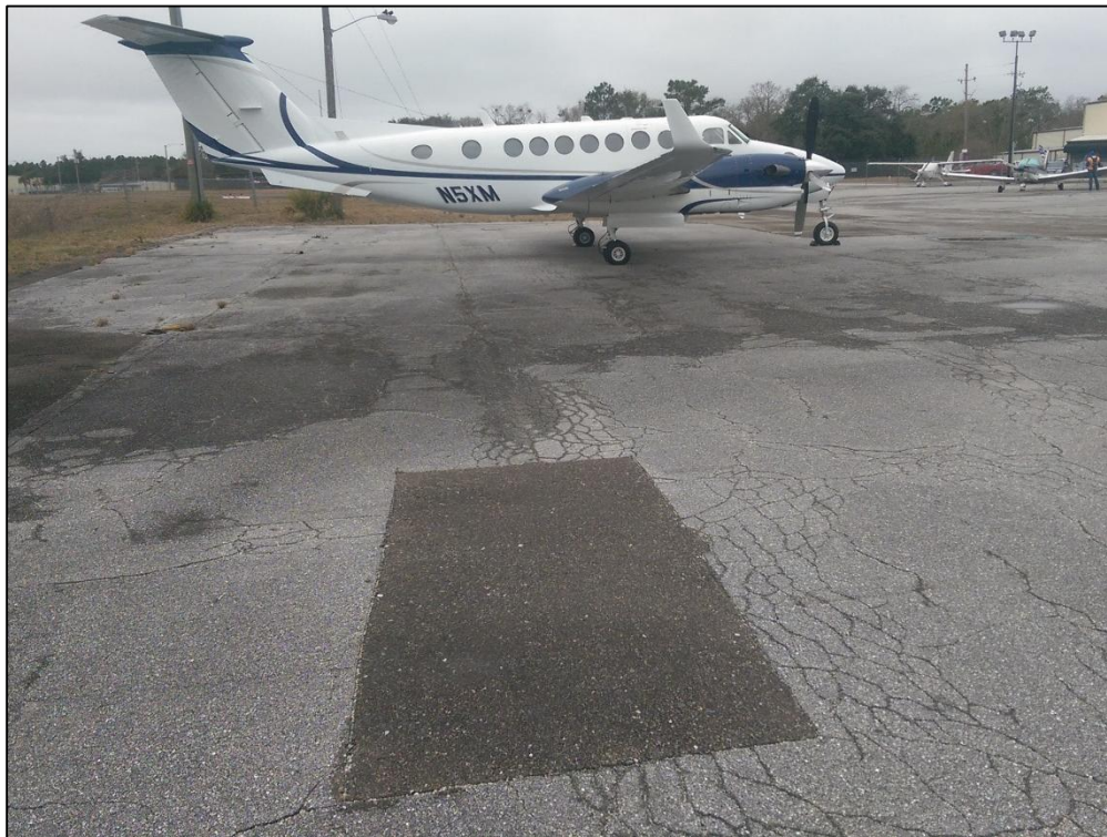
Apron Northwest, Section 4315, Sample Unit 103 – Medium Severity (41) Alligator Cracking, Low Severity (43) Block Cracking, Medium Severity (45) Depression, Medium Severity (50) Patching, Low Severity (52) Raveling, Medium Severity (57) Weathering
