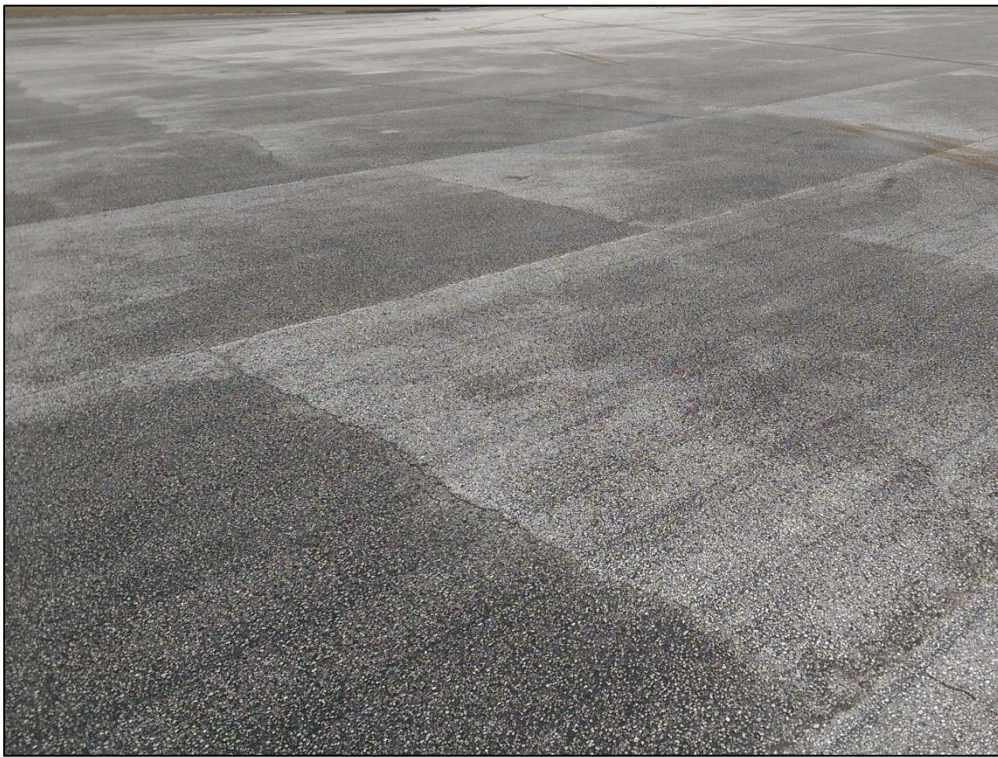
Apron Northwest, Section 4310, Sample Unit 251 – Low Severity (43) Block Cracking, Low Severity (52) Raveling, Medium Severity (57) Weathering
