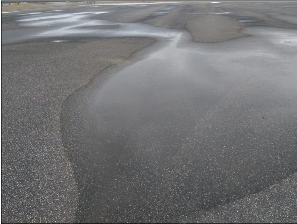
Apron FAA, Section 4510, Sample Unit 603 – Low Severity (45) Depression, Low Severity (57) Weathering
