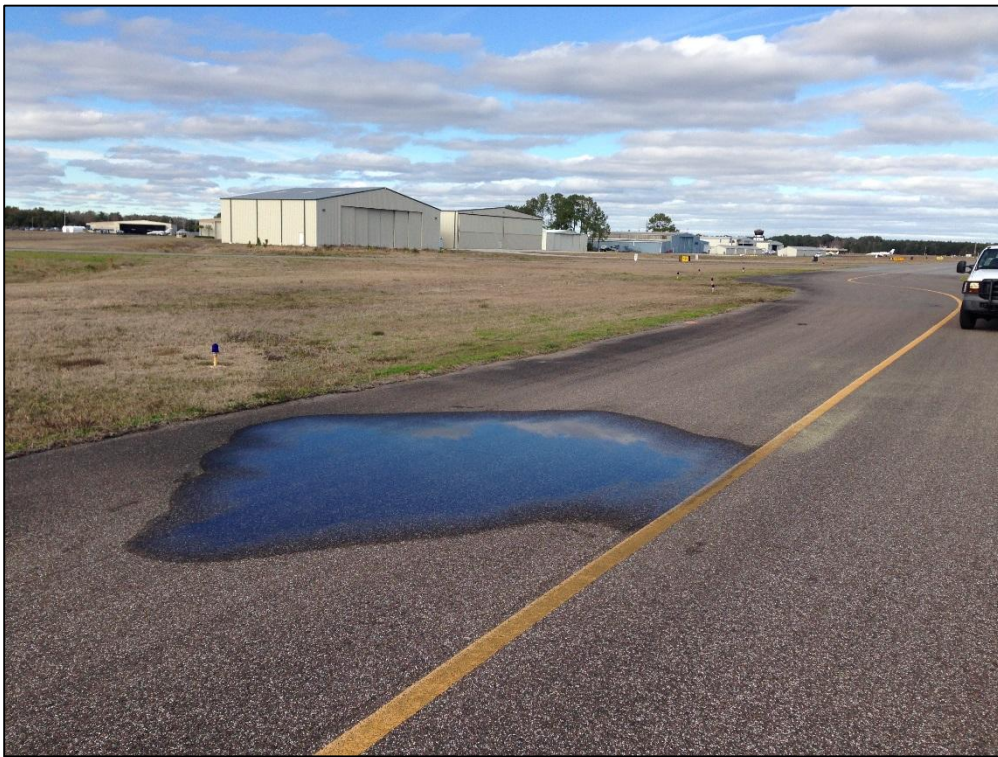
Taxiway Bravo, Section 235, Sample Unit 127 – Low Severity (45) Depression, Low Severity (52) Raveling, Low Severity (57) Weathering
