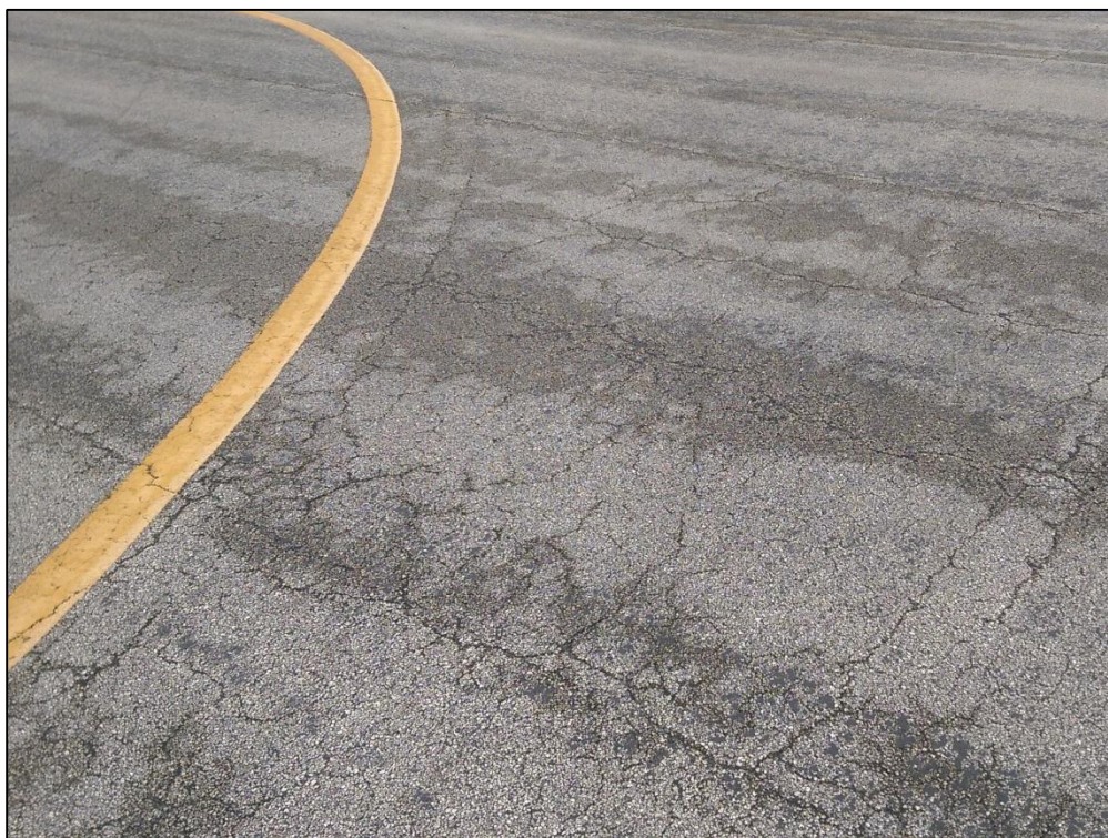
Apron North, Section 4210, Sample Unit 406 – Low Severity (43) Block Cracking, Low Severity (56) Swelling, Low Severity (57) Weathering
