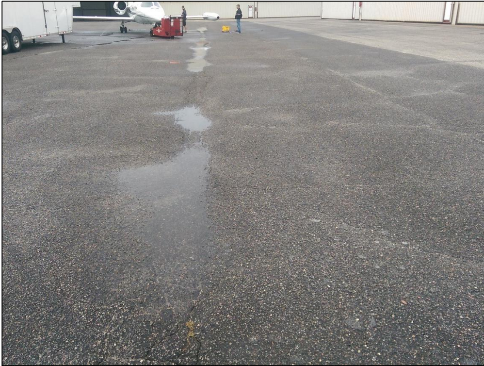
Apron Northwest, Section 4310, Sample Unit 554 – Low Severity (43) Block Cracking, Low Severity (45) Depression, Low Severity (52) Raveling, Medium Severity (57) Weathering
