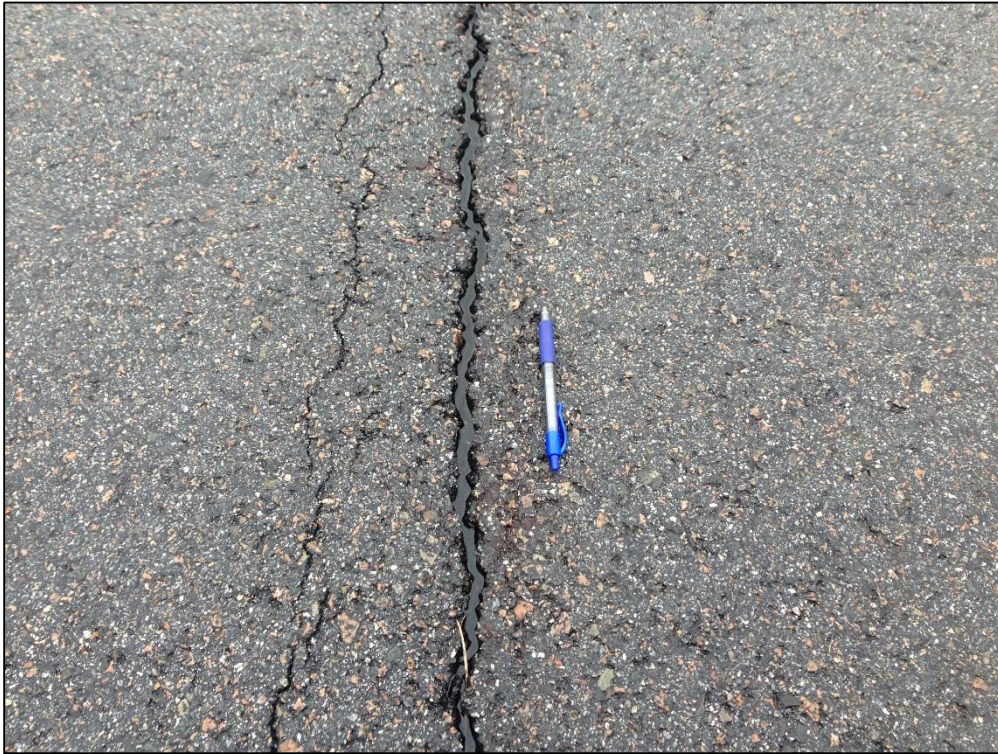
Runway 14-32, Section 6210, Sample Unit 163 – Low and Medium Severity (48) Longitudinal and Transverse Cracking, Low Severity (57) Weathering
