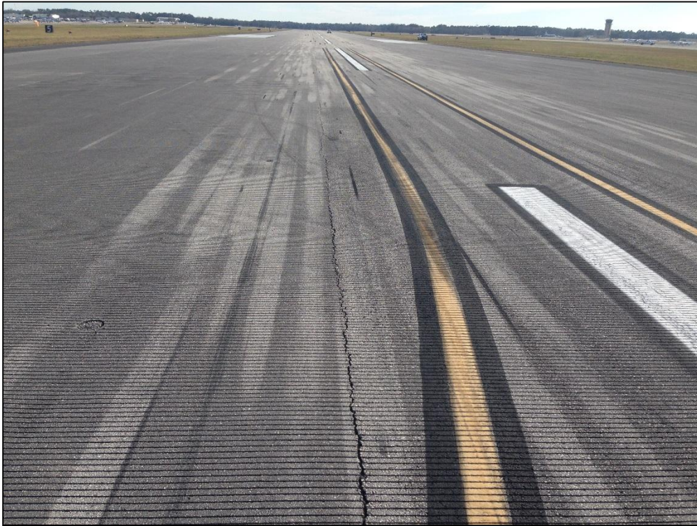
Runway 16-34, Section 6215, Sample Unit 407 – Low and Medium Severity (48) Longitudinal and Transverse Cracking, Low Severity (52) Raveling, Low Severity (57) Weathering
