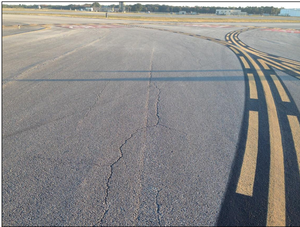
Taxiway N6, Section 1460, Sample Unit 610 – Low and Medium Severity (48) Longitudinal and Transverse Cracking, Low Severity (52) Raveling, Low Severity (56) Swelling
