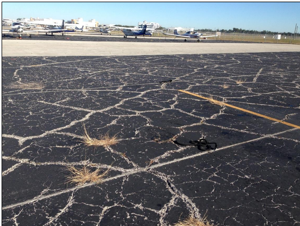
Nova Apron, Section 4305, Sample Unit 501 – Medium Severity (43) Block Cracking, Low Severity (52) Raveling
