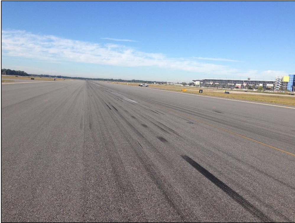
Runway 7L-25R, Section 6130, Sample Unit 385 – Low Severity (57) Weathering
