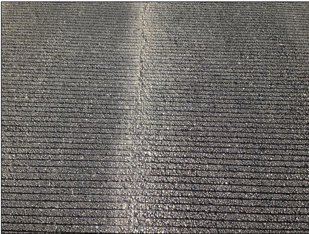
Runway 16-34, Section 6215, Sample Unit 344 – Low Severity (48) Longitudinal and Transverse Cracking, Low Severity (52) Raveling, Medium Severity (52) Raveling
