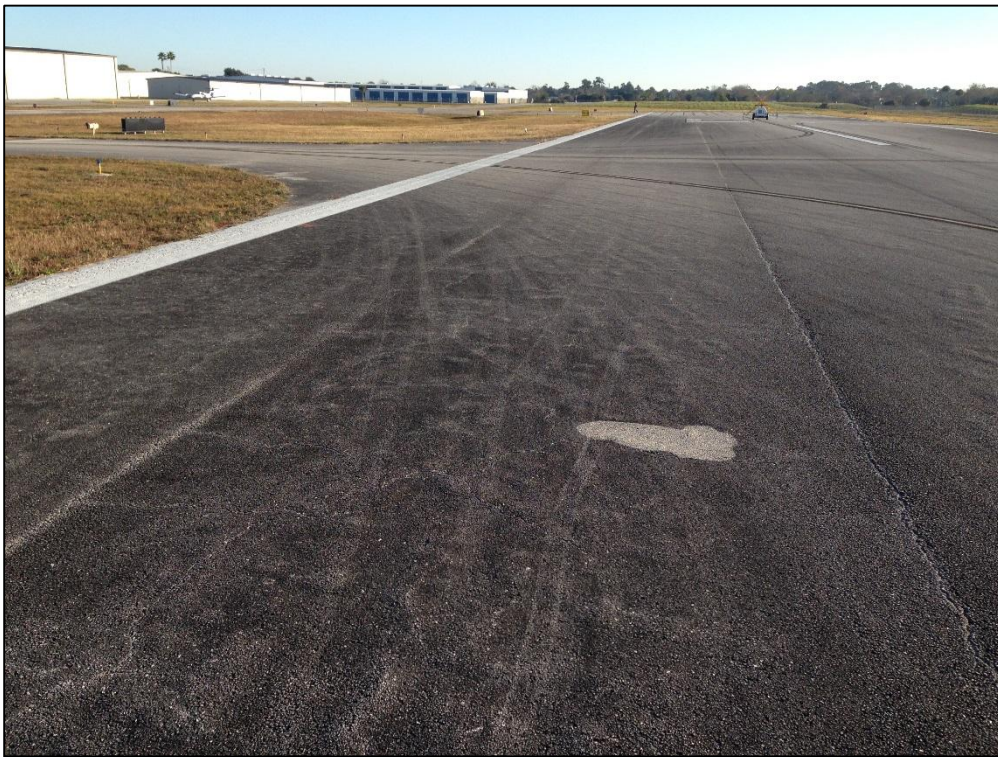
Runway 7R-25L, Section 6305, Sample Unit 151 – Low and Medium Severity (48) Longitudinal and Transverse Cracking, Low Severity (52) Raveling, Low Severity (56) Swelling
