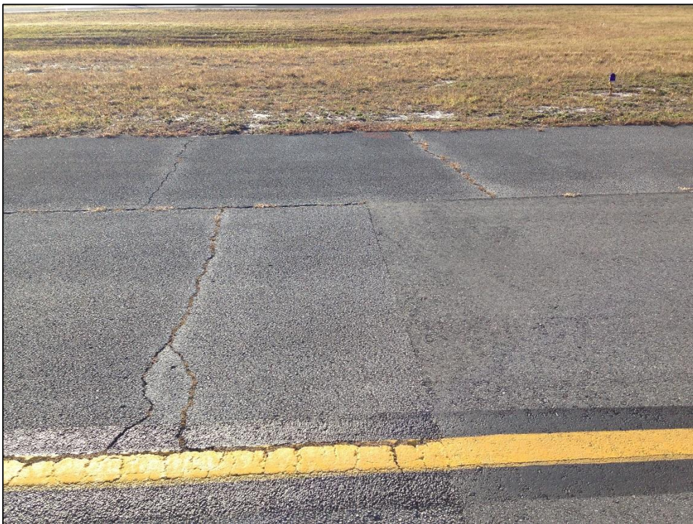
Taxiway Sierra, Section 1932, Sample Unit 205 – Medium Severity (43) Block Cracking, Low Severity (50) Patching, Low Severity (52) Raveling
