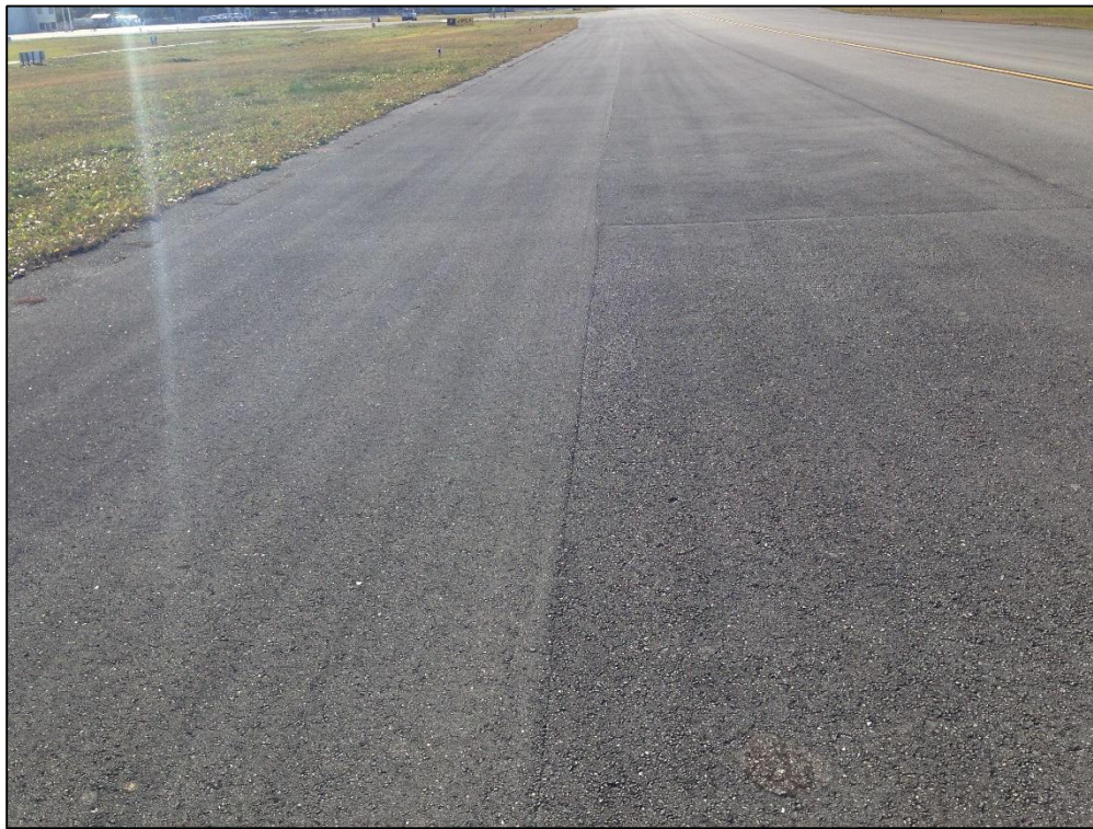
Taxiway Papa, Section 805, Sample Unit 180 – Low Severity (57) Weathering
