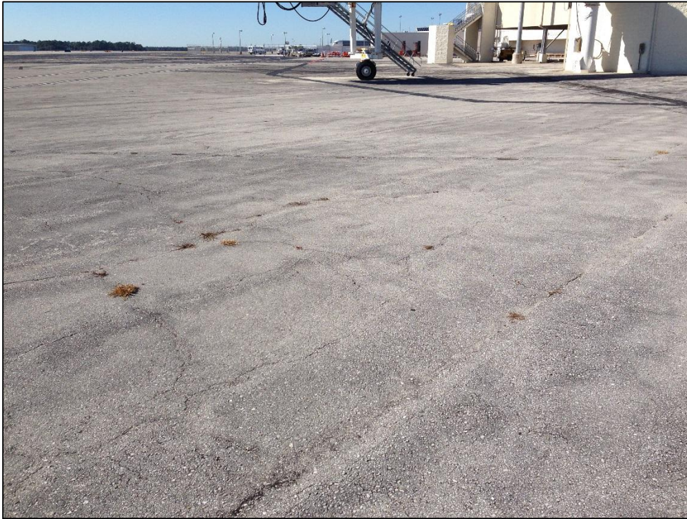
Apron NE, Section 4240, Sample Unit 557 – Low Severity (43) Block Cracking, Low Severity (52) Raveling, Low Severity (56) Swelling, Medium Severity (56) Swelling
