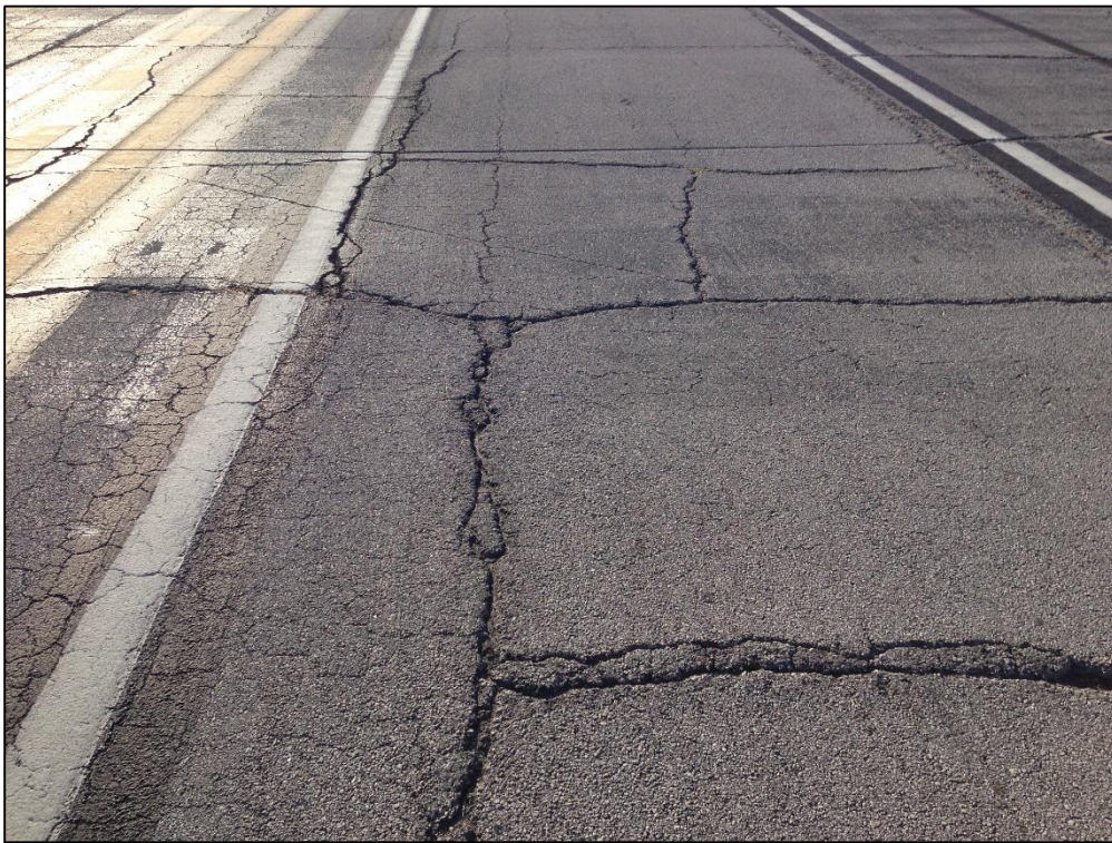
Apron NE, Section 4220, Sample Unit 159 – Medium Severity (43) Block Cracking, High Severity (43) Block Cracking, High Severity (47) Joint Reflection Cracking, Low Severity (52) Raveling
