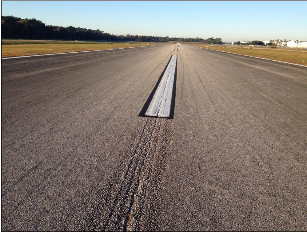
Runway 7R-25L, Section 6305, Sample Unit 130 – Low and Medium Severity (48) Longitudinal and Transverse Cracking, Low Severity (52) Raveling, High Severity (52) Raveling, Low Severity (56) Swelling
