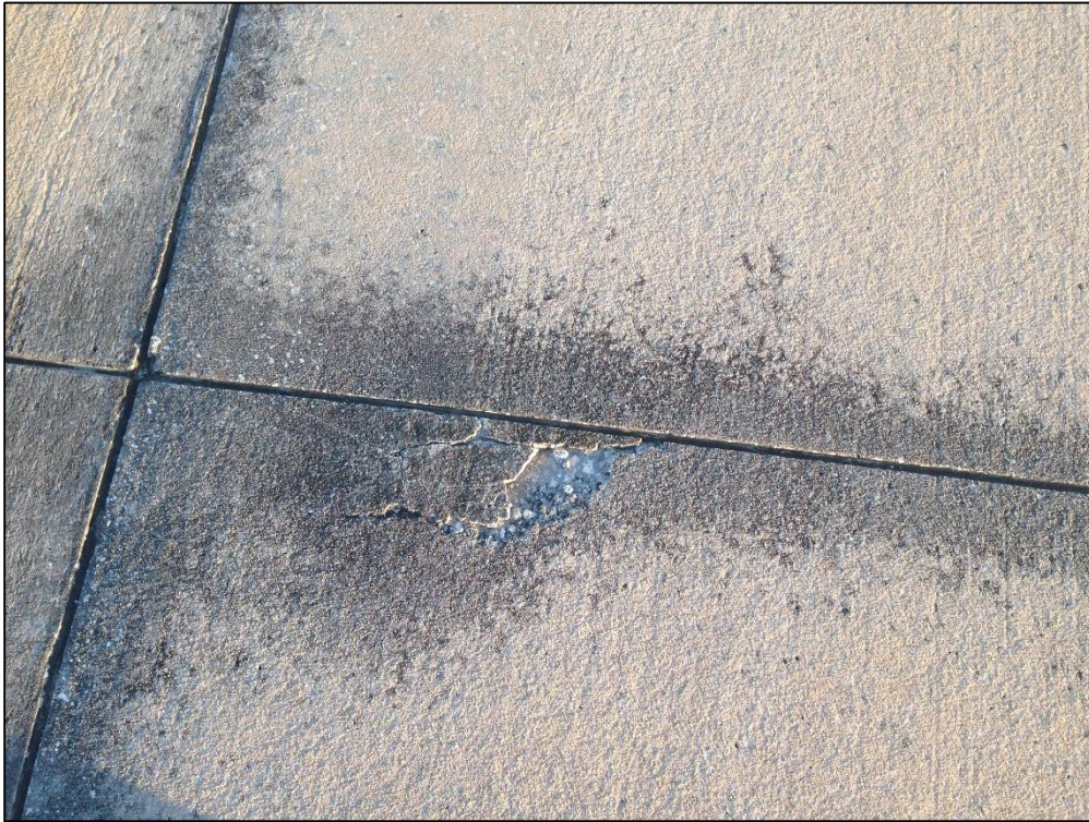
Terminal Apron, Section 4105, Sample Unit 102 – Medium Severity (74) Joint Spalling
