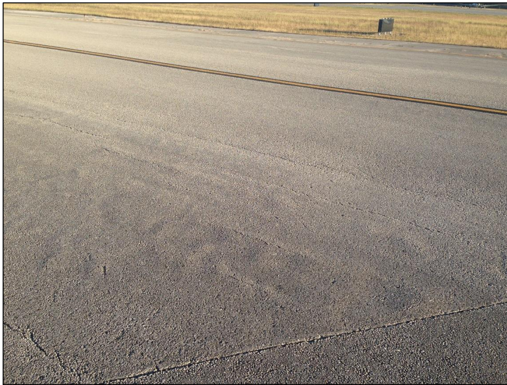
Taxiway November, Section 1408, Sample Unit 242 – Low Severity (48) Longitudinal and Transverse Cracking, Medium Severity (52) Raveling, Low Severity (56) Swelling
