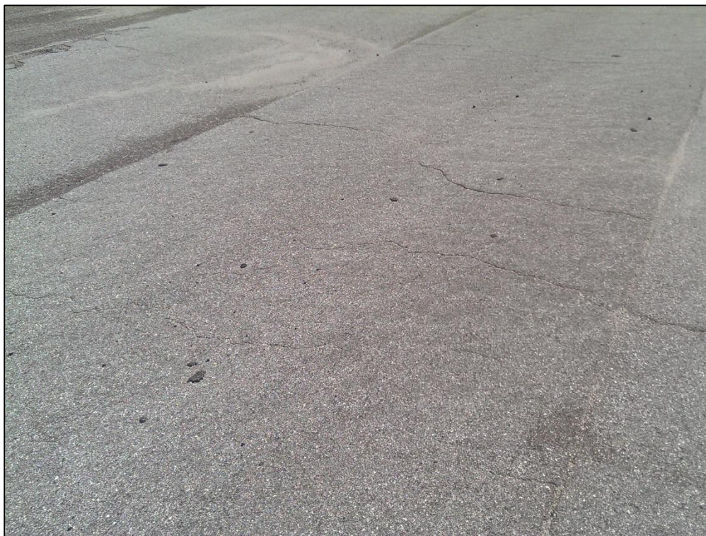
West Ramp, Section 162, Sample Unit 226 – Low Severity (43) Block Cracking, Low Severity (52) Raveling
