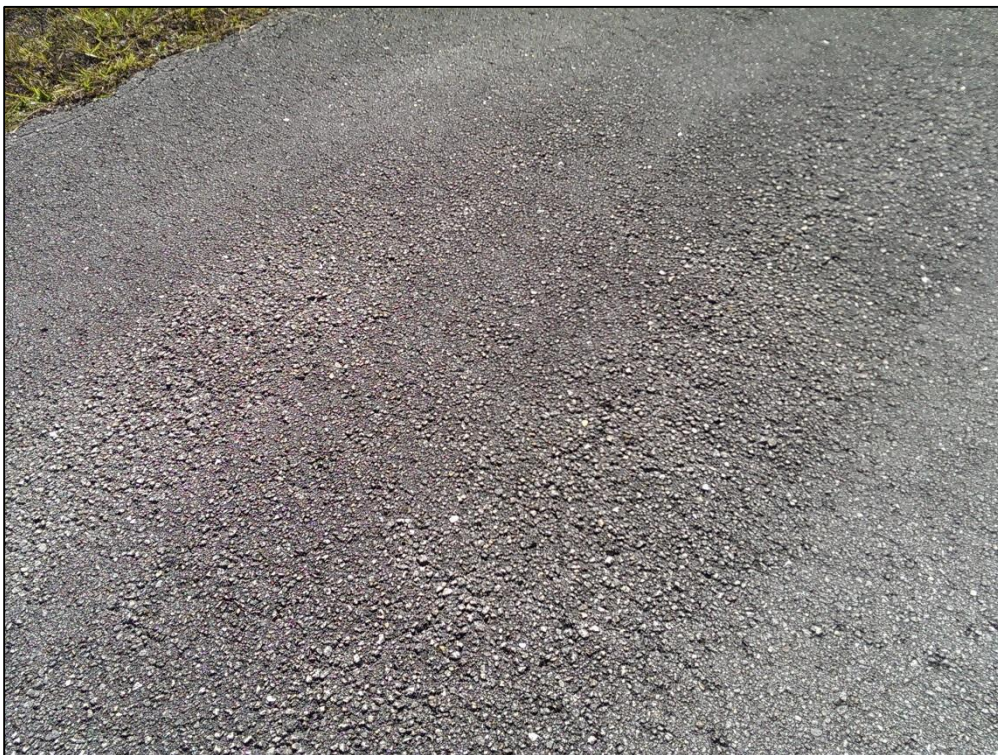
Apron South, Section 5305, Sample Unit 301 – Low Severity (52) Raveling, Low Severity (57) Weathering
