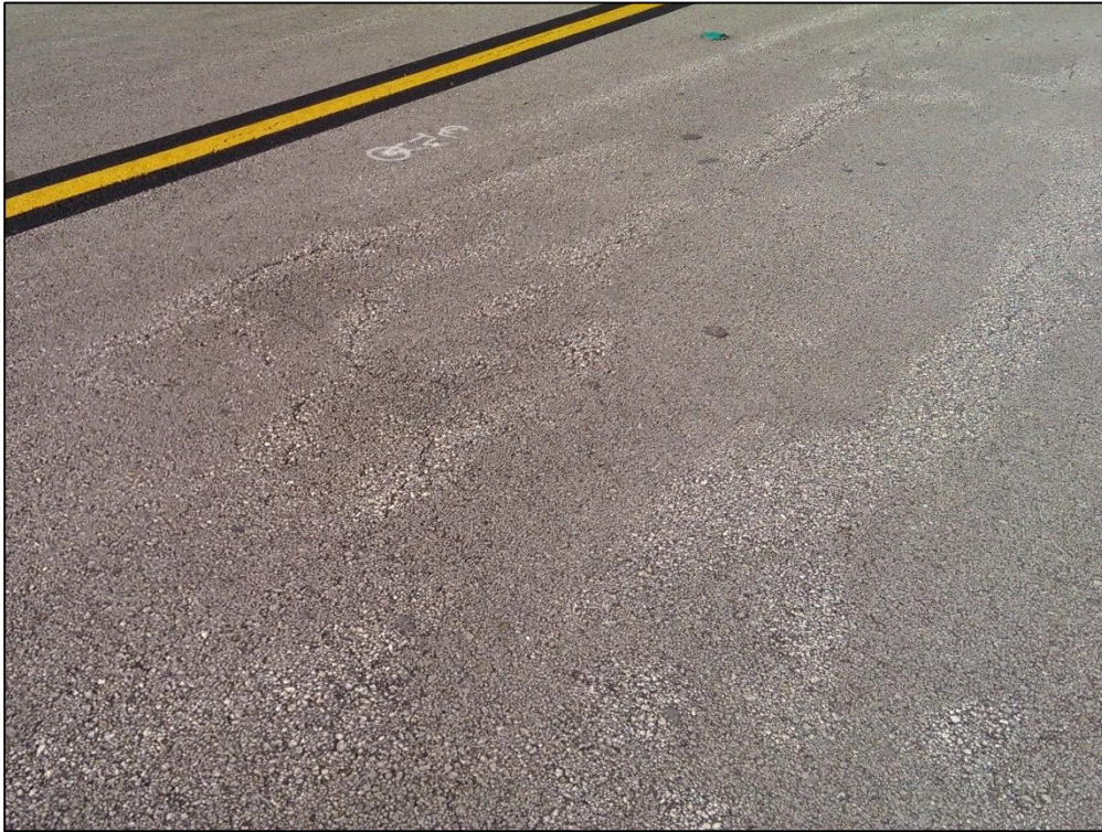
Taxiway Bravo, Section 220, Sample Unit 219 – Low Severity (48) Longitudinal and Transverse Cracking, Low Severity (52) Raveling, Low Severity (57) Weathering
