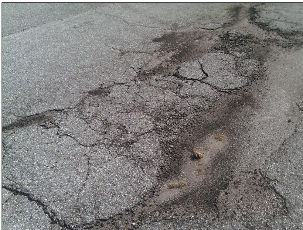
West Ramp, Section 160, Sample Unit 123 – Low Severity (43) Block Cracking, Low Severity (45) Depression, Low Severity (52) Raveling, Medium Severity (52) Raveling
