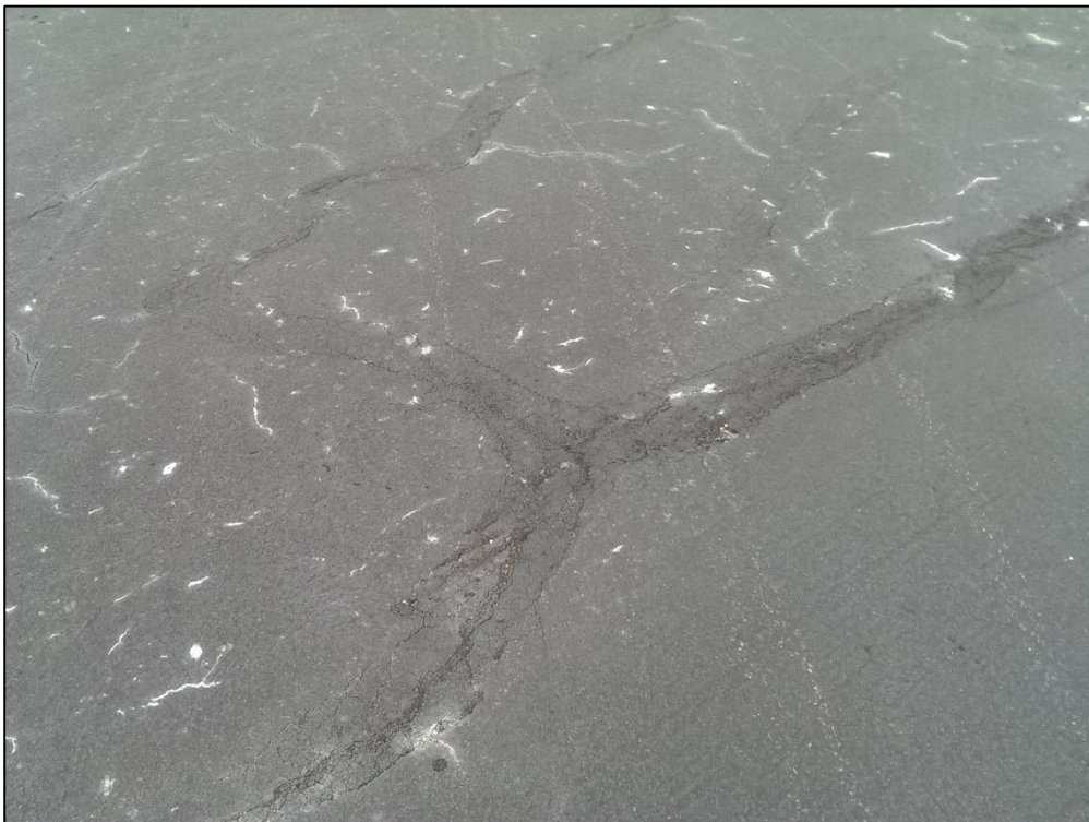
Apron SE, Section 4112, Sample Unit 250 – Low Severity (48) Longitudinal and Transverse Cracking
