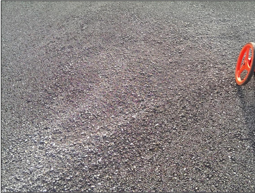
Taxiway Bravo, Section 205, Sample Unit 203 – Low Severity (52) Raveling, Medium Severity (52) Raveling
