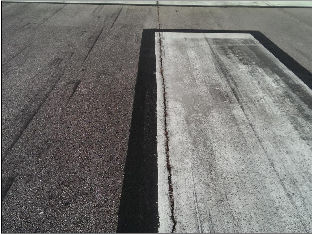
Runway 5-23, Section 6210, Sample Unit 108 – Low and Medium Severity (48) Longitudinal and Transverse Cracking, Low Severity (57) Weathering
