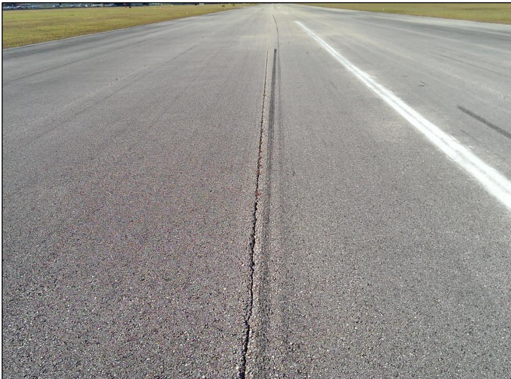
Runway 5-23, Section 6210, Sample Unit 156 – Low and Medium Severity (48) Longitudinal and Transverse Cracking, Low Severity (57) Weathering
