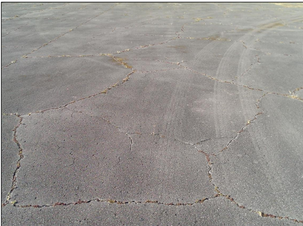
Apron East, Section 4210, Sample Unit 103 – Medium Severity (43) Block Cracking, Low Severity (57) Weathering
