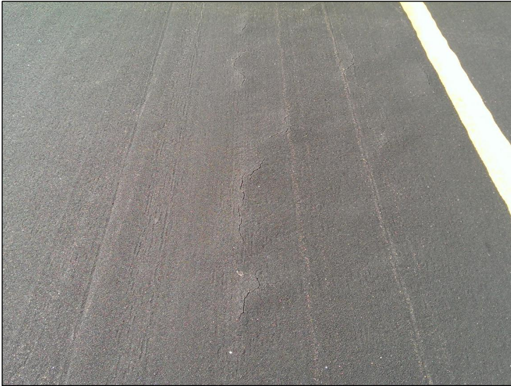
Taxiway Alpha, Section 110, Sample Unit 522 – Low Severity (48) Longitudinal and Transverse Cracking
