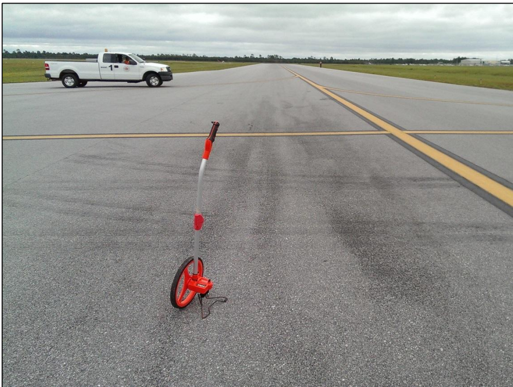
Taxiway Delta, Section 405, Sample Unit 266 – (42) Bleeding, Low Severity (57) Weathering
