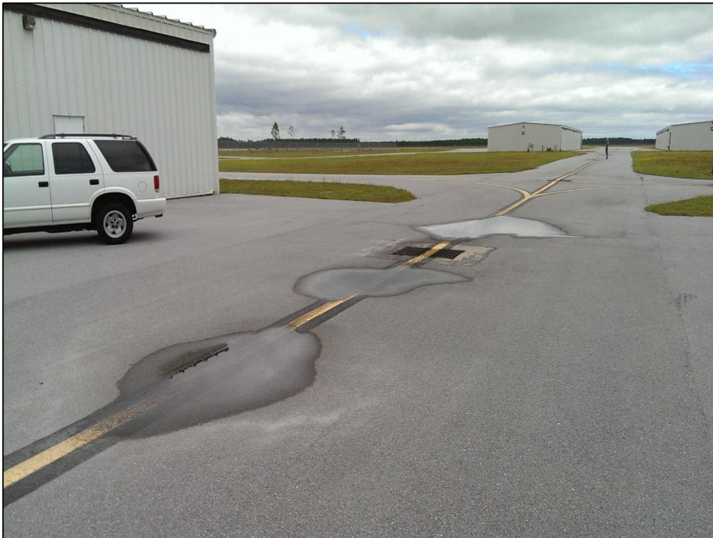
Apron T-Hangar, Section 4310, Sample Unit 304 – Low Severity (45) Depression, Low Severity (57) Weathering
