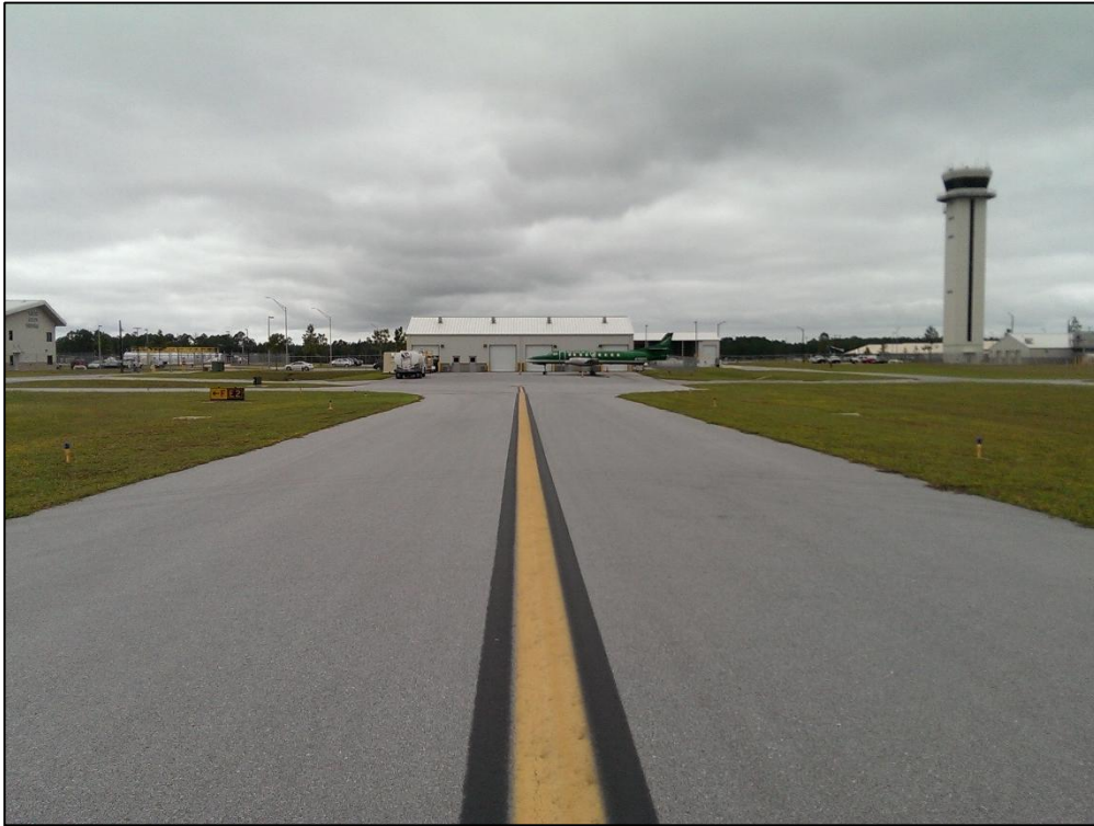
Taxiway E2, Section 505, Sample Unit 351 – Low Severity (57) Weathering
