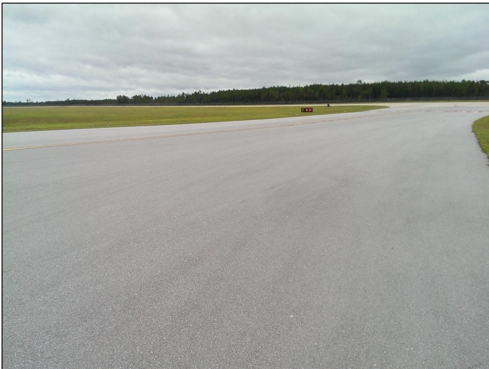
Taxiway Papa, Section 1610, Sample Unit 408 – Low Severity (57) Weathering
