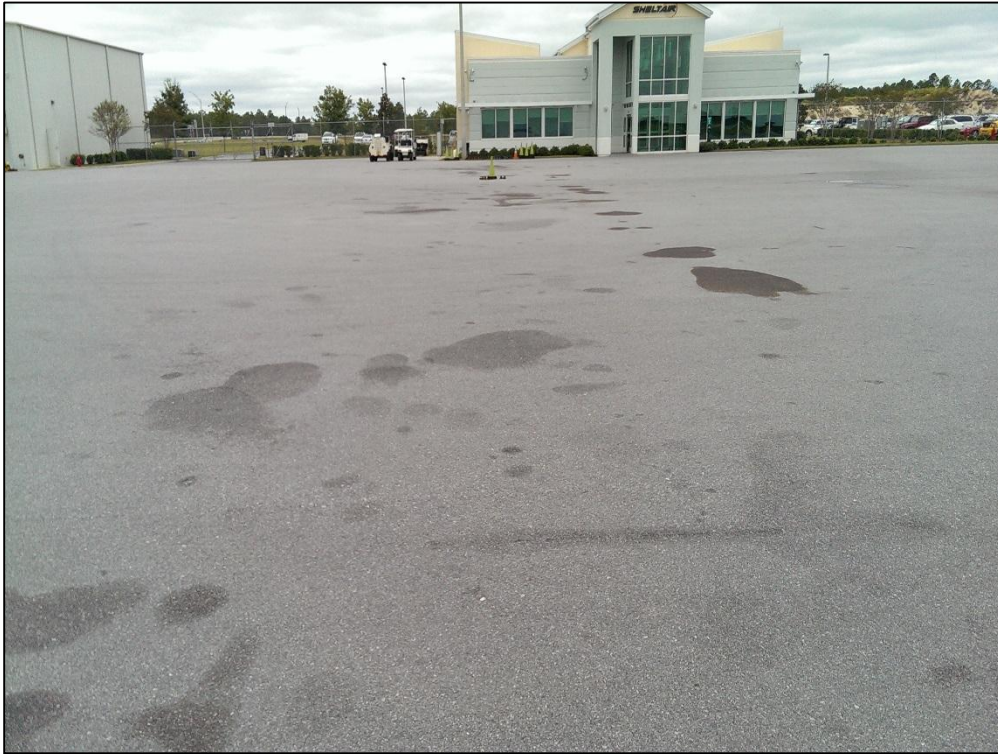
Apron GA, Section 4405, Sample Unit 251 – (49) Oil Spillage, Low Severity (57) Weathering
