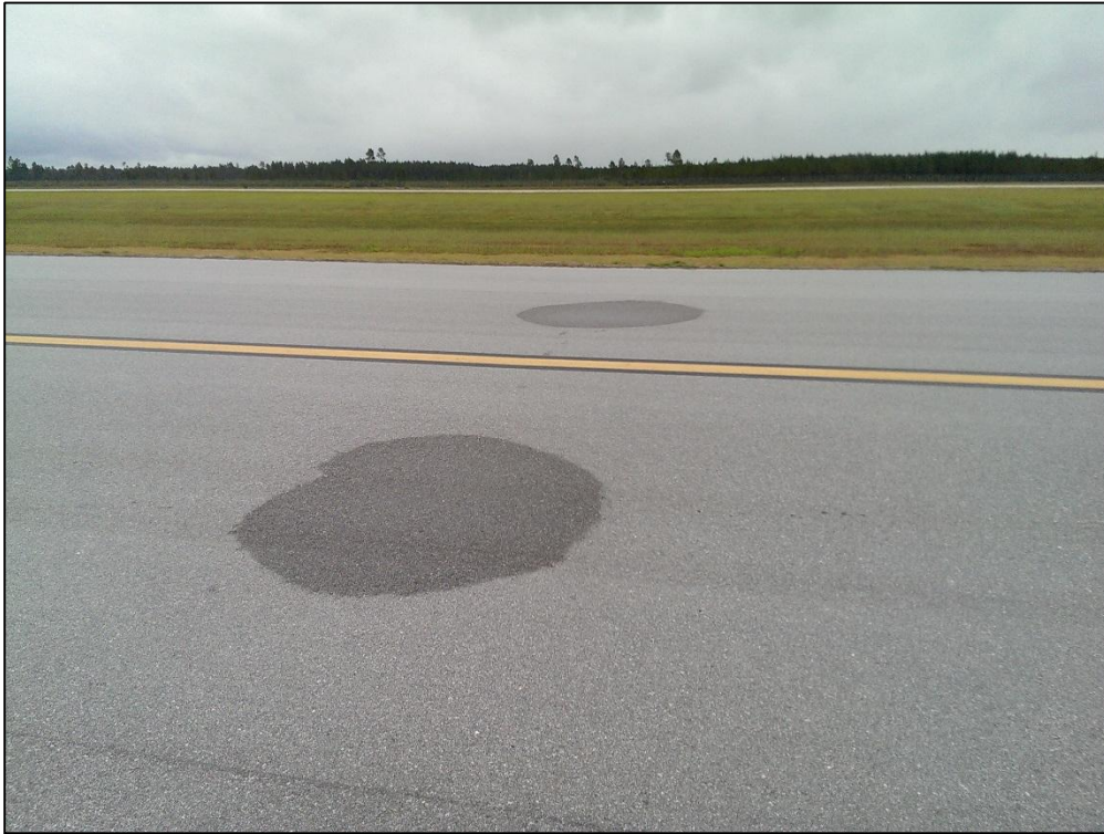
Taxiway Delta, Section 405, Sample Unit 159 – Low Severity (45) Depression, Low Severity (57) Weathering
