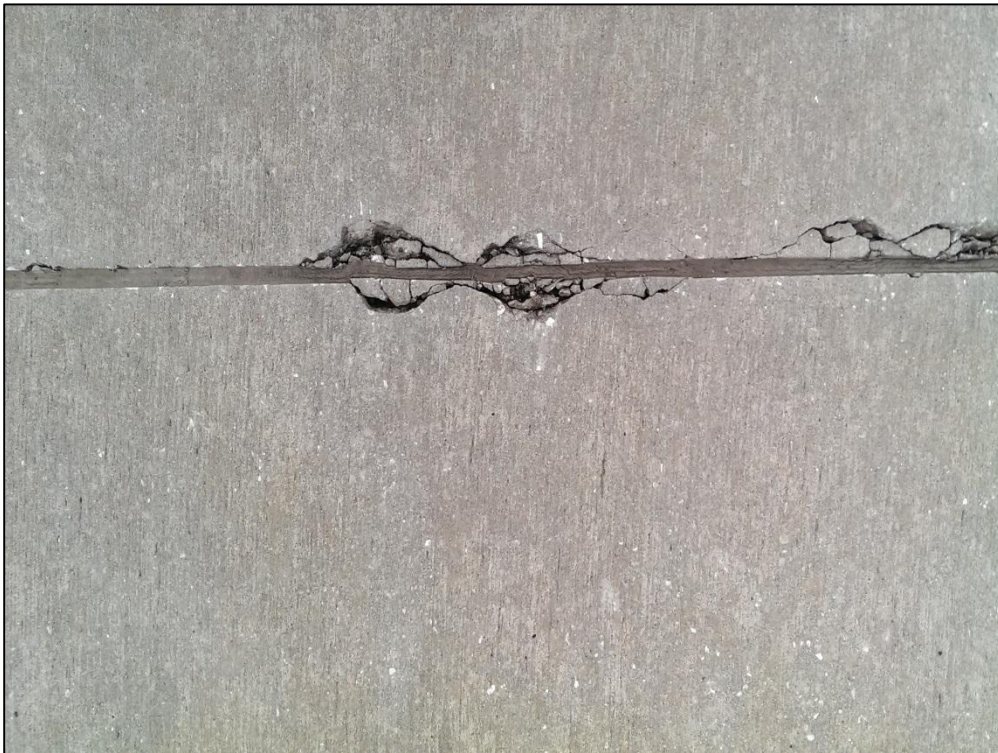
Taxiway Sierra, Section 1905, Sample Unit 300 – Low Severity (74) Joint Spalling
