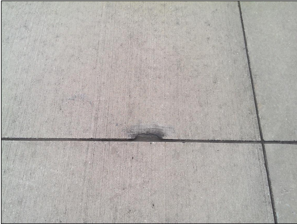
Taxiway Uniform, Section 2105, Sample Unit 100 – Low Severity (74) Joint Spalling
