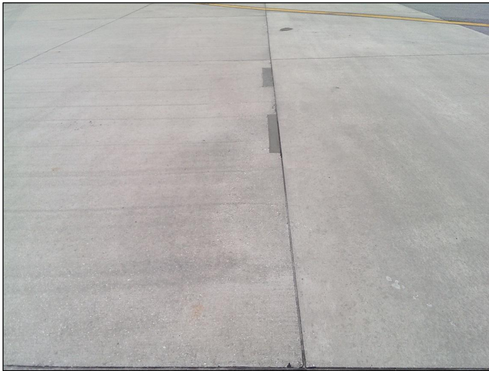
Terminal Apron, Section 4115, Sample Unit 950 – Low Severity (66) Small Patching
