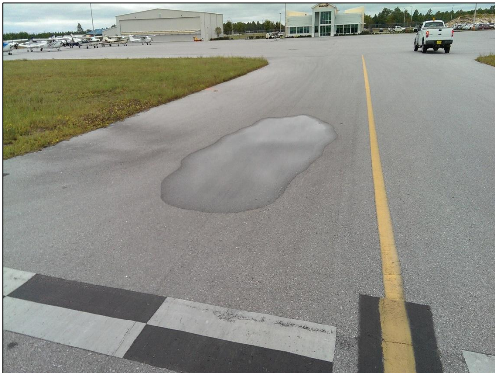
Taxiway Juliet, Section 1020, Sample Unit 754 – Medium Severity (45) Depression, Low Severity (57) Weathering
