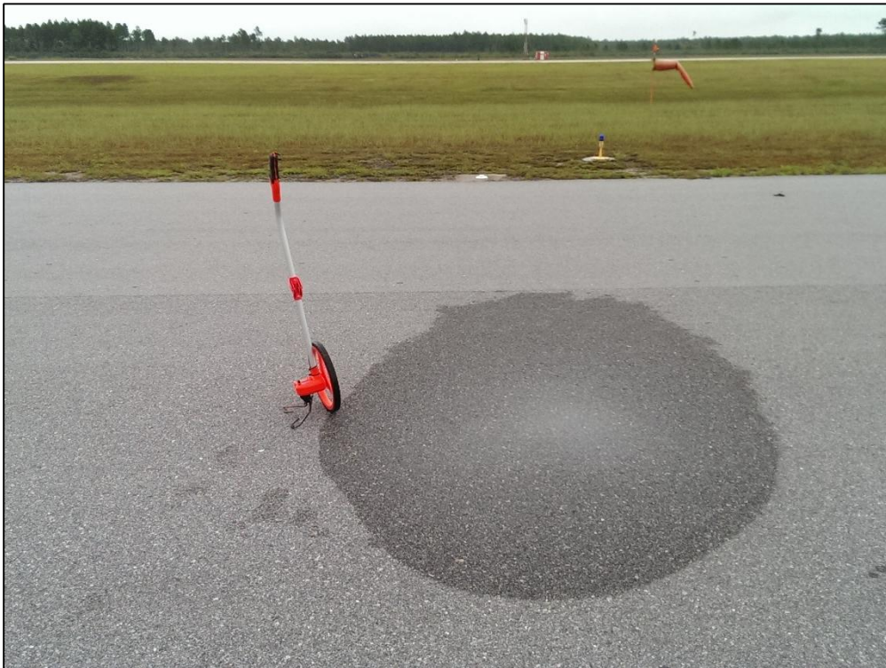
Taxiway Delta, Section 405, Sample Unit 129 – Low Severity (45) Depression, Low Severity (57) Weathering
