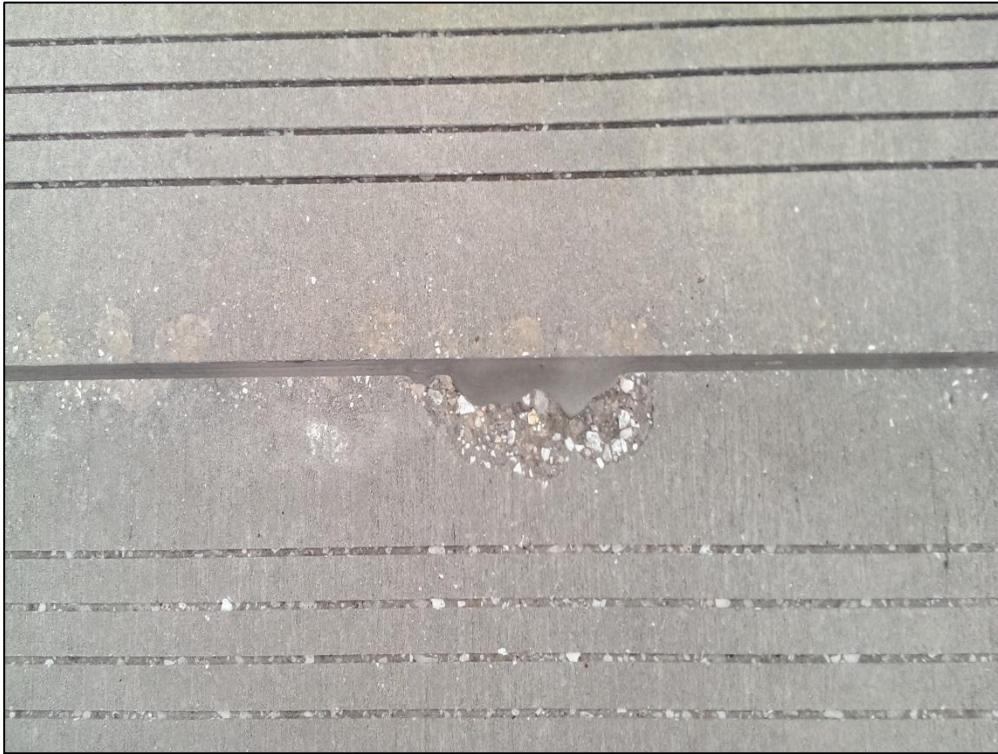
Runway 16-34, Section 6105, Sample Unit 379 – Low Severity (74) Joint Spalling
