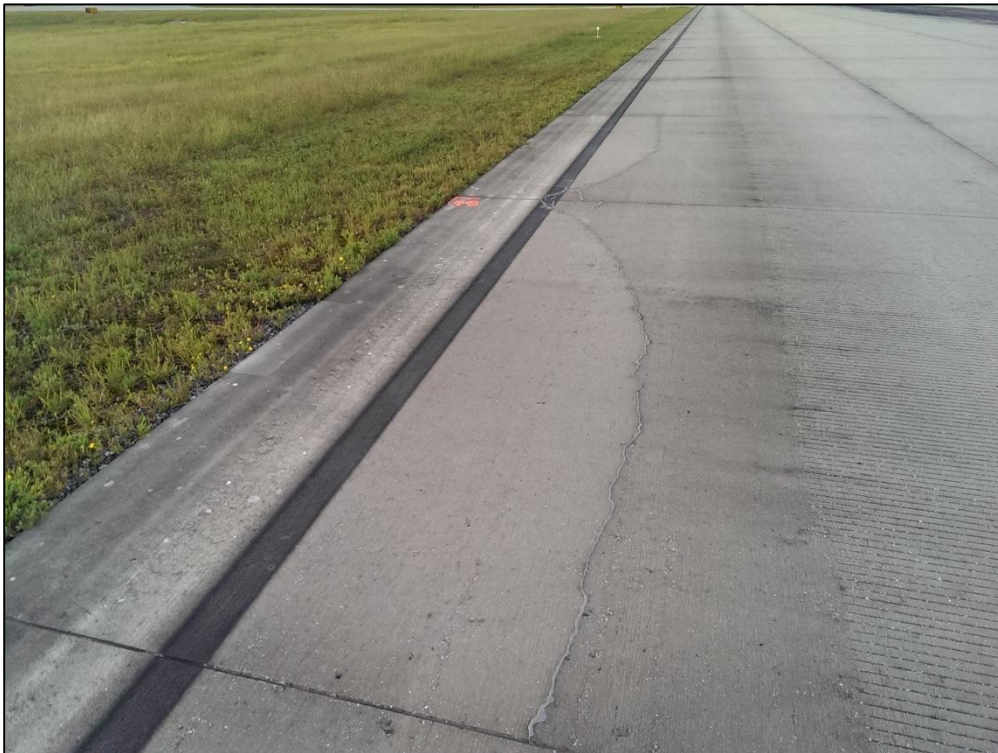
Runway 16-34, Section 6110, Sample Unit 248 – Low Severity (63) Longitudinal, Transverse, and Diagonal Cracking
