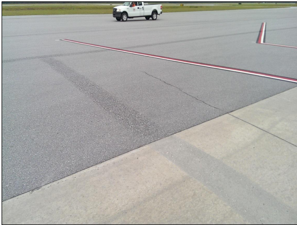
Terminal Apron, Section 4110, Sample Unit 204 – Low Severity (48) Longitudinal and Transverse Cracking, Low Severity (52) Raveling, Low Severity (57) Weathering
