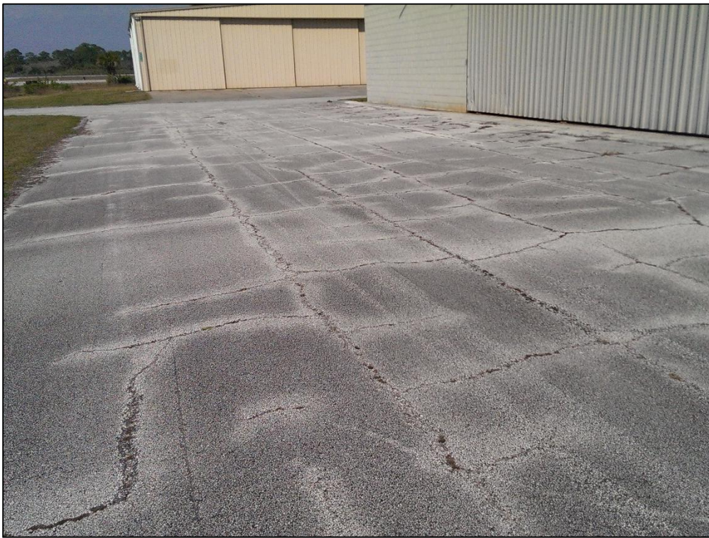
Apron, Section 4140, Sample Unit 316 – Medium Severity (43) Block Cracking, Low Severity (52) Raveling, Medium Severity (57) Weathering
