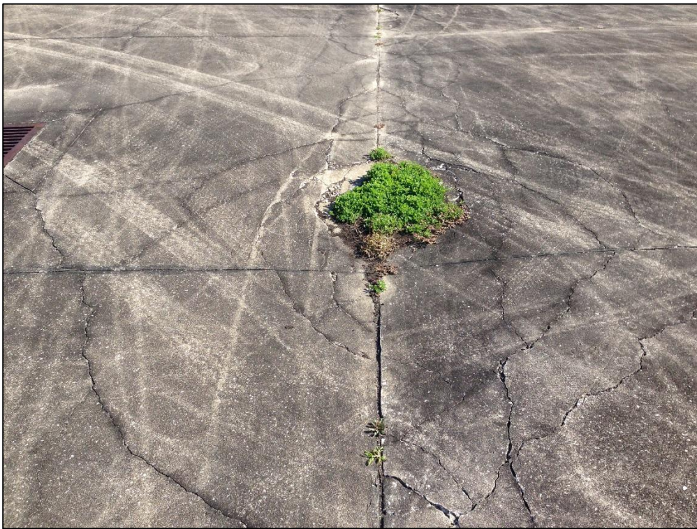
Apron, Section 4102, Sample Unit 101 – Low Severity (72) Shattered Slab, Low Severity (62) Corner Break
