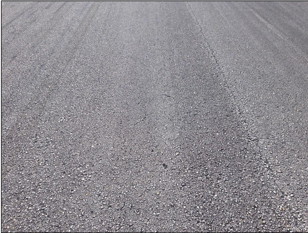
Runway 7-25, Section 6205, Sample Unit 114 – Low Severity (48) Longitudinal and Transverse Cracking, Low Severity (52) Raveling, Low Severity (57) Weathering
