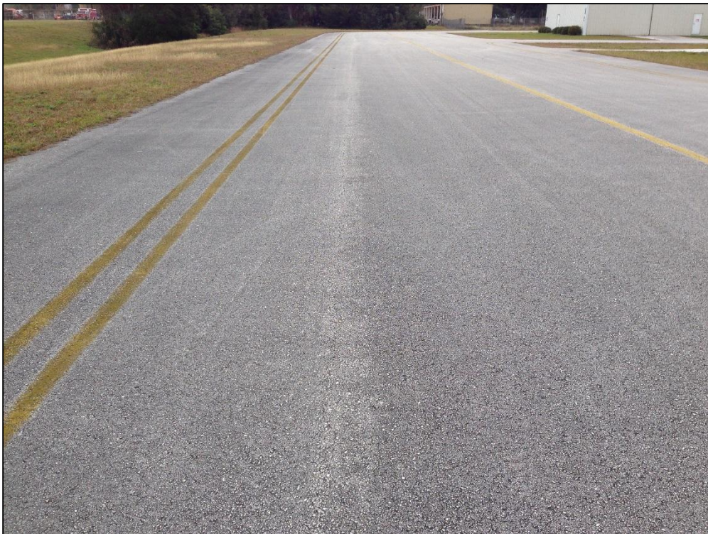
Taxiway Charlie, Section 315, Sample Unit 154 – Low Severity (52) Raveling, Low Severity (57) Weathering
