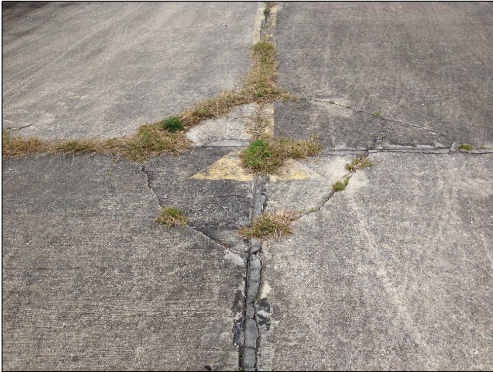
Apron South, Section 4220, Sample Unit 100 – High Severity (62) Corner Break, High Severity (65) Joint Seal Damage, Medium Severity (66) Small Patching
