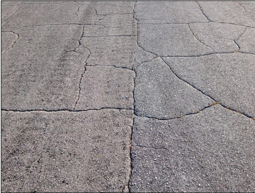
Runway 02-20, Section 6405, Sample Unit 102 – Medium Severity (43) Block Cracking, Low Severity (52) Raveling
