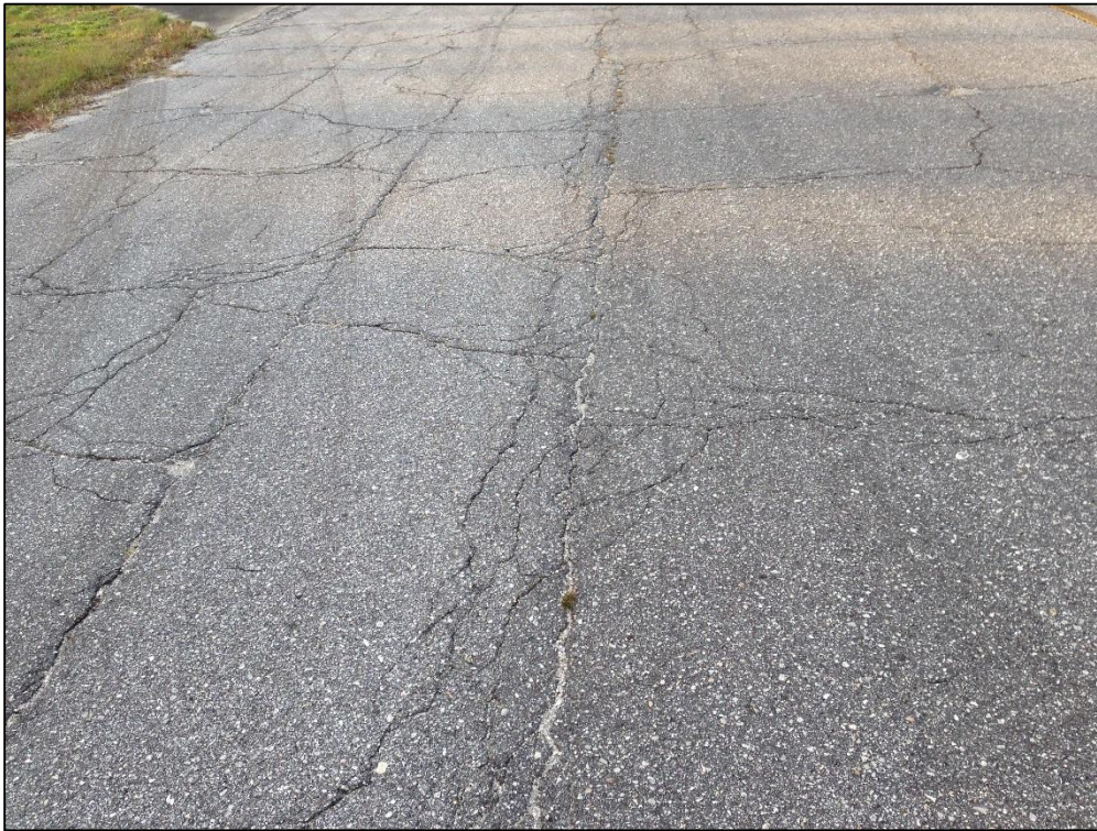
Taxiway Delta, Section 415, Sample Unit 105 – Low Severity (43) Block Cracking, Medium Severity (43) Block Cracking, Low Severity (52) Raveling, Medium Severity (57) Weathering
