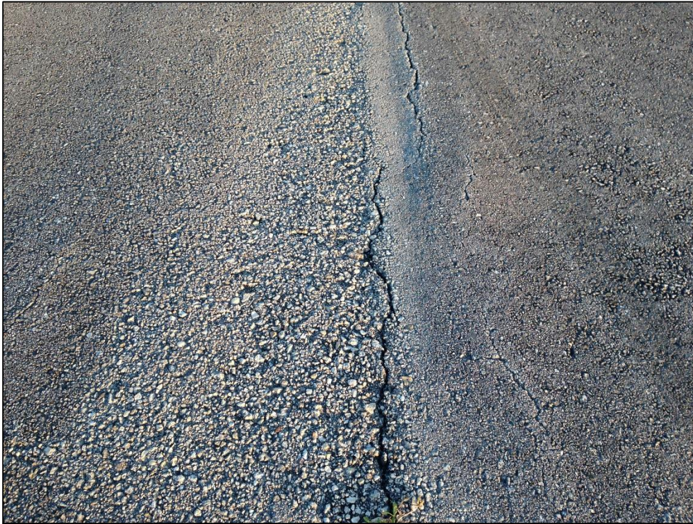
Taxiway Alpha, Section 125, Sample Unit 108 – Low Severity (48) Longitudinal and Transverse Cracking, Low Severity (52) Raveling, Medium Severity (52) Raveling, Low Severity (56) Swelling
