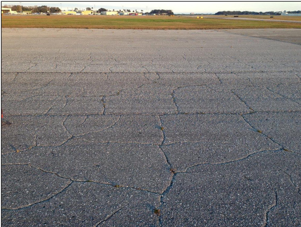
Runway 02-20, Section 6425, Sample Unit 153 – Medium Severity (43) Block Cracking, Low Severity (52) Raveling
