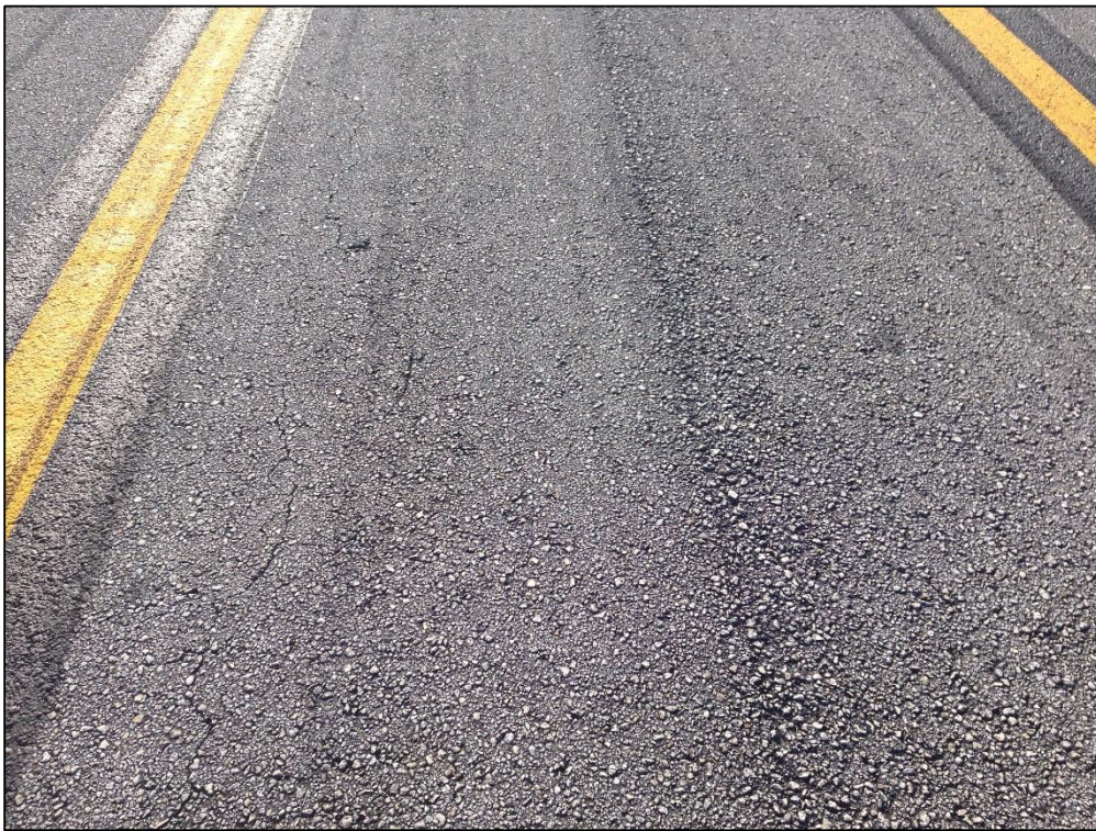
Runway 7-25, Section 6205, Sample Unit 176 – Low Severity (48) Longitudinal and Transverse Cracking, Low Severity (52) Raveling
