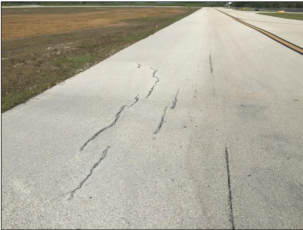
Taxiway Alpha, Section 110, Sample Unit 137 – Low Severity (48) Longitudinal and Transverse Cracking, Low Severity (52) Raveling, Low Severity (53) Rutting, Low Severity (57) Weathering
