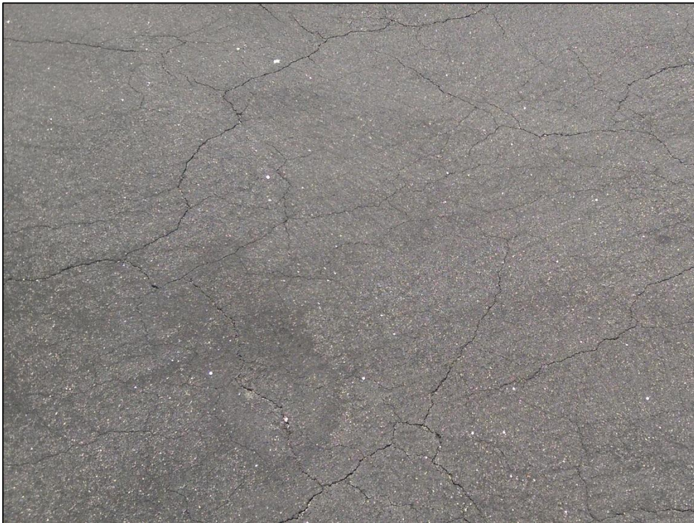
Apron East, Section 4150, Sample Unit 912 – Low Severity (43) Block Cracking, Low Severity (52) Raveling
