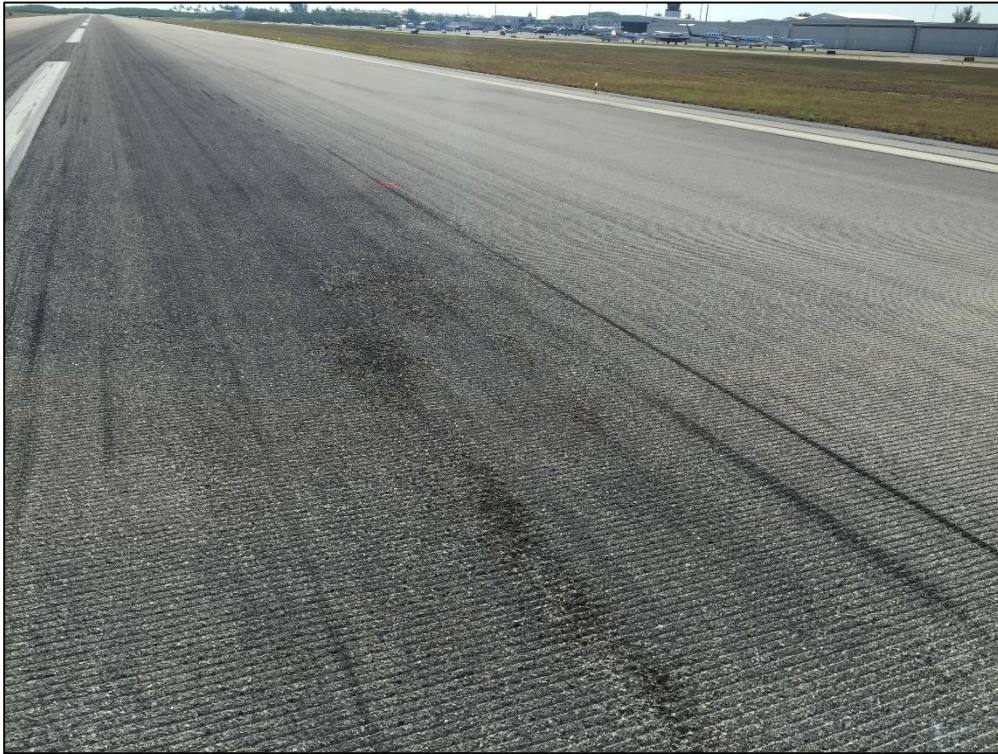
Runway 9-27, Section 6105, Sample Unit 142 – Low Severity (48) Longitudinal and Transverse Cracking, Low Severity (52) Raveling, Medium Severity (52) Raveling
