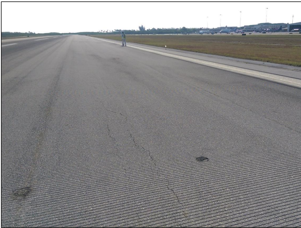
Runway 9-27, Section 6110, Sample Unit 325 – Low Severity (48) Longitudinal and Transverse Cracking, Low Severity (50) Patching, Low Severity (52) Raveling
