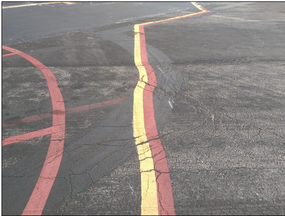
Apron East, Section 4120, Sample Unit 703 – Low Severity (50) Patching, (55) Slippage Cracking, Low Severity (41) Alligator Cracking
