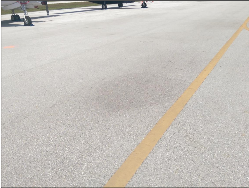
Apron West, Section 4215, Sample Unit 603 – Low Severity (45) Depression, Low Severity (52) Raveling
