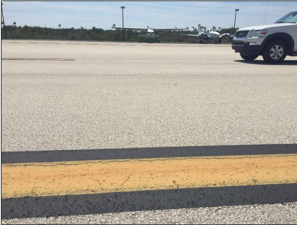
Taxiway Alpha, Section 105, Sample Unit 117 – Low Severity (48) Longitudinal and Transverse Cracking, Low Severity (53) Rutting, Low Severity (57) Weathering
