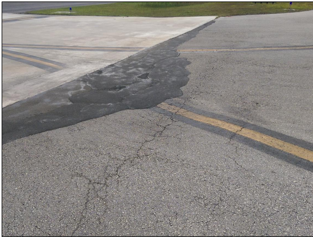
Apron East, Section 4150, Sample Unit 300 – Low Severity (41) Alligator Cracking, Low Severity (45) Depression, Medium Severity (50) Patching, Low and Medium Severity (48) Longitudinal and Transverse Cracking
