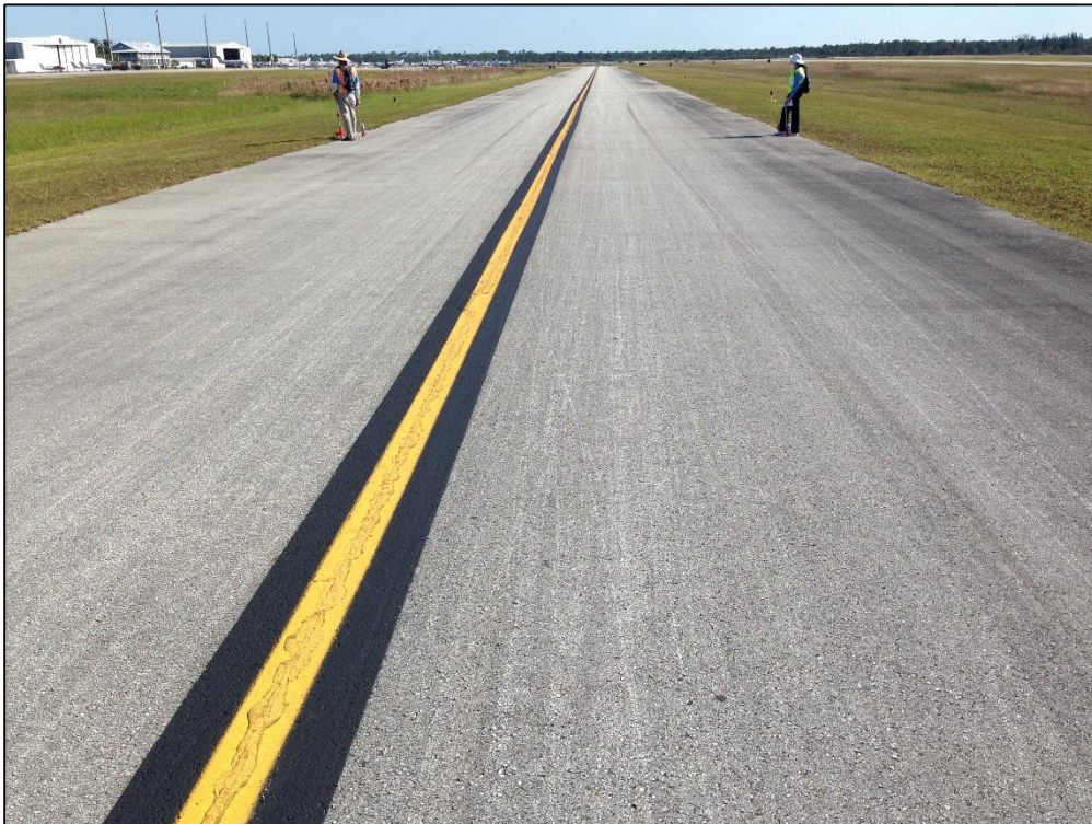
Taxiway Foxtrot, Section 605, Sample Unit 134 – Low Severity (48) Longitudinal and Transverse Cracking, Low Severity (57) Weathering
