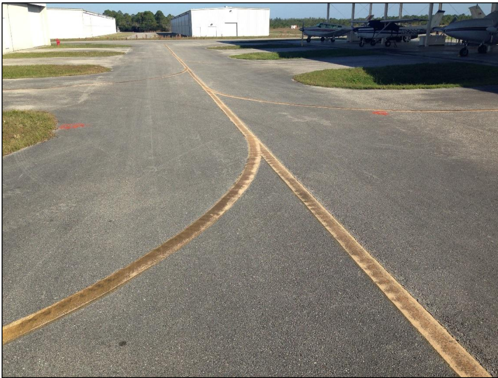
Apron T-Hangar, Section 4205, Sample Unit 302 – Low Severity (48) Longitudinal and Transverse Cracking, Low Severity (52) Raveling, Low Severity (57) Weathering
