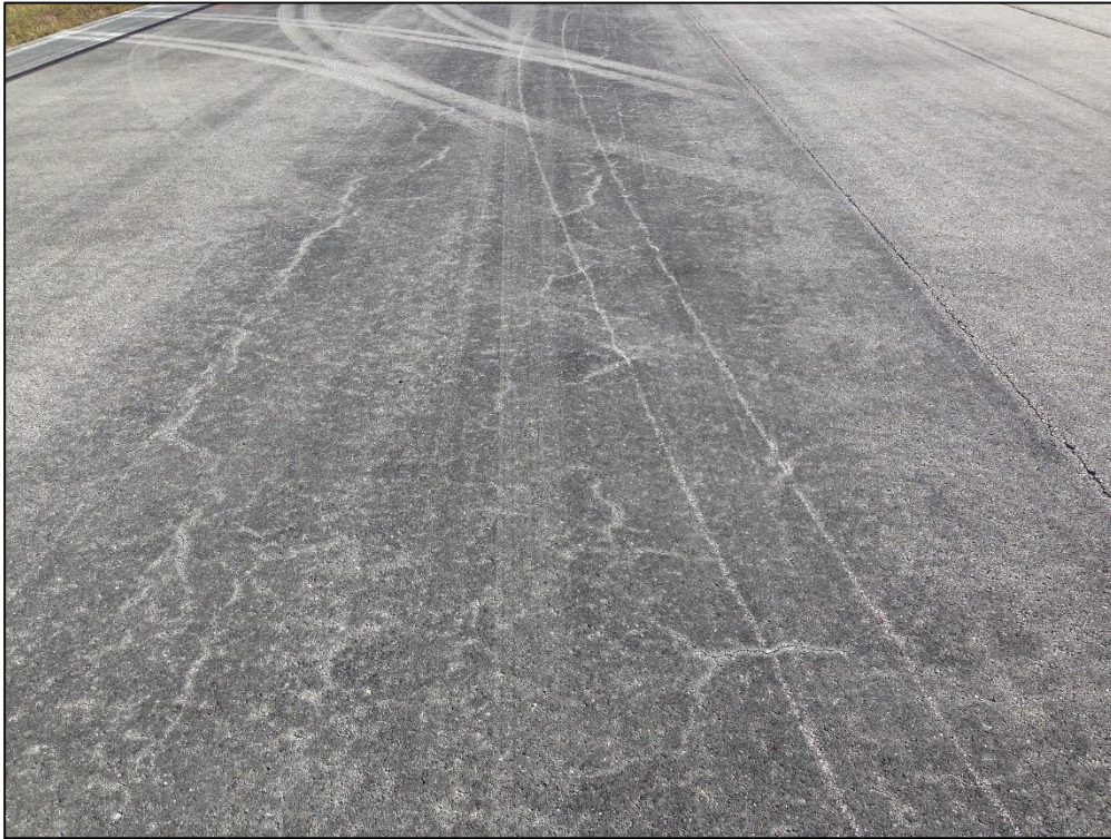
Runway 8R-26L, Section 6105, Sample Unit 134 – Low Severity (48) Longitudinal and Transverse Cracking, Low Severity (56) Swelling, Low Severity (57) Weathering
