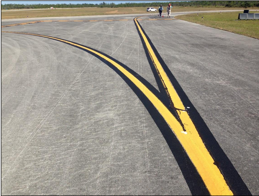
Taxiway Romeo, Section 1805, Sample Unit 101 – Low Severity (48) Longitudinal and Transverse Cracking, Low Severity (52) Raveling, Low Severity (57) Weathering
