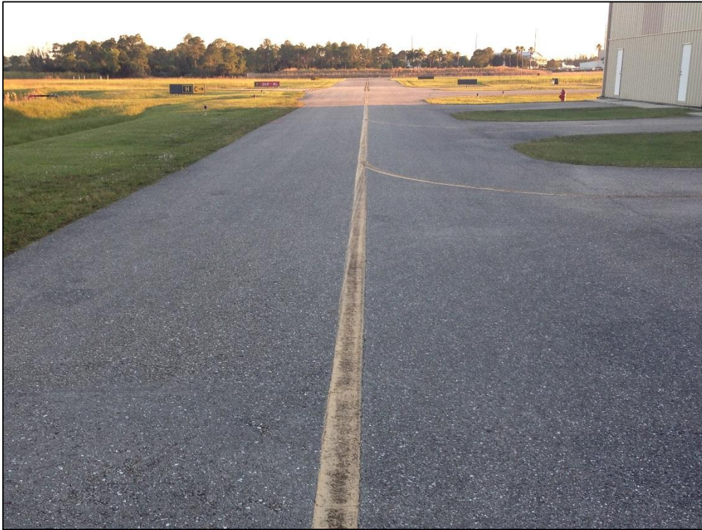
Apron T-Hangar, Section 4305, Sample Unit 801 – Low Severity (57) Weathering
