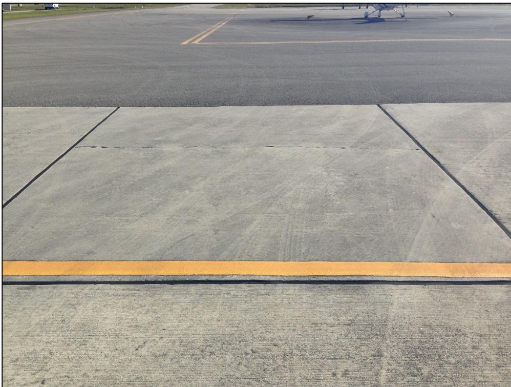
Apron North, Section 4115, Sample Unit 751 – Medium Severity (63) Longitudinal, Transverse, and Diagonal Cracking
