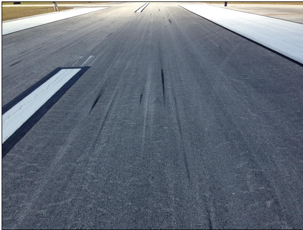
Runway 13-31, Section 6205, Sample Unit 120 – Low Severity (41) Alligator Cracking, Low Severity (52) Raveling, Low Severity (57) Weathering
