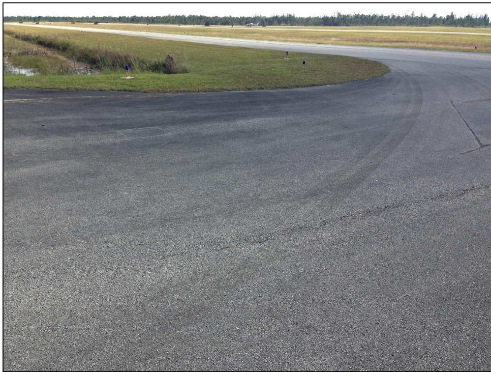
Taxiway Juliet, Section 1010, Sample Unit 100 – Low Severity (48) Longitudinal and Transverse Cracking, Low Severity (50) Patching, Low Severity (52) Raveling, Low Severity (57) Weathering
