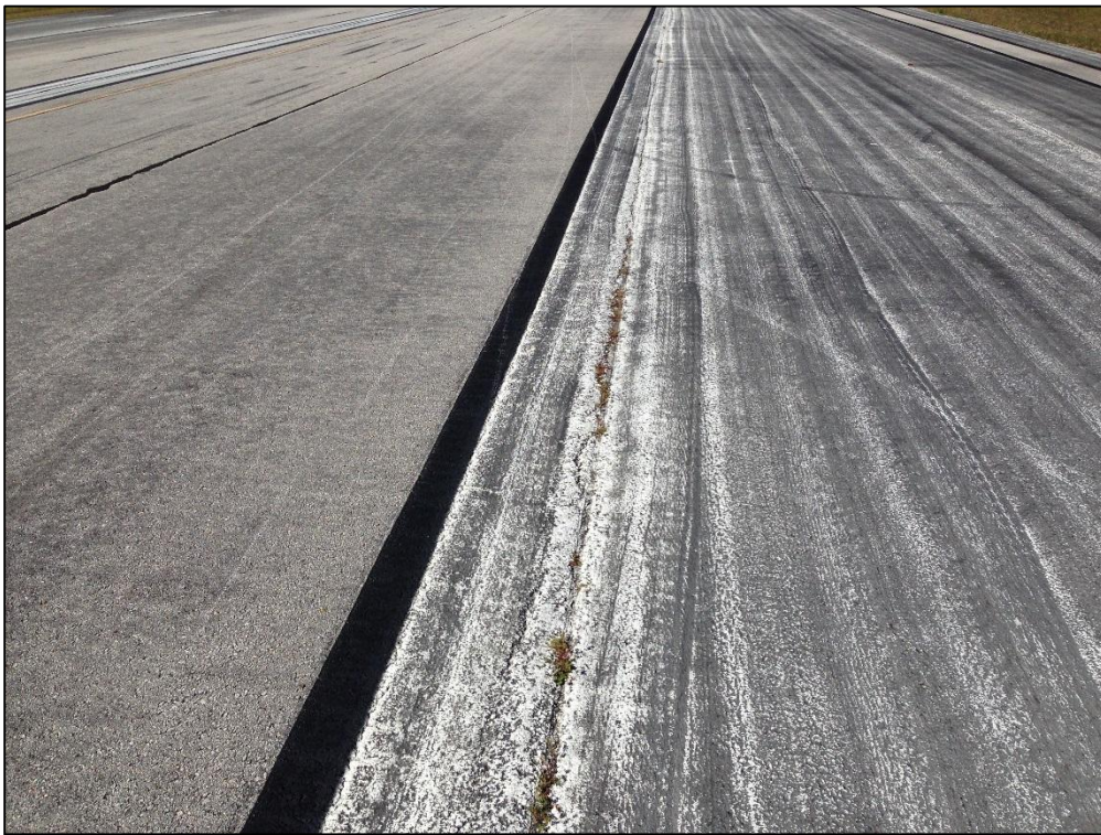
Runway 8R-26L, Section 6105, Sample Unit 122 – Low and Medium Severity (48) Longitudinal and Transverse Cracking, Low Severity (41) Alligator Cracking, Low Severity (52) Raveling, Low Severity (57) Weathering
