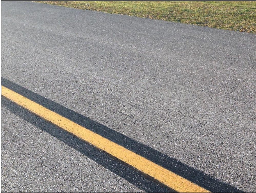
Taxiway Charlie, Section 305, Sample Unit 105 – Low Severity (57) Weathering
