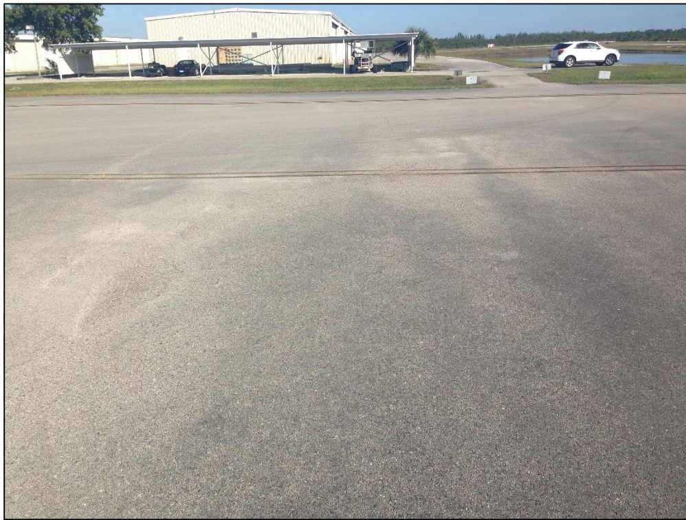
Apron North, Section 4105, Sample Unit 117 – Low Severity (48) Longitudinal and Transverse Cracking, Low Severity (52) Raveling, Low Severity (57) Weathering
