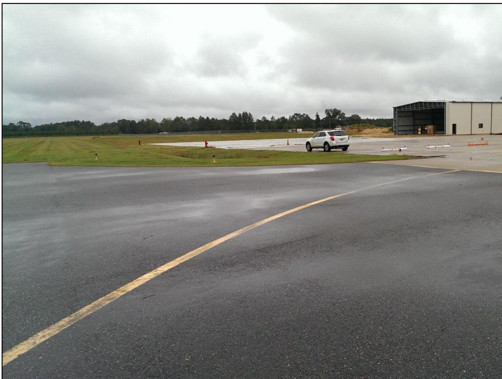
Apron GA, Section 4150, Sample Unit 200 – Low Severity (45) Depression, Low Severity (52) Raveling, Low Severity (57) Weathering
