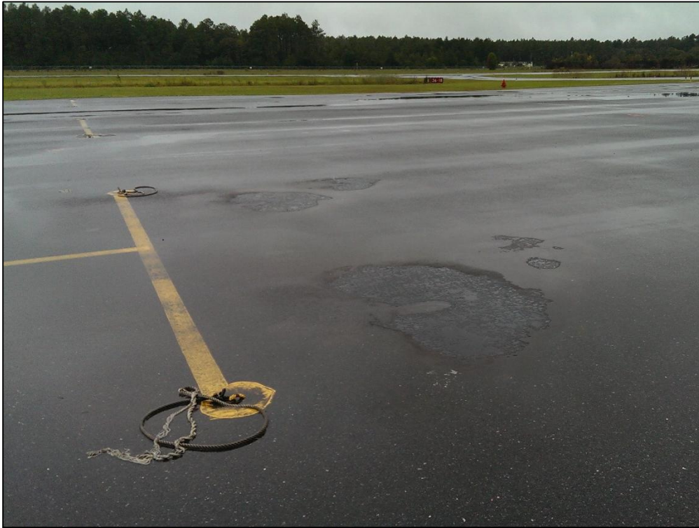
Apron GA, Section 4115, Sample Unit 202 – (49) Oil Spillage, Low Severity (57) Weathering
