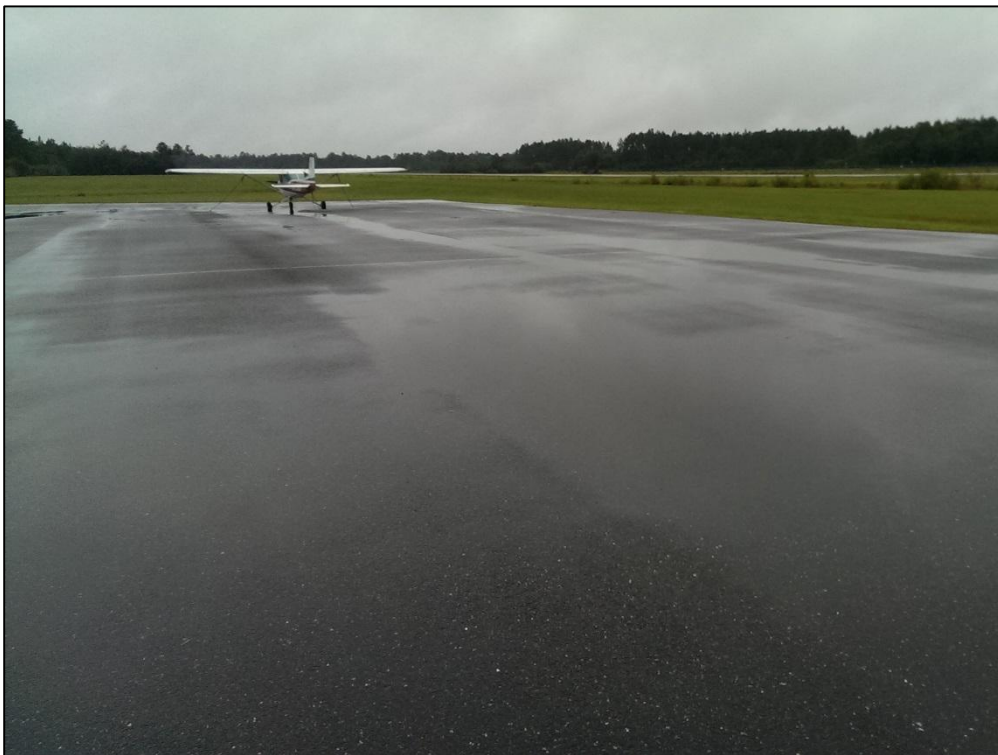
Apron GA, Section 4115, Sample Unit 103 – Low Severity (45) Depression, Low Severity (57) Weathering
