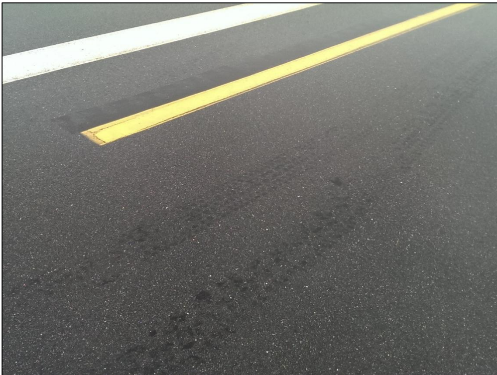
Runway 18-36, Section 6105, Sample Unit 134 – (42) Bleeding, Low Severity (57) Weathering
