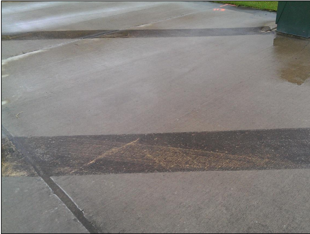
Apron GA, Section 4105, Sample Unit 113 – Low Severity (63) Longitudinal, Transverse, and Diagonal Cracking
