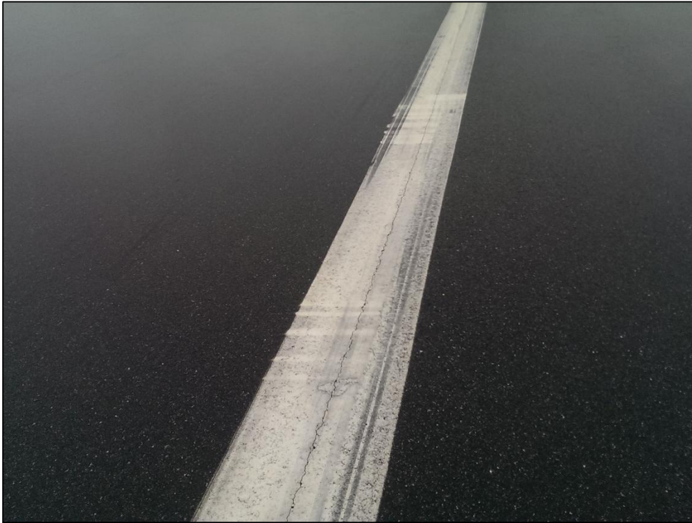
Runway 18-36, Section 6105, Sample Unit 160 – Low Severity (48) Longitudinal and Transverse Cracking, Low Severity (57) Weathering
