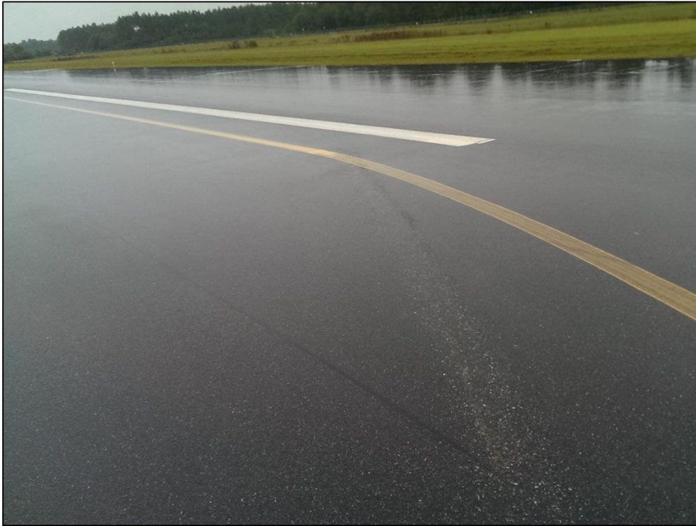
Runway 18-36, Section 6105, Sample Unit 138 – Low Severity (52) Raveling, Low Severity (57) Weathering
