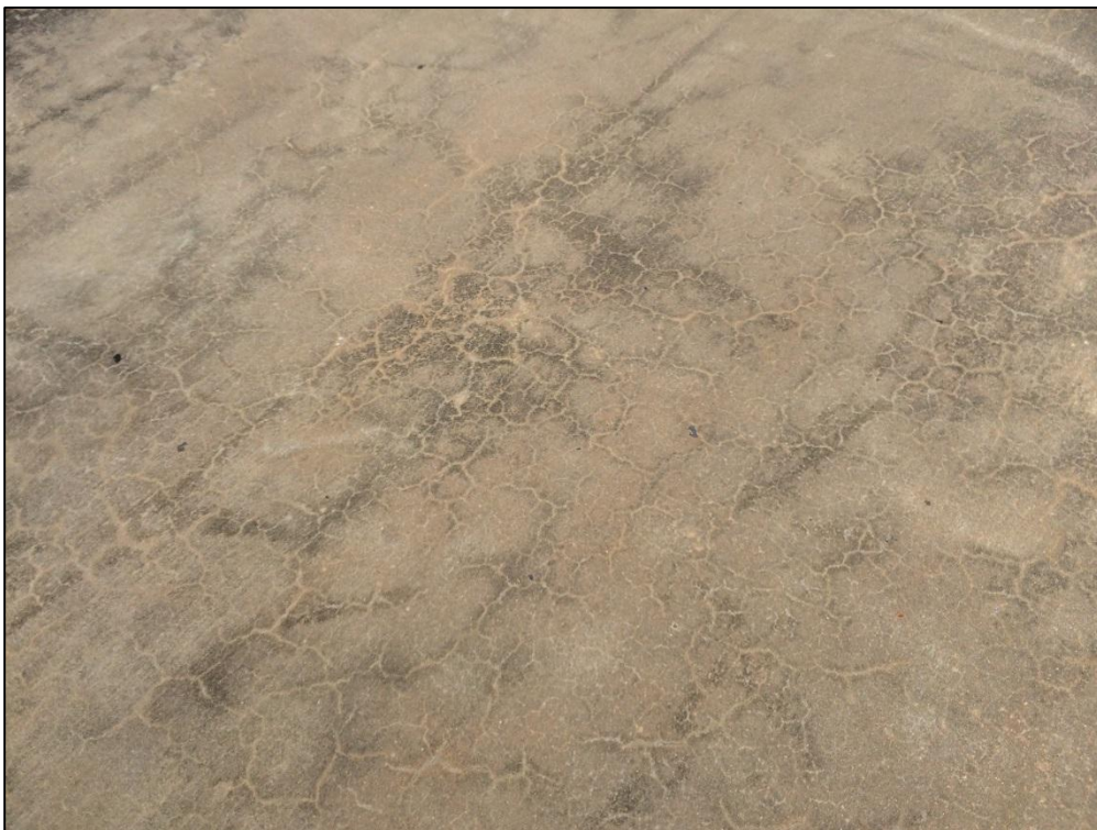
Apron GA, Section 4205, Sample Unit 209 – Low Severity (70) Scaling, Map Cracking, Crazing
