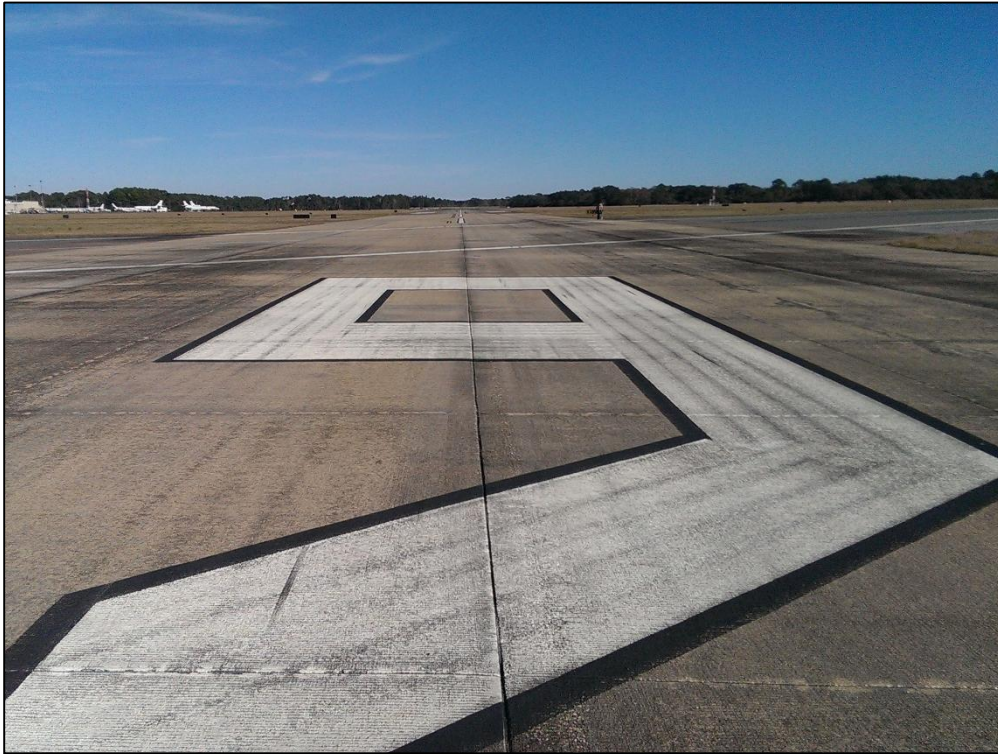
Runway 9-27, Section 6305, Sample Unit 301 – Low Severity (65) Joint Seal Damage
