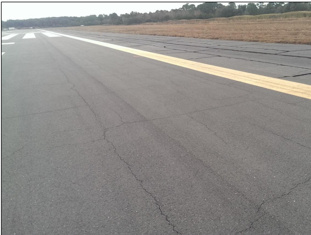
Runway 4-22, Section 6105, Sample Unit 312 – Low Severity (43) Block Cracking, Low Severity (48) Longitudinal and Transverse Cracking, Low Severity (57) Weathering
