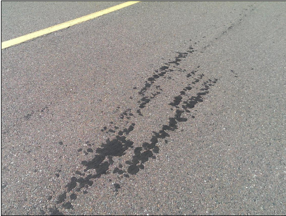
Taxiway Alpha, Section 325, Sample Unit 125 – (42) Bleeding, Low Severity (48) Longitudinal and Transverse Cracking, Low Severity (57) Weathering
