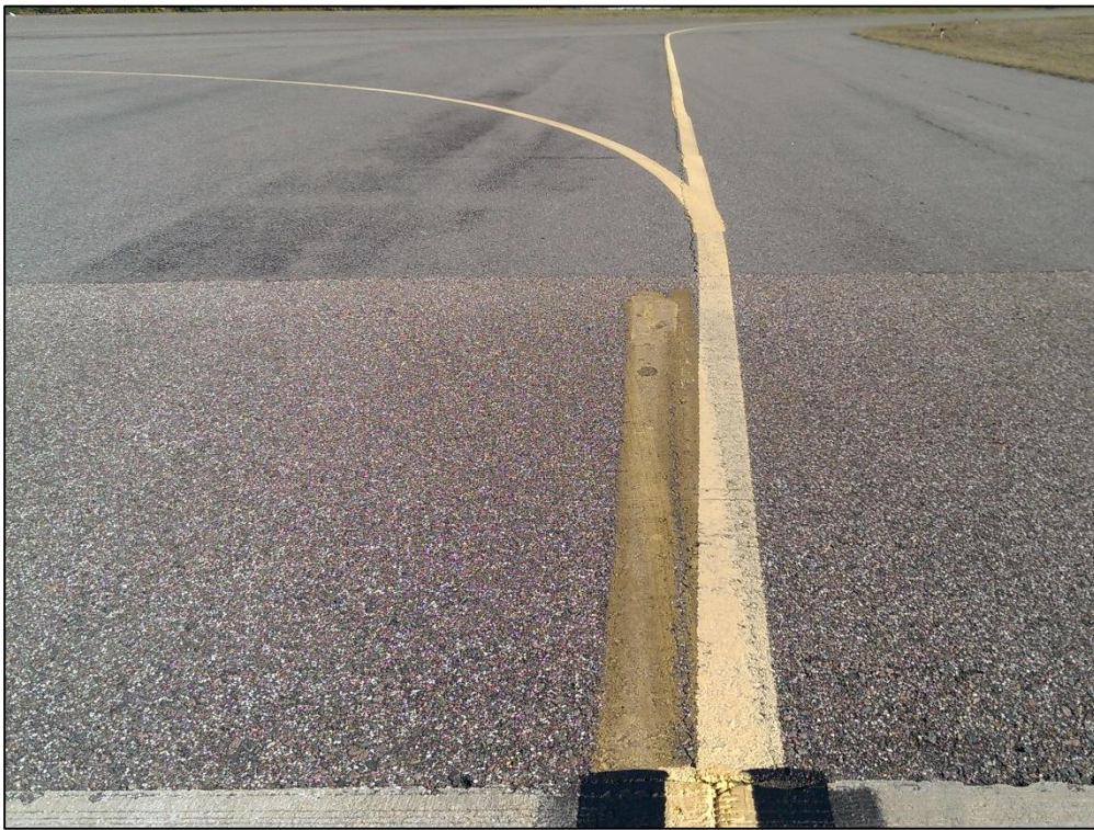
Taxiway Charlie, Section 145, Sample Unit 138 – (42) Bleeding, Low Severity (48) Longitudinal and Transverse Cracking, Low Severity (50) Patching, Low Severity (57) Weathering
