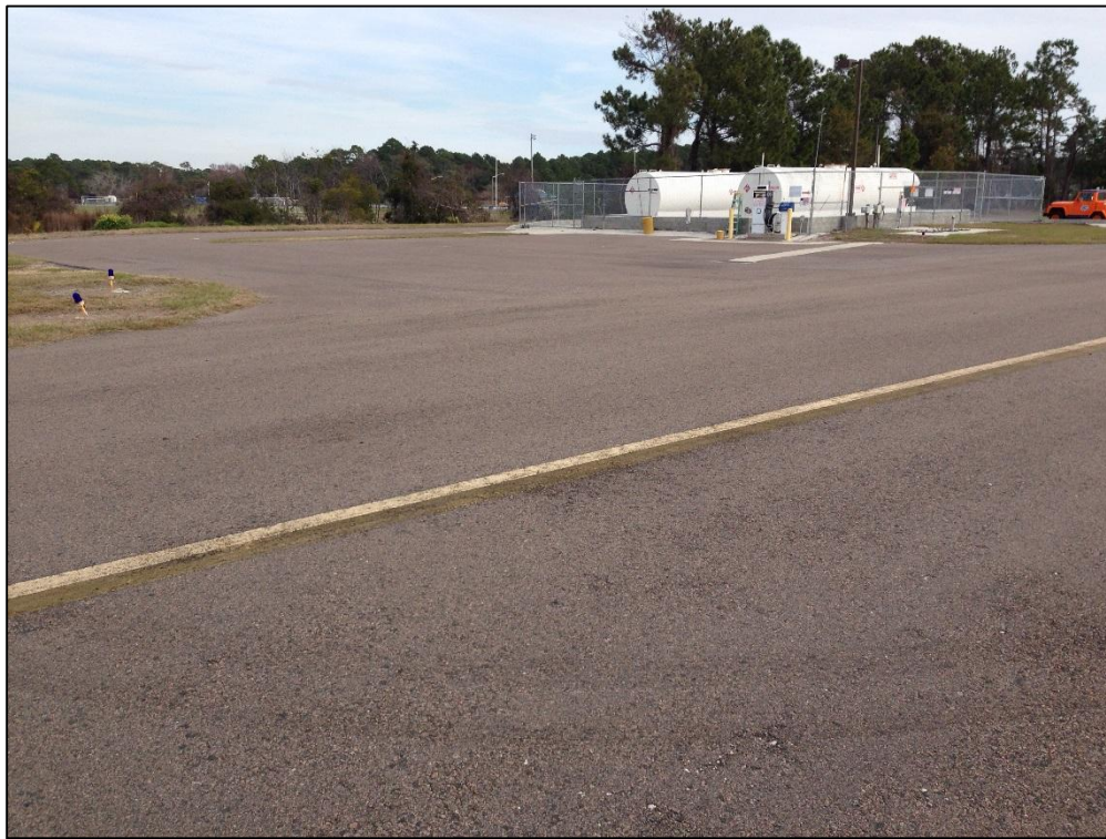
Taxiway Delta, Section 405, Sample Unit 101 – Low Severity (57) Weathering
