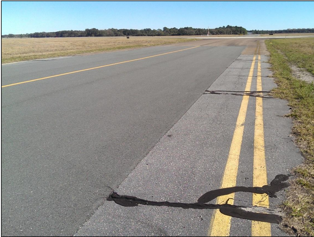
Taxiway Bravo, Section 235, Sample Unit 147 – Low Severity (48) Longitudinal and Transverse Cracking, Low Severity (52) Raveling, Low Severity (57) Weathering
