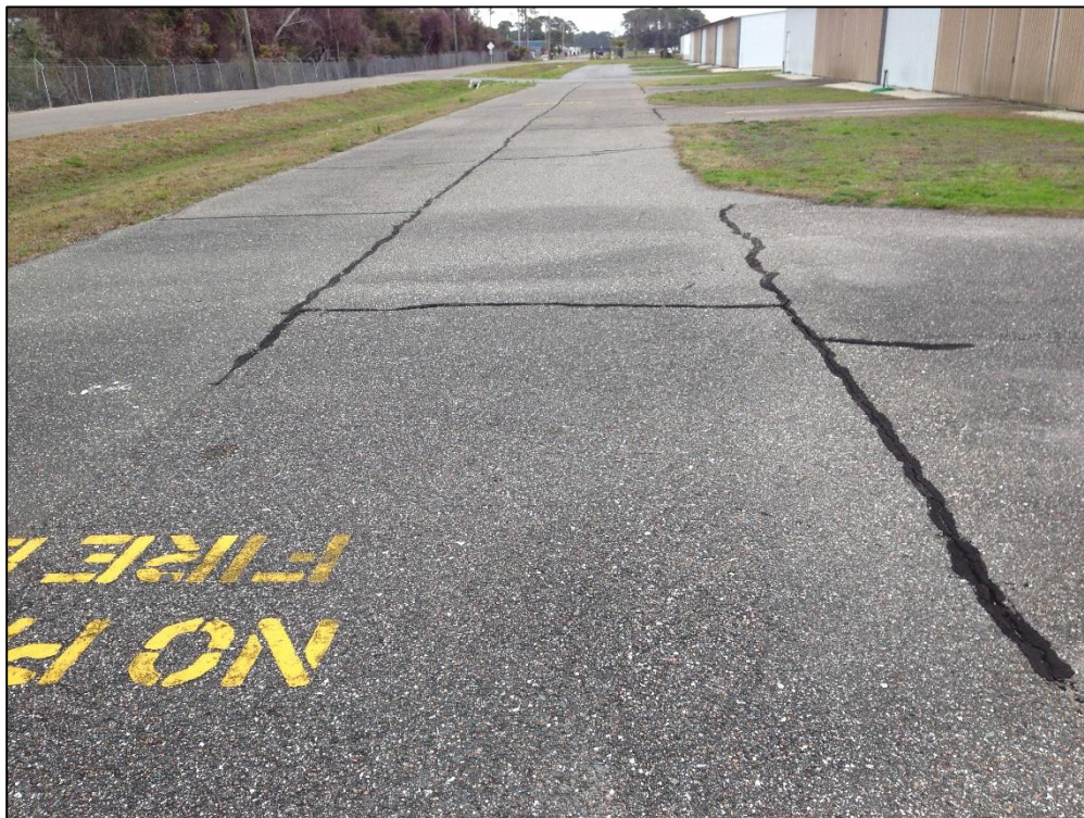
Apron T-Hangar, Section 4310, Sample Unit 106 – Low Severity (48) Longitudinal and Transverse Cracking, Low Severity (57) Weathering
