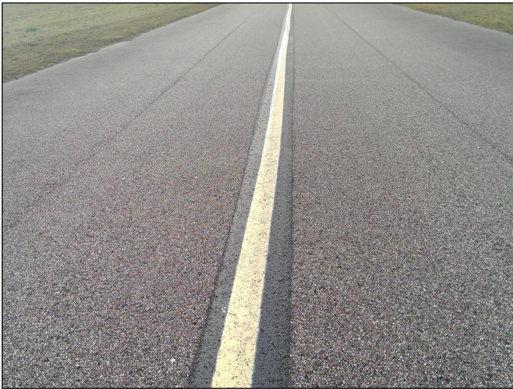
Taxiway Delta, Section 420, Sample Unit 119 – Low Severity (48) Longitudinal and Transverse Cracking, Low Severity (52) Raveling, Low Severity (57) Weathering
