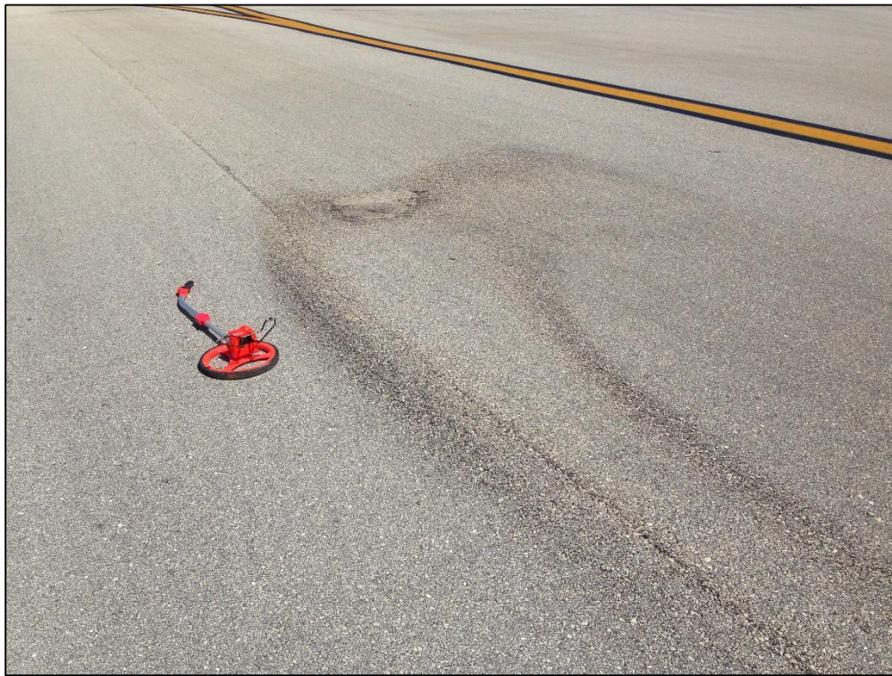
Taxiway Charlie, Section 325, Sample Unit 821 – Low Severity (48) Longitudinal and Transverse Cracking, Low Severity (53) Rutting, (55) Slippage Cracking, Medium Severity (57) Weathering
