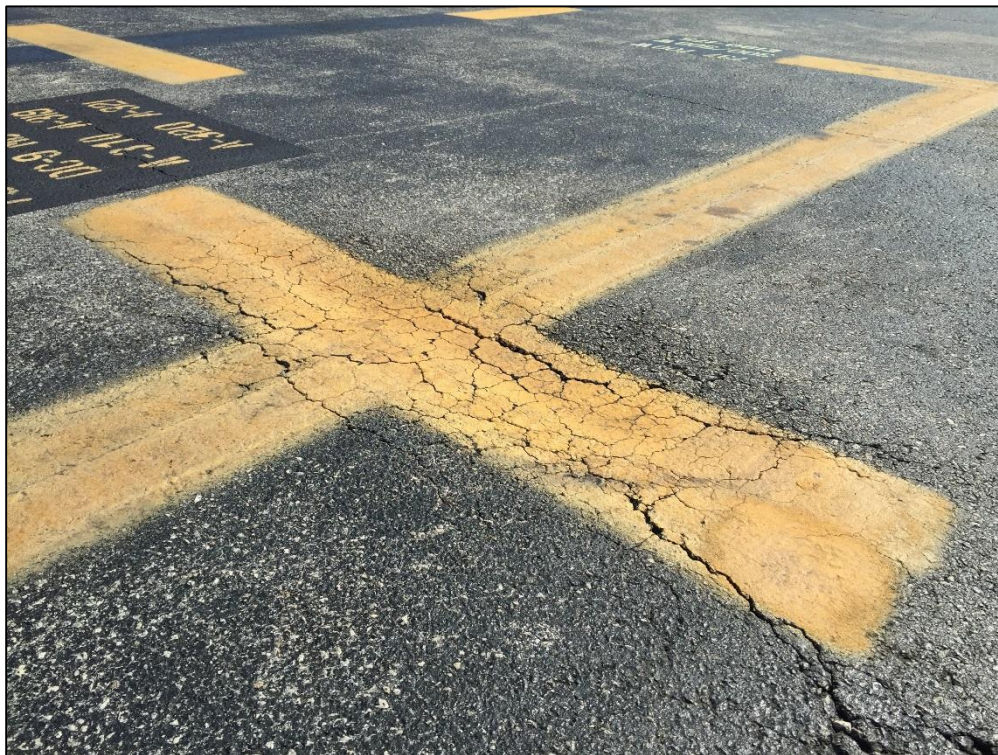
Common Apron, Section 4020, Sample Unit 465 – Low Severity (41) Alligator Cracking, High Severity (45) Depression, Low Severity (52) Raveling
