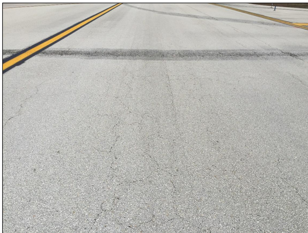
Taxiway November, Section 435, Sample Unit 484 – Low Severity (43) Block Cracking, Low Severity (52) Raveling, Medium Severity (52) Raveling, Low Severity (53) Rutting
