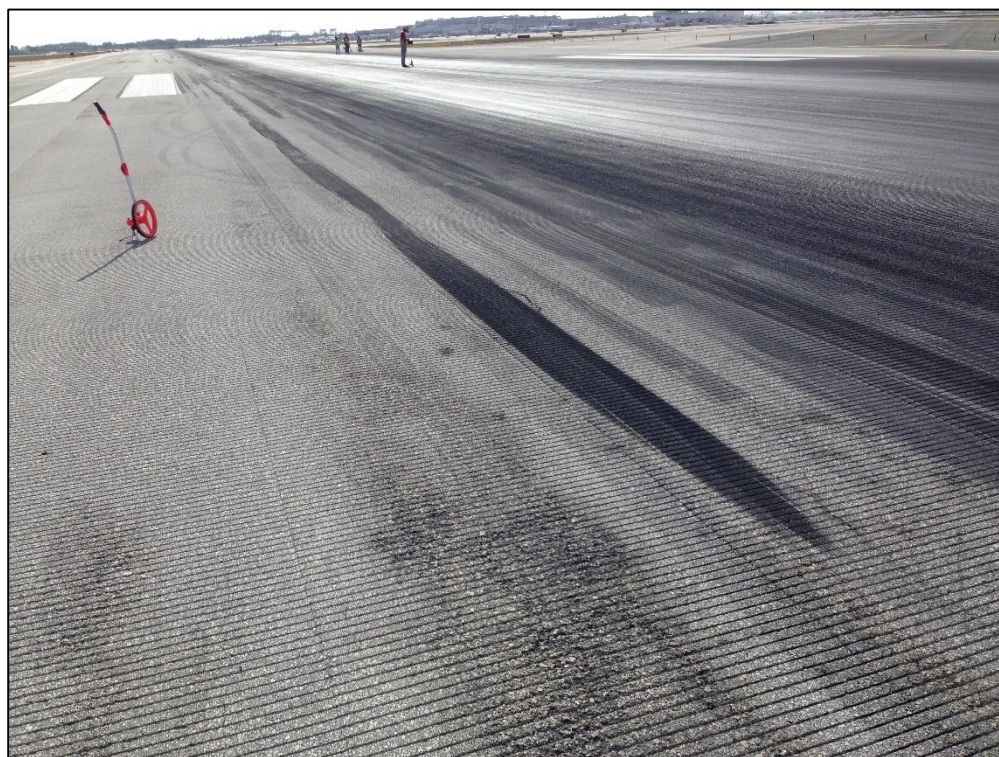
Runway 10L-28R, Section 6140, Sample Unit 125 – Low Severity (48) Longitudinal and Transverse Cracking, Low Severity (52) Raveling, Medium Severity (52) Raveling
