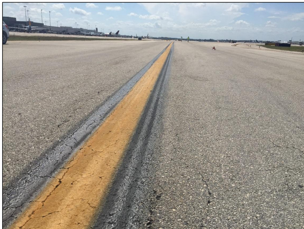
Taxiway B8, Section 290, Sample Unit 207 – Low Severity (48) Longitudinal and Transverse Cracking, Low Severity (52) Raveling, Low Severity (53) Rutting, Medium Severity (57) Weathering
