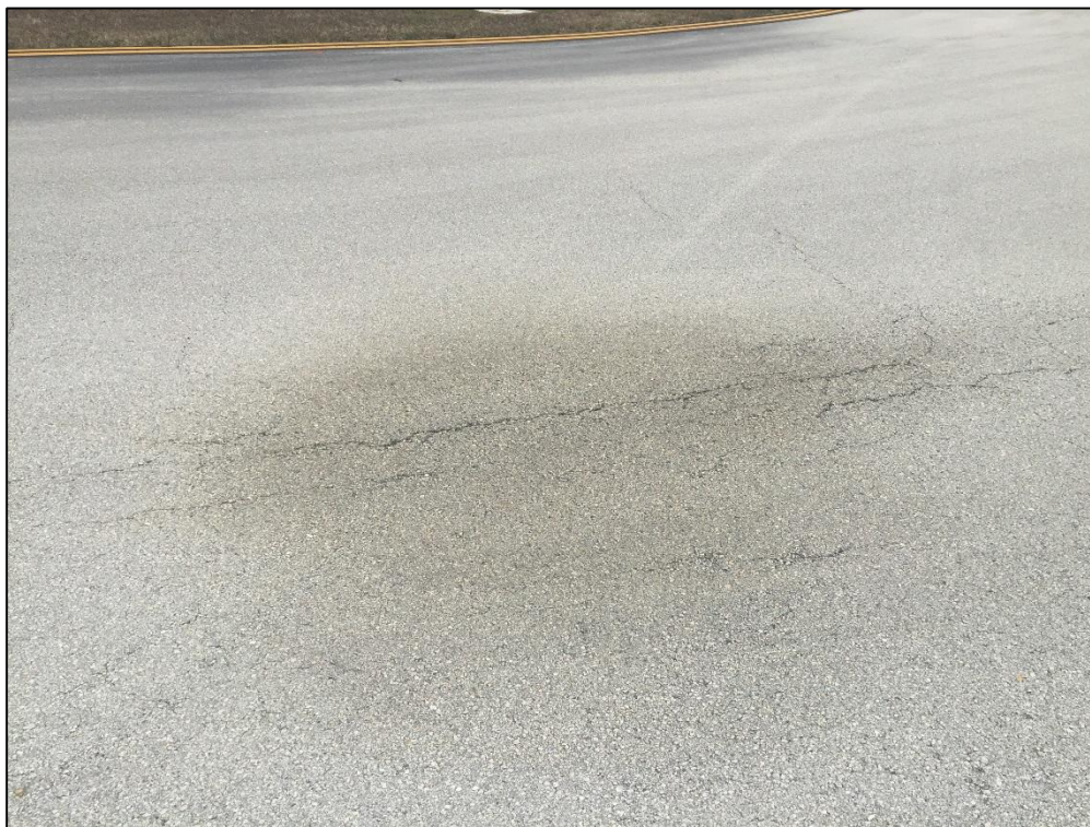
Taxiway Alpha, Section 126, Sample Unit 101 – Medium Severity (45) Depression, Low Severity (48) Longitudinal and Transverse Cracking, Low Severity (52) Raveling, Medium Severity (57) Weathering
