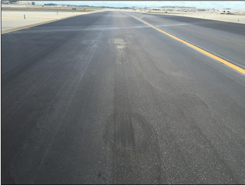
Taxiway Bravo, Section 215, Sample Unit 560 – Low Severity (48) Longitudinal and Transverse Cracking, Low Severity (53) Rutting, Medium Severity (53) Rutting, Low Severity (57) Weathering, Medium Severity (57) Weathering
