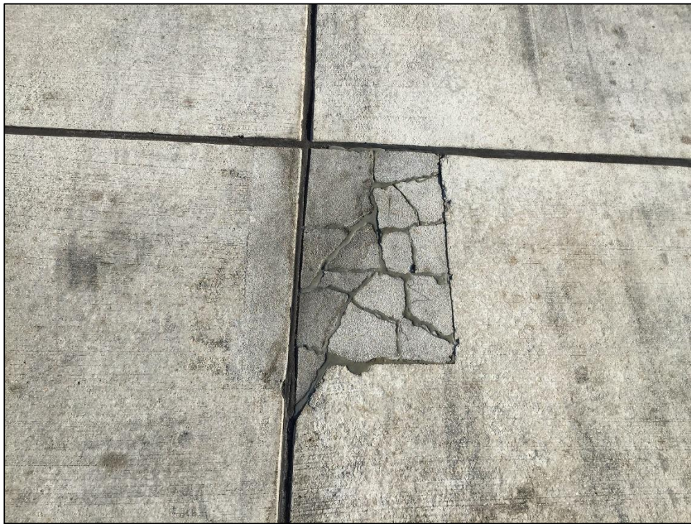
Apron Concourse D, Section 4205, Sample Unit 325 – High Severity (66) Small Patching
