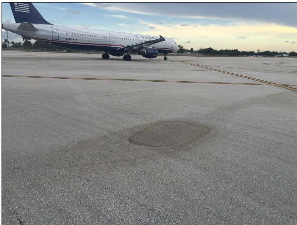
Taxiway Echo, Section 526, Sample Unit 729 – Low Severity (48) Longitudinal and Transverse Cracking, Low Severity (45) Depression, Medium Severity (57) Weathering
