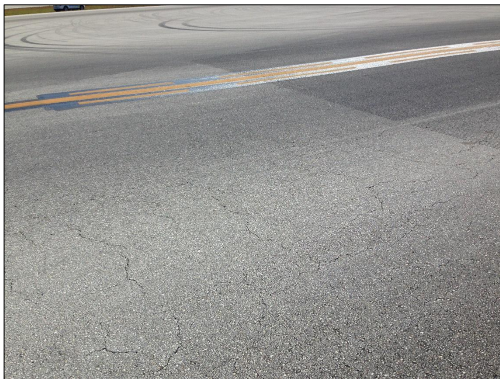
Taxiway B6, Section 280, Sample Unit 110 – Low Severity (43) Block Cracking, Low Severity (52) Raveling, Low Severity (53) Rutting, Low Severity (57) Weathering
