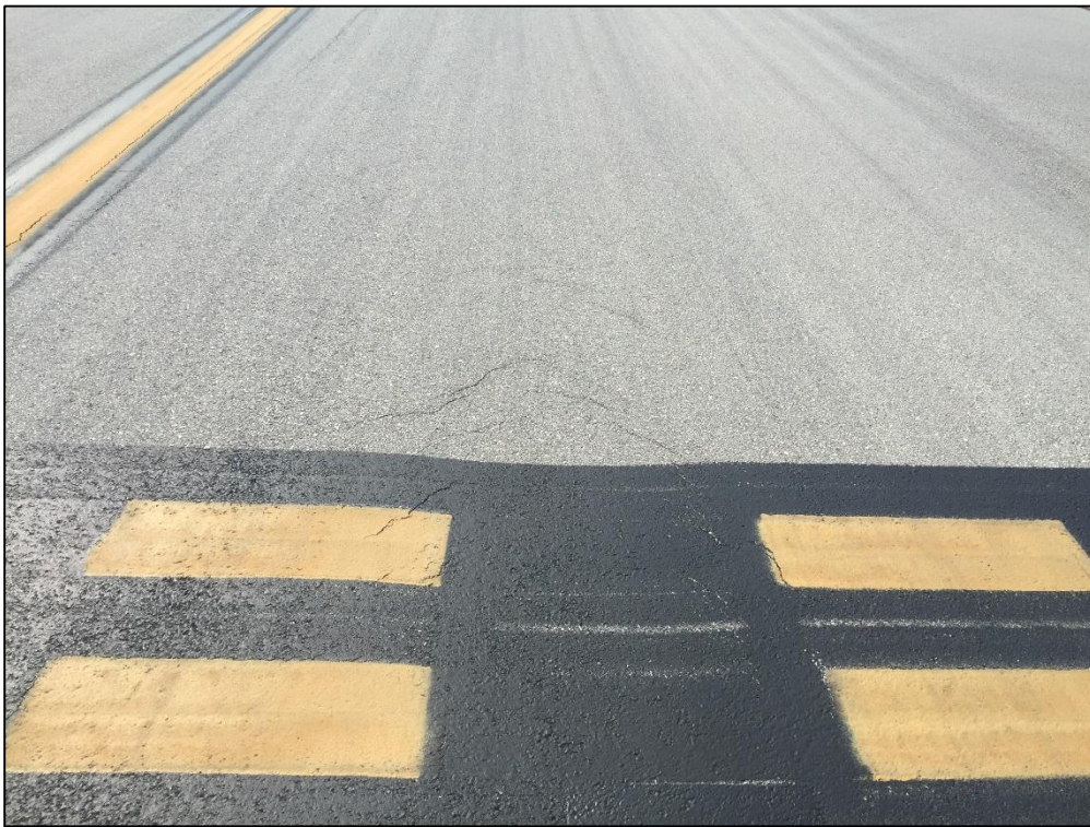
Taxiway B4, Section 278, Sample Unit 107 – Low Severity (48) Longitudinal and Transverse Cracking, (55) Slippage Cracking, Low Severity (57) Weathering, Medium Severity (57) Weathering
