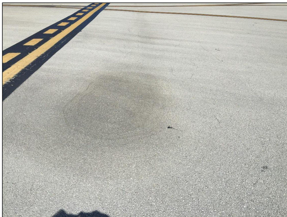
Taxiway T3, Section 2025, Sample Unit 100 – Medium Severity (45) Depression, Low Severity (48) Longitudinal and Transverse Cracking, Low Severity (52) Raveling, Low Severity (57) Weathering
