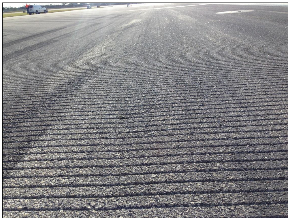
Runway 10L-28R, Section 6155, Sample Unit 379 – Low Severity (48) Longitudinal and Transverse Cracking, Low Severity (52) Raveling, Low Severity (53) Rutting
