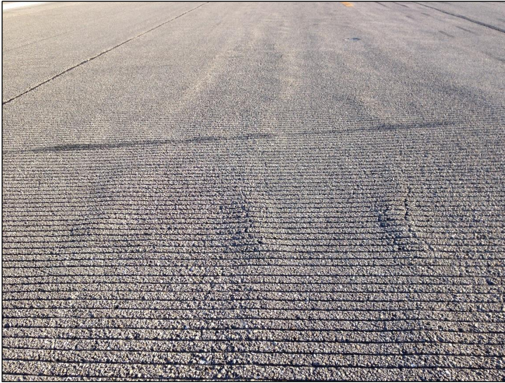
Runway 5-23, Section 6125, Sample Unit 378 – Low Severity (48) Longitudinal and Transverse Cracking, Low Severity (56) Swelling, Medium Severity (56) Swelling, Low Severity (57) Weathering
