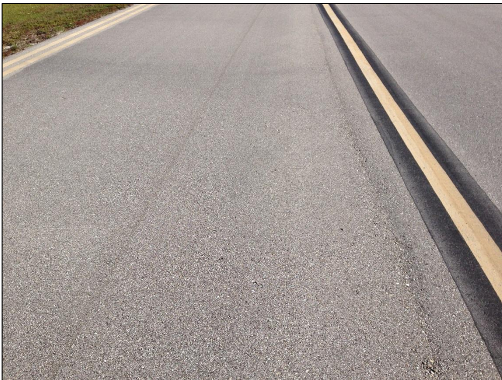
Taxiway E2, Section 530, Sample Unit 504 – Low Severity (52) Raveling, Low Severity (57) Weathering
