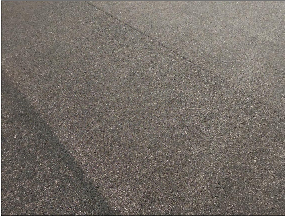
Apron West, Section 4805, Sample Unit 607 – Low Severity (57) Weathering
