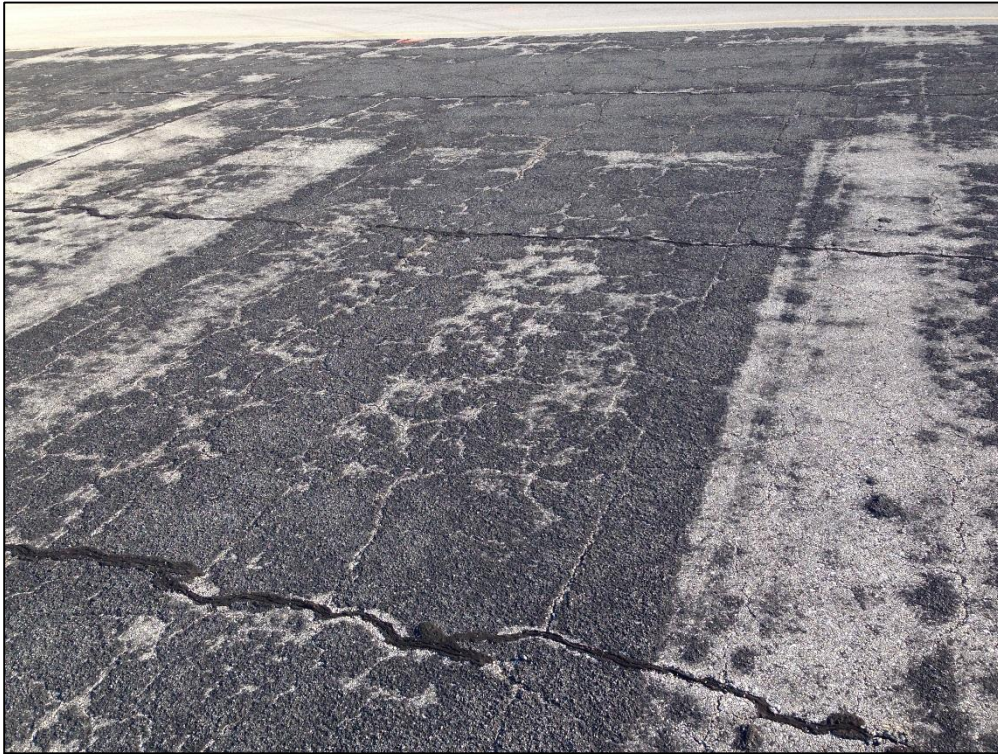
Apron South & Southeast, Section 4415, Sample Unit 210 – Low Severity (43) Block Cracking, Low Severity (52) Raveling
