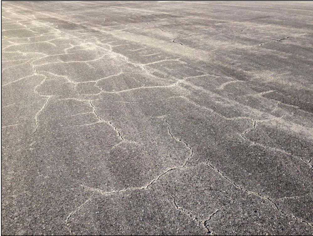
Runway 13-31, Section 6210, Sample Unit 156 – Low Severity (43) Block Cracking, Low Severity (52) Raveling
