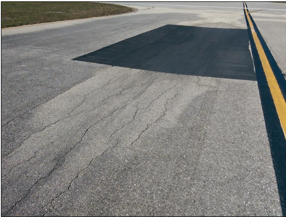
Taxiway Bravo, Section 212, Sample Unit 124 – Low Severity (41) Alligator Cracking, Low Severity (50) Patching, Low Severity (52) Raveling, Low Severity (57) Weathering
