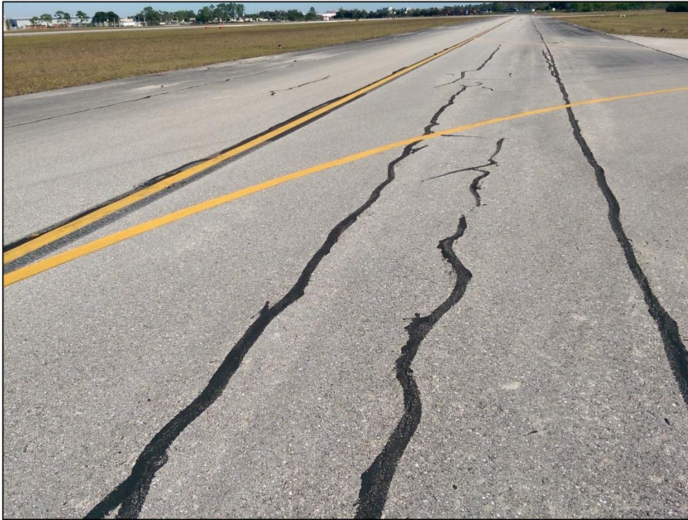
Taxiway Alpha, Section 110, Sample Unit 118 – Low Severity (48) Longitudinal and Transverse Cracking, Low Severity (53) Rutting, Low Severity (57) Weathering
