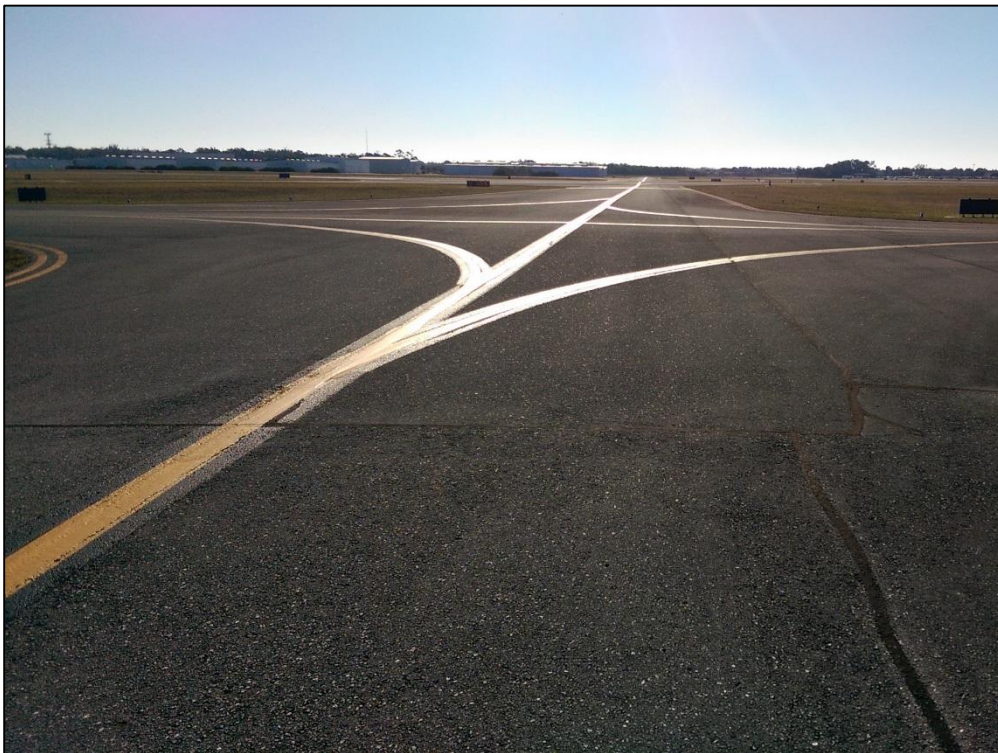
Taxiway Bravo, Section 205, Sample Unit 130 – Low Severity (48) Longitudinal and Transverse Cracking, Low Severity (52) Raveling, Low Severity (57) Weathering
