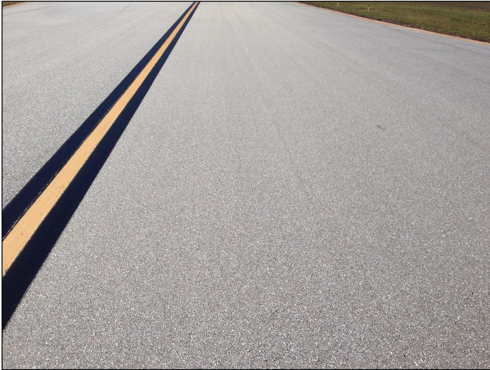
Taxiway Charlie, Section 305, Sample Unit 218 – Low Severity (48) Longitudinal and Transverse Cracking, Low Severity (57) Weathering
