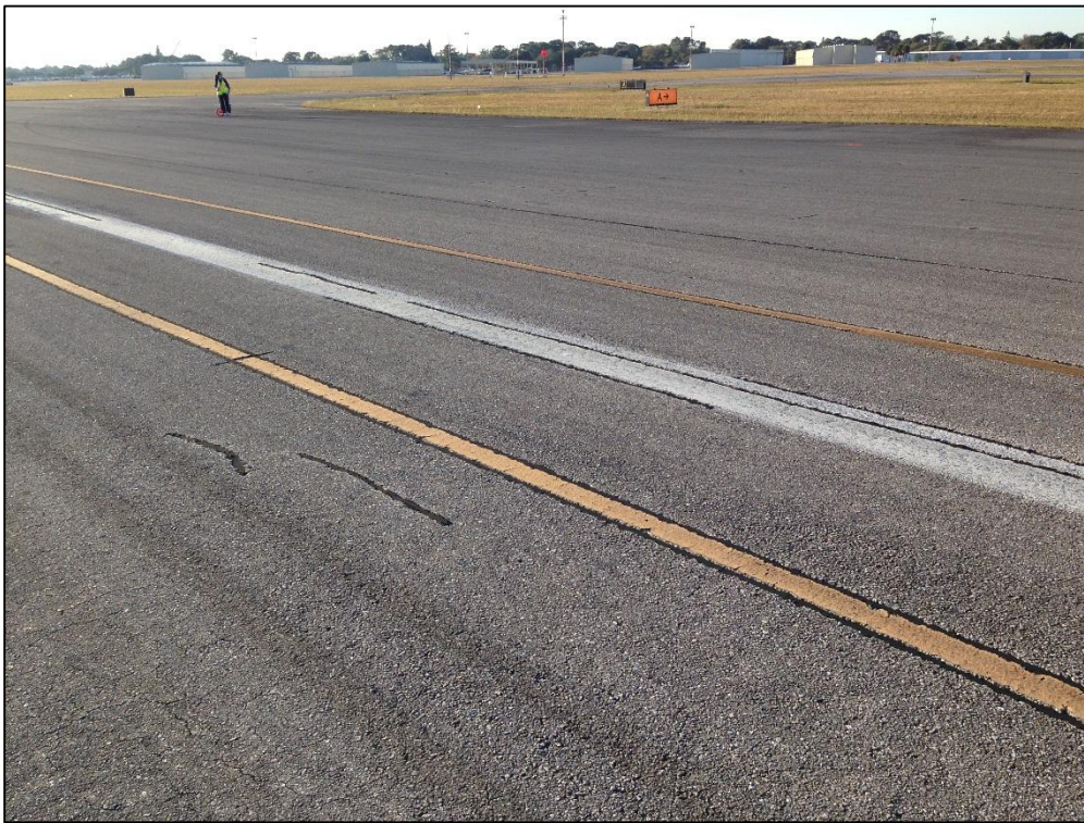
Runway 13-31, Section 6205, Sample Unit 343 – Low Severity (48) Longitudinal and Transverse Cracking, Low Severity (53) Rutting, Medium Severity (57) Weathering
