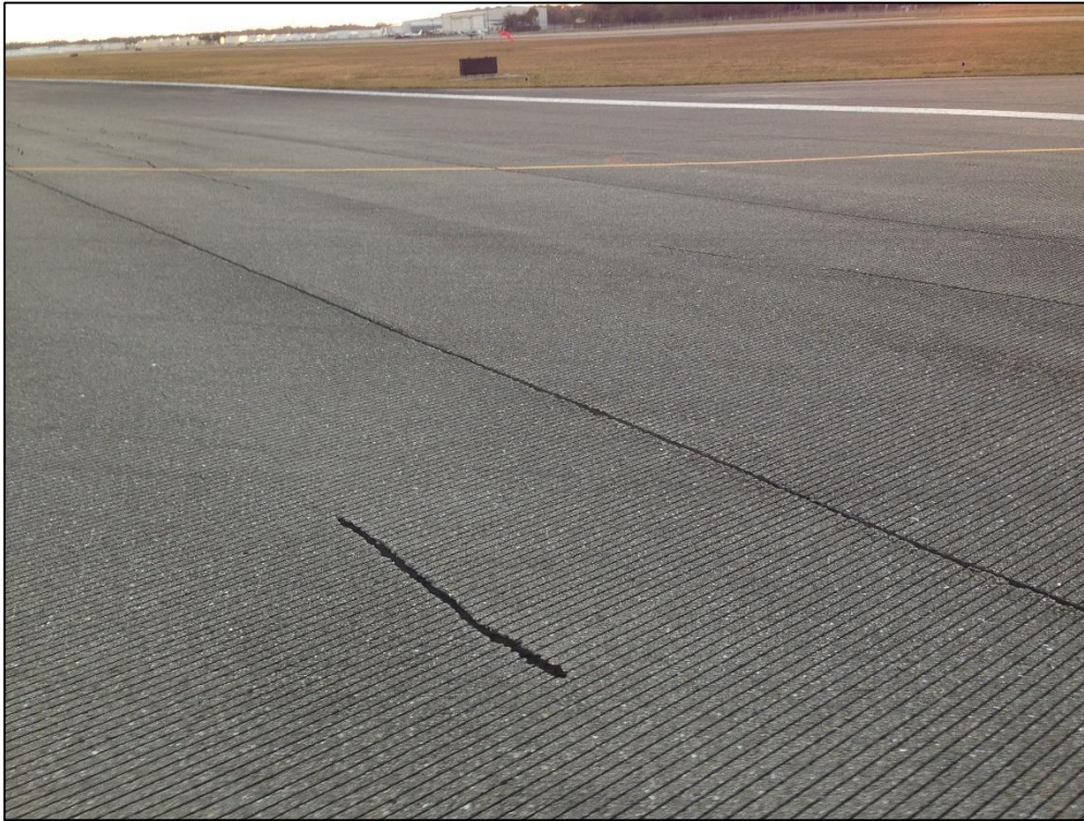
Runway 5-23, Section 6105, Sample Unit 301 – Low Severity (48) Longitudinal and Transverse Cracking, Low Severity (56) Swelling, Low Severity (57) Weathering
