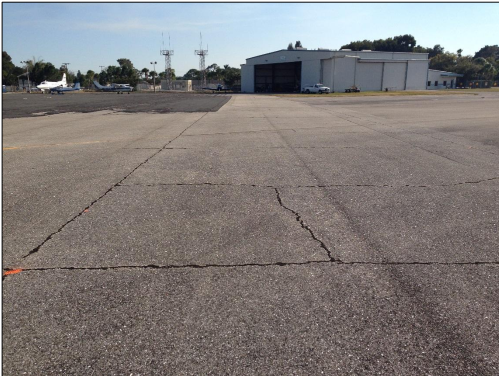
Apron Southwest, Section 4215, Sample Unit 450 – Low Severity (48) Longitudinal and Transverse Cracking, Low Severity (52) Raveling, Low Severity (57) Weathering
