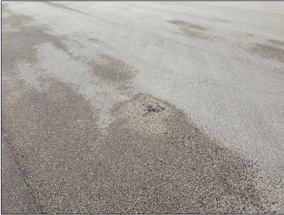
Apron South, Section 5905, Sample Unit 402 – Low Severity (48) Longitudinal and Transverse Cracking, High Severity (52) Raveling
