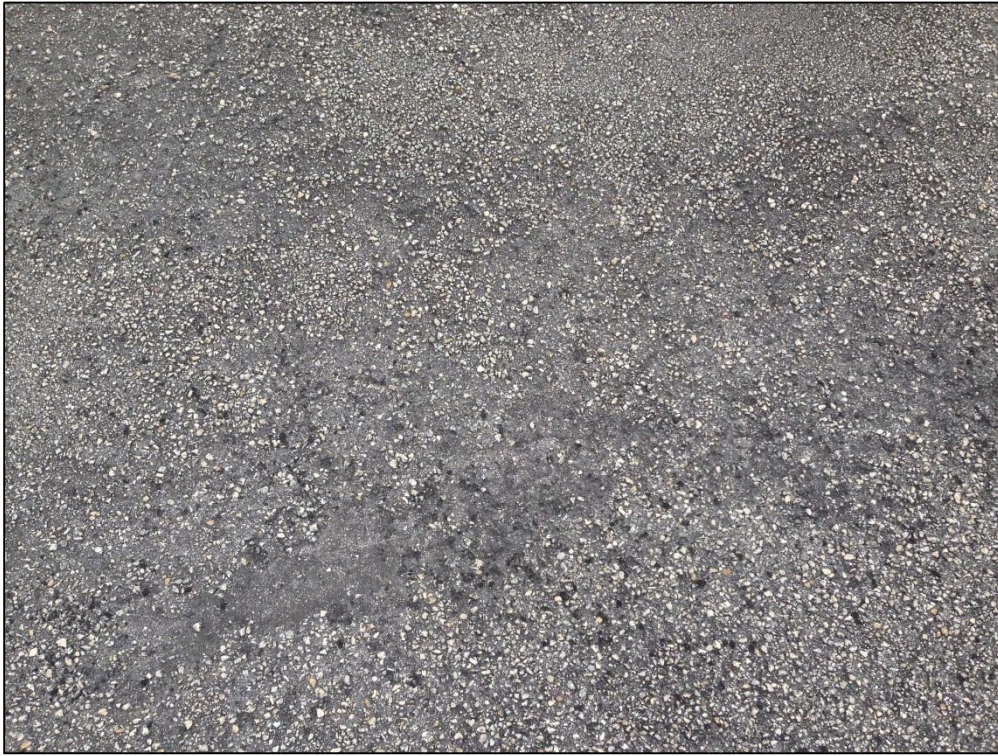
Taxiway South 2, Section 1910, Sample Unit 104 – Low Severity (52) Raveling, Low Severity (57) Weathering
