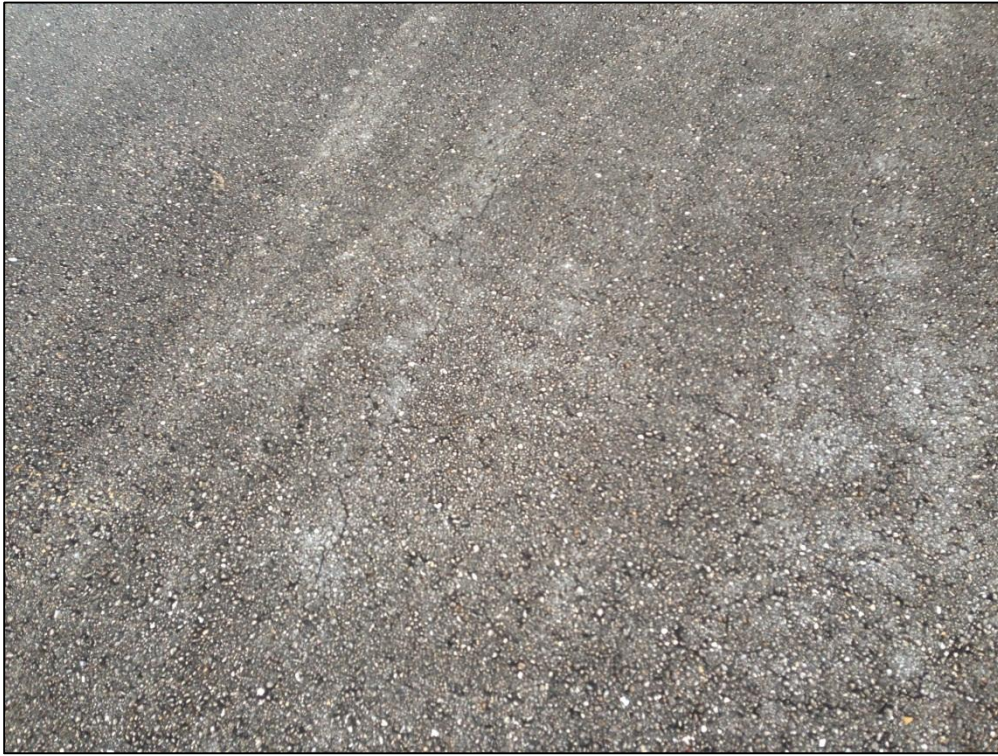
Taxiway Foxtrot 5, Section 630, Sample Unit 201 – Low Severity (52) Raveling, Low Severity (57) Weathering
