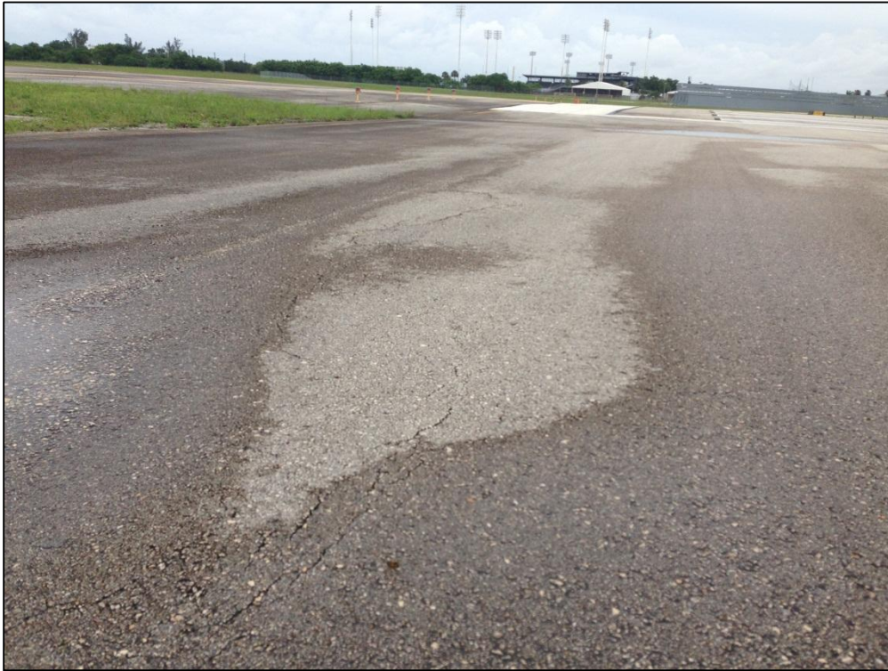
Taxiway South, Section 1905, Sample Unit 101 – Low Severity (48) Longitudinal and Transverse Cracking, Low Severity (52) Raveling, Low Severity (57) Weathering, Low Severity (56) Swelling
