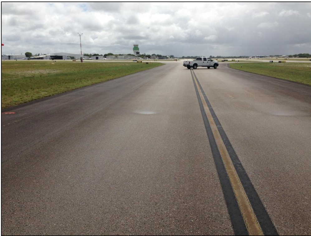
Taxiway East, Section 530, Sample Unit 149 – Low Severity (45) Depression, Low Severity (48) Longitudinal and Transverse Cracking, Low Severity (52) Raveling, Low Severity (57) Weathering
