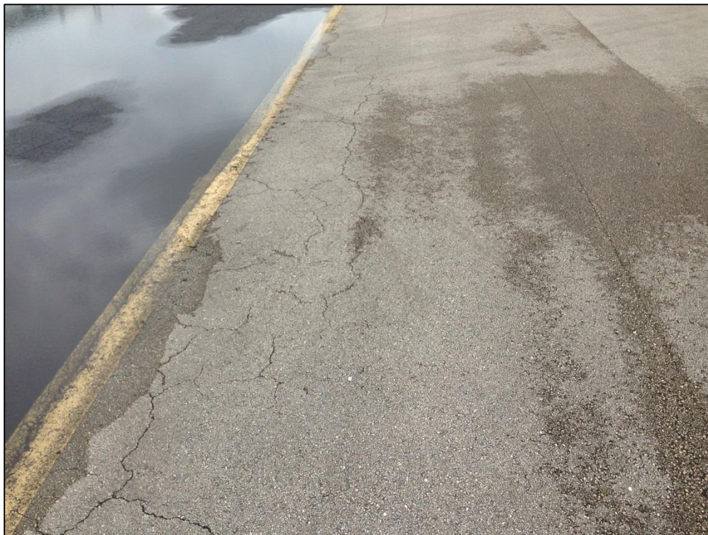
Apron South, Section 5905, Sample Unit 402 – Low Severity (43) Block Cracking, Low Severity (48) Longitudinal and Transverse Cracking, Low Severity (52) Raveling, Low Severity (57) Weathering
