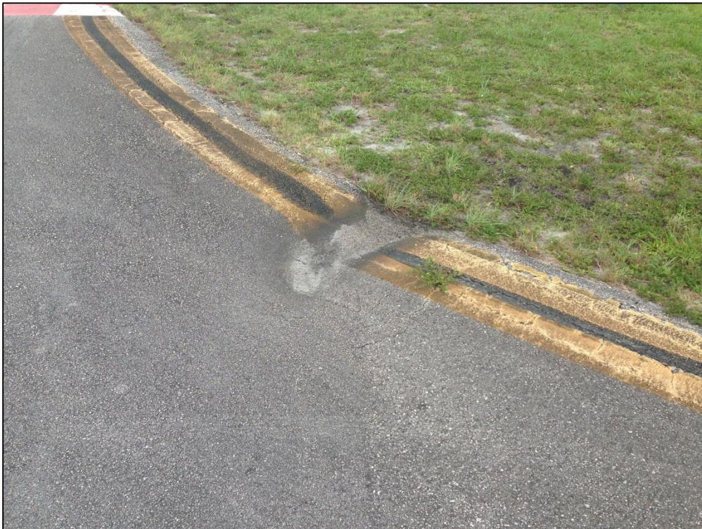
Taxiway South 1, Section 1950, Sample Unit 150 – High Severity (45) Depression, Low Severity (48) Longitudinal and Transverse Cracking, Low Severity (52) Raveling, Medium Severity (52) Raveling, Low Severity (57) Weathering, Medium Severity (57) Weathering
