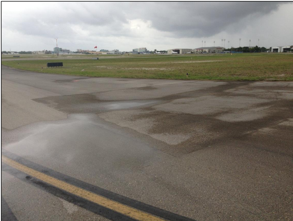
Taxiway North, Section 1425, Sample Unit 104 – Low Severity (45) Depression, Low Severity (50) Patching, Low Severity (57) Weathering
