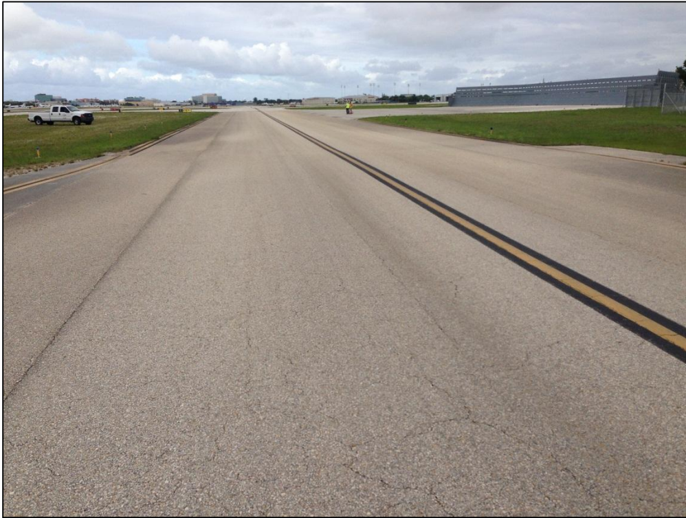
Taxiway East, Section 520, Sample Unit 123 – Low Severity (43) Block Cracking, Low Severity (52) Raveling, Low Severity (53) Rutting, Low Severity (57) Weathering
