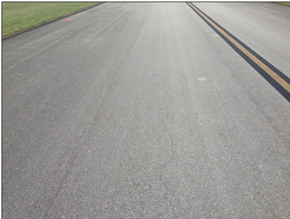
Taxiway Foxtrot, Section 605, Sample Unit 107 – Low Severity (48) Longitudinal and Transverse Cracking, Low Severity (52) Raveling, Low Severity (57) Weathering
