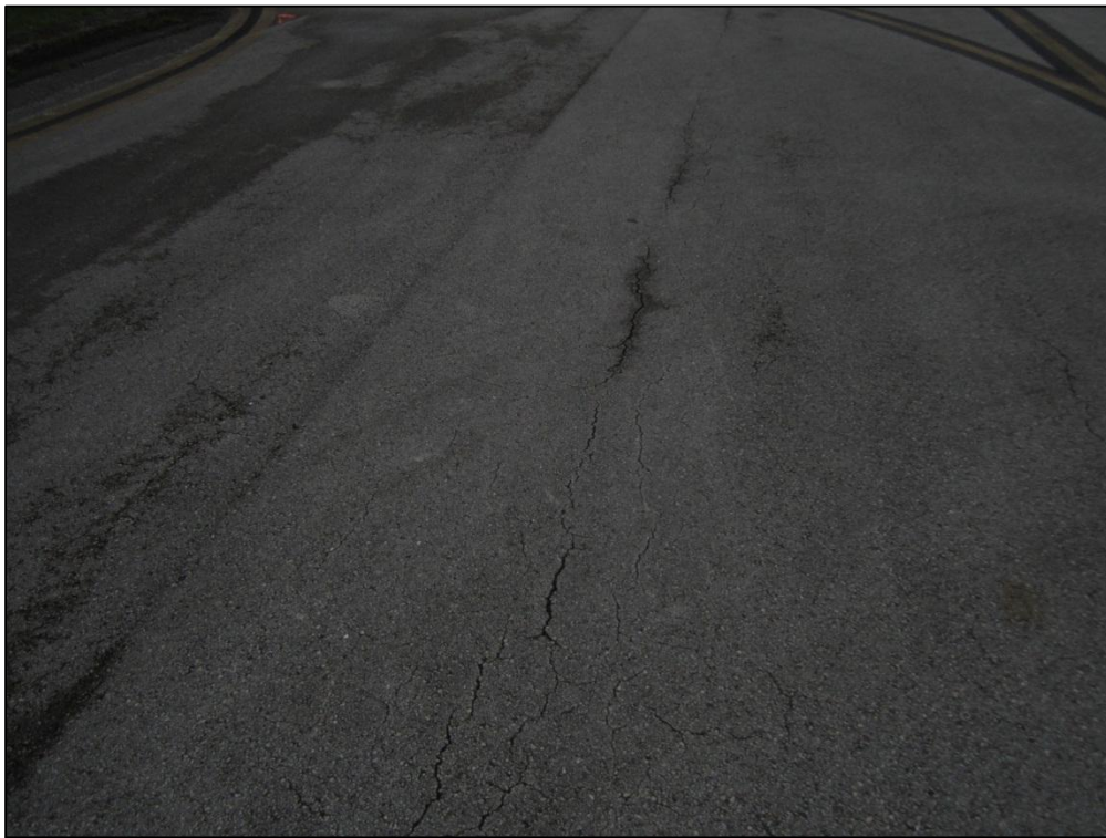
Taxiway Charlie, Section 305, Sample Unit 297 – Low and Medium Severity (48) Longitudinal and Transverse Cracking, Low Severity (52) Raveling, Low Severity (57) Weathering
