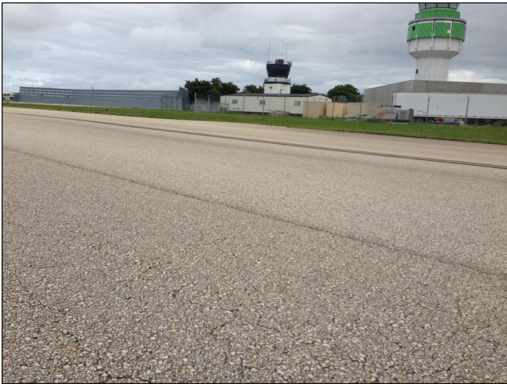
Taxiway East, Section 520, Sample Unit 123 – Low Severity (52) Raveling, Low Severity (57) Weathering, Low Severity (53) Rutting
