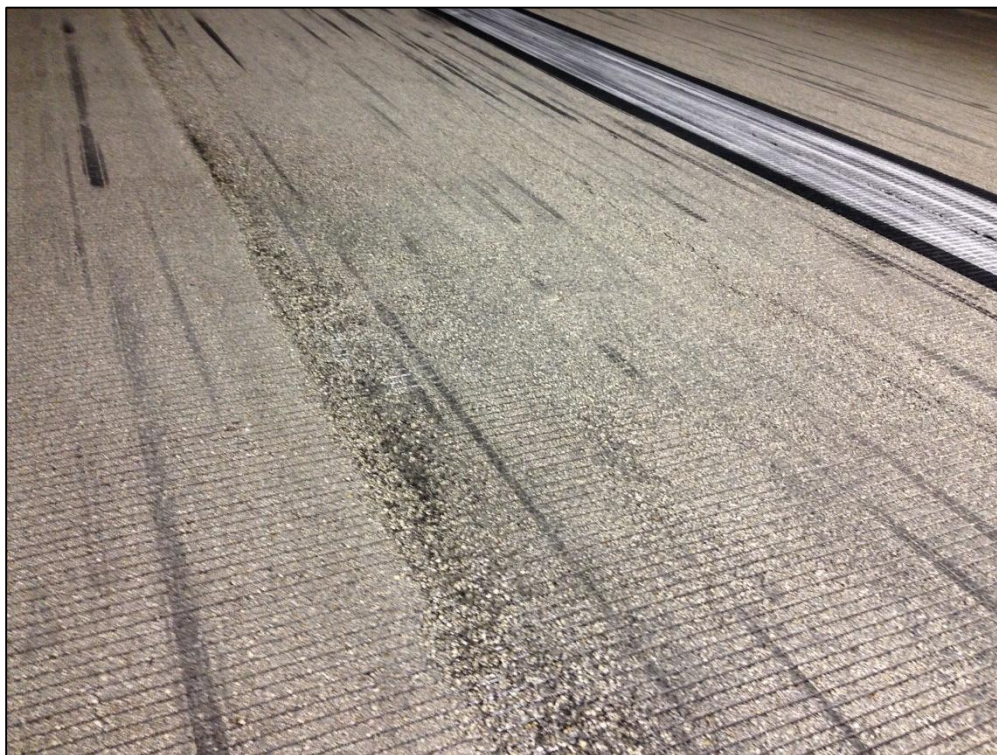
Runway 8-26, Section 6105, Sample Unit 347 – Low Severity (48) Longitudinal and Transverse Cracking, Low Severity (57) Weathering, Medium Severity (57) Weathering
