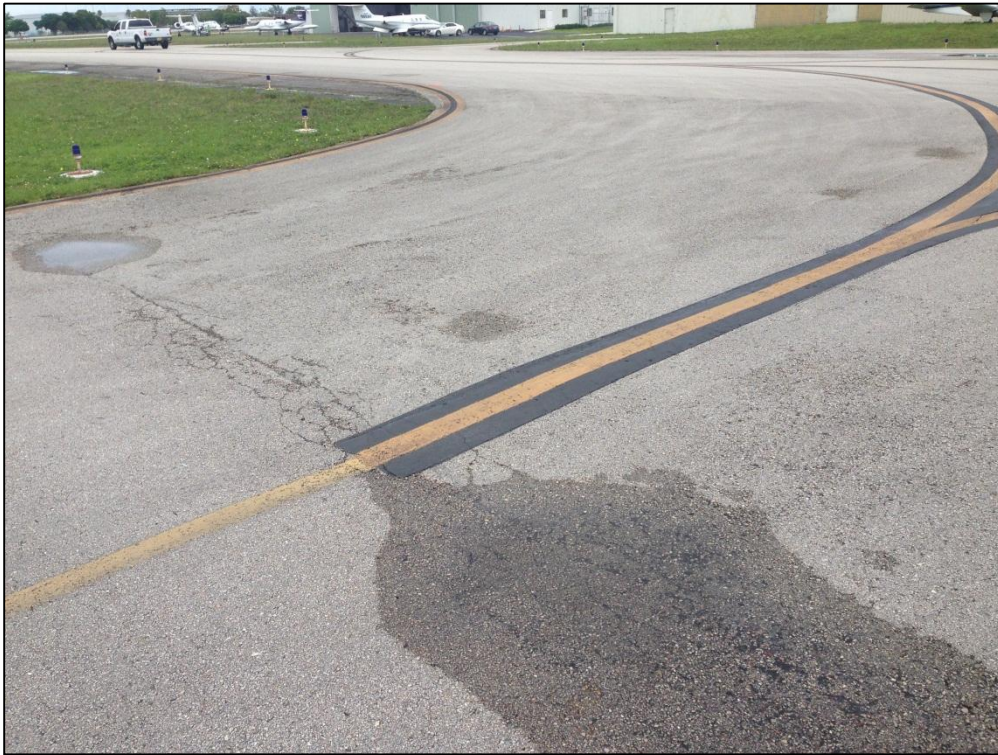
Taxiway Hangar 8, Section 395, Sample Unit 100 – Low Severity (45) Depression, Low Severity (48) Longitudinal and Transverse Cracking, Low Severity (52) Raveling, Low Severity (57) Weathering
