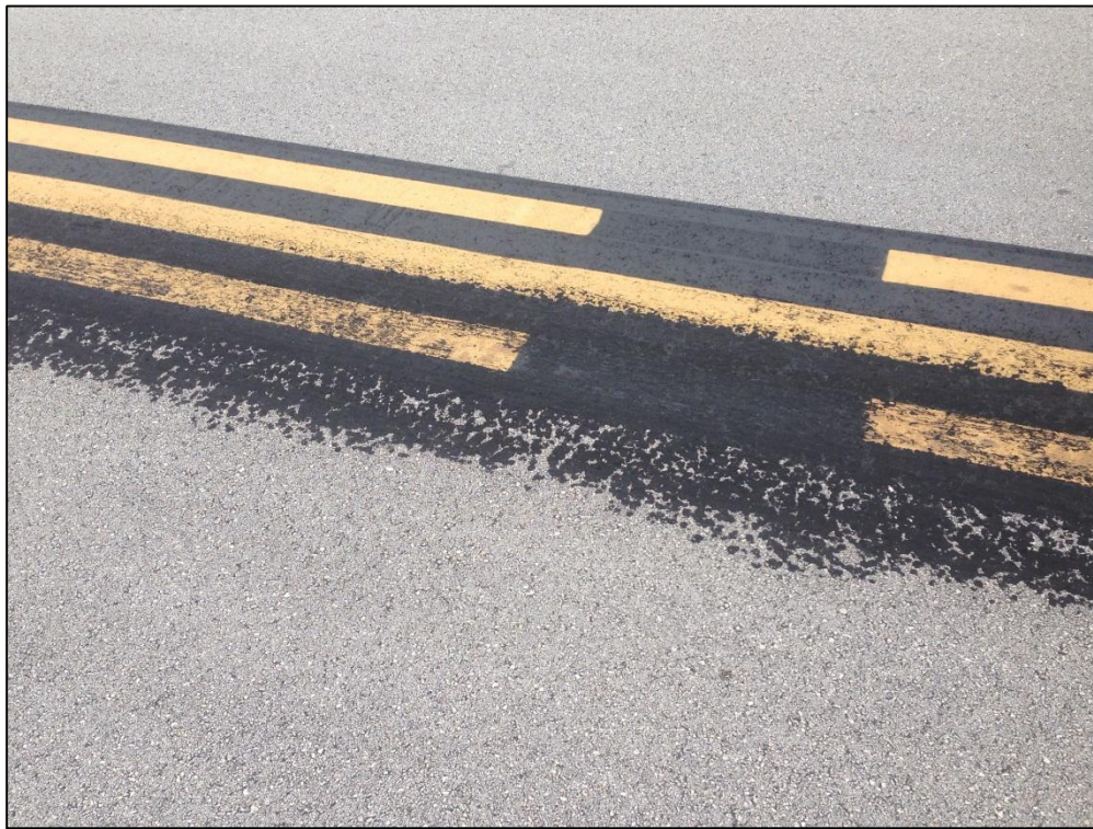
Taxiway Bravo, Section 212, Sample Unit 138 – (42) Bleeding, Low Severity (57) Weathering
