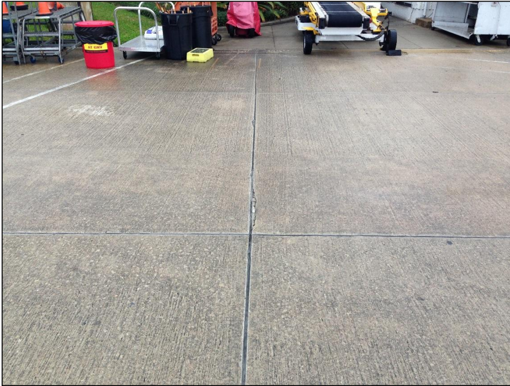
Apron South, Section 4115, Sample Unit 352 – Low Severity (70) Scaling, Map Cracking, Crazeing, Medium Severity (74) Joint Spalling
