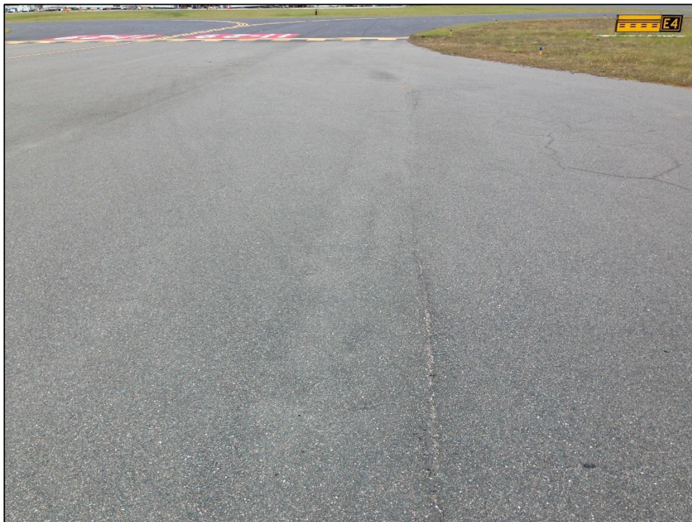
Taxiway E4, Section 540, Sample Unit 401 – Low Severity (48) Longitudinal and Transverse Cracking, Low Severity (57) Weathering
