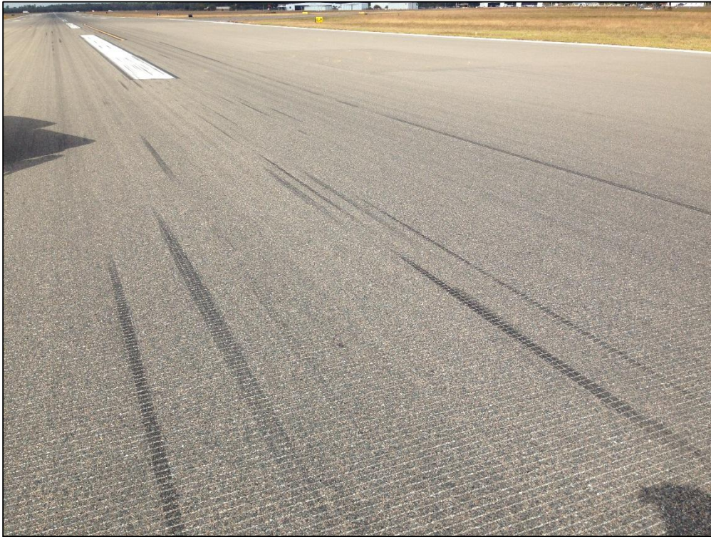
Runway 11-29, Section 6205, Sample Unit 365 – Low Severity (52) Raveling, Low Severity (57) Weathering
