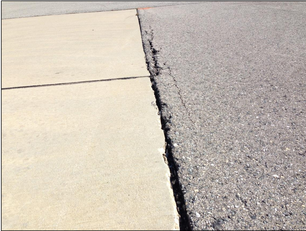
Apron SW, Section 4325, Sample Unit 204 – Low Severity (48) Longitudinal and Transverse Cracking, Low Severity (54) Shoving, Medium Severity (57) Weathering
