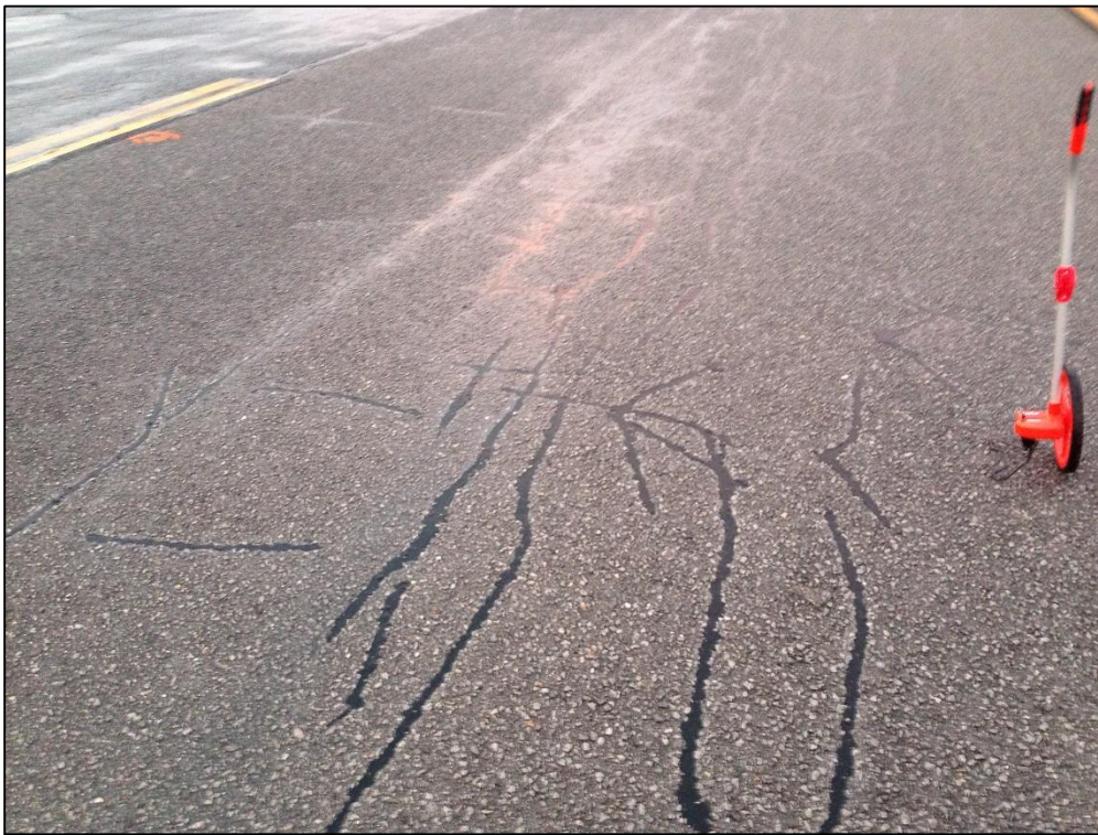
Taxiway Alpha, Section 105, Sample Unit 109 – Low Severity (48) Longitudinal and Transverse Cracking, Low Severity (43) Block Cracking, Medium Severity (52) Raveling
