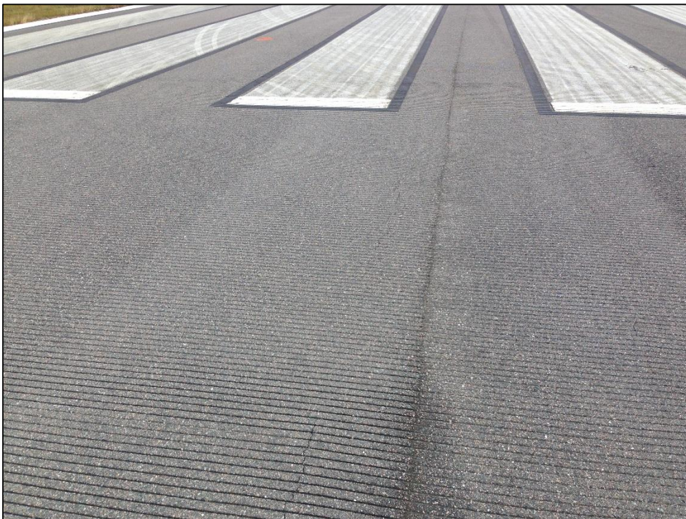
Runway 11-29, Section 6202, Sample Unit 300 – Low Severity (48) Longitudinal and Transverse Cracking, Medium Severity (52) Raveling, Low Severity (56) Swelling
