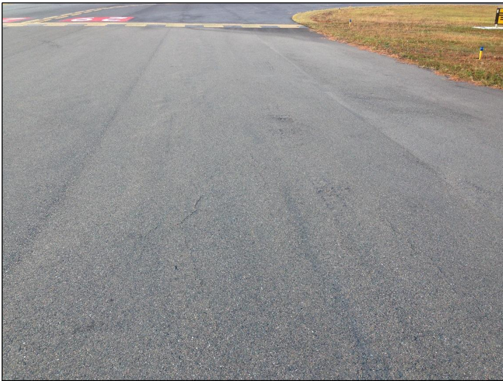
Taxiway E1, Section 515, Sample Unit 102 – Low Severity (48) Longitudinal and Transverse Cracking, Low Severity (57) Weathering
