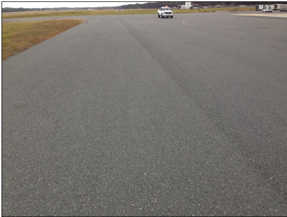
Apron 4105, Section 4105, Sample Unit 105 – Low Severity (57) Weathering
