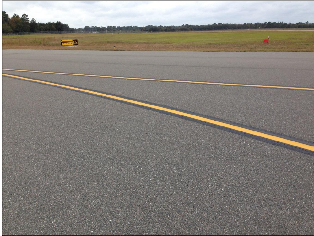
Taxiway E5, Section 550, Sample Unit 501 – Low Severity (48) Longitudinal and Transverse Cracking, Low Severity (57) Weathering
