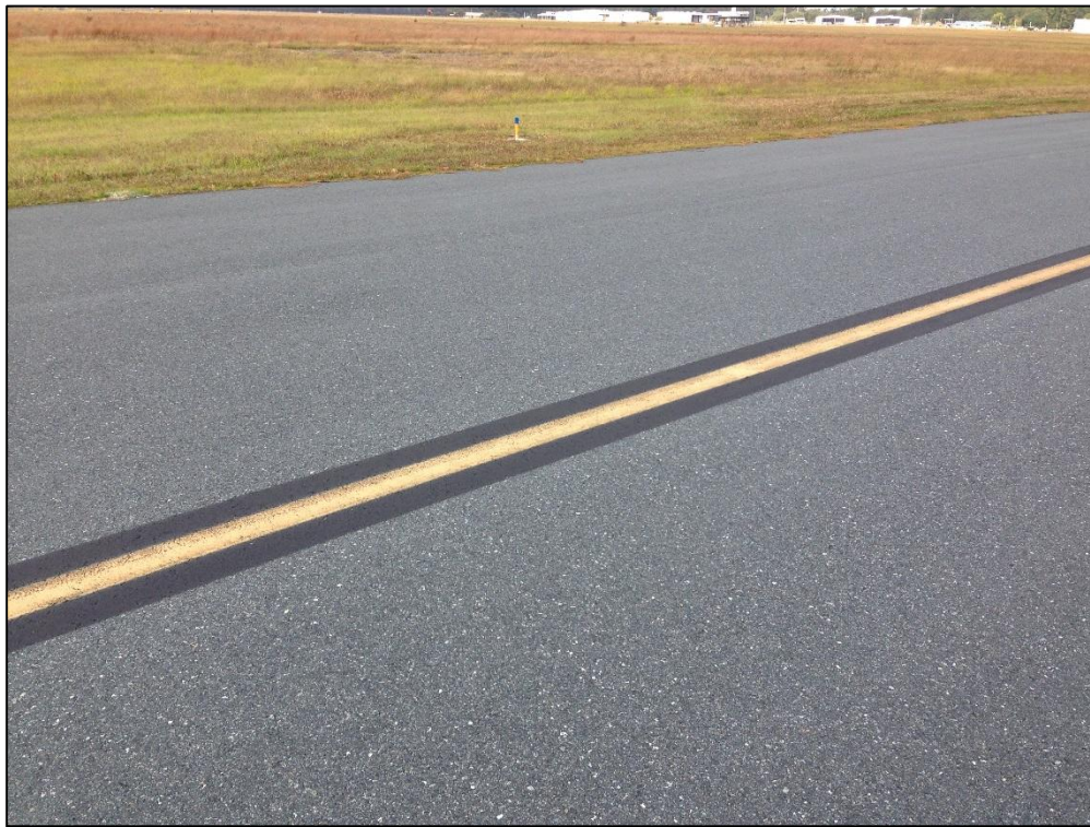
Taxiway Bravo, Section 210, Sample Unit 206 – Low Severity (57) Weathering
