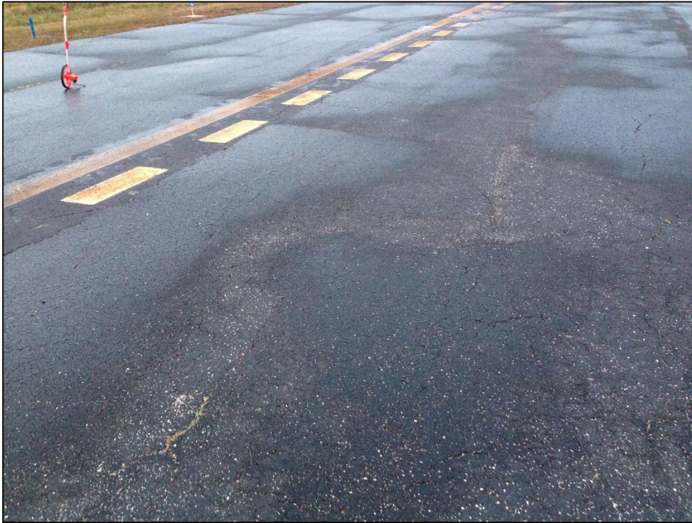
Apron Run-Up RW 7, Section 5205, Sample Unit 100 – Low Severity (43) Block Cracking, Low Severity (52) Raveling
