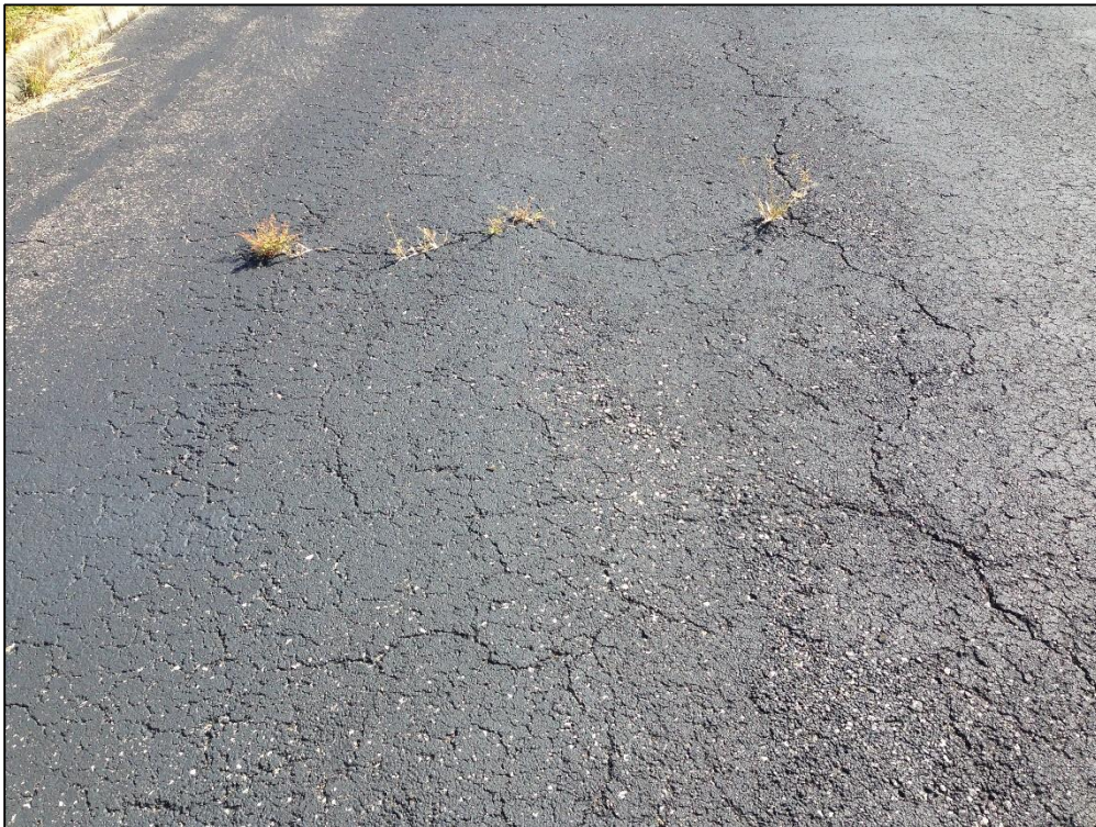
Apron SW, Section 4310, Sample Unit 102 – Low Severity (43) Block Cracking, Medium Severity (52) Raveling
