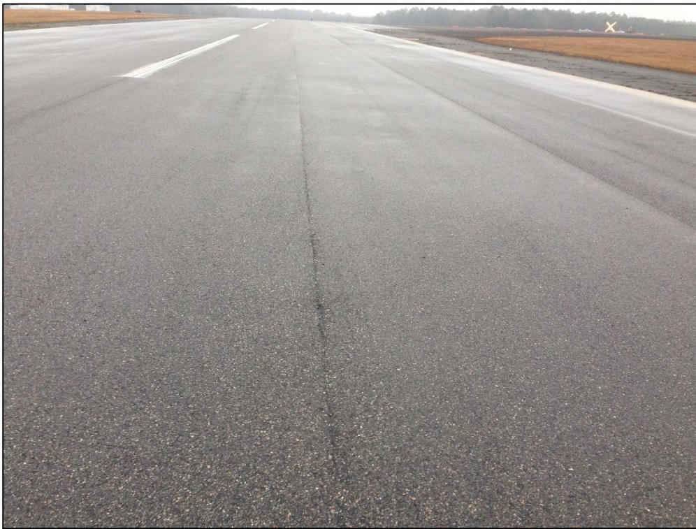
Runway 7-25, Section 6110, Sample Unit 133 – Low Severity (57) Weathering
