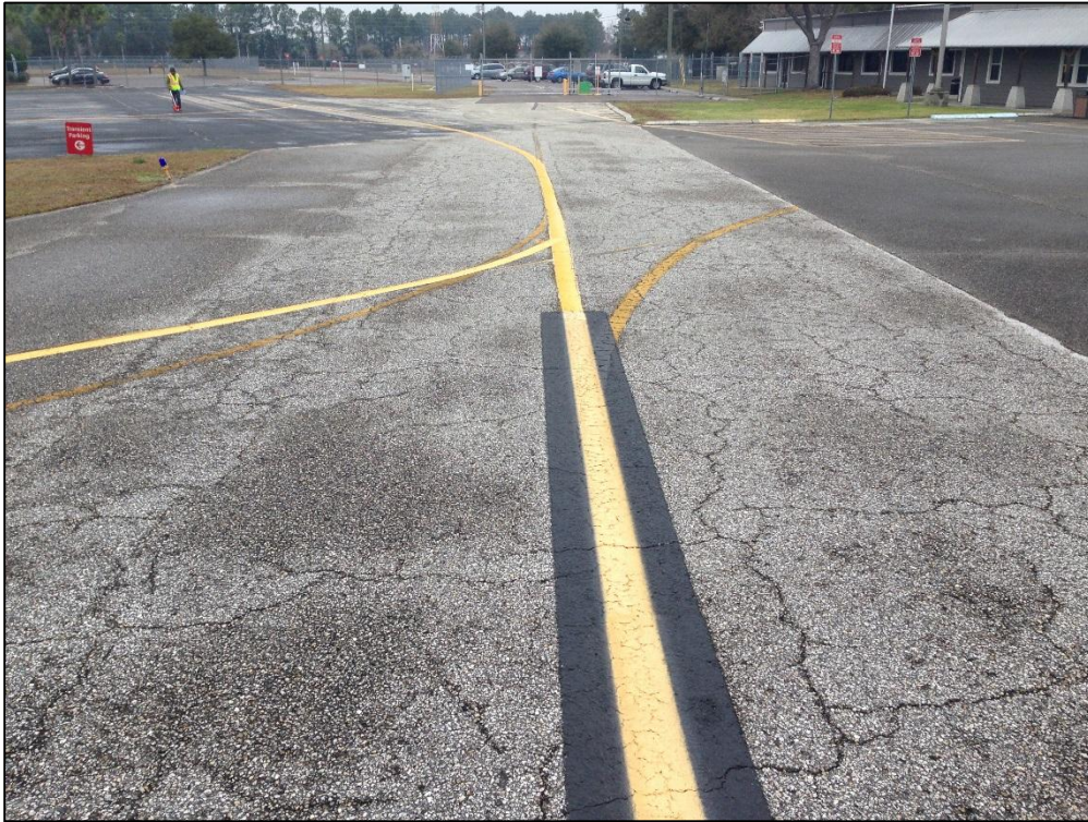
Taxiway East Connector to NW Apron, Section 405, Sample Unit 100 – Low Severity (43) Block Cracking, Low Severity (52) Raveling, Medium Severity (52) Raveling
