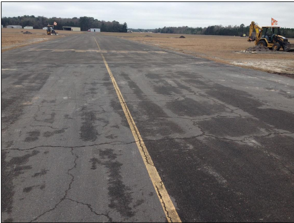
Taxiway Connector to Runway, Section 620, Sample Unit 100 – Low Severity (43) Block Cracking, Low Severity (52) Raveling
