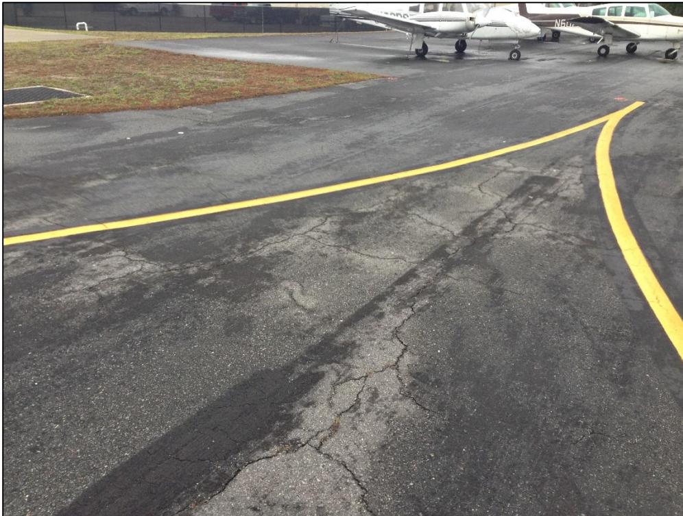
Taxiway T-Hangar, Section 905, Sample Unit 100 – Low Severity (43) Block Cracking, Low Severity (52) Raveling
