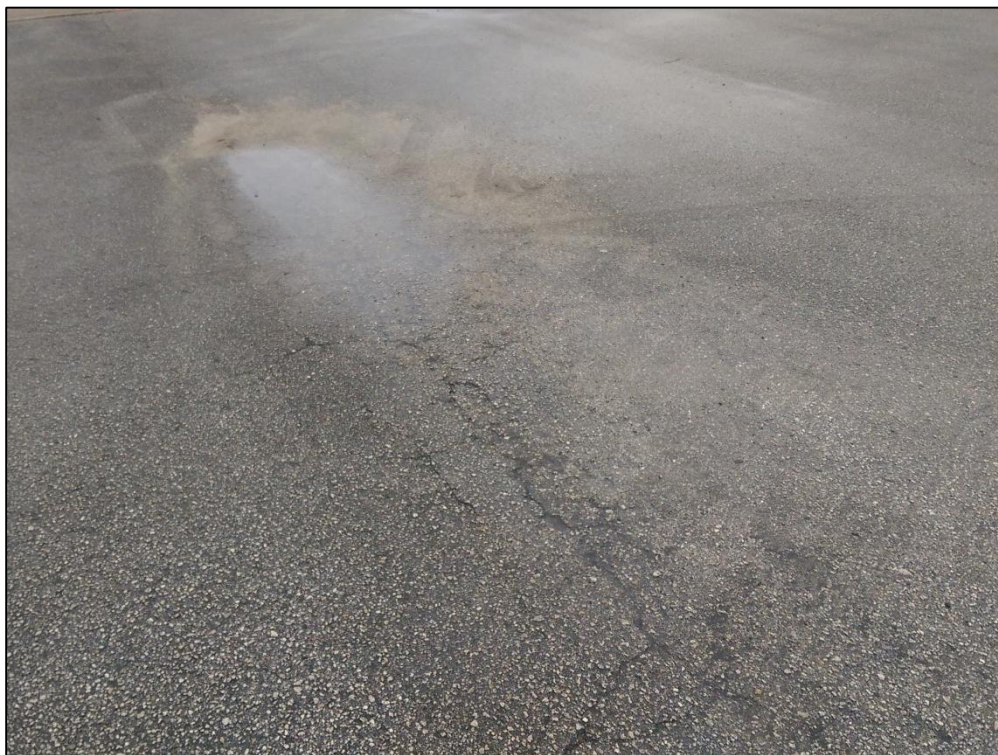
Apron Northeast, Section 4405, Sample Unit 401 – Low Severity (41) Alligator Cracking, Low Severity (53) Rutting, Low Severity (52) Raveling
