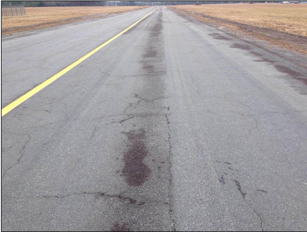
Taxiway Delta, Section 205, Sample Unit 120 – Low Severity (43) Block Cracking, Low Severity (48) Longitudinal and Transverse Cracking, Low Severity (52) Raveling
