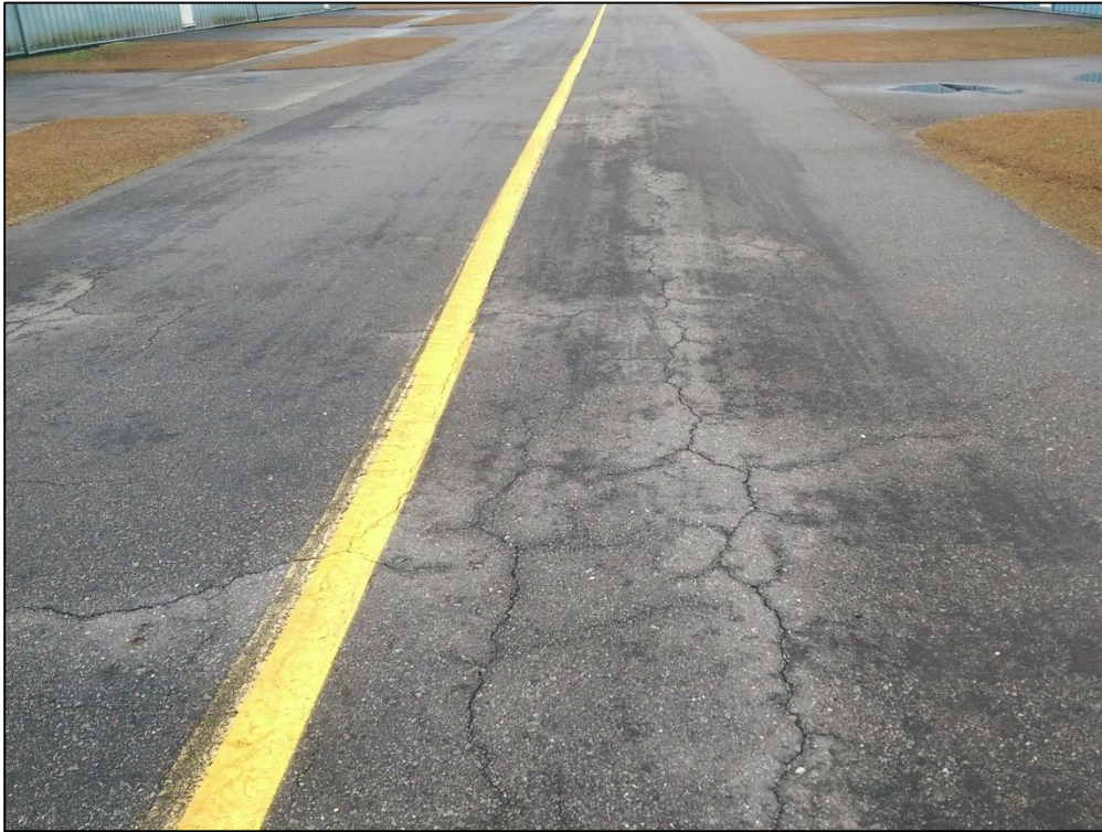
Taxiway T-Hangar, Section 915, Sample Unit 300 – Low Severity (43) Block Cracking, Low Severity (48) Longitudinal and Transverse Cracking, Low Severity (52) Raveling, Low Severity (57) Weathering
