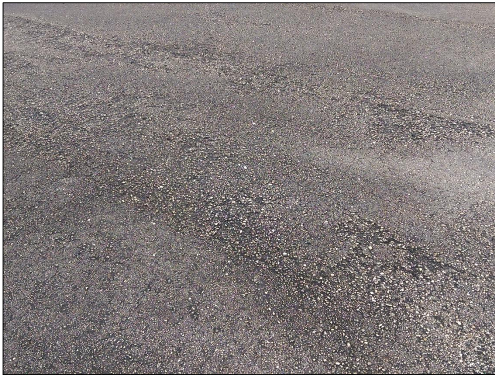
Apron Run-Up, Section 5105, Sample Unit 100 – Low Severity (48) Longitudinal and Transverse Cracking, Low Severity (52) Raveling, Medium Severity (52) Raveling
