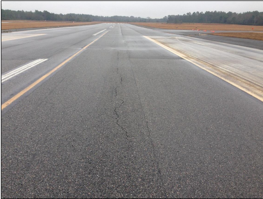
Runway 7-25, Section 6105, Sample Unit 157 – Low Severity (48) Longitudinal and Transverse Cracking, Low Severity (57) Weathering
