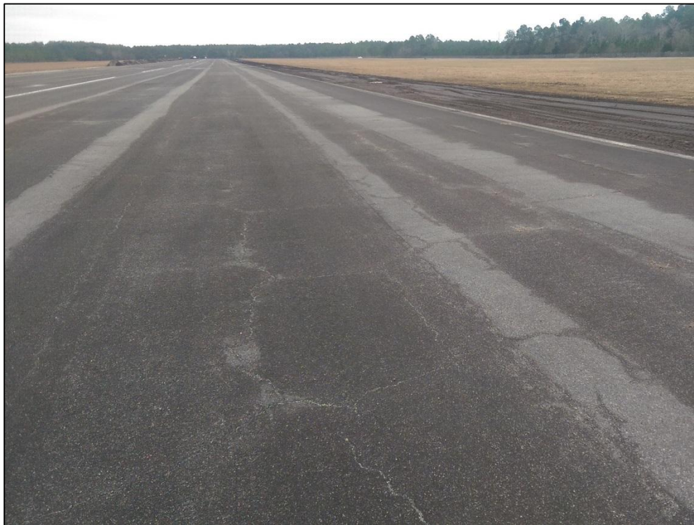
Runway 11-29, Section 6205, Sample Unit 149 – Low Severity (41) Alligator Cracking
