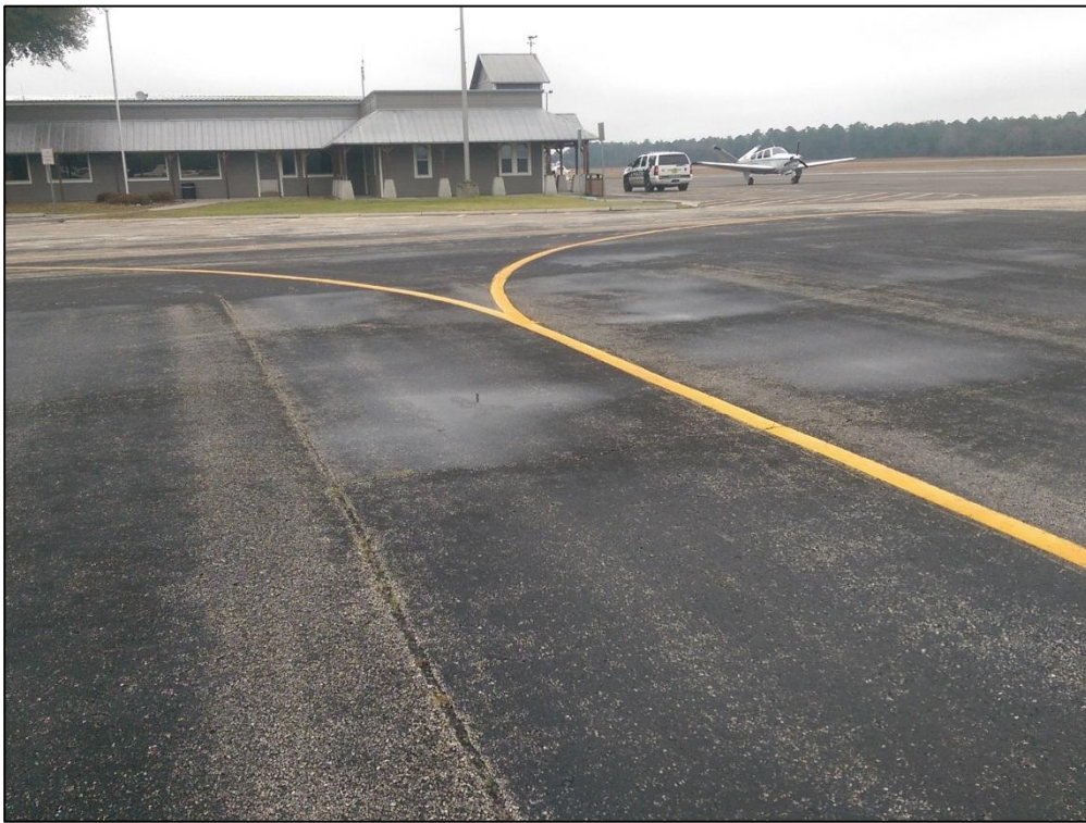
Apron Northwest, Section 4105, Sample Unit 254 – Low and Medium Severity (48) Longitudinal and Transverse Cracking, Low Severity (52) Raveling
