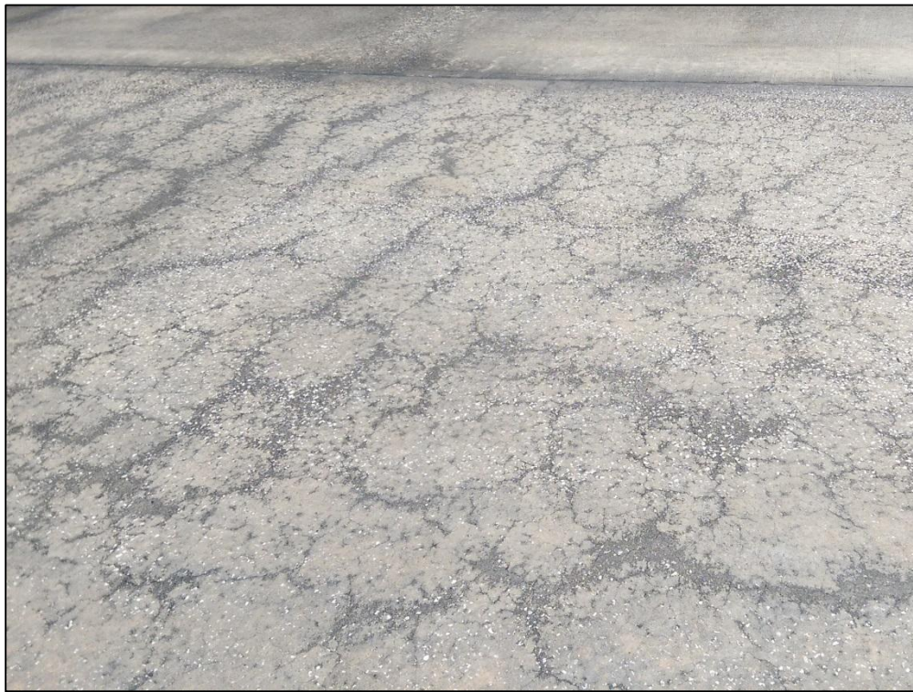
Taxiway Golf, Section 1020, Sample Unit 100 – Medium Severity (70) Scaling, Map Cracking, Crazing
