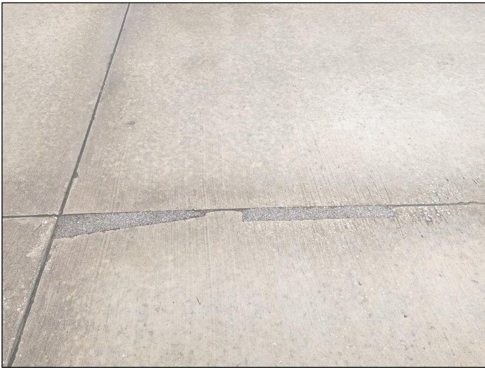
Terminal Apron, Section 4310, Sample Unit 102 – Low Severity (66) Small Patching, Low Severity (70) Scaling, Map Cracking, Cracking
