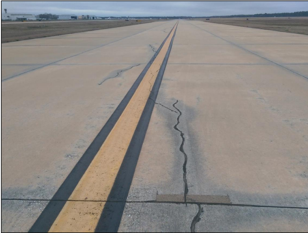
Taxiway Alpha, Section 125, Sample Unit 149 – Low Severity (63) Longitudinal, Transverse, and Diagonal Cracking, Low Severity (66) Small Patching
