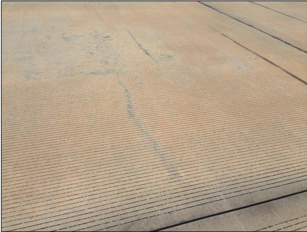
Runway 8-26, Section 6105, Sample Unit 369 - (73) Shrinkage Cracks
