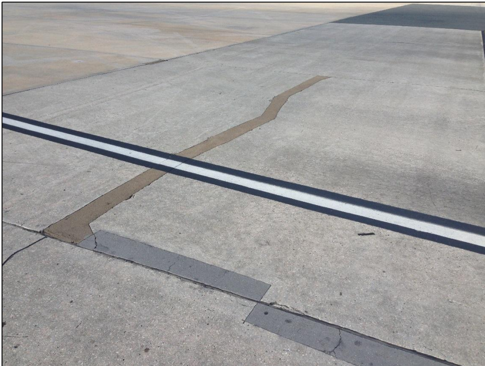
Terminal Apron, Section 4430, Sample Unit 405 – Low Severity (66) Small Patching, Low Severity (67) Large Patching, Low Severity (74) Joint Spalling
