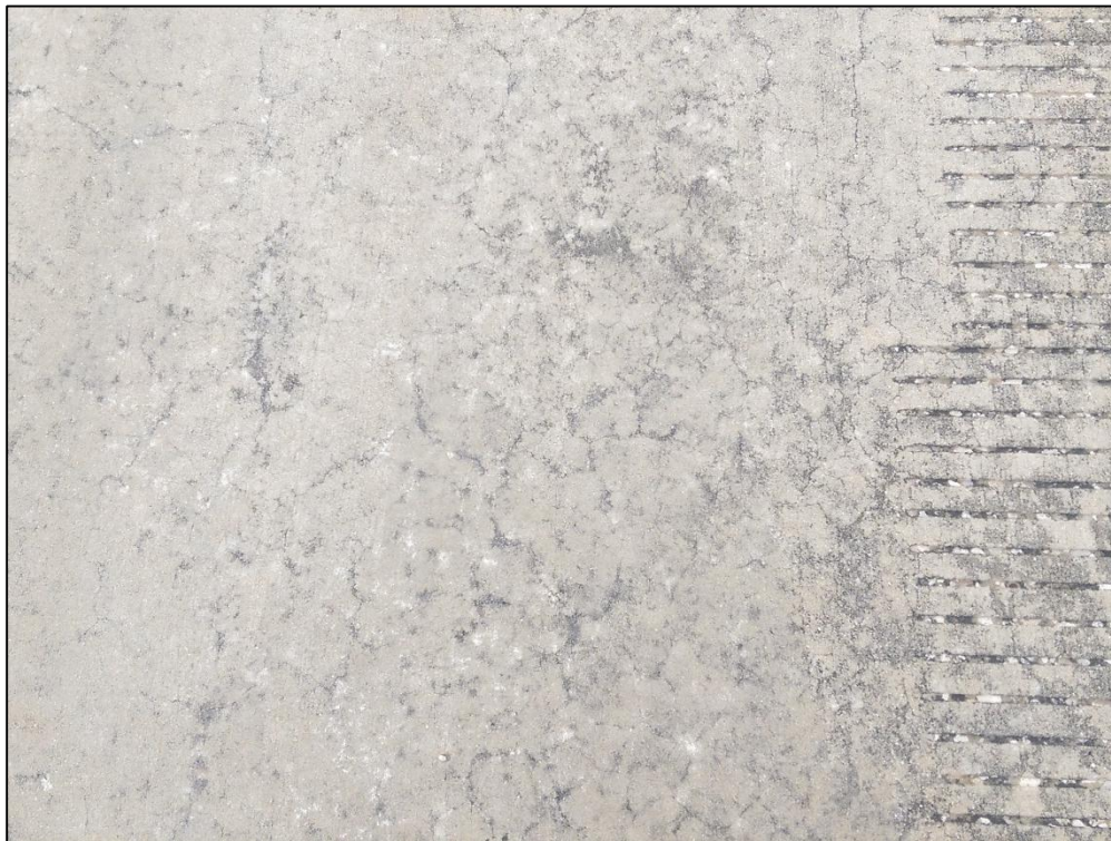
Runway 14-32, Section 6215, Sample Unit 113 – Low Severity (70) Scaling, Map Cracking, Crazing
