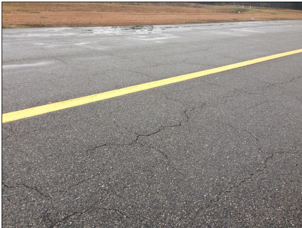
Taxiway Foxtrot, Section 1155, Sample Unit 106 – Low Severity (43) Block Cracking, Low Severity (52) Raveling
