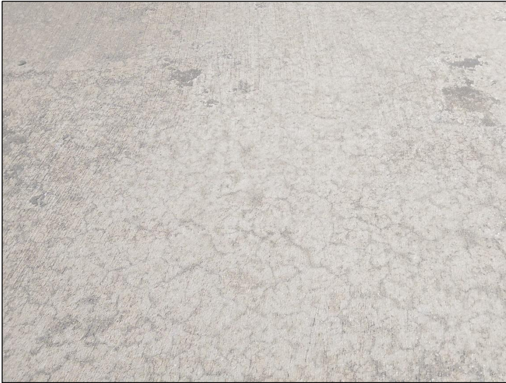
Terminal Apron, Section 4445, Sample Unit 804 – Low Severity (70) Scaling, Map Cracking, Crazing
