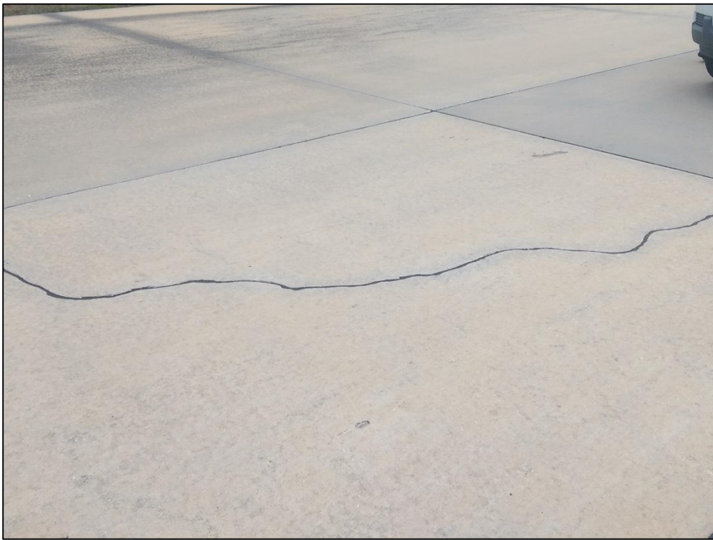
Taxiway Hotel, Section 555, Sample Unit 101 – Low Severity (63) Longitudinal, Transverse, and Diagonal Cracking
