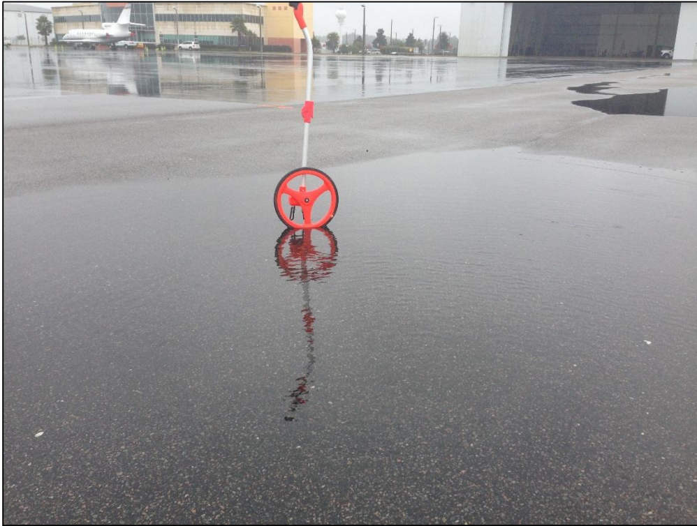
Apron GA, Section 5105, Sample Unit 89 – Medium Severity (45) Depression, Low Severity (52) Raveling
