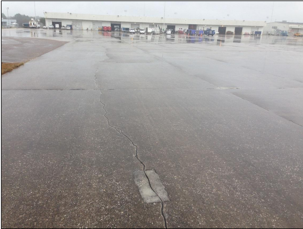
Apron Cargo, Section 4120, Sample Unit 405 – Low Severity (63) Longitudinal, Transverse, and Diagonal Cracking, Low Severity (66) Small Patching
