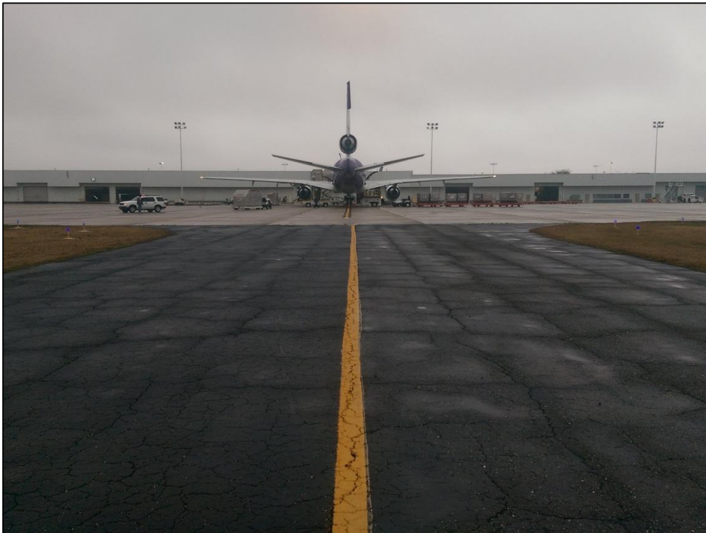
Taxiways within Apron, Section 2720, Sample Unit 101 – Medium Severity (43) Block Cracking, Medium Severity (57) Weathering
