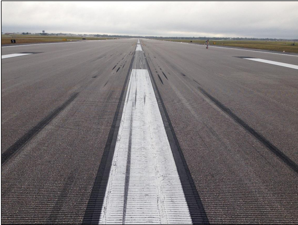
Runway 9-27, Section 6115, Sample Unit 360 – Low Severity (48) Longitudinal and Transverse Cracking, Low Severity (52) Raveling, Low Severity (57) Weathering
