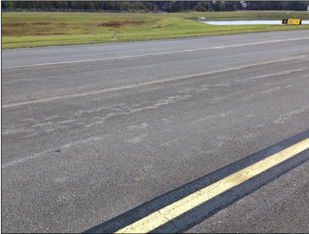
Taxiway Alpha, Section 105, Sample Unit 121 – Low Severity (48) Longitudinal and Transverse Cracking, Low Severity (52) Raveling, Low Severity (56) Swelling, Low Severity (57) Weathering
