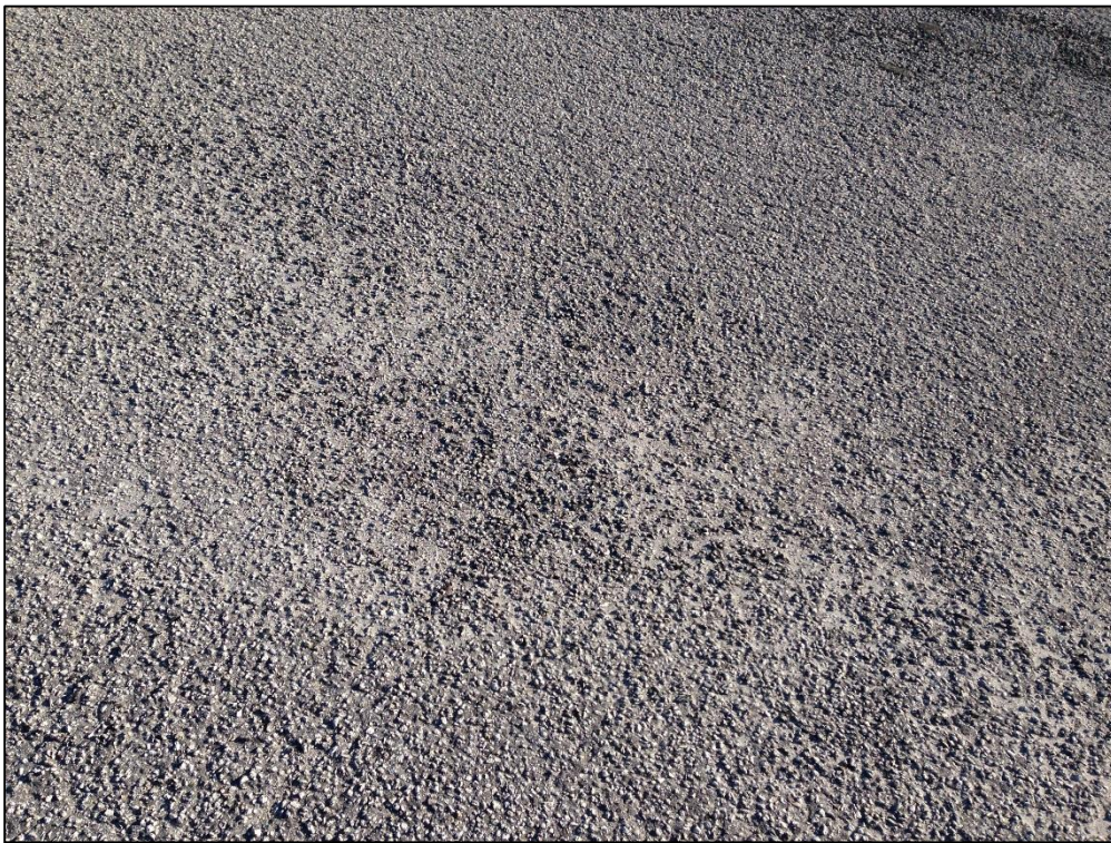
Apron North, Section 4125, Sample Unit 103 – High Severity (52) Raveling
