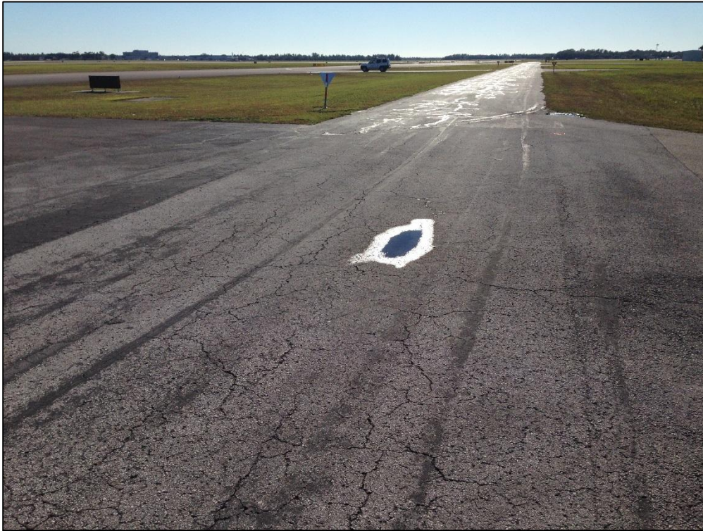
Apron NE, Section 4215, Sample Unit 200 – Low Severity (43) Block Cracking, Low Severity (52) Raveling, Medium Severity (53) Rutting, Low Severity (57) Weathering
