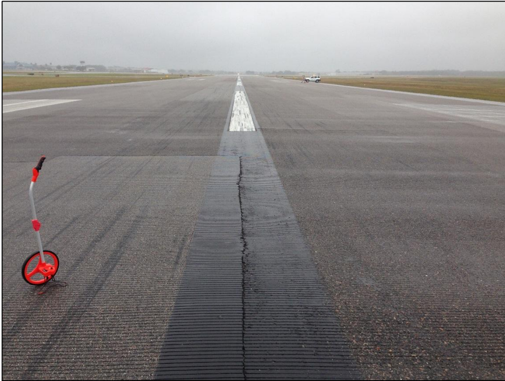
Runway 5-23, Section 6215, Sample Unit 322 – Low and Medium Severity (48) Longitudinal and Transverse Cracking, Low Severity (52) Raveling, Medium Severity (57) Weathering
