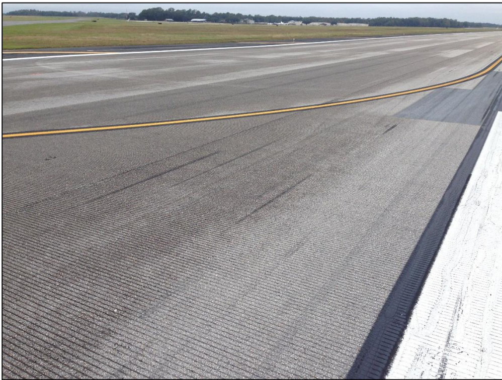
Runway 9-27, Section 6150, Sample Unit 414 – Low Severity (48) Longitudinal and Transverse Cracking, Low Severity (52) Raveling, Low Severity (57) Weathering
