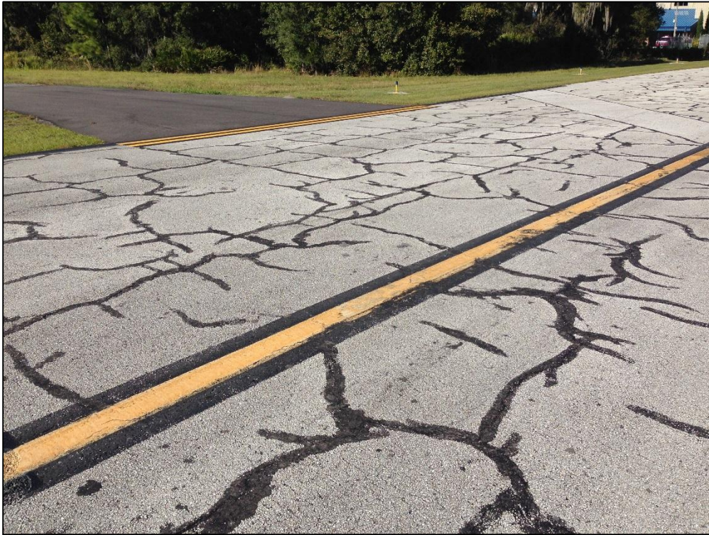
Taxiway Hotel, Section 805, Sample Unit 122 – Low Severity (43) Block Cracking, Low Severity (50) Patching, Low Severity (52) Raveling
