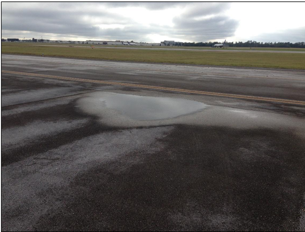
Taxiway Delta, Section 415, Sample Unit 200 – High Severity (45) Depression, Low Severity (48) Longitudinal and Transverse Cracking, Low Severity (52) Raveling, High Severity (52) Raveling
