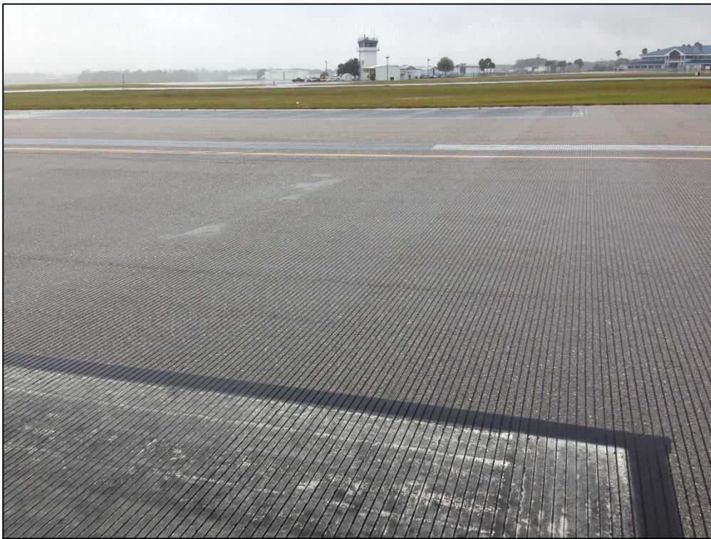
Runway 5-23, Section 6245, Sample Unit 379 – Low Severity (48) Longitudinal and Transverse Cracking, Medium Severity (57) Weathering
