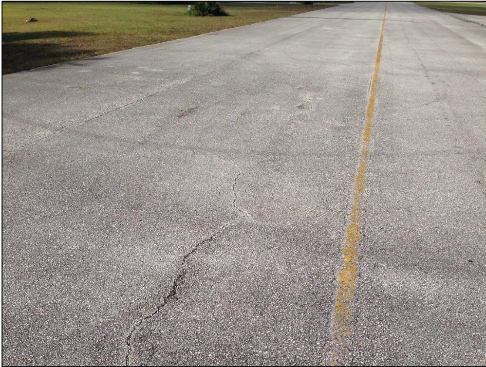
Taxiway Sierra, Section 905, Sample Unit 901 – Low Severity (48) Longitudinal and Transverse Cracking, Low Severity (52) Raveling, Medium Severity (52) Raveling
