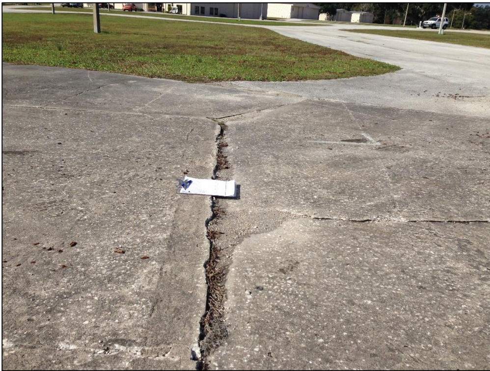
Taxiway Sierra, Section 922, Sample Unit 601 – Medium Severity (63) Longitudinal, Transverse, and Diagonal Cracking, High Severity (71) Faulting, Medium Severity (75) Corner Spalling
