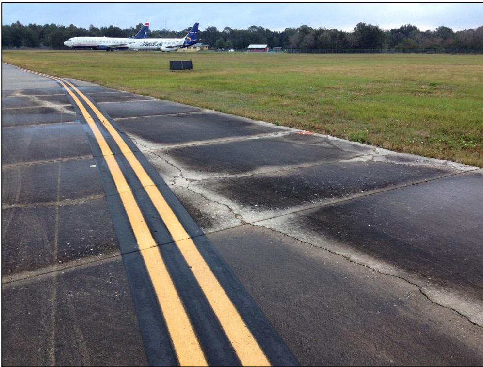
Taxiway Echo, Section 520, Sample Unit 125 – Medium Severity (63) Longitudinal, Transverse, and Diagonal Cracking, High Severity (65) Joint Seal Damage, High Severity (72) Shattered Slab
